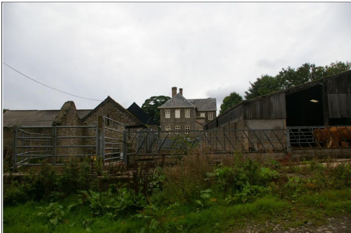
2. GREAT POTHRIDGE HOUSE, VIEWED FROM WITHIN THE FARMYARD WHICH WILL BE THE SUBJECT OF THE PROPOSALS; FROM THE EAST.
