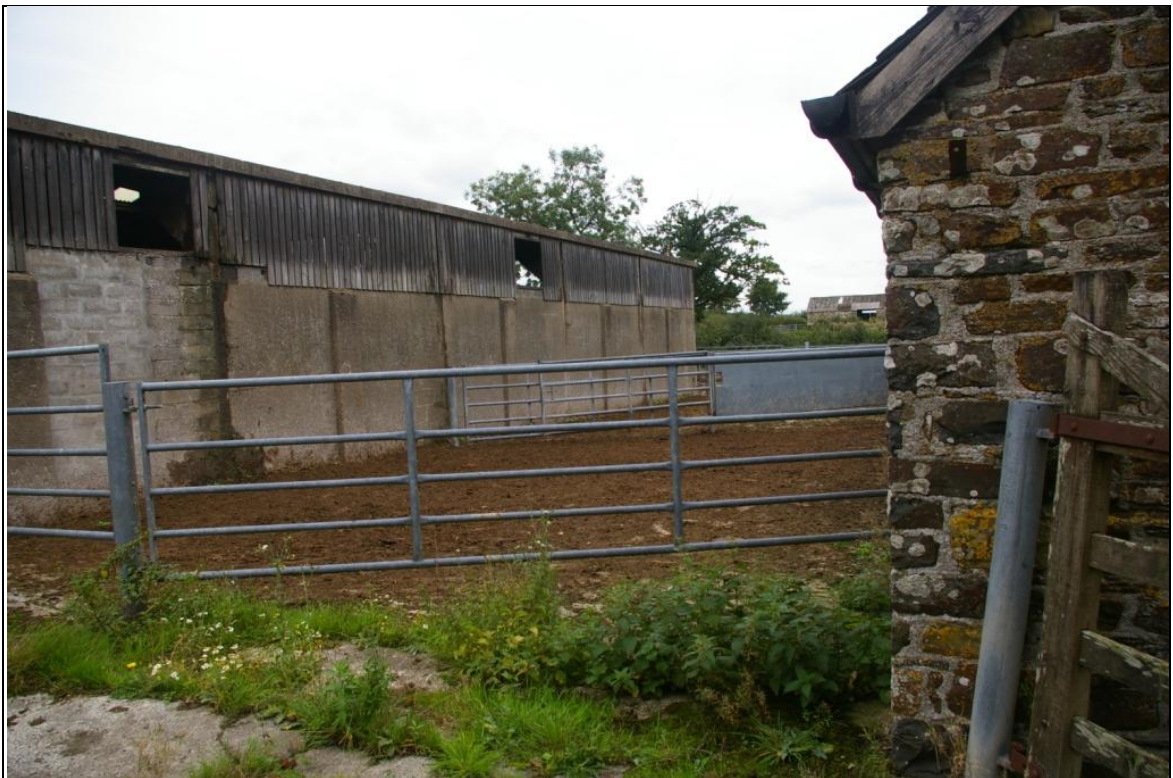
18. PART OF PROPOSAL AREA BETWEEN THE EXTANT MODERN BUILDING AND THE NORTH ELEVATION OF THE LOW 19 TH CENTURY NORTH RANGE; FROM THE SOUTH-WEST.
