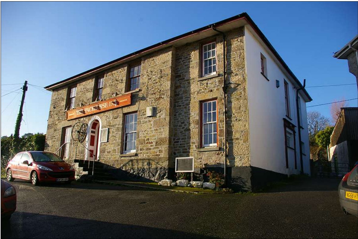
PHOTO 1: VIEW OF THE NORTH AND EAST ELEVATIONS OF THE PACKHORSE INN; FACING SOUTH-WEST.
