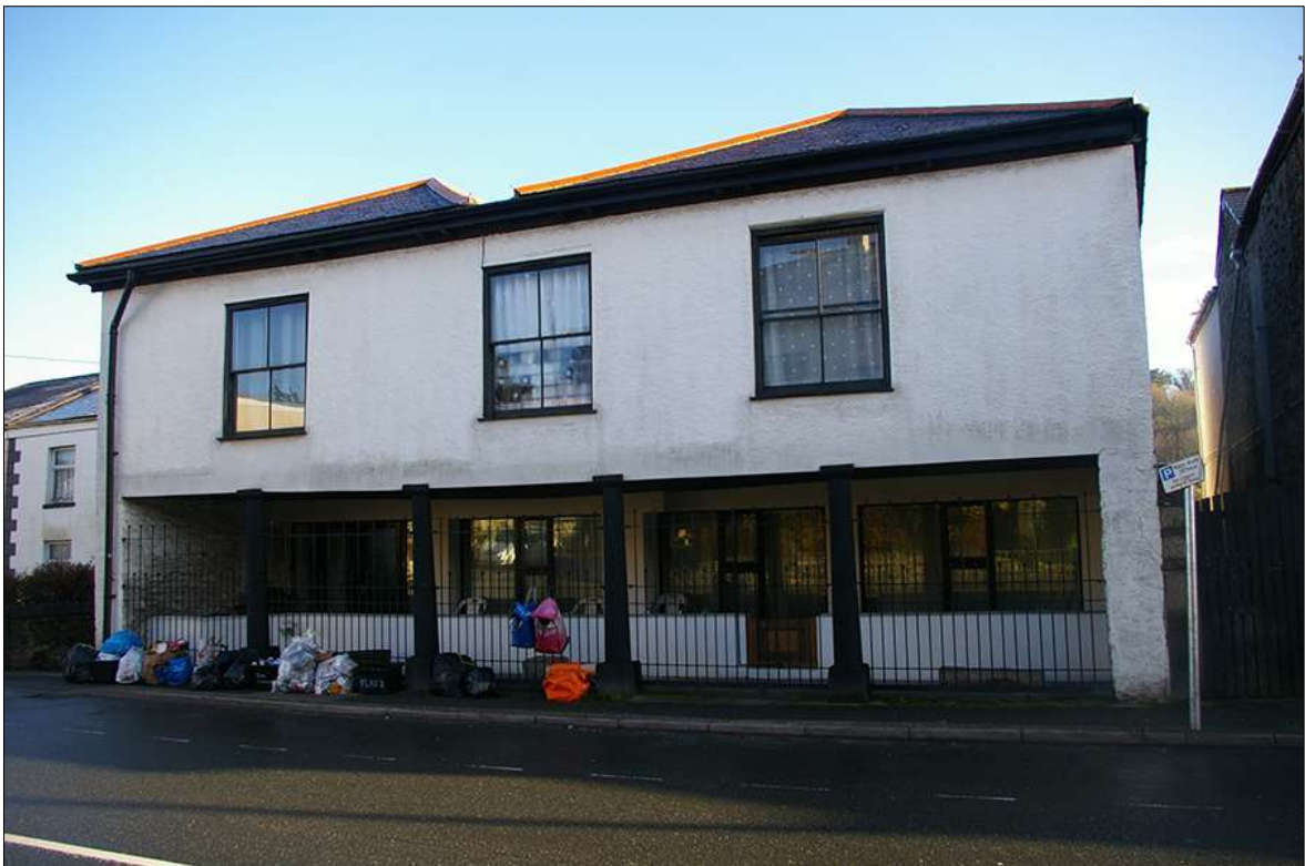
PHOTO 18: THE FORMER MARKET HOUSE SHOWING THE OPEN FRONTING AND JETTIED 1 ST FLOOR; FACING NORTH-EAST.
