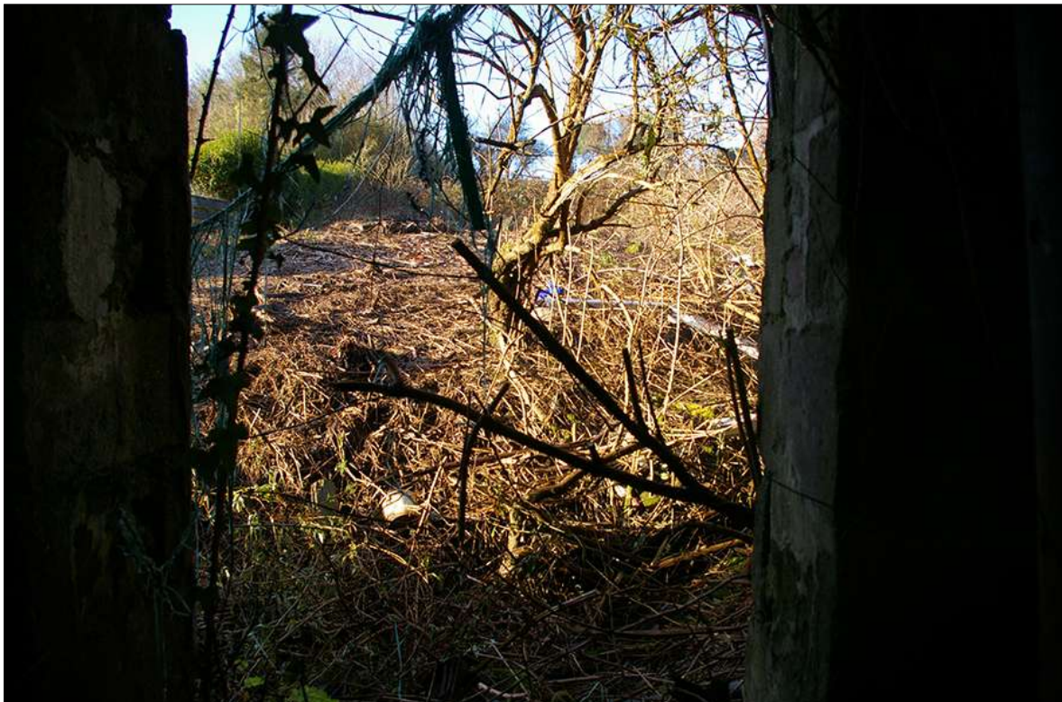
FIGURE 9: VIEW ACROSS FIELD 1 FROM THE INTERIOR OF THE DERELICT OUTBUILDING; FACING WEST.
