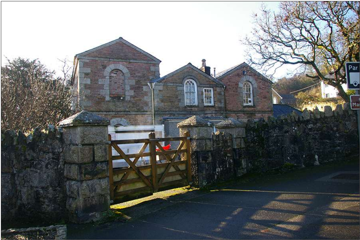
PHOTO 13: THE VICARAGE, LOCATED TO THE SOUTH OF THE CHURCH; FACING WEST.
