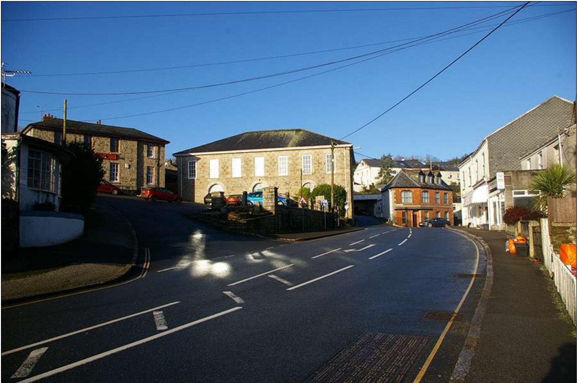
PHOTO 4: VIEW OF THE PACKHORSE INN AND FORMER TOWN HALL/RAINBOW ROOMS WITHIN THE WIDER SETTING OF THE TOWN SQUARE; FACING NORTH-WEST.
