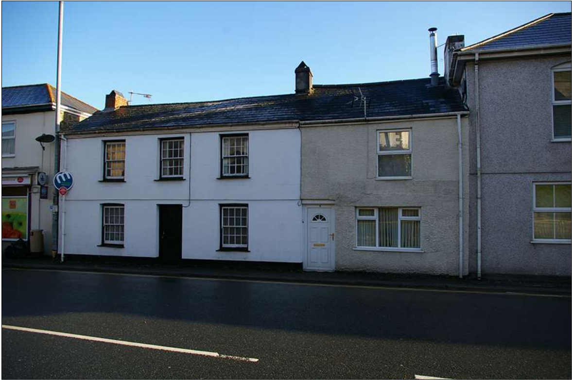
PHOTO 17: NUMBERS 8-10 FORE STREET, SHOWING THE GOOD FACADE OF NUMBER 10, AND THE SHELL STUDDED STUCCO OF NUMBER 8; FACING EAST.
