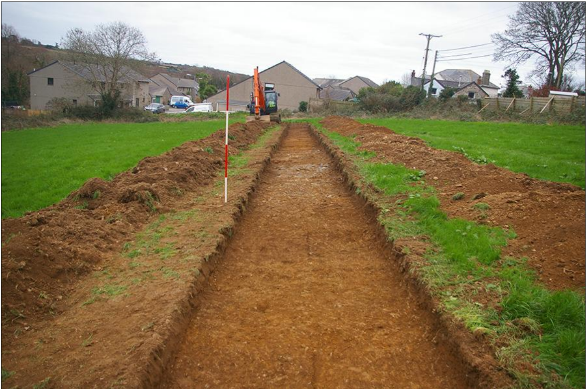
67. TRENCH 05, POST-EXCAVATION; VIEWED FROM THE NORTH-WEST (2M SCALE).
