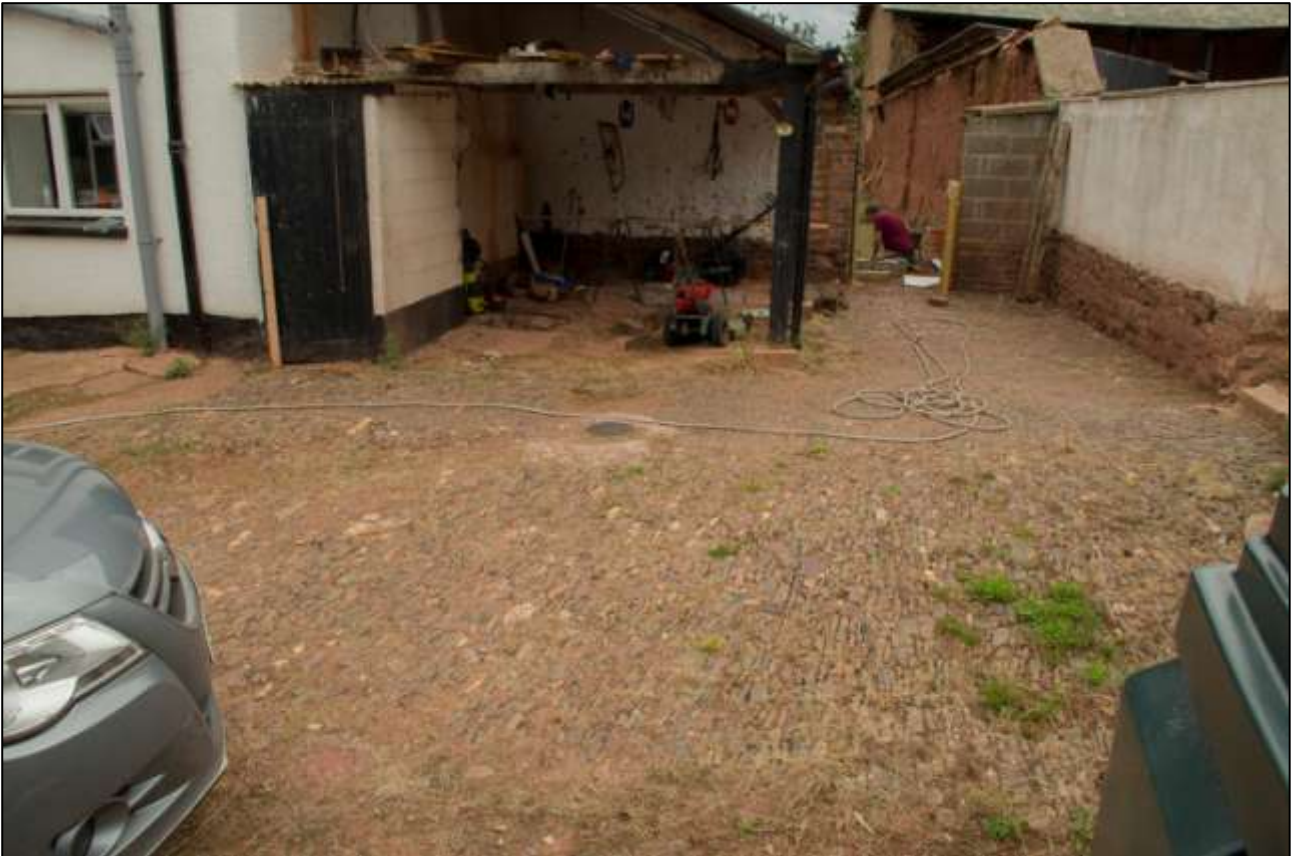
DETAIL OF THE FINE COBBLING AROUND THE FARMHOUSE; VIEWED FROM THE NORTH.
