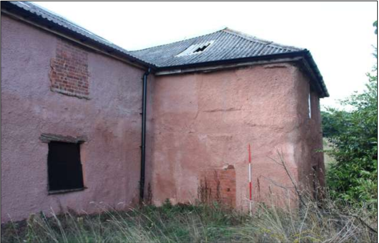
B1 EXTERIOR, THE SOUTH ELEVATION; VIEWED FROM THE SSE (SCALE 2).
