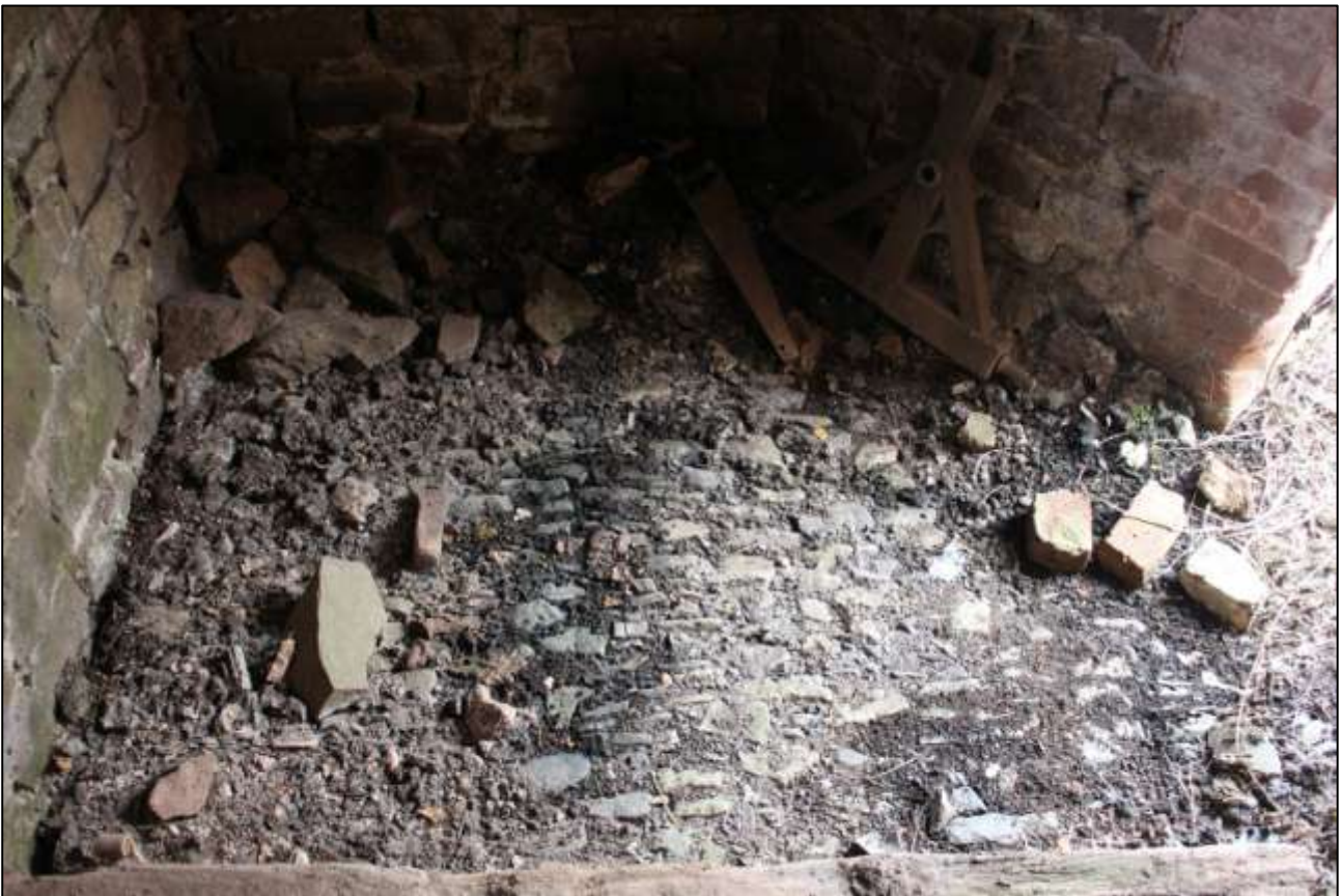
B3 INTERIOR, THE COBBLED SURFACE; VIEWED FROM THE SOUTH-WEST.
