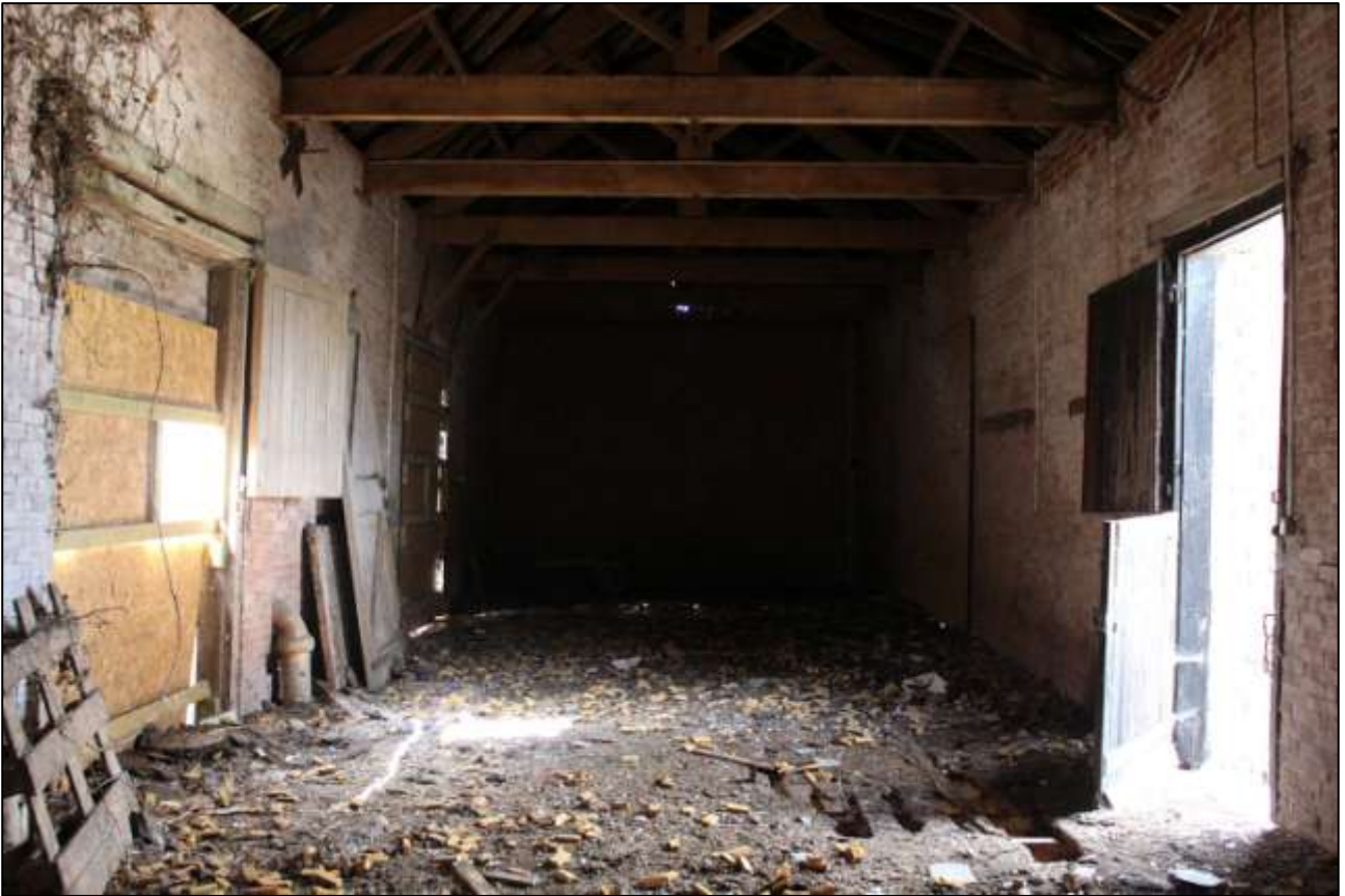
B6 FF INTERIOR; VIEWED FROM THE SOUTH.
