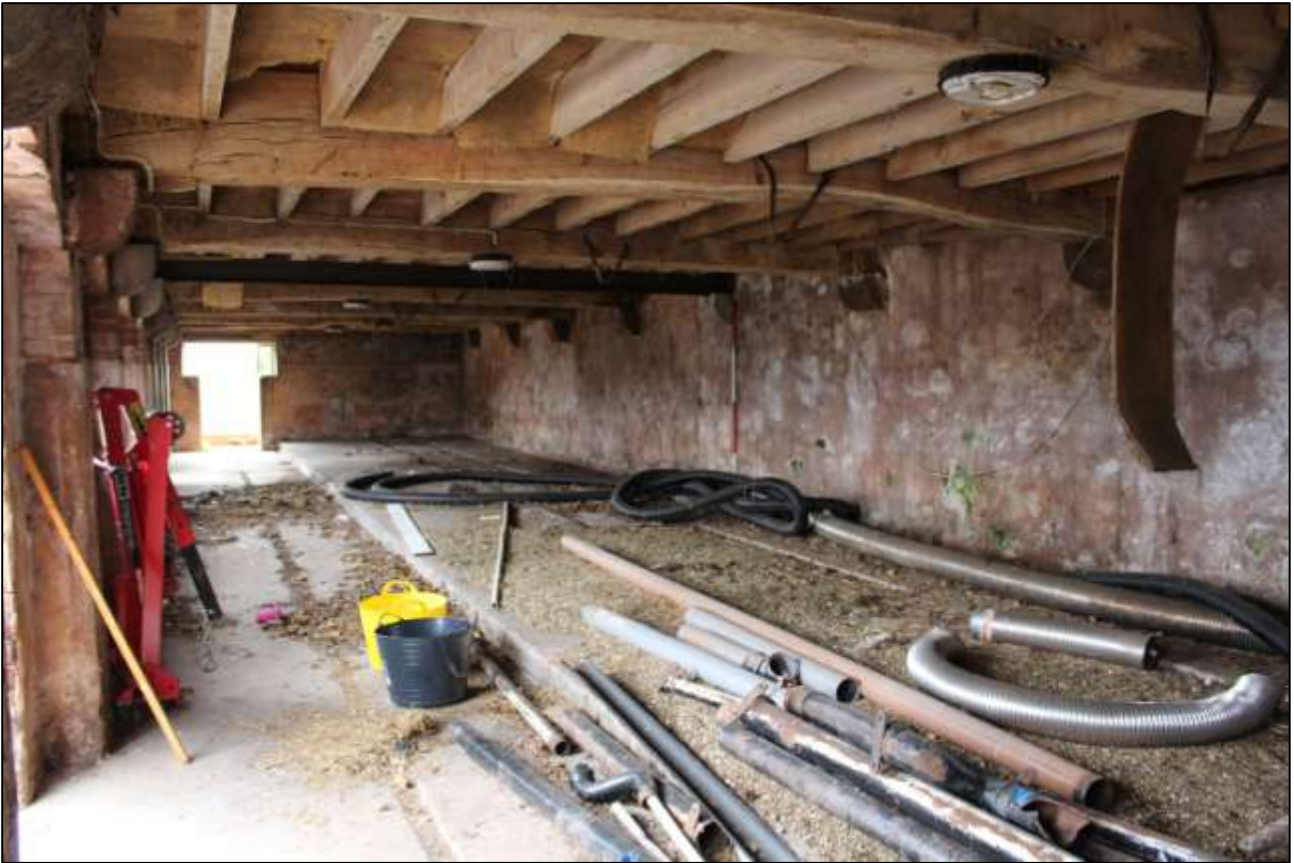
B6 GF INTERIOR; VIEWED FROM THE NNE (SCALE 2M).
