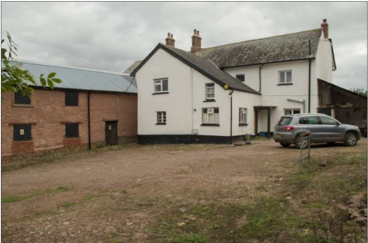
FIGURE 29: THE NORTH ELEVATION OF THE FARMHOUSE; VIEWED FROM THE NORTH-WEST.
