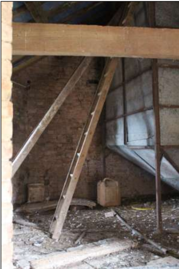
LEFT: B5 FF INTERIOR, THE SOUTH-EAST CORNER; VIEWED FROM THE NORTH.
