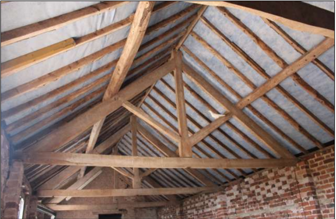
AS ABOVE, SHOWING MORE DETAIL OF THE ROOF TRUSSES.
