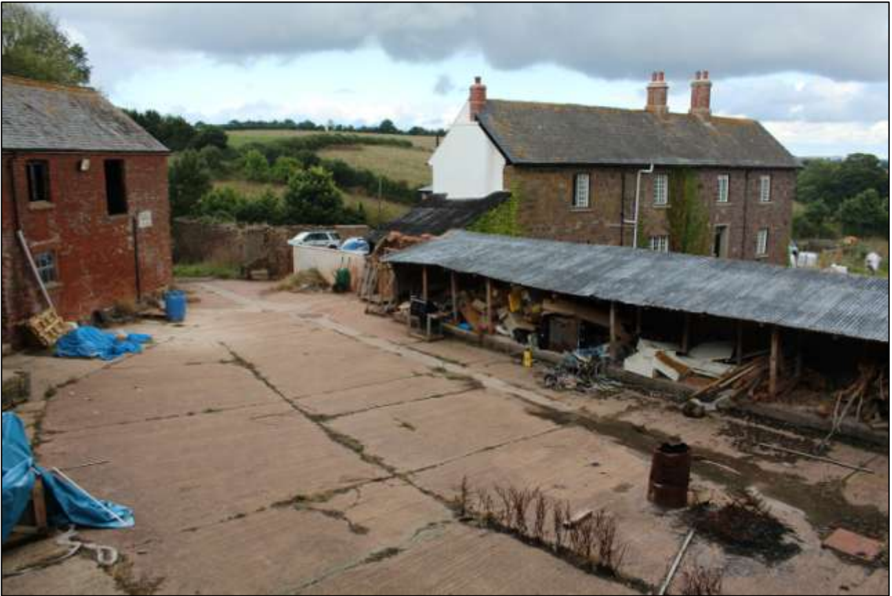
THE FARMHOUSE AS VIEWED FROM B6, WITH B10 IN THE FOREGROUND; VIEWED FROM THE SOUTH-WEST.
