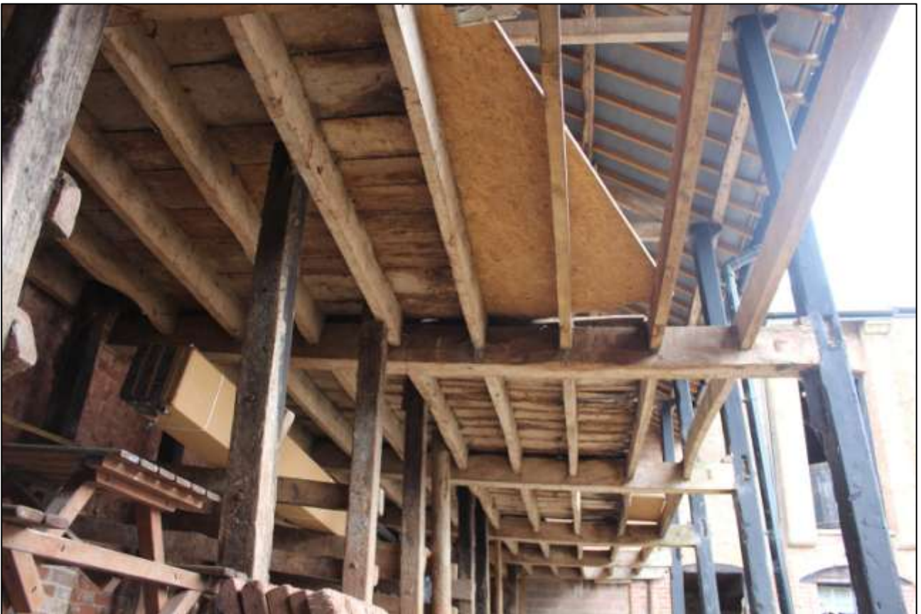
AS ABOVE, SHOWING DETAIL OF THE CEILING.
