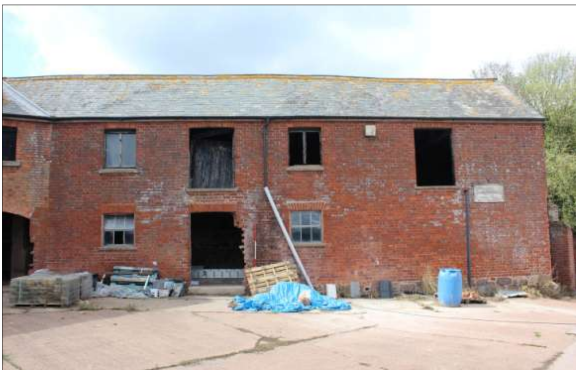
FIGURE 18: THE SOUTH-EAST ELEVATION OF B4; VIEWED FROM THE SOUTH-EAST (SCALE 2M).
