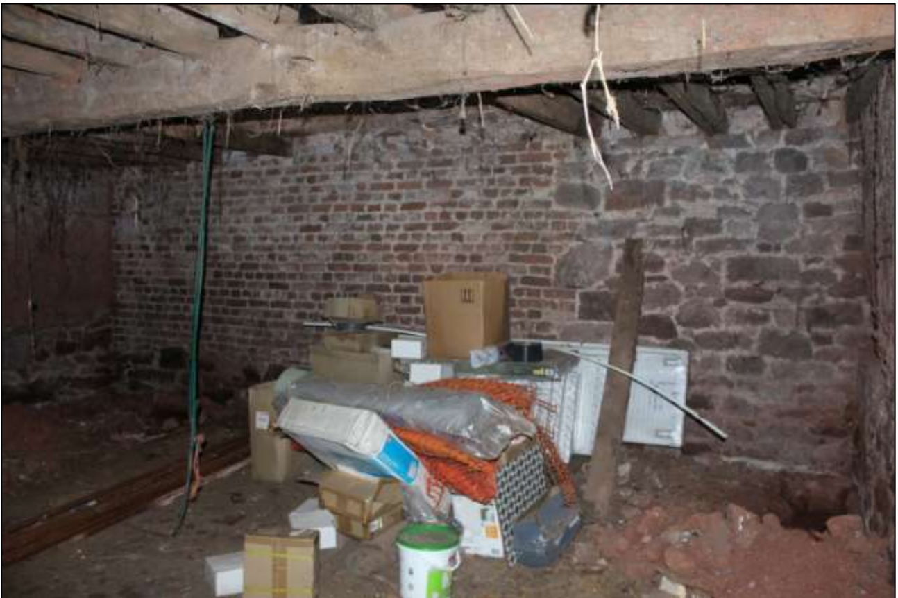
B2 GF INTERIOR; THE WALL OF THE FARMHOUSE AT THE SOUTH END OF THE BUILDING; VIEWED FROM THE NNW.
