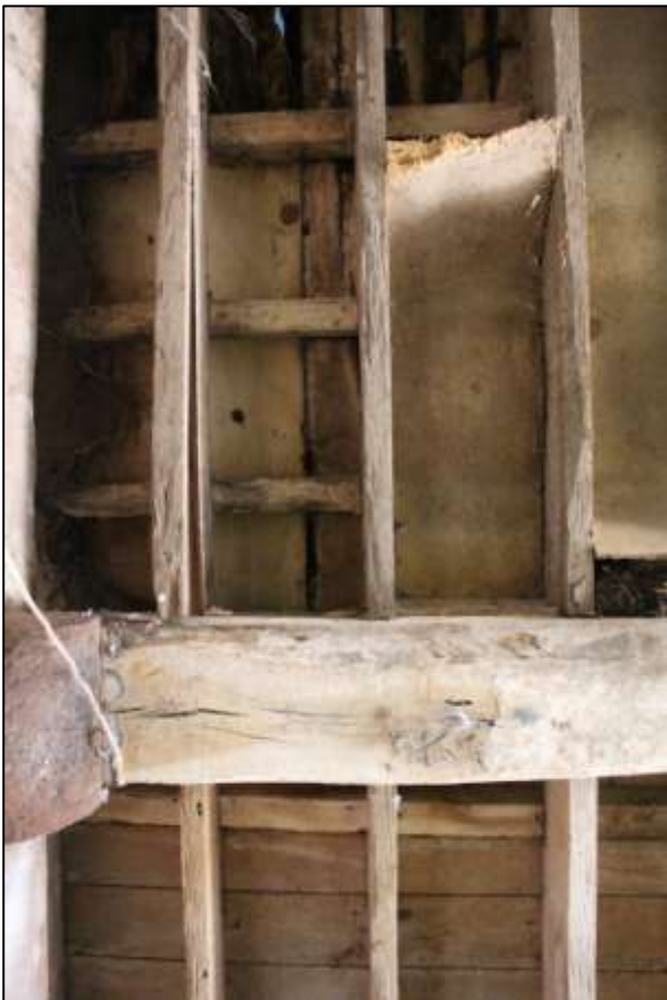
B6 GF INTERIOR, DETAIL OF THE REINFORCED FLOORS BENEATH THE THRESHING FLOORS BETWEEN THE WINNOWING DOORS, NORTH DOOR ON THE WEST SIDE; VIEWED FROM BELOW.
