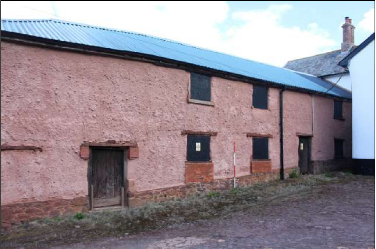
B2 EXTERIOR, WEST ELEVATION; VIEWED FROM THE NORTH-WEST (SCALE 2M).
