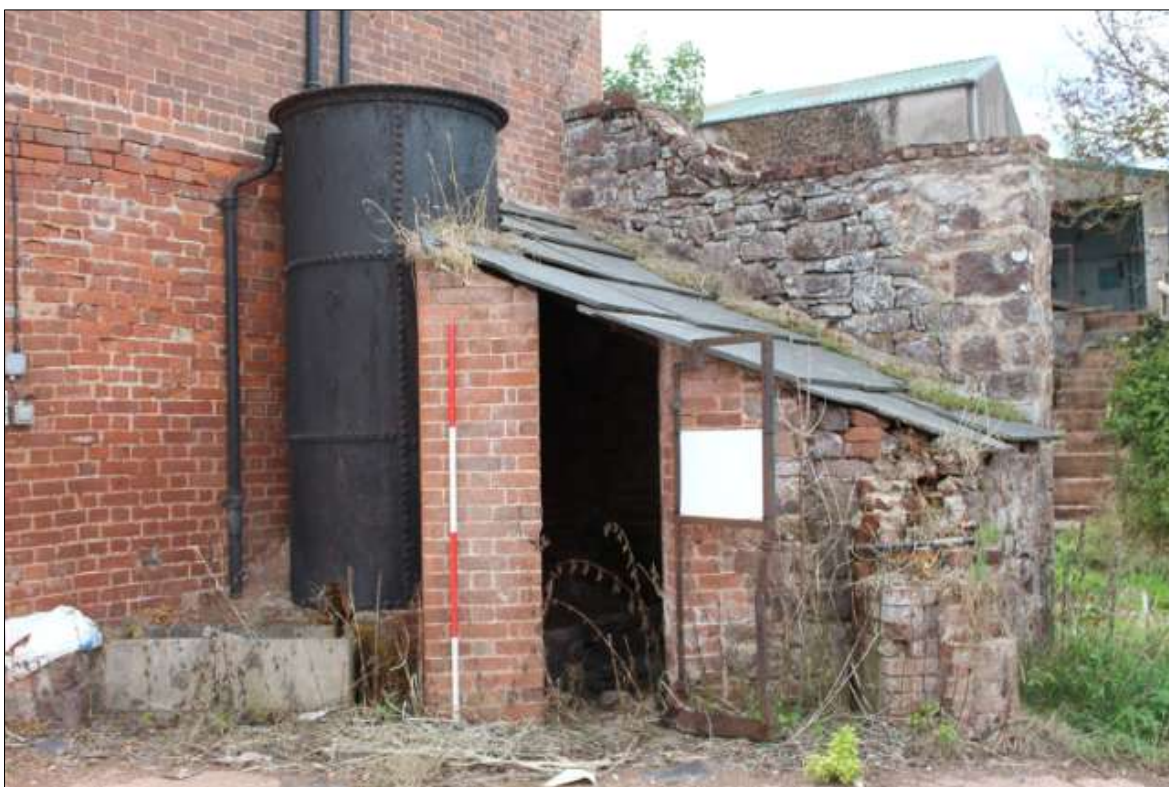
FIGURE 17: B3 WITH LARGE BOILER; VIEWED FROM THE SOUTH-EAST (SCALE 2M).
