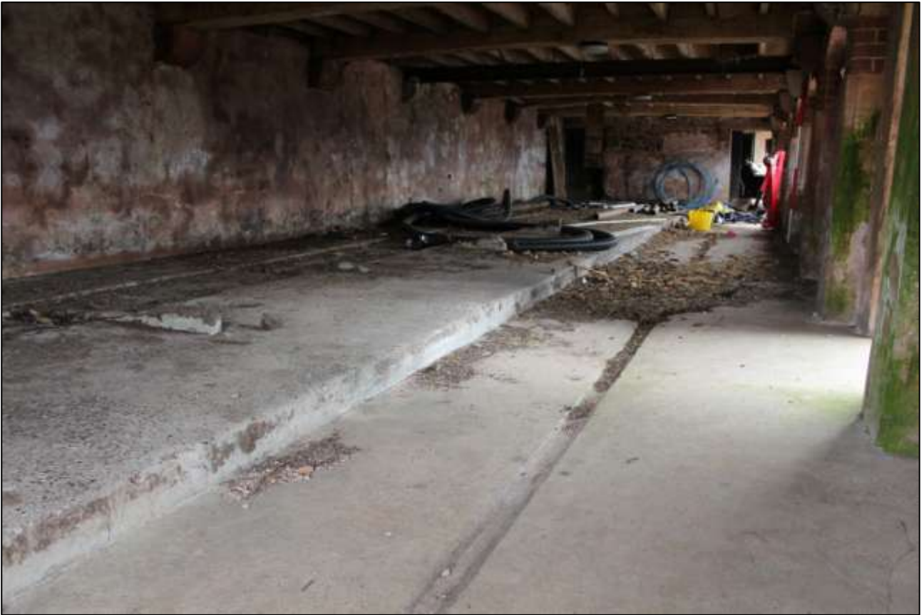
B6 GF INTERIOR; VIEWED FROM THE SSE (SCALE 2M).
