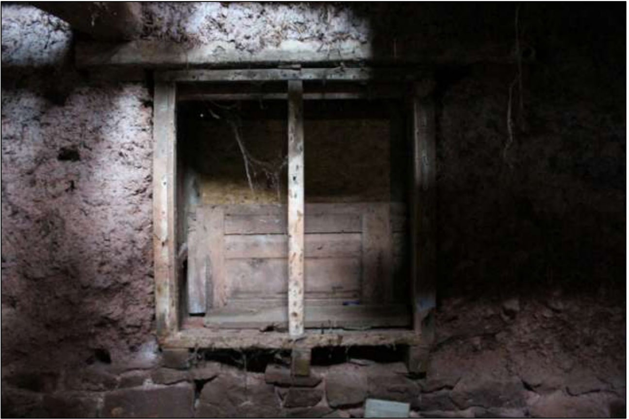
B2 GF INTERIOR, WEST WALL, DETAIL OF W1; VIEWED FROM THE EAST.
