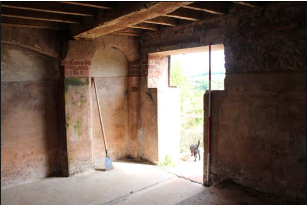
AS ABOVE; VIEWED FROM THE NORTH-WEST.
