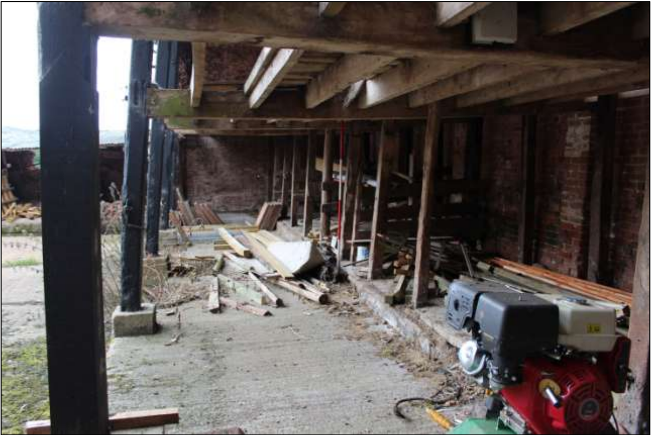
B7 GF INTERIOR; VIEWED FROM THE WEST (SCALE 2M).
