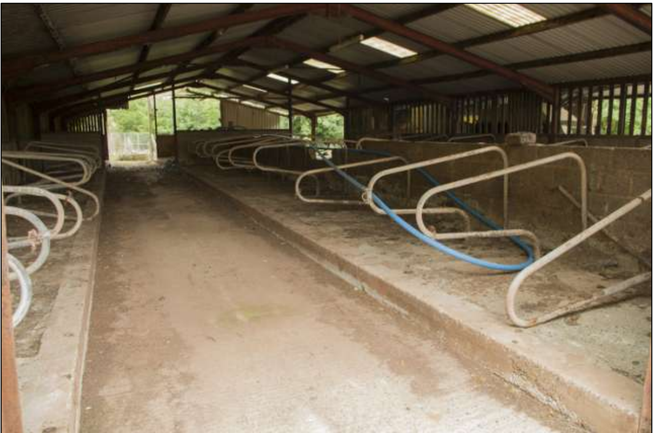
B11, THE INTERIOR OF THE MODERN COW CUBICLES; VIEWED FROM THE SOUTH.
