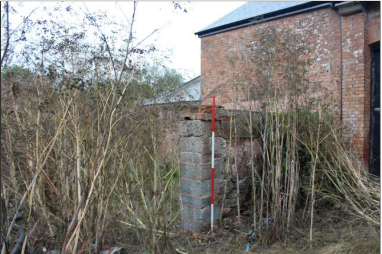
B9 EXTERIOR, THE REBUILT END OF THE BRICK AND STONE WALL; VIEWED FROM THE WEST (SCALE 2M).
