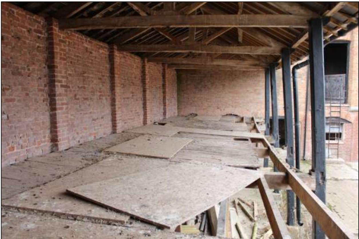
B7 FF INTERIOR; VIEWED FROM THE EAST.
