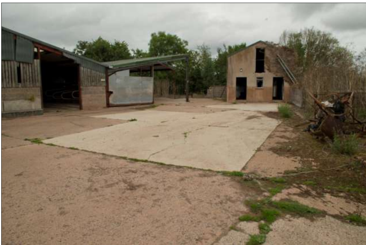
FIGURE 27: B11 THE MODERN COW CUBICLES (LEFT) AND B12 MILKING PARLOUR (RIGHT); VIEWED FROM THE SOUTH-WEST.
