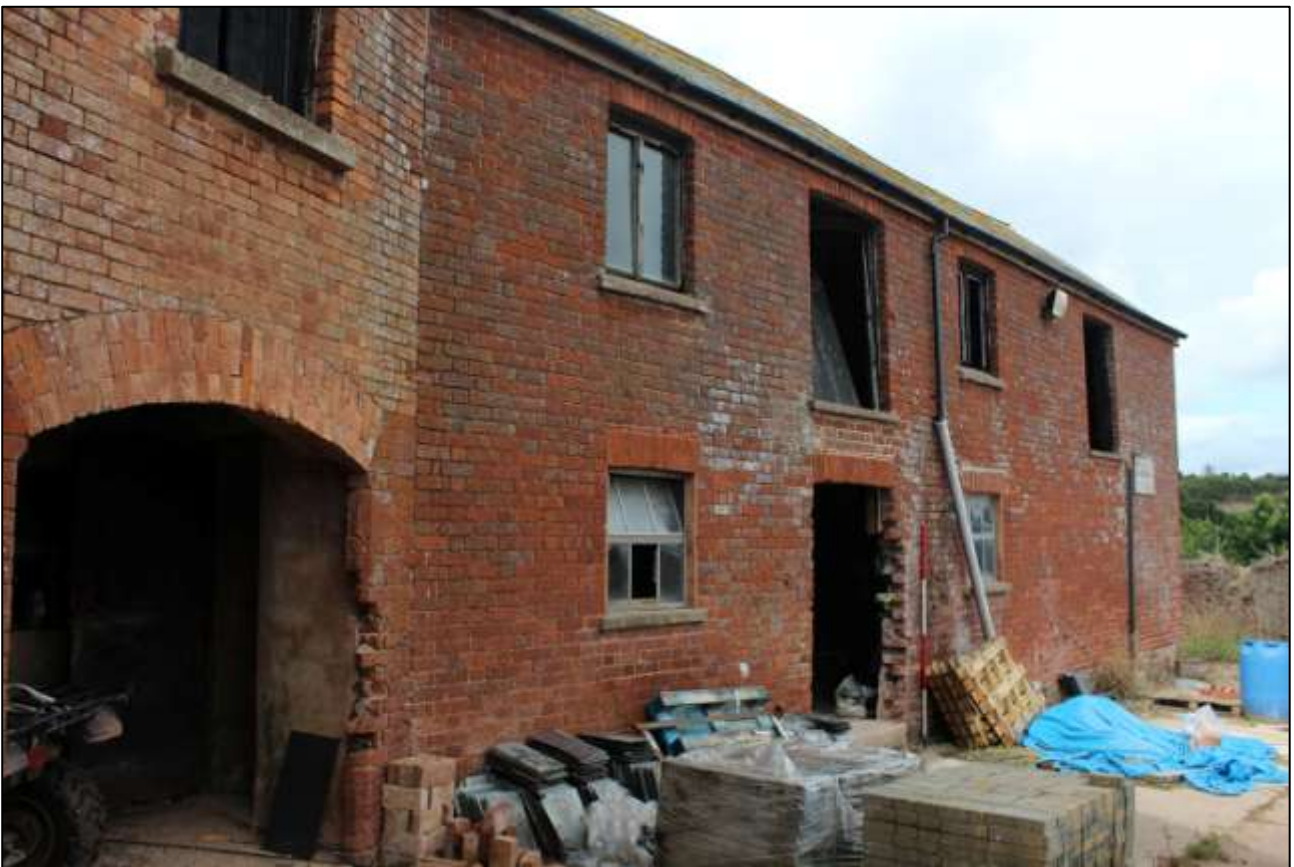
B4 EXTERIOR ELEVATION, SOUTH-EAST WALL; VIEWED FROM THE SOUTH-WEST (SCALE 2M).
