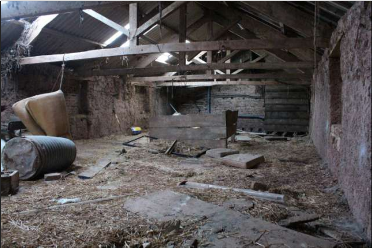
B2 FF INTERIOR; VIEWED FROM THE NNW.
