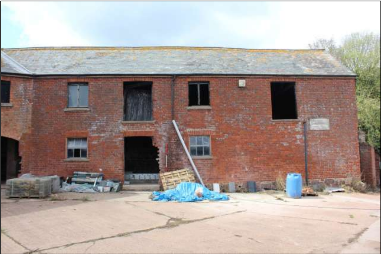
B4 EXTERIOR ELEVATION, SOUTH-EAST WALL; VIEWED FROM THE SOUTH-EAST (SCALE 2M).
