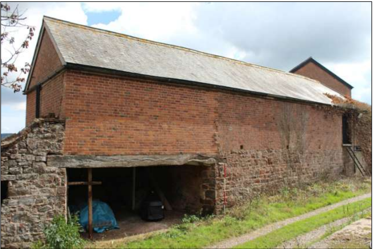
B4 EXTERIOR, NORTH-WEST WALL; VIEWED FROM THE NNW (SCALE 2M).
