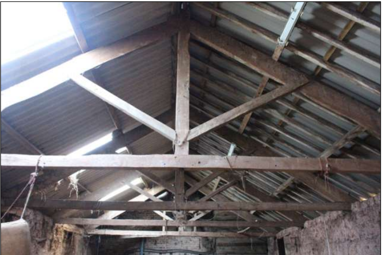
B2 FF INTERIOR, SHOWING THE KINGPOST ROOF TRUSSES; VIEWED FROM THE SOUTH.
