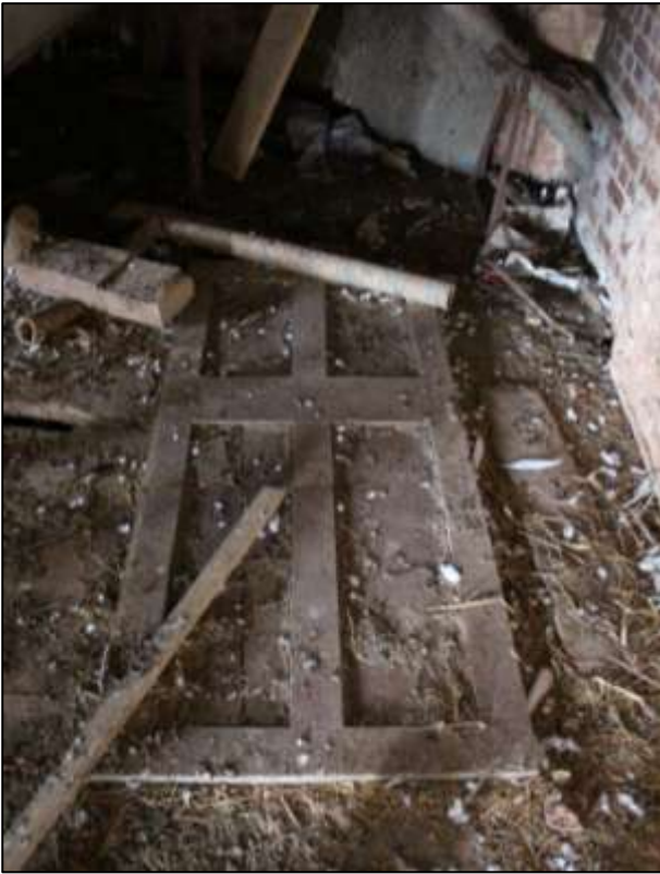
RIGHT: B5 FF INTERIOR, EX SITU DOOR ON THE FLOOR; VIEWED FROM THE EAST.
