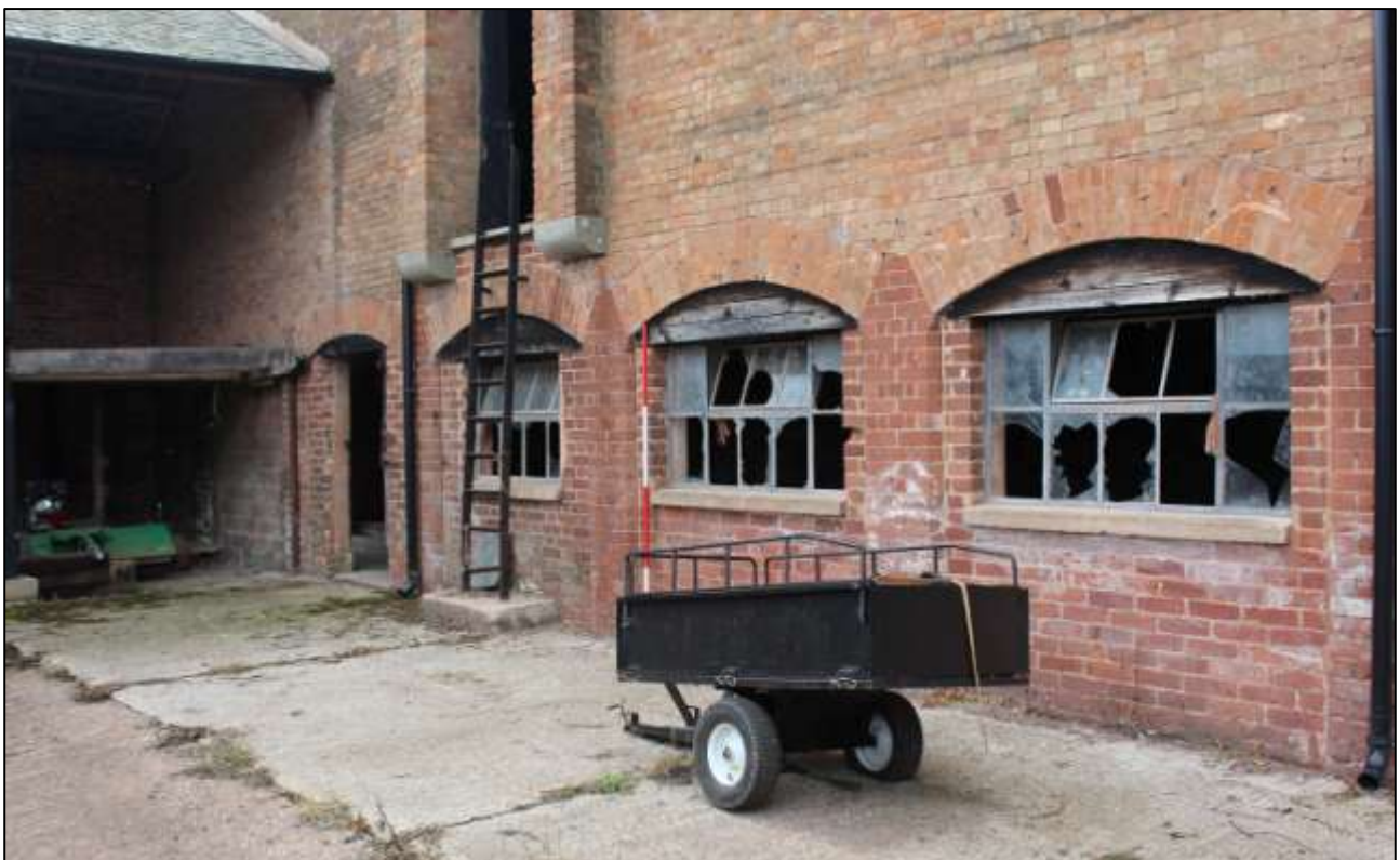
B6 EXTERIOR, EAST WALL, DETAIL OF THE BLOCKED GF OPENINGS; VIEWED FROM THE NORTH-EAST (SCALE 2M).
