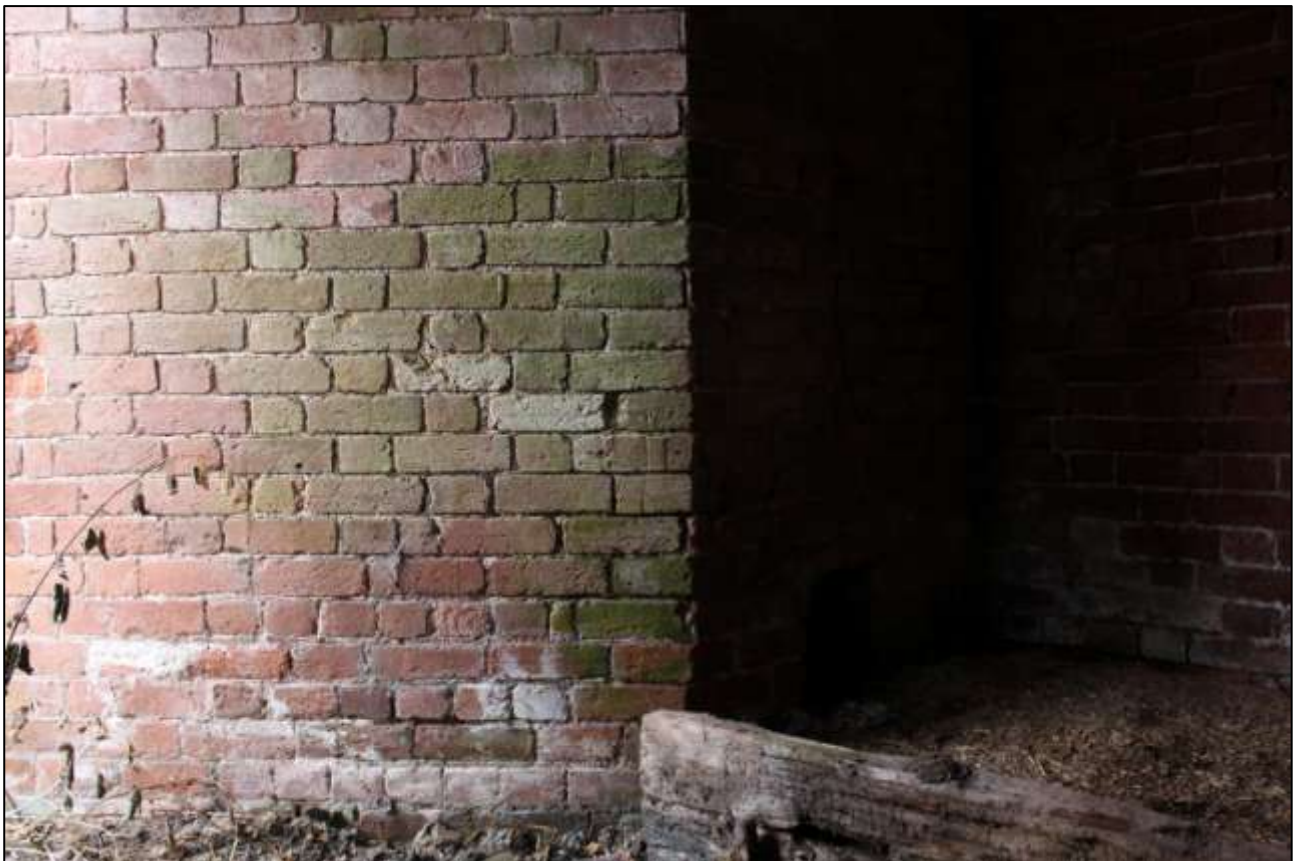
B3, INTERIOR, THE BRICKWORK ENCASING THE BOILER; VIEWED FROM THE NORTH-EAST.
