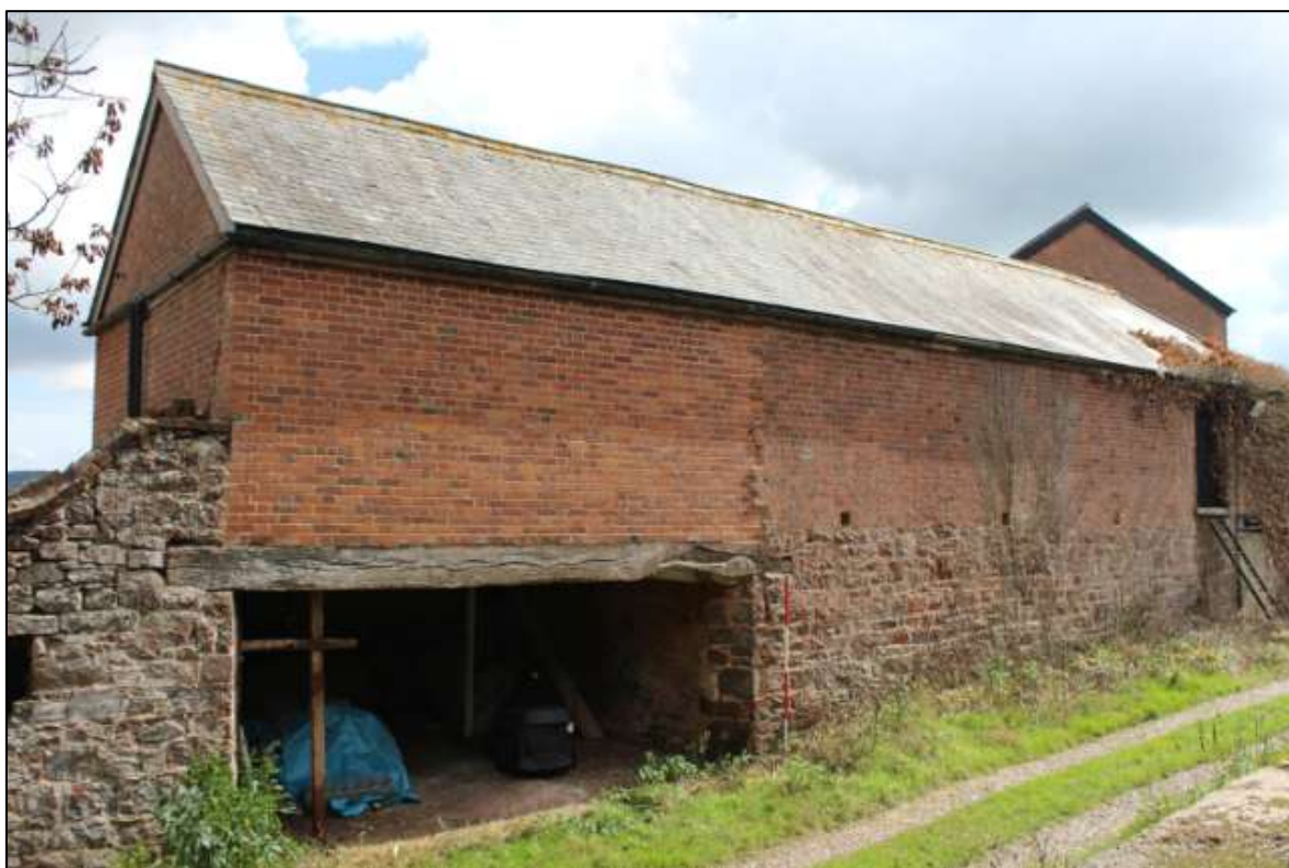
FIGURE 19: THE NORTH-WEST ELEVATION OF B4; VIEWED FROM THE NORTH (SCALE 2M).
