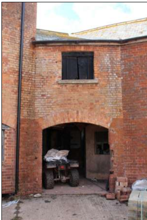
FIGURE 20: THE SOUTH-EAST ELEVATION OF B5; VIEWED FROM THE SOUTH-EAST.
