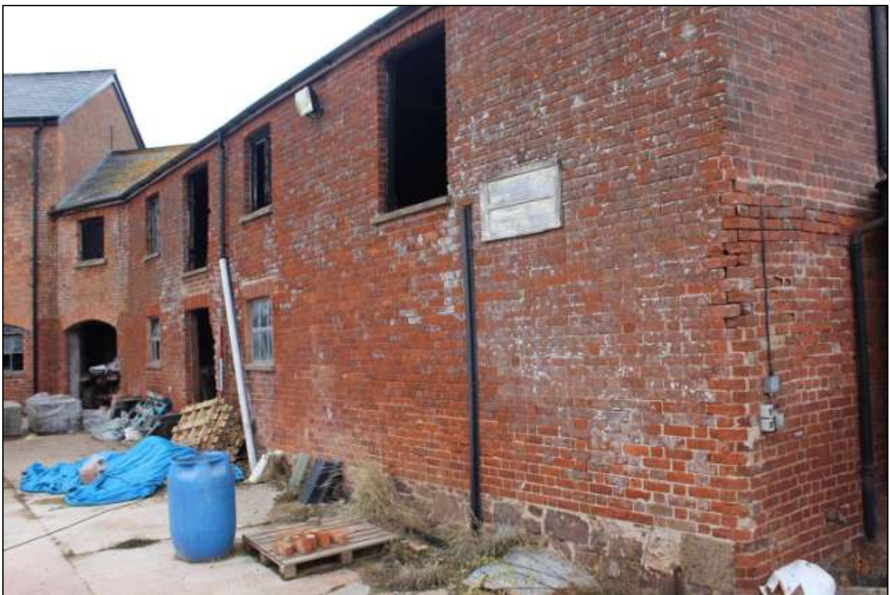
B4 EXTERIOR ELEVATION, SOUTH-EAST WALL; VIEWED FROM THE NORTH-EAST (SCALE 2M).
