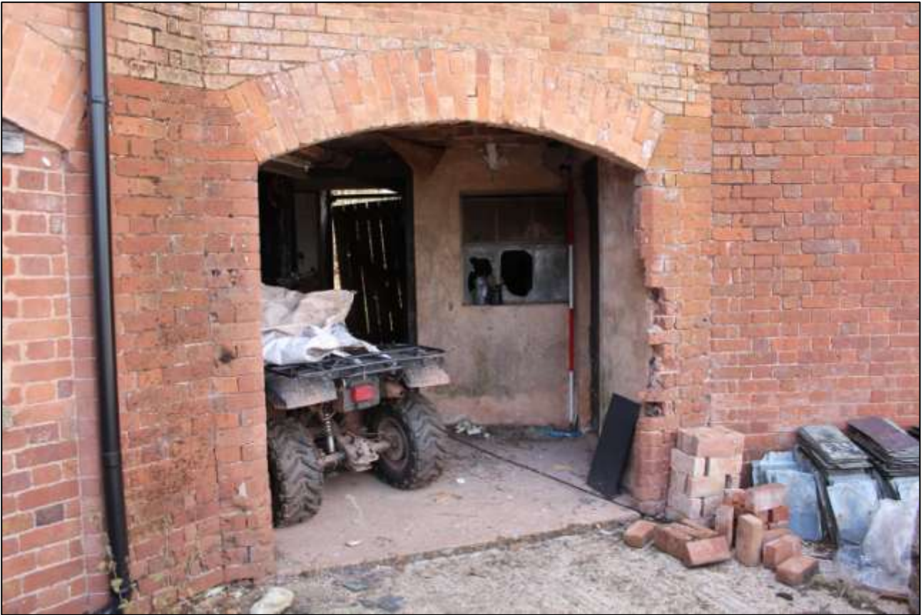
AS ABOVE, DETAIL OF THE GF OPENING; VIEWED FROM THE ESE.
