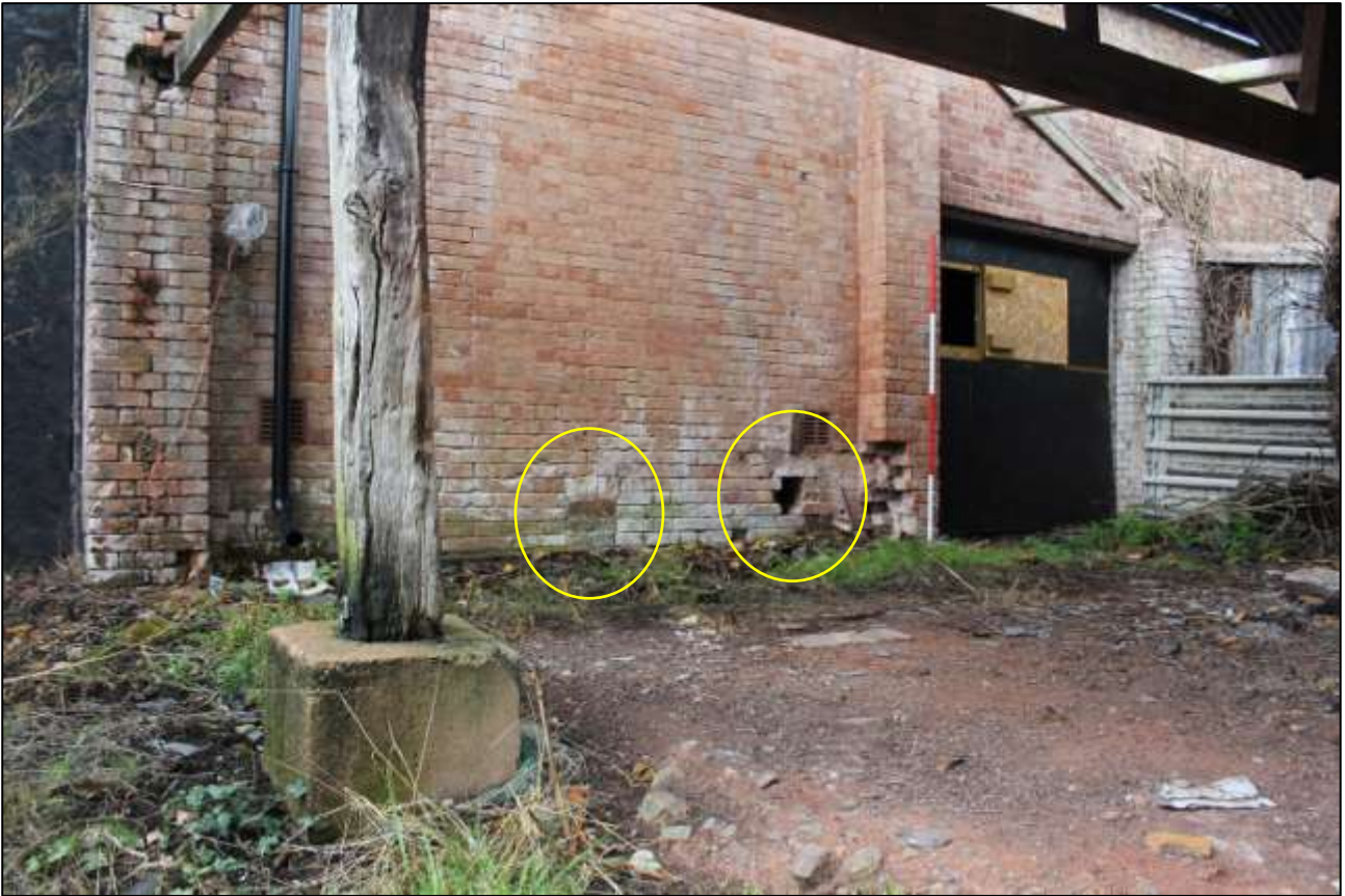
B6 EXTERIOR, WEST WALL, SHOWING THE BLOCKED AND FORCED SHAFT OPENINGS (INDICATED); VIEWED FROM THE WNW.
