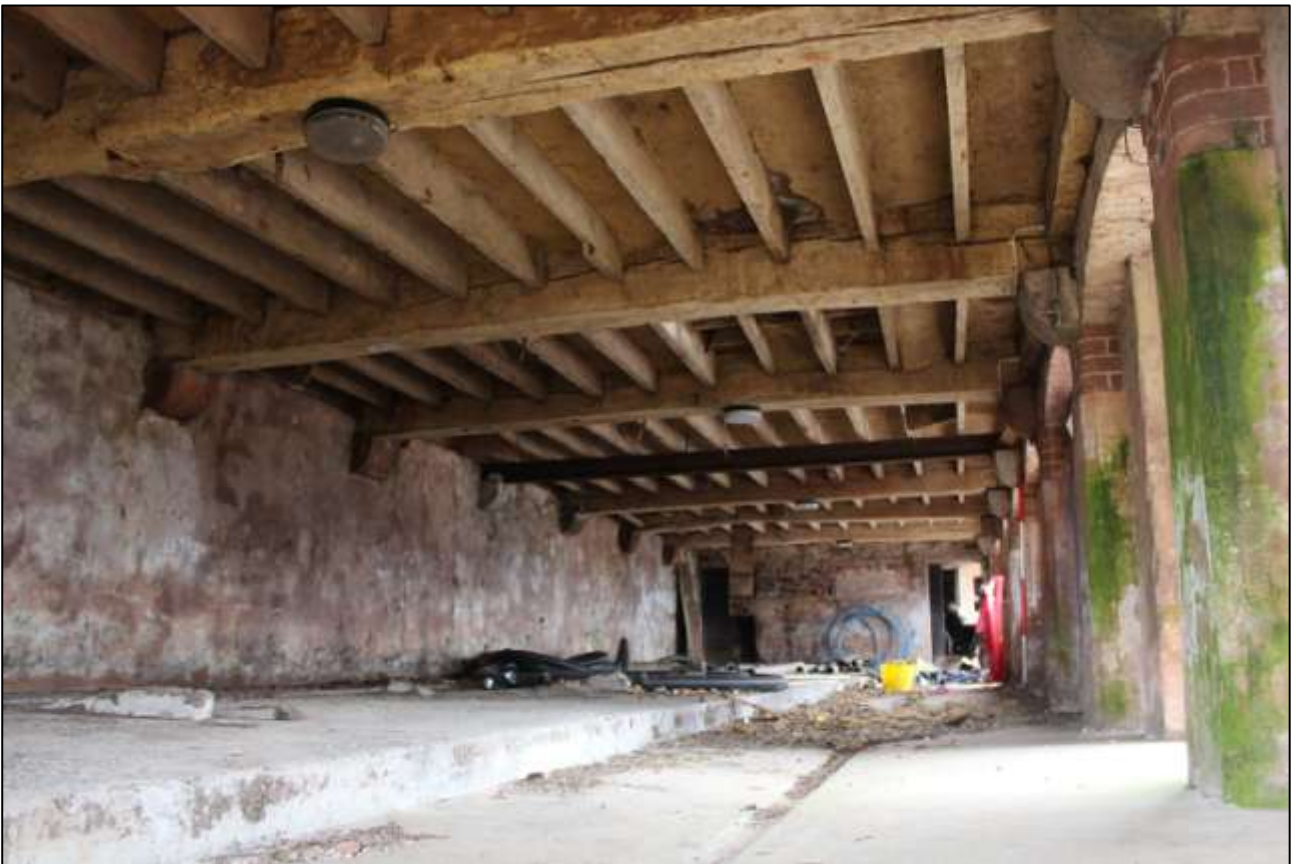
AS ABOVE, DETAIL OF THE CEILING.
