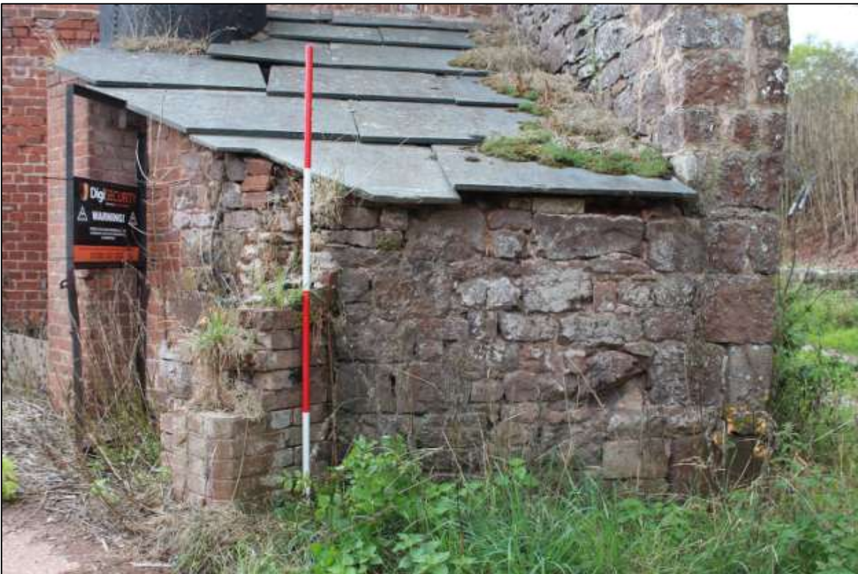
B3, EXTERIOR ELEVATION, NORTH-EAST WALL AND WEST SIDE OF THE ENTRANCE; VIEWED FROM THE NORTH-EAST (SCALE 2M).
