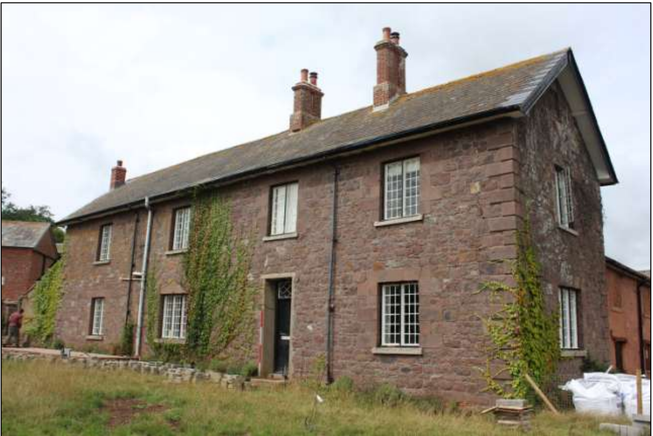
THE SOUTH ELEVATION OF THE FARMHOUSE; VIEWED FROM THE SOUTH-EAST (SCALE 2M).
