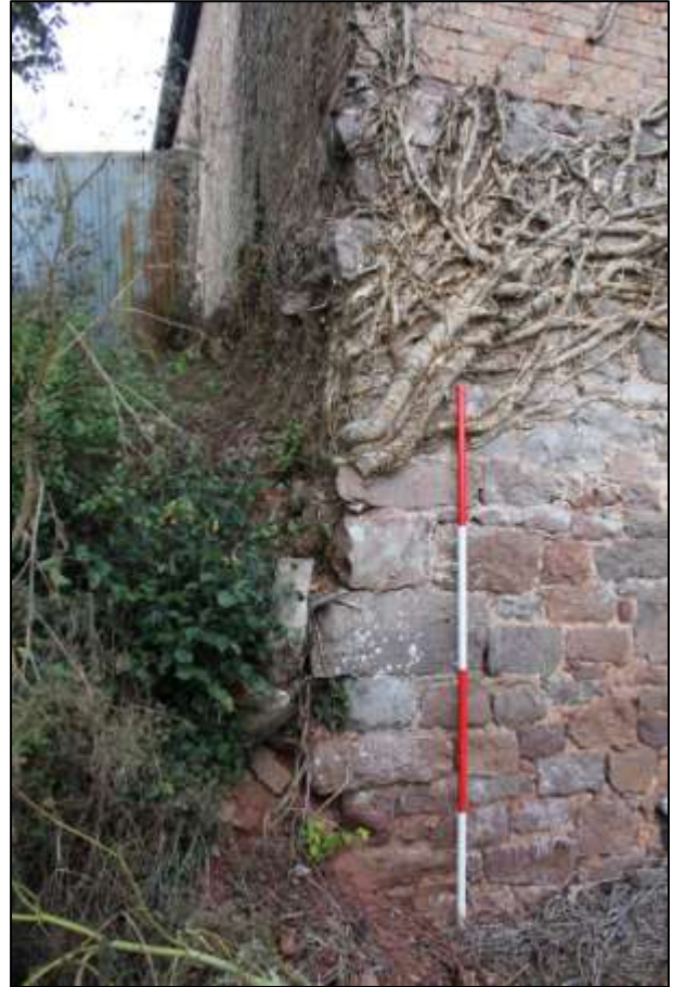
RIGHT: B6 EXTERIOR, SHOWING THE RAGGED CORNER TO THE STONE PLINTH; VIEWED FROM THE SOUTH (SCALE 2M).
