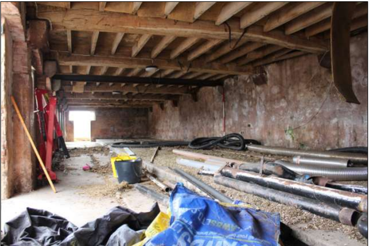
AS ABOVE, WITH DETAIL OF THE CEILING.
