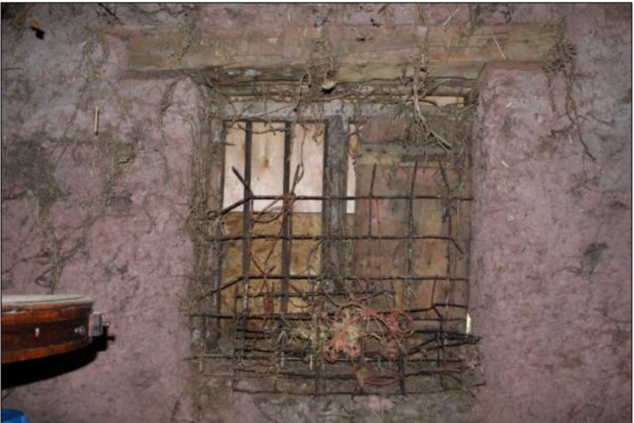
B2 GF INTERIOR, EAST WALL, DETAIL OF W8; VIEWED FROM THE WEST.
