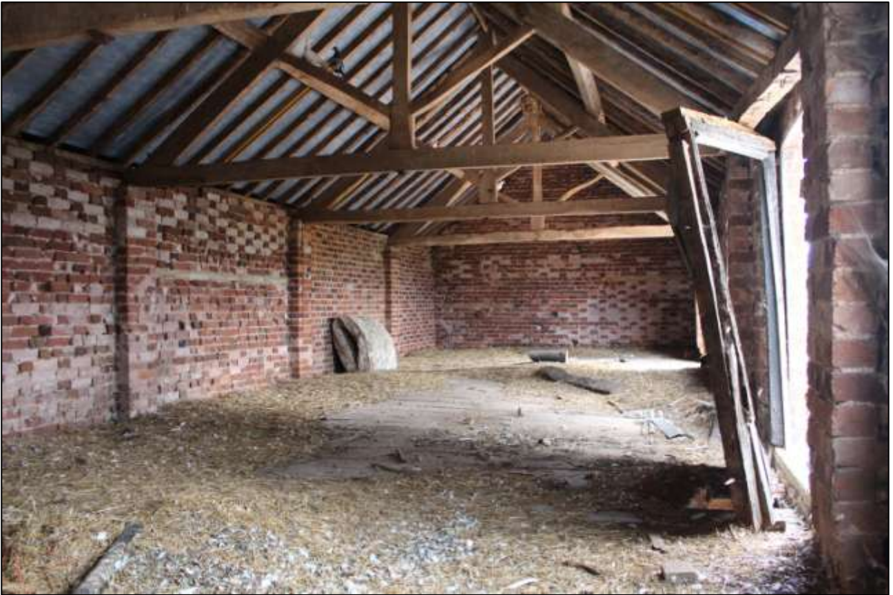
B4 FF INTERIOR; VIEWED FROM THE SOUTH-WEST.
