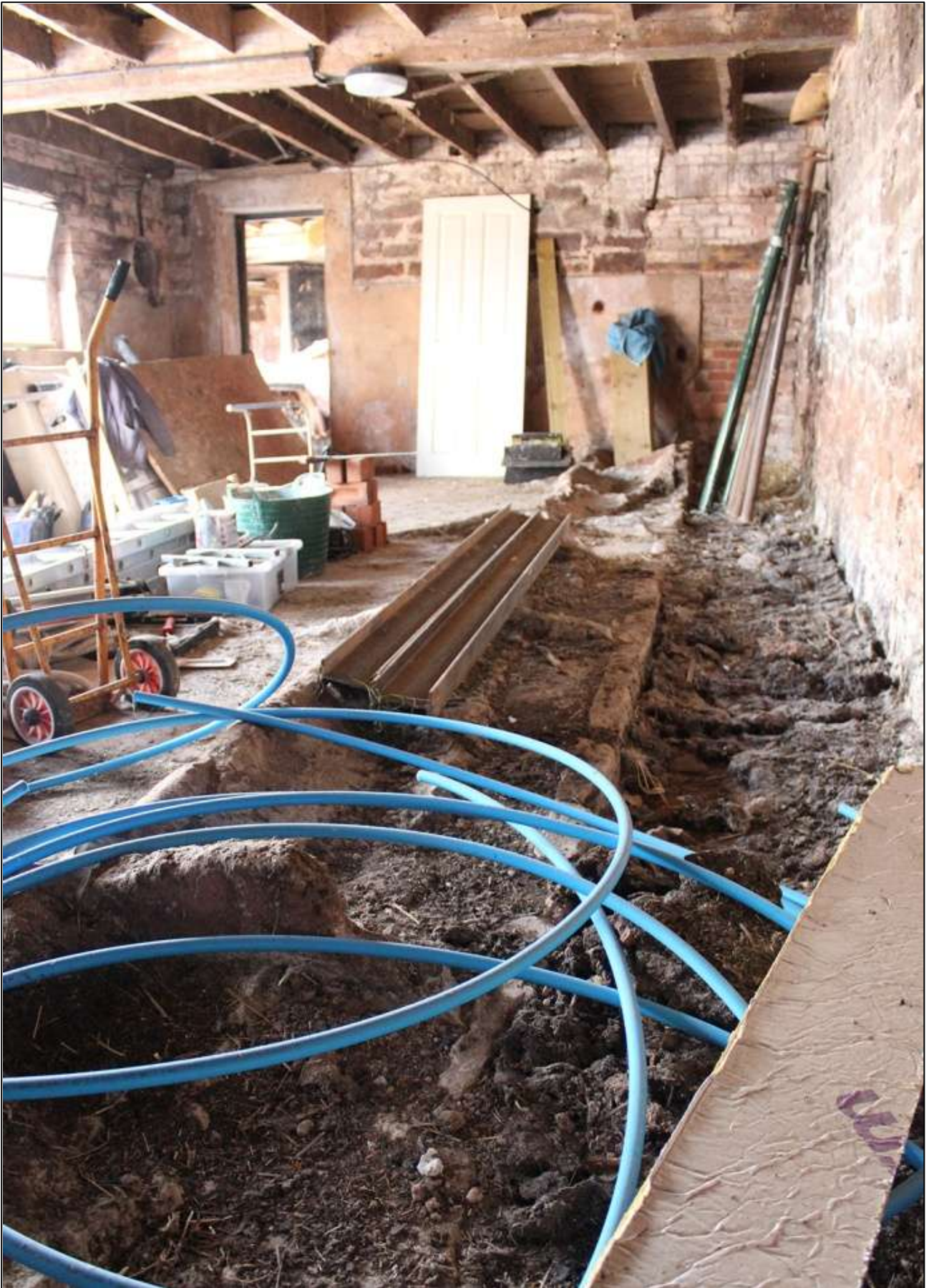
B4A INTERIOR; VIEWED FROM THE NORTH-EAST.
