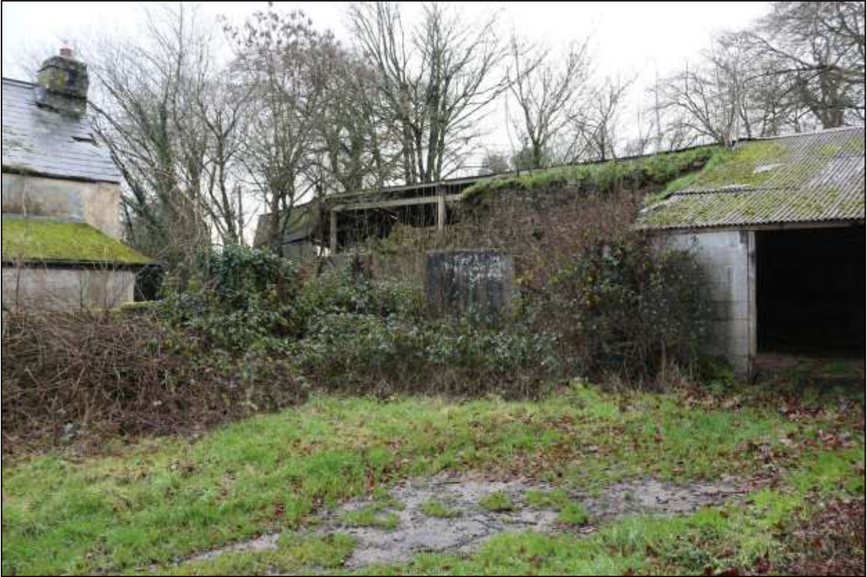
136. REMAINS OF WESTERN LINHAY RANGE ON THE SOUTH-WEST SIDE OF THE FARMYARD. RUBBLE WALL TO REAR OF LINHAY, THE REST LARGELY REBUILT IN THE MID-20 TH CENTURY. HOUSE TO LEFT. VIEWED FROM THE NORTH.
