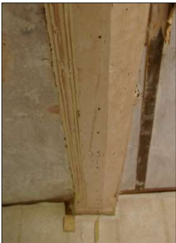
LEFT FIGURE 9: MOULDED AND CHAMFERED BEAM IN THE HALL; VIEWED FROM THE NORTH-EAST.
