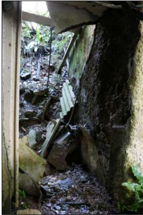
37. RIGHT: PRIVY R8 FILLED WITH COLLAPSED COB FROM BACK WALL OF R1 (THROUGH D13); VIEWED FROM THE NORTH-WEST.
