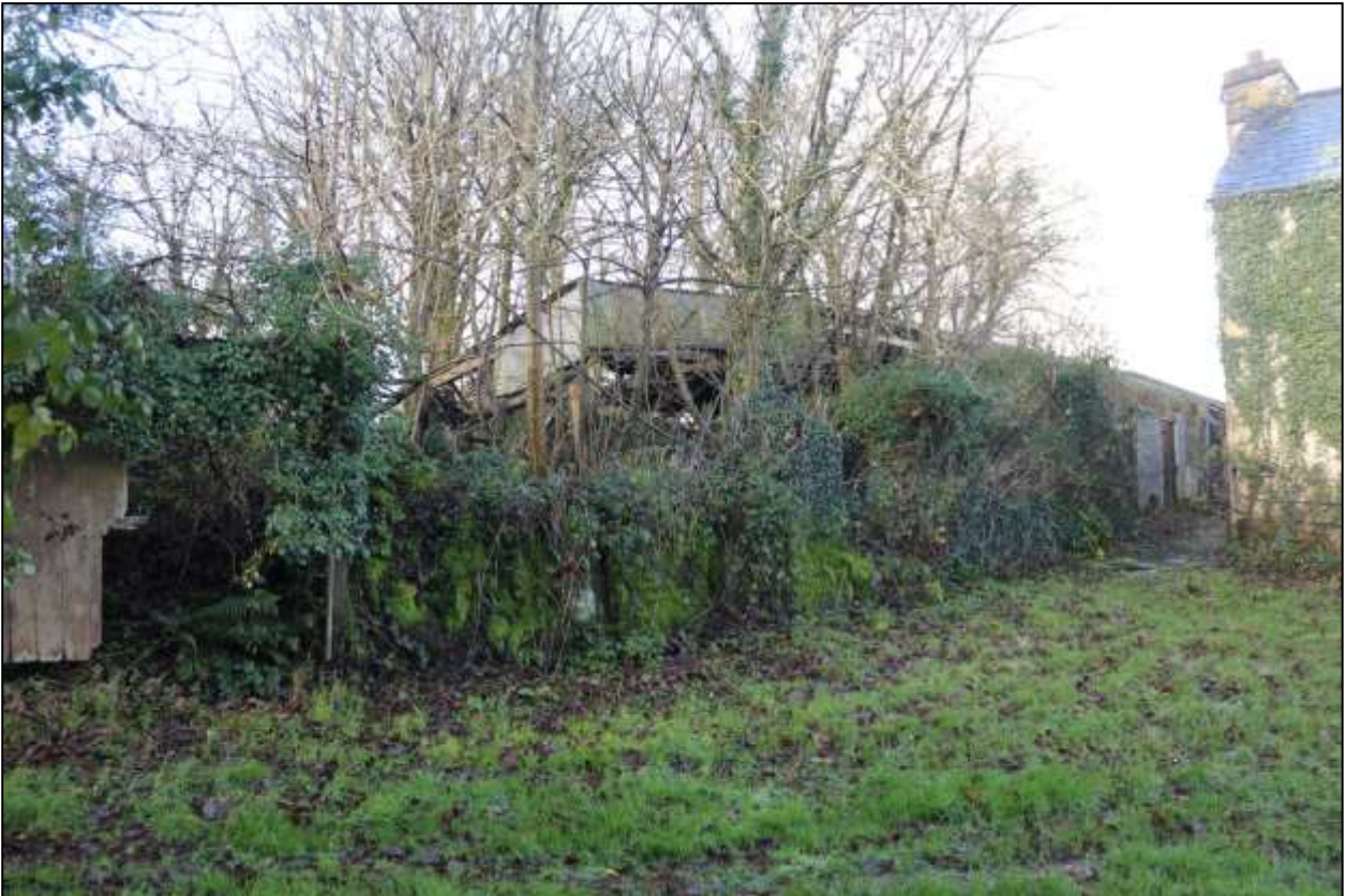
138. RUIN OF THE THRESHING BARN ON SOUTH-WEST SIDE OF THE HOUSE. LOW WALLS ARE THE RUBBLE STONE PLINTHS FOR A COB BUILDING ALMOST ALL OF WHICH HAS COLLAPSED INWARDS. REMAINS OF TIMBER AND CORRUGATED IRON GARAGE ON LEFT ABOUT THE BARN. SOUTH-WEST CORNER OF FARMHOUSE TO RIGHT. VIEWED FROM THE SOUTH.
