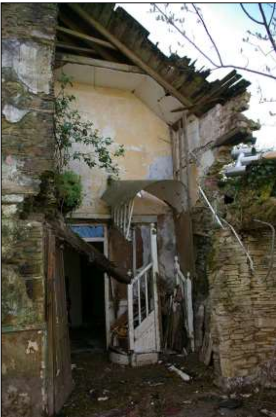
118. LEFT: LATE 17 TH OR EARLY 18 TH CENTURY-FRAMED STAIR TO THE FIRST FLOOR IN R2B BETWEEN R2 AND R3; VIEWED FROM THE ENE.
