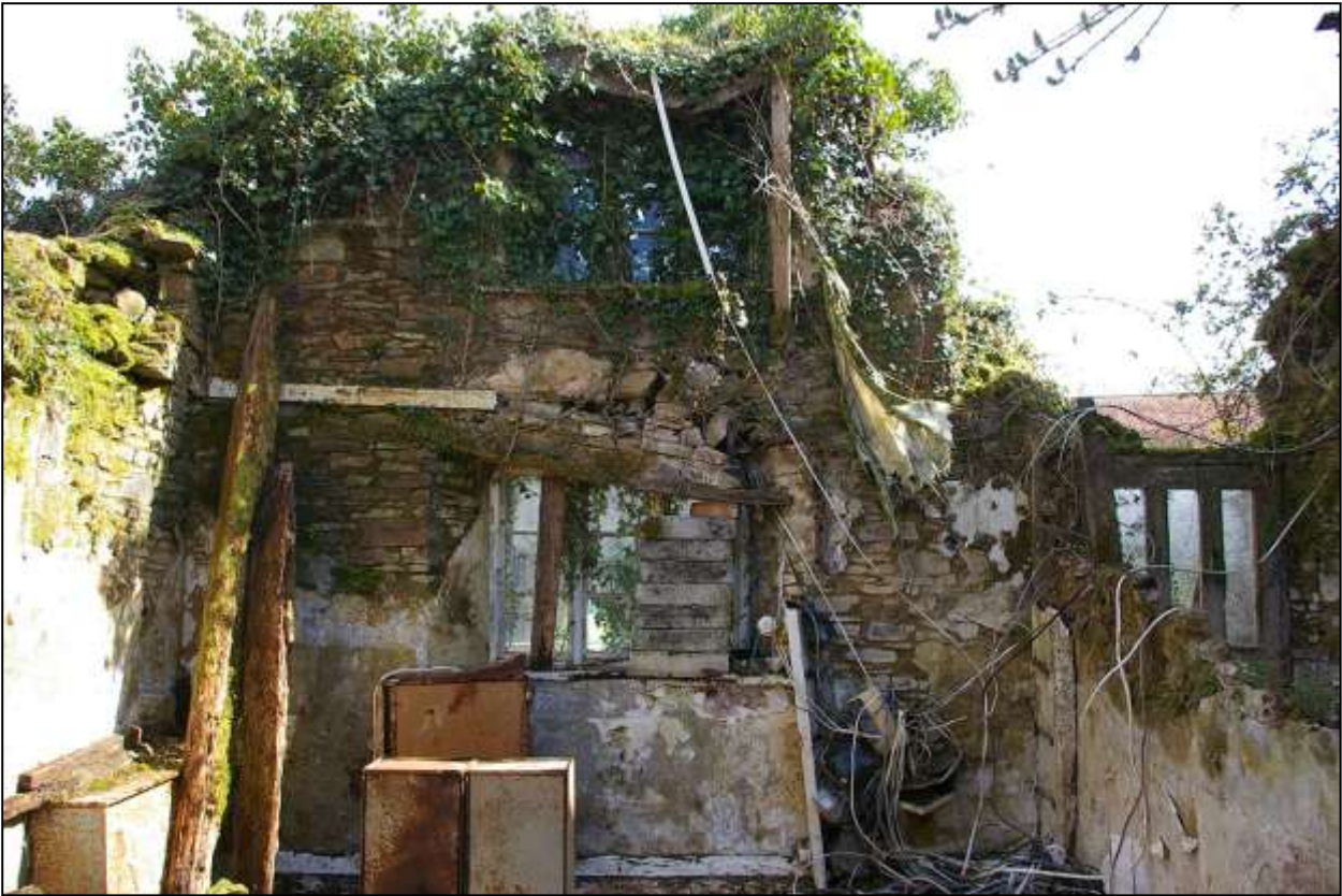
66. SOUTH-EAST FRONT WALL OF HOUSE IN R2 (SHOWING W2 AND W8). REBUILT IN STONE RUBBLE PROBABLY IN THE 17 TH CENTURY, RUINOUS PARTITION TO CROSS PASSAGE R2A IS VISIBLE TO RIGHT. VIEWED FROM THE NORTH-WEST.
