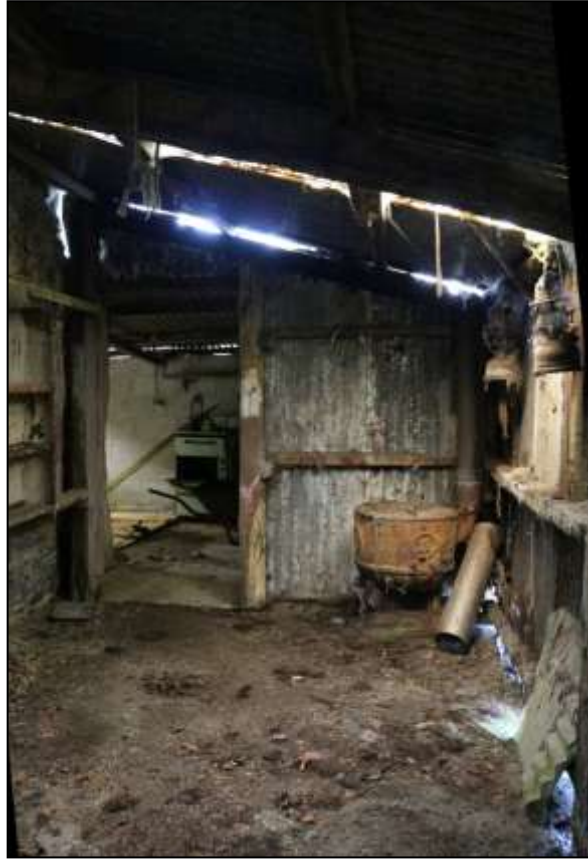
43. RIGHT: THE CORRUGATED IRON SHED, 19 TH CENTURY CAST IRON SWILL BOILER IN THE WEST CORNER; VIEWED FROM THE SOUTH-EAST.
