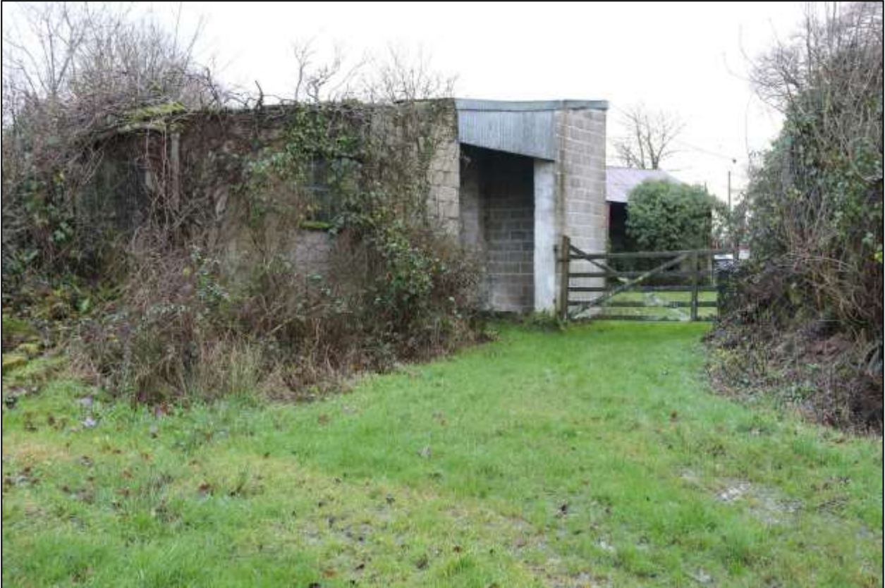
132. NORTH END OF LINHAY WING; MOSTLY MID-20 TH CENTURY CONSTRUCTION, NEAR BLOCKWORK FACING RUBBLE. VIEWED FROM THE NORTH.
