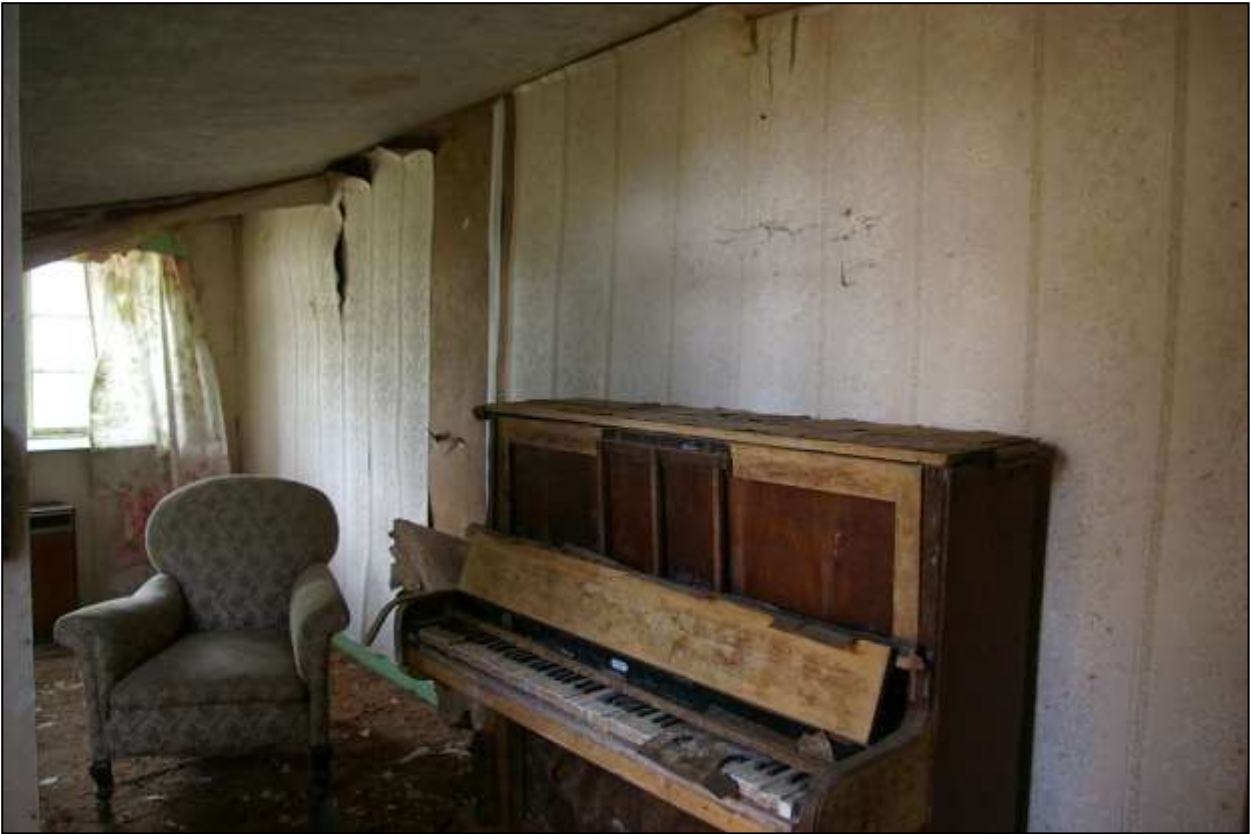
79. WEST WALL OF R3; VIEWED FROM THE NORTH.
