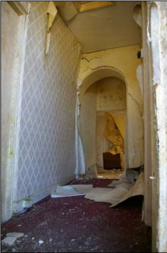
120. LEFT: R9, THE FIRST-FLOOR CORRIDOR, LOOKING THROUGH THE FORCED OPENING IN THE COB WALL BETWEEN THE MEDIEVAL AND THE 17 TH CENTURY EXTENSION. VIEWED FROM THE NORTH-EAST.
