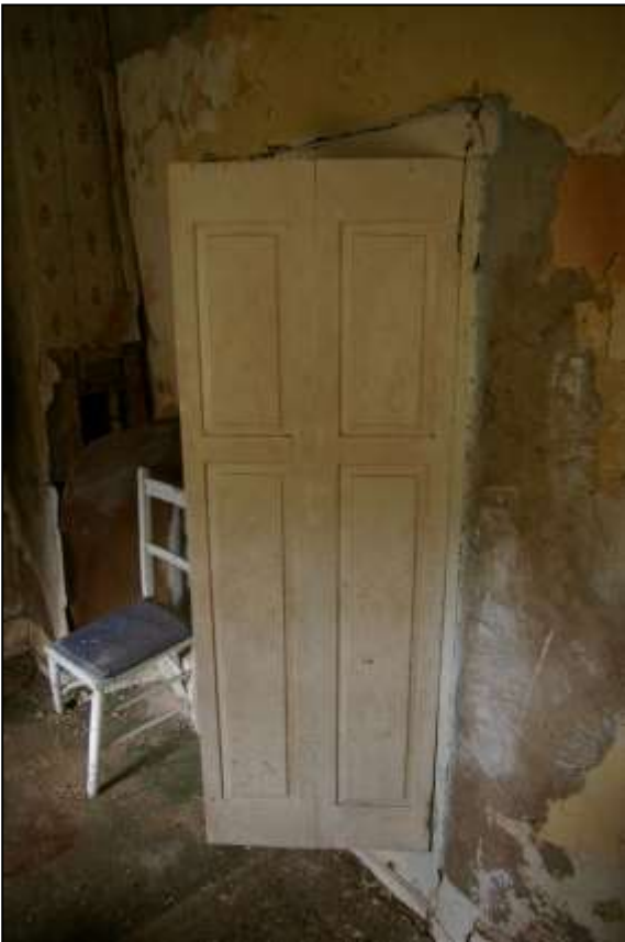
102. LEFT: VIEW OF THE BLOCKED DOOR (BO3) TO R3 IN R5, NOW USED AS A CUPBOARD, WITH RESET RAISED AND FIELDDED LATER 17 TH OR EARLY 18 TH CENTURY SHUTTERS. VIEWED FROM THE WEST
