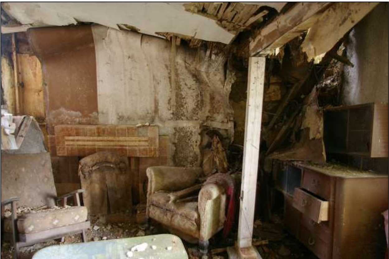
76. THE NORTH-EAST WALL OF R3, WITH THE MASSIVE INFILLED HEARTH, NOW SET WITH SMALL MID-20 TH CENTURY TILED FIREPLACE; VIEWED FROM THE SOUTH-WEST. NOTE 19 TH CENTURY LATH AND PLASTER CEILING AND BOXED CHAMFERED BEAM SUPPORTED ON POLE.
