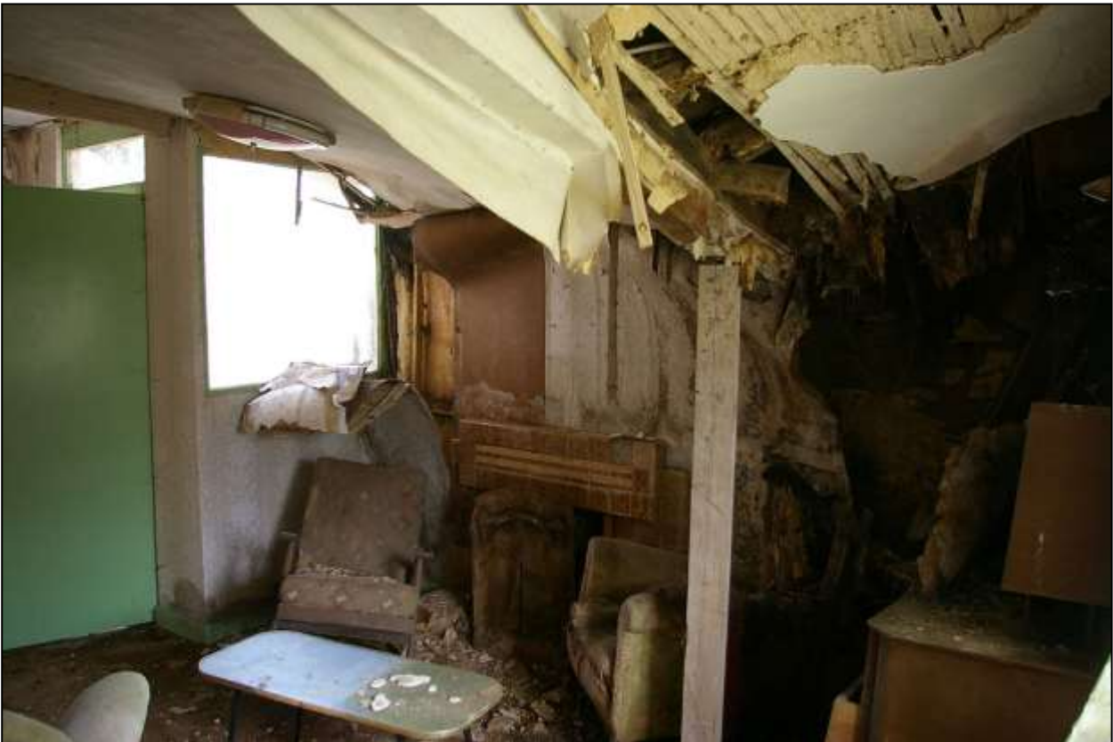
74. R3, WITH 1950S TILED HEARTH AGAINST STACK WALL. SOUTHERN CHAMFERED BEAM IS PROPPED UP ON A POLE IN RIGHT FOREGROUND. VIEWED FROM THE SOUTH-WEST.
