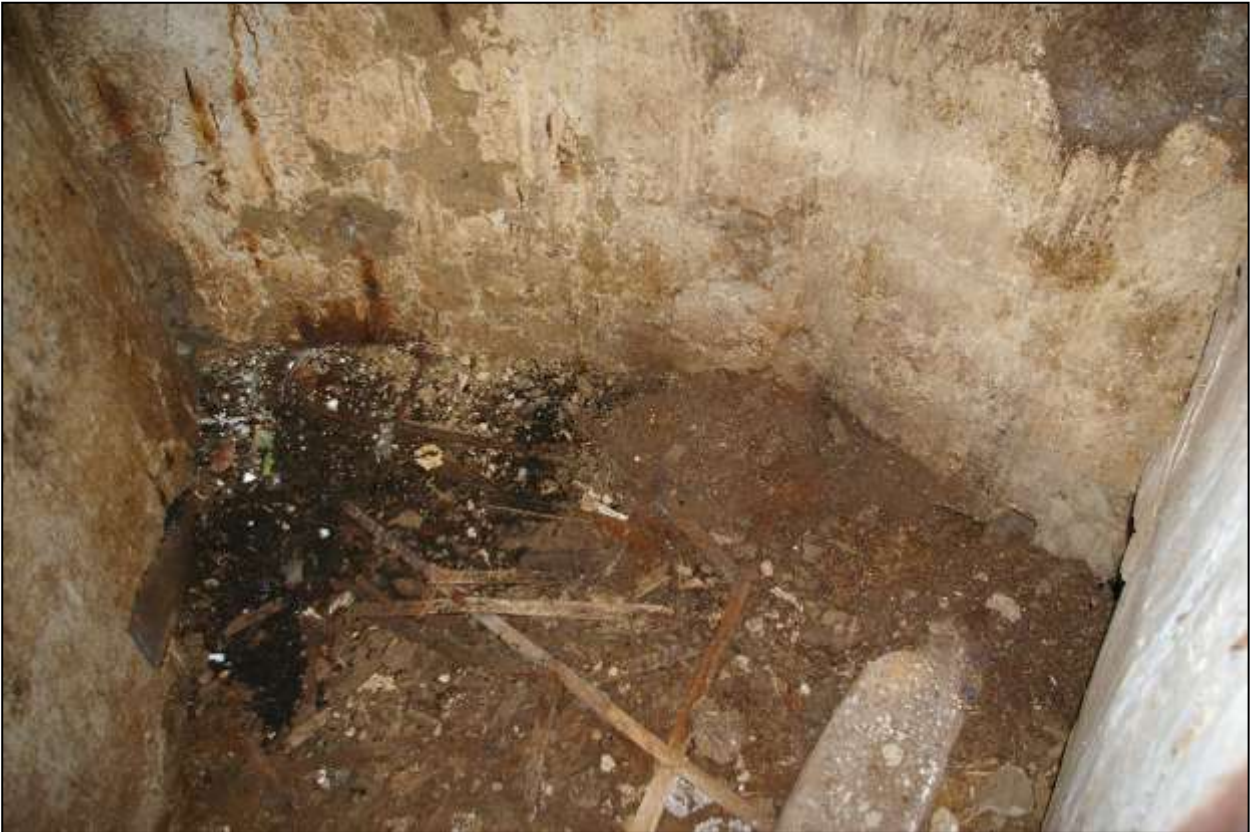
99. FLOOR OF CUPBOARD IN FORMER STAIR ALCOVE; VIEWED FROM THE NORTH-EAST.
