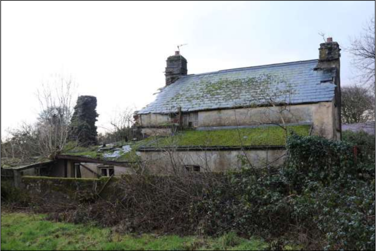
17. GENERAL VIEW OF REAR OF HOUSE; VIEWED FROM THE NORTH-WEST.
