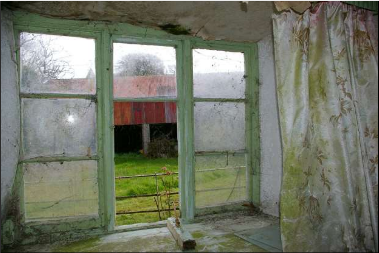
77. THE 19 TH CENTURY THREE-LIGHT CASEMENT WINDOW (W3) IN THE SOUTH WALL OF R3, OVERLOOKING THE YARD TO THE SOUTH; VIEWED FROM THE NORTH.
