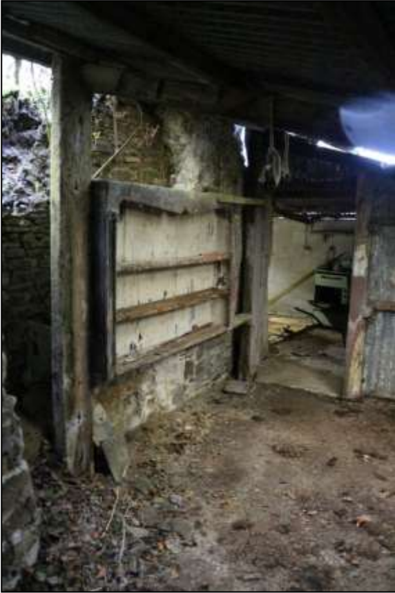
42. LEFT: THE NORTH-EAST CORNER OF R1; VIEWED FROM THE SOUTH.
