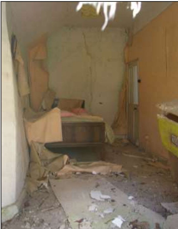
126. LEFT: R13, LOOKING NORTH-EAST WITH STAIR ALCOVE JUST VISIBLE TO LEFT.
