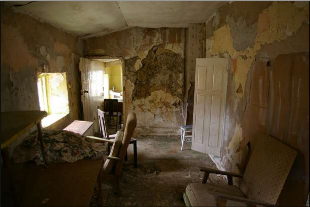
101. R5; VIEWED FROM THE SOUTH-WEST.
