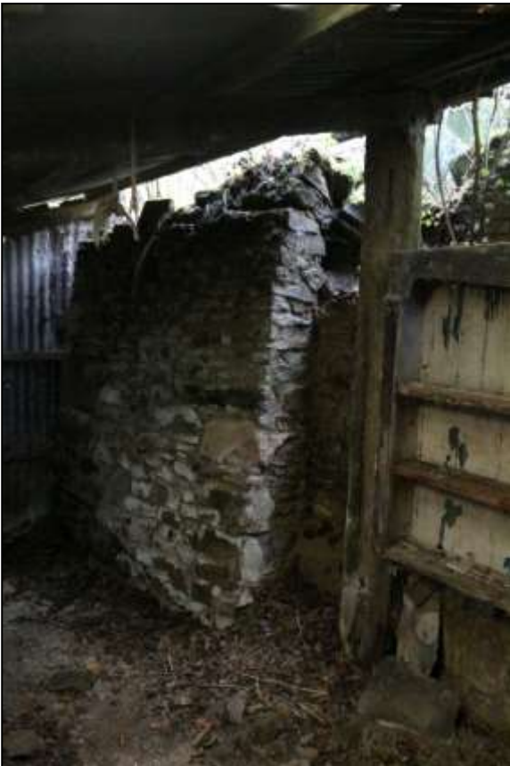
41. RUBBLE BUTTRESS BUILT AGAINST THE NORTH-EAST GABLE; VIEWED FROM THE NORTH.
