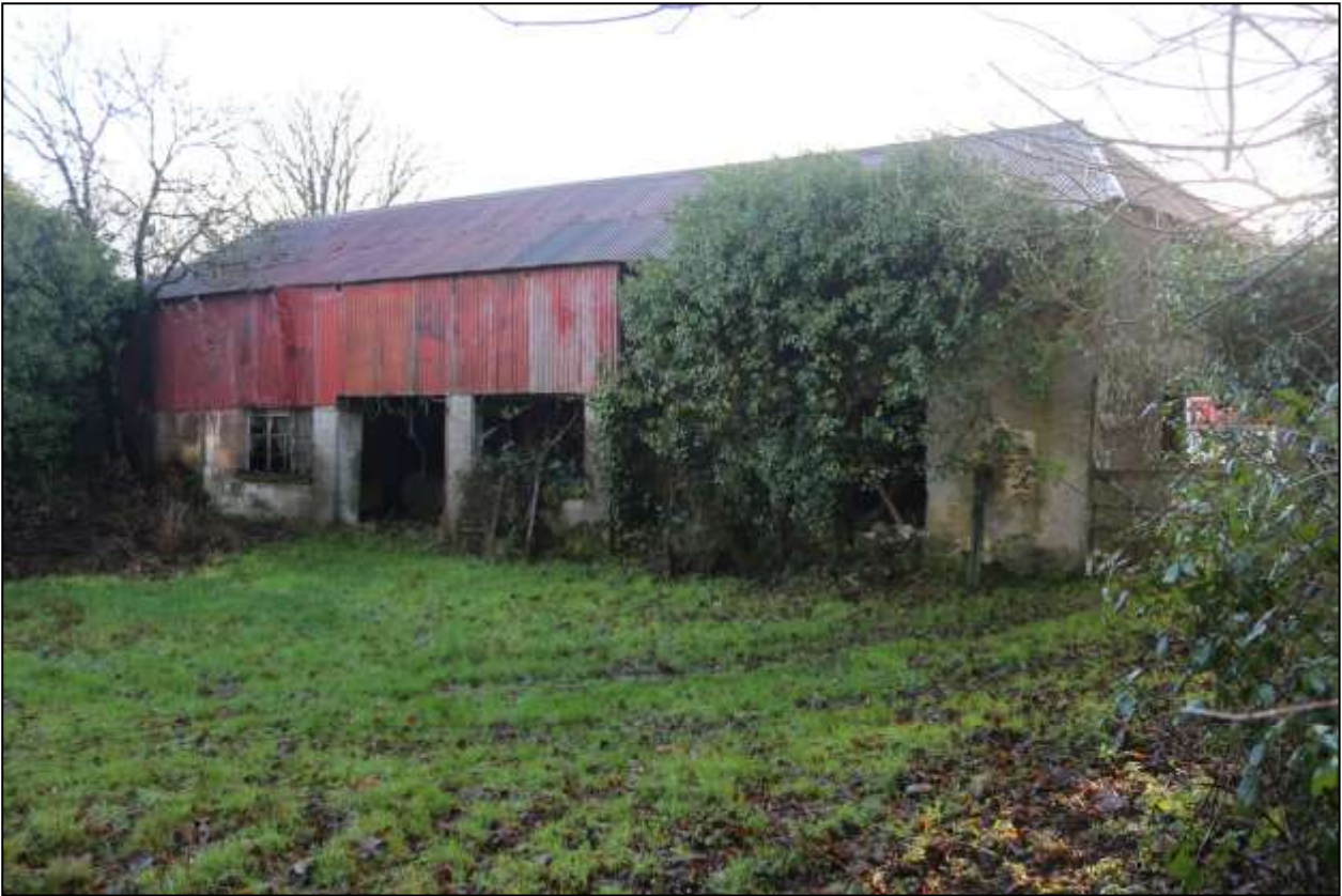
128. LINHAY RANGE ALONG THE ROAD. RUBBLE AND COB CONSTRUCTION; FRONTAGE REBUILT IN MID-20 TH CENTURY. VIEWED FROM THE NORTH-WEST.
