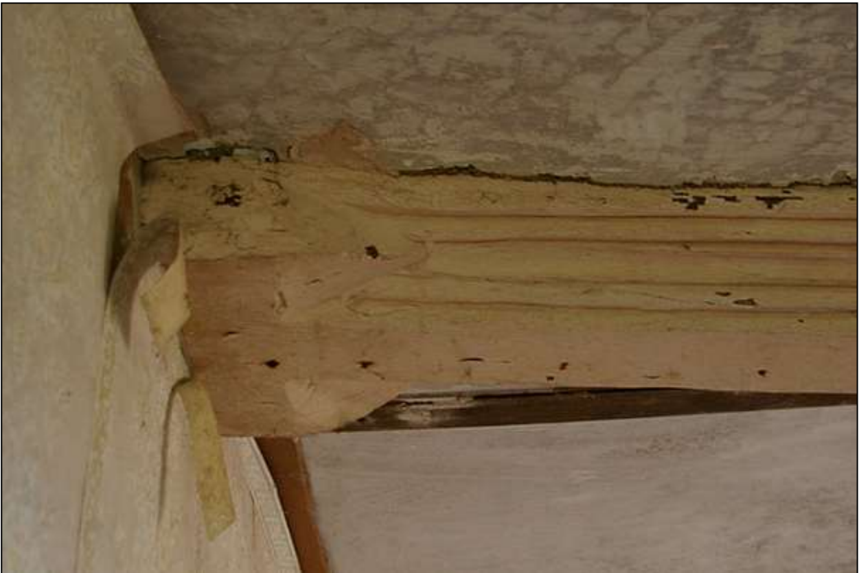
80. DETAIL OF THE PYRAMIDAL STOP ENDS ON THE NORTHERN CARVED BEAM IN R3, LOOKING NORTH-WEST.
