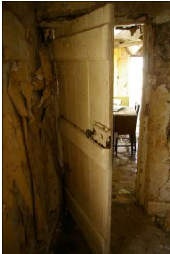
102. LEFT: VIEW OF THE BLOCKED DOOR (BO3) TO R3 IN R5, NOW USED AS A CUPBOARD, WITH RESET RAISED AND FIELDDED LATER 17 TH OR EARLY 18 TH CENTURY SHUTTERS. VIEWED FROM THE WEST
