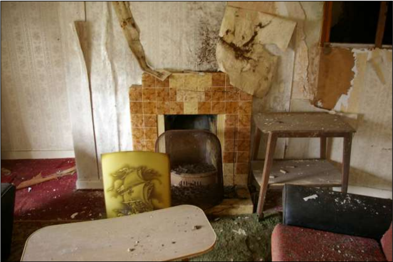
88. R4, 1950s tiled fireplace fronting older blocked fireplace (FP3); viewed from the north-east.
