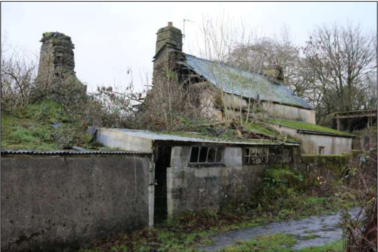
12. DETAIL OF ABOVE; VIEWED FROM THE NNE.
