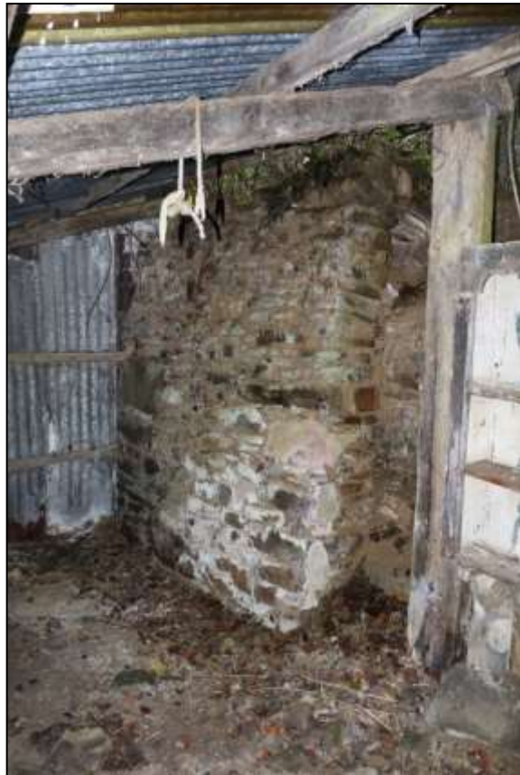
41. RUBBLE BUTTRESS BUILT AGAINST THE NORTH-EAST GABLE; VIEWED FROM THE NORTH.
