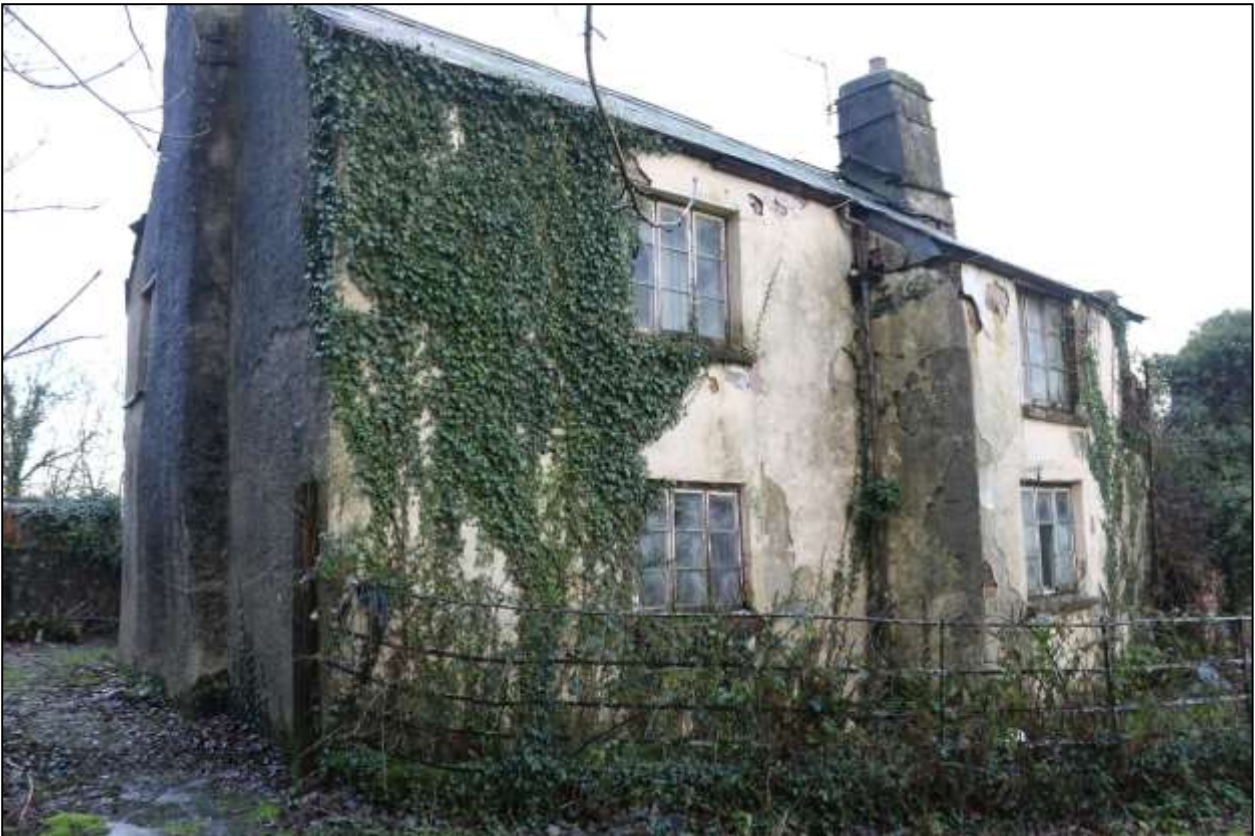
2. SOUTH-EAST ELEVATION OF R4 WITH 'HALL PROJECTION' FRONTING R3 TO RIGHT. NOTE RAISED SLATE WEATHERINGS ON EARLIER CHIMNEY FOR THATCHED ROOF. VIEWED FROM THE SOUTH.
