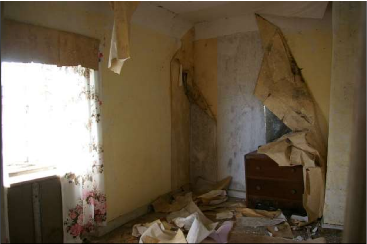
123. R12; VIEWED FROM THE NORTH-EAST.
