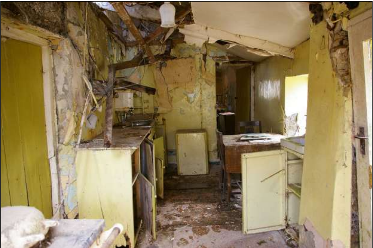
107. R6; VIEWED FROM THE NORTH-EAST.
