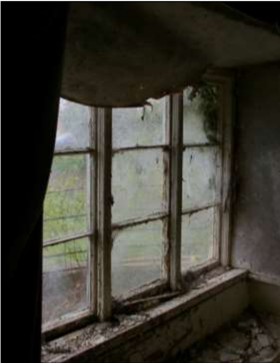
94. 19 TH CENTURY THREE-LIGHT CASEMENT WINDOW (W4) IN SOUTH WALL OF R4; VIEWED FROM THE NORTH-EAST.
