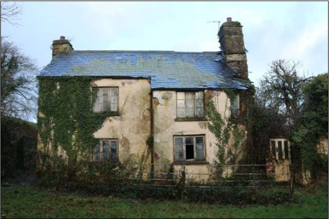
3. SOUTH-EAST ELEVATION OF ROOFED PART OF HOUSE, WITH 'HALL PROJECTION' TO RIGHT OF CENTRE AND CROSS-PASSAGE FRONT DOOR; VIEWED FROM THE SOUTH-EAST.
