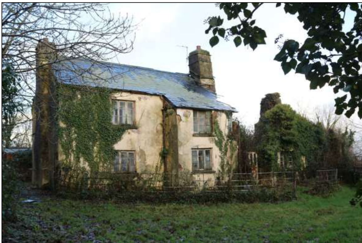
FIGURE 7: THE FRONT ELEVATION OF THE FARMHOUSE AT TOWN BARTON; VIEWED FROM THE SOUTH.
