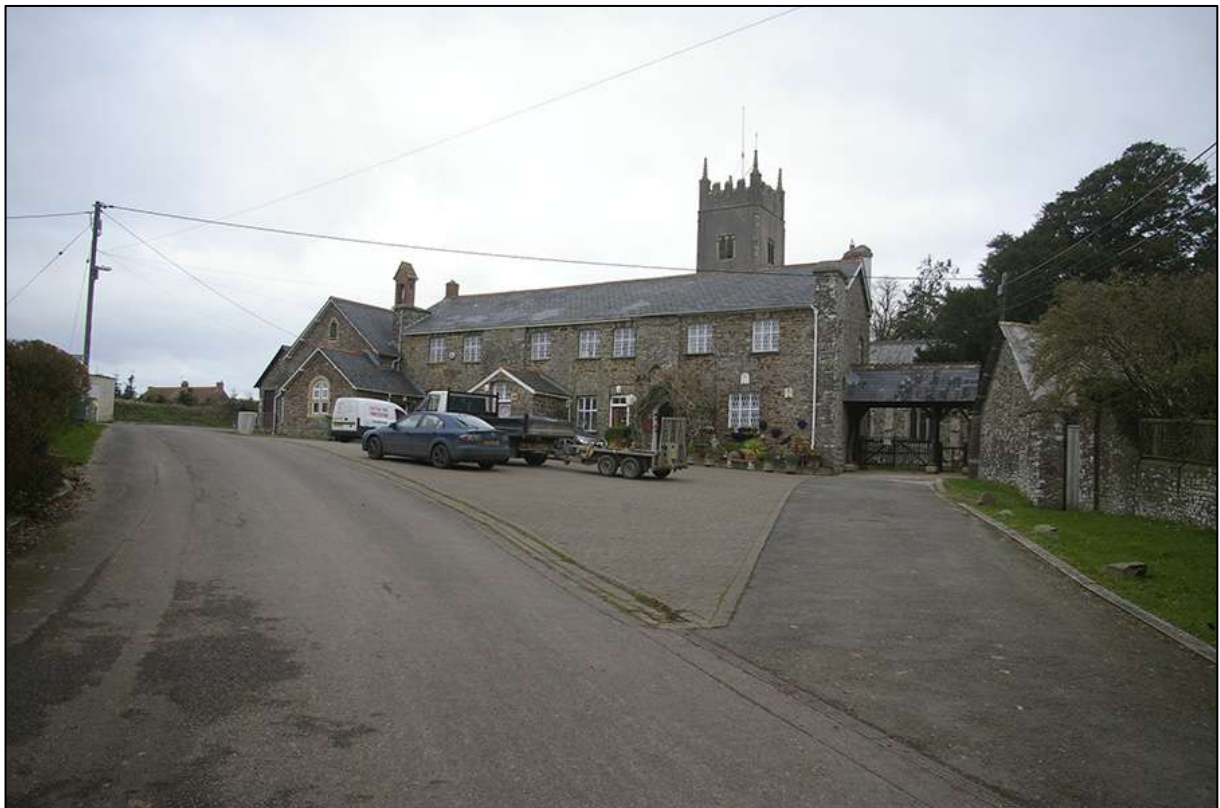
12. VIEW OF ST JAMES'S CHURCH; VIEWED FROM THE SOUTH-SOUTH-EAST (NO SCALE).
