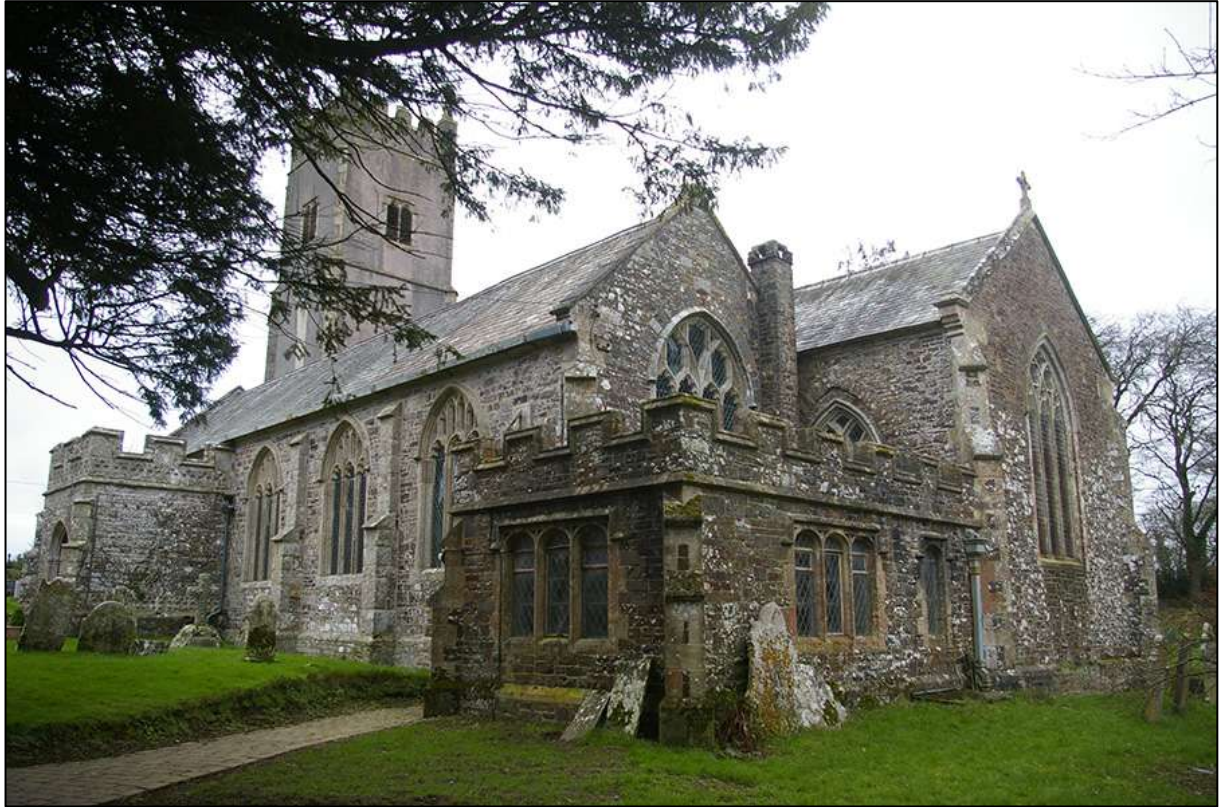
13. VIEW OF ST JAMES'S CHURCH; VIEWED FROM THE SOUTH-EAST (NO SCALE).
