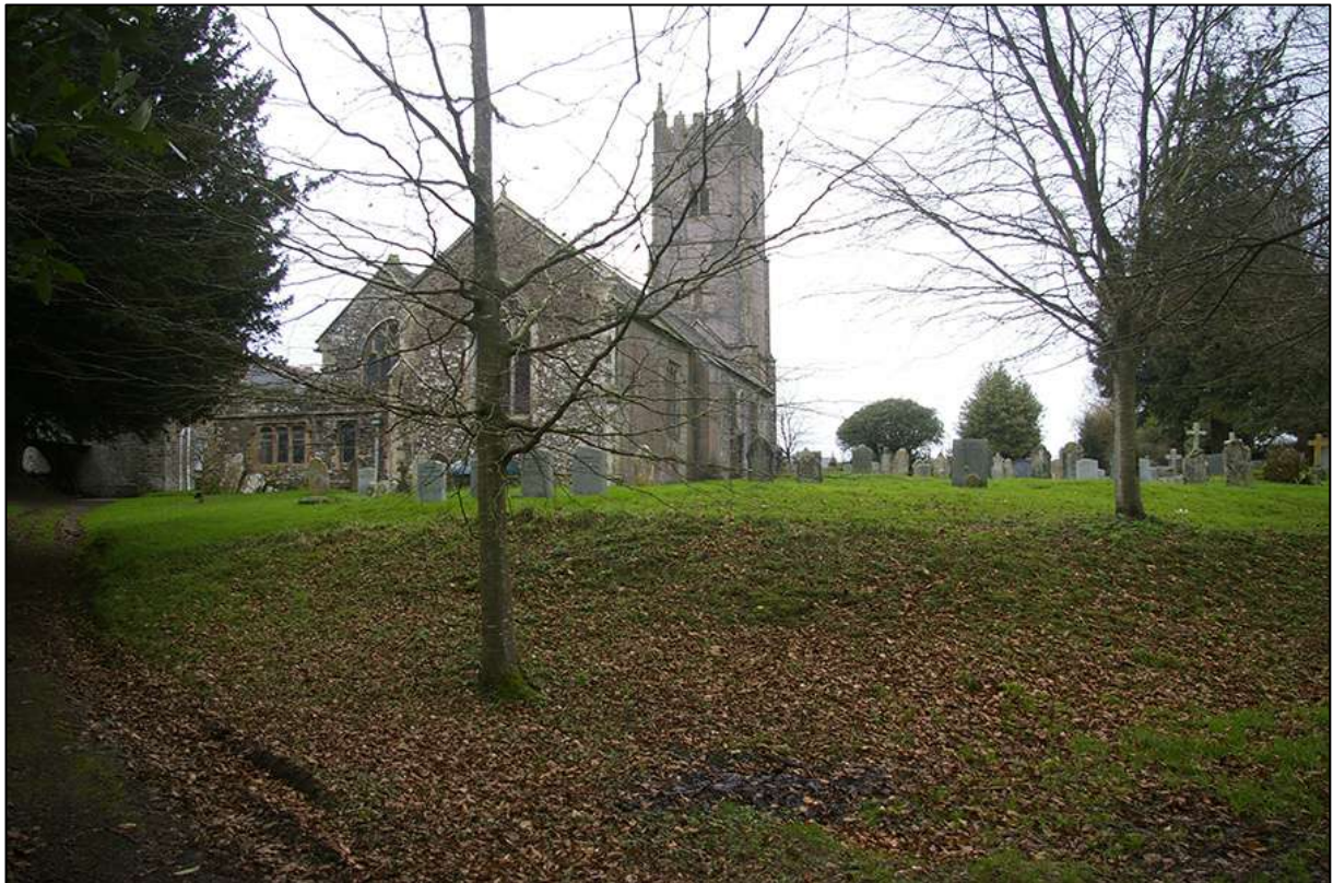
14. VIEW OF ST JAMES'S CHURCH; VIEWED FROM THE NORTH-EAST (NO SCALE).
