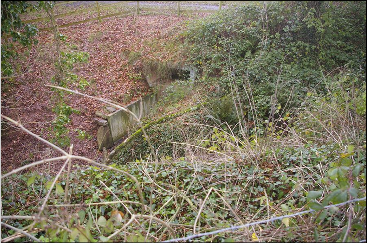
15. VIEW ACROSS LARGE/DEEP DRAIN ALONG THE SOUTH-WEST BOUNDARY OF THE SITE, SHOWING AN ADIT FROM THE ADJACENT CLAY PIT TO THE WEST; VIEWED FROM THE EAST (NO SCALE).
