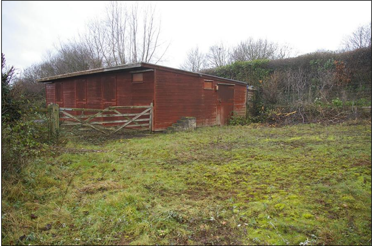
27. THE STABLE ALONG THE NORTH-WEST BOUNDARY OF THE SITE; VIEWED FROM THE EAST (NO SCALE).
