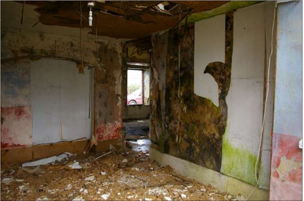
50. ROOM 4, THE NORTH WALL WITH SHALLOW BASKET ARCHED ALCOVE WITH BEAD MOULDING AND EAST PARTITION; FROM THE SOUTH-WEST.
