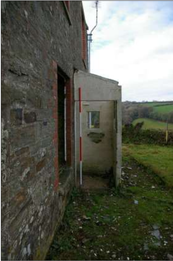
12. LEFT: THE REAR PORCH TO THE NORTH ELEVATION, CONCRETE BLOCK, 2M SCALE; FROM THE EAST. 13. RIGHT: THE EAST ELEVATION, BOTH THE EXTENSION AND HOUSE, WITH LARGE HISTORIC STACK TO SOUTH AND CAPPED NARROWER STACK TO NORTH EXTENSION, WITH 2M SCALE; FROM THE NORTH-EAST.
