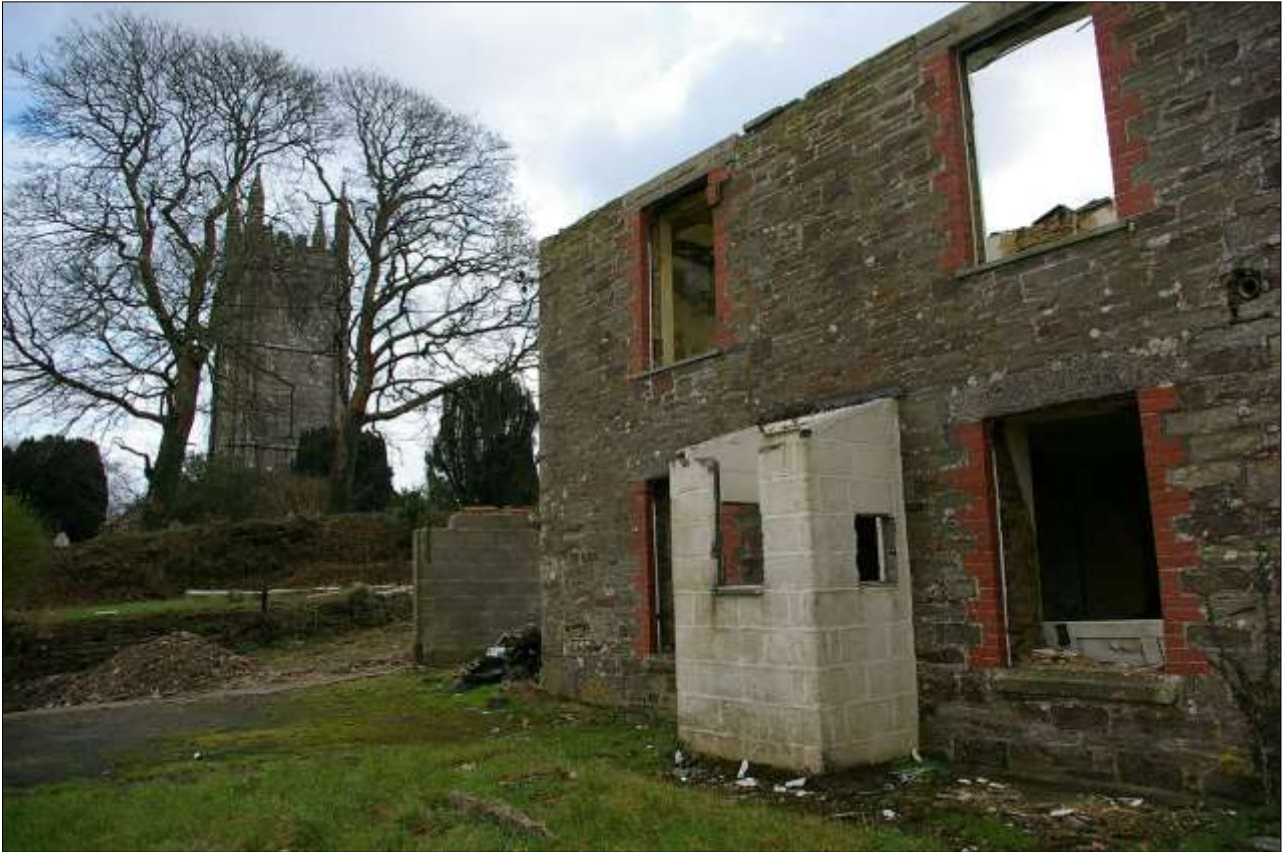
5. THE HOUSE AND CHURCH FROM THE NORTH-WEST, SHOWING SETTING.
