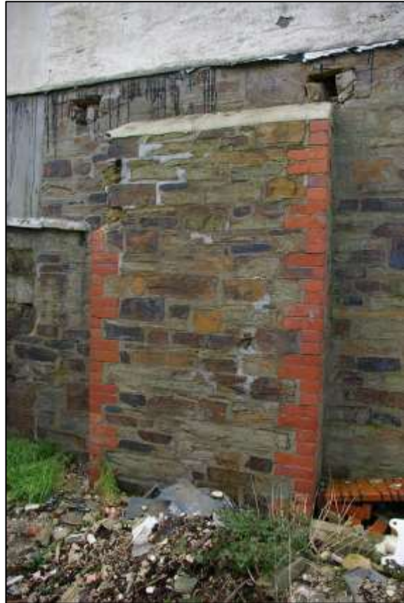
14. LEFT: DETAIL OF THE LARGE STACK TO THE MAIN HOUSE, WITH 2M SCALE; FROM THE NORTH-EAST. 15. RIGHT: THE RECENTLY CAPPED STACK WITH BRICK AND CEMENT REPAIRS, TO THE 19TH CENTURY EXTENSION, TO THE EAST, NORTH-EAST.
