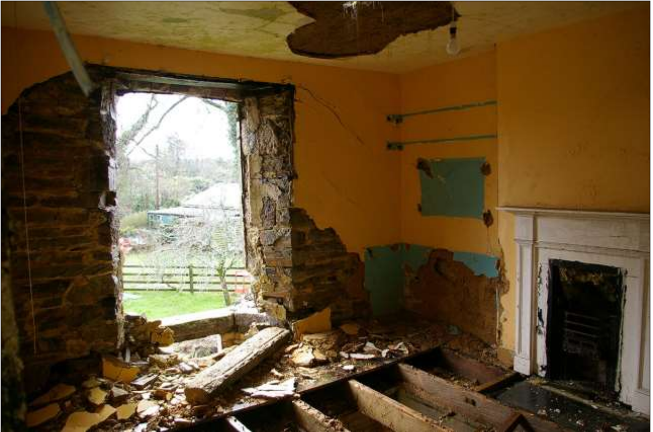
71. THE SOUTH WALL OF ROOM 10, THE WINDOW WITH COLLAPSED STONE CARVED SILL, SHALLOW SLOPING SIDES; FROM THE NORTH-EAST.
