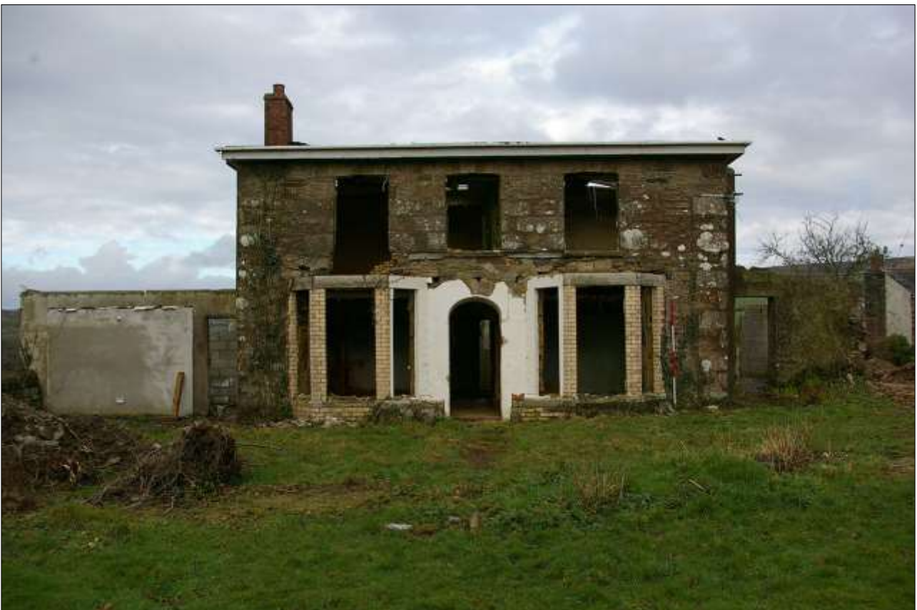
19. THE SOUTH ELEVATION OF THE HOUSE, WITH BAY WINDOWS AND CONCRETE EXTENSION TO THE WEST AND STONE RUBBLE LEAN-TO TO THE EAST, WITH 2M SCALE; FROM THE SOUTH.
