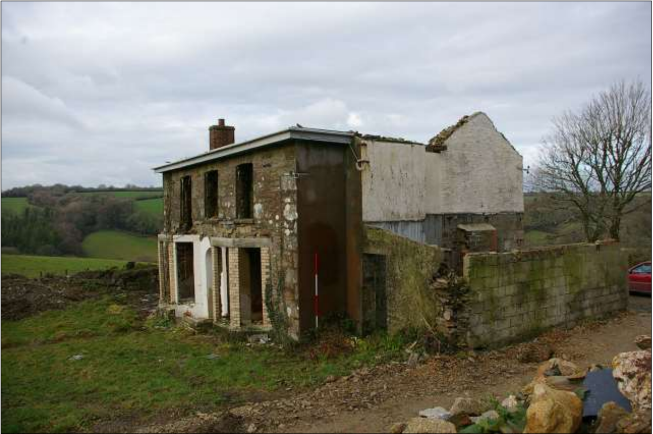
18. THE HOUSE, FROM THE SOUTH-EAST, WITH 2M SCALE.
