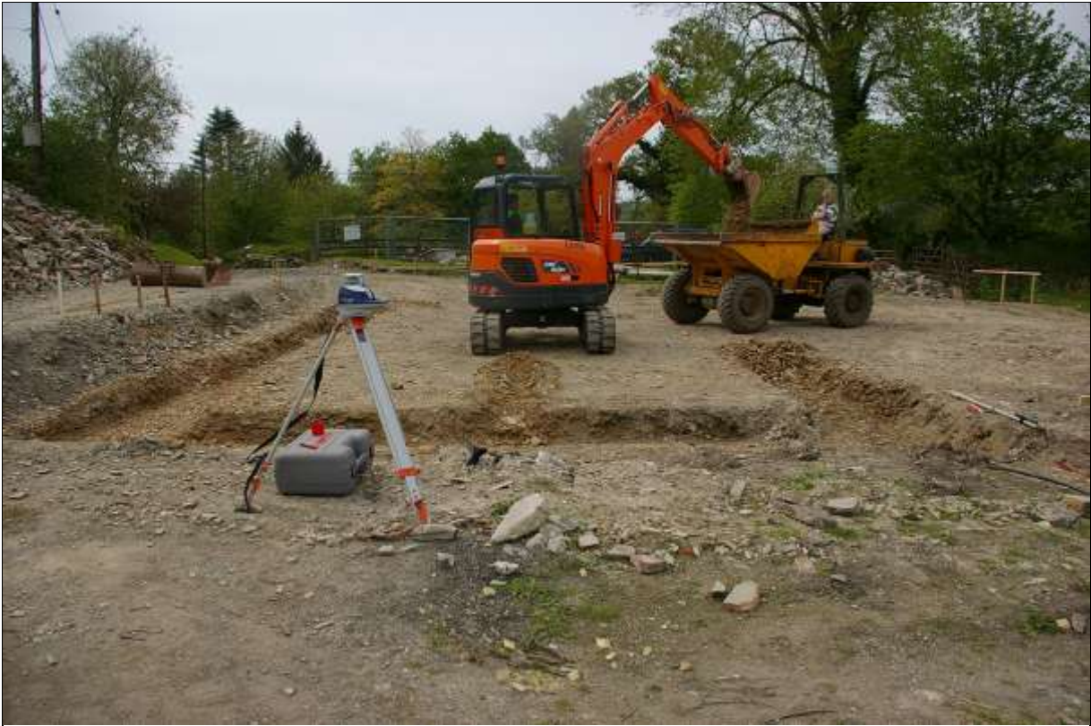
1. THE SITE; FROM THE NORTH DURING MONITORING OF THE FOUNDATION TRENCHES.
