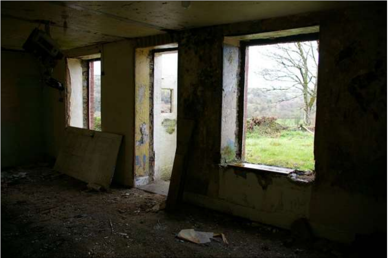
58. THE NORTH WALL OF ROOM 6, WITH TWO WINDOWS, BEAD MOULDED STRAIGHT EDGED OPENINGS, THE CENTRAL DOORWAY IS ALSO BEAD MOULDED TO EDGE; FROM THE SOUTH-EAST.
