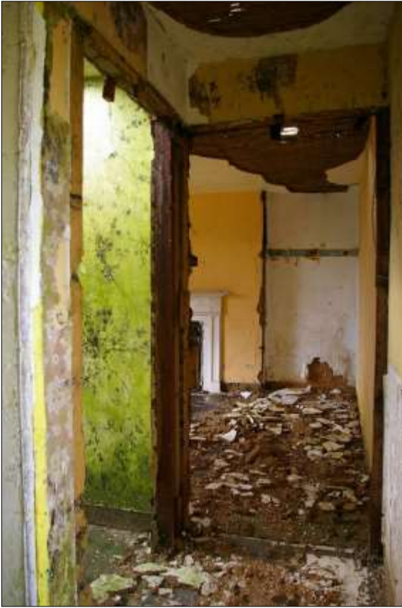
68. LEFT: THE SMALL EXTENSION TO THE LANDING, FORMED WITHIN ROOM 10, BY THE CREATION OF ROOM 9 BY LATHE AND PLASTER PARTITIONS; FROM THE EAST, NORTH-EAST. 69. RIGHT: ROOM 9, A SMALL POSSIBLE FORMER BATHROOM FORMED WITHIN ROOM 10 OVER THE HALLWAY; FROM THE NORTH.
