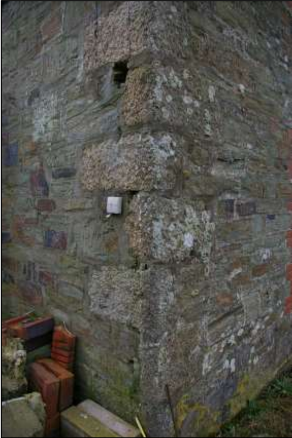
9. LEFT: THE GRANITE BLOCK QUOINS, ROUGHLY DRESSED WHICH TO THE CORNERS OF THE HOUSE. 10. RIGHT: THE WEST ELEVATION, BOTH THE EXTENSION AND HOUSE, WITH BRICK SHAFT TO HOUSE AND CONCRETE BLOCK SINGLE STOREY EXTENSIONS; FROM THE NORTH-WEST.
