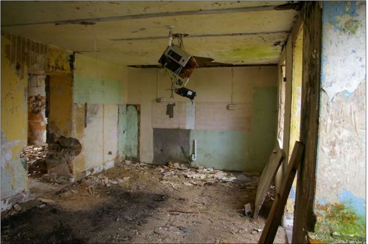
56. ROOM 6; FROM THE NORTH-EAST.
