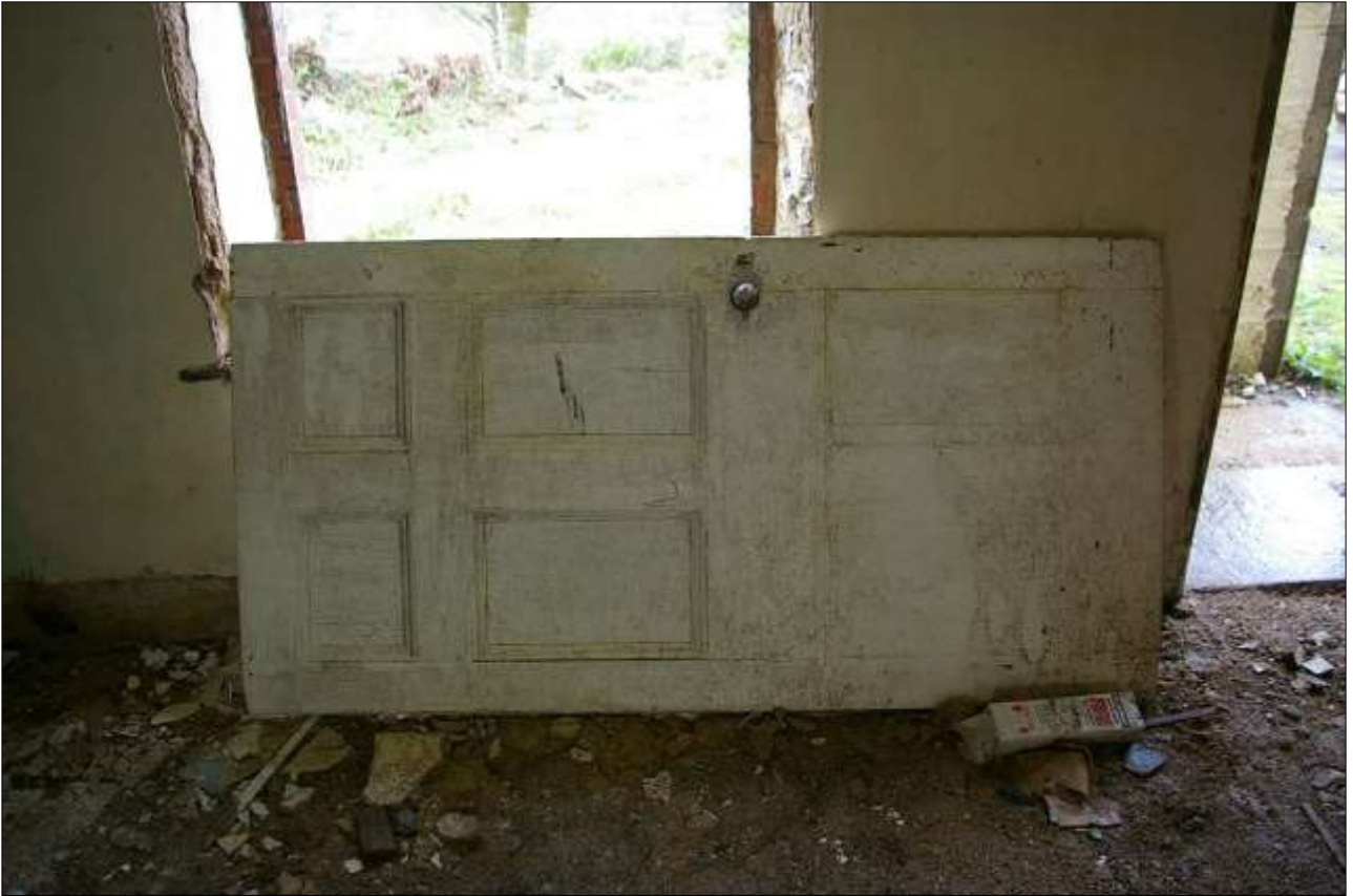
52. THE FRONT DOOR, SIX PANEL OGEE MOULDED; FROM THE SOUTH.
