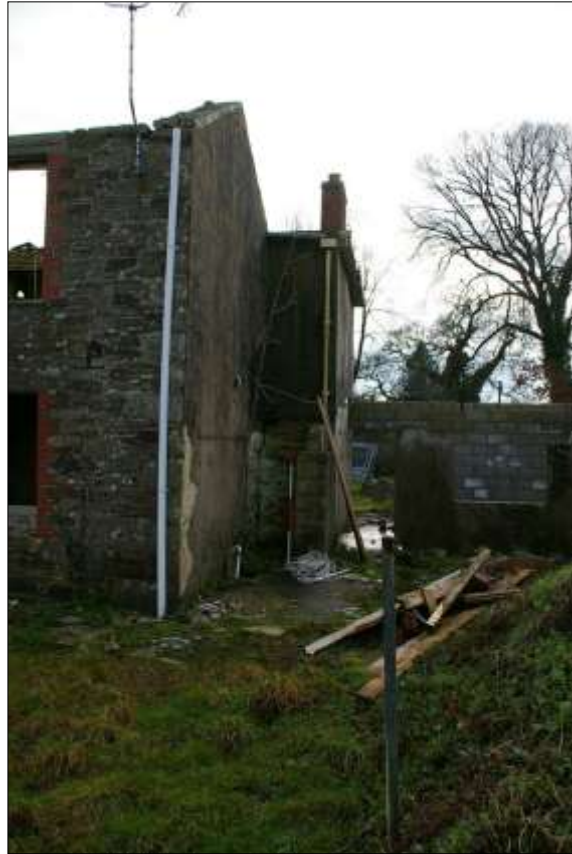
9. LEFT: THE GRANITE BLOCK QUOINS, ROUGHLY DRESSED WHICH TO THE CORNERS OF THE HOUSE. 10. RIGHT: THE WEST ELEVATION, BOTH THE EXTENSION AND HOUSE, WITH BRICK SHAFT TO HOUSE AND CONCRETE BLOCK SINGLE STOREY EXTENSIONS; FROM THE NORTH-WEST.
