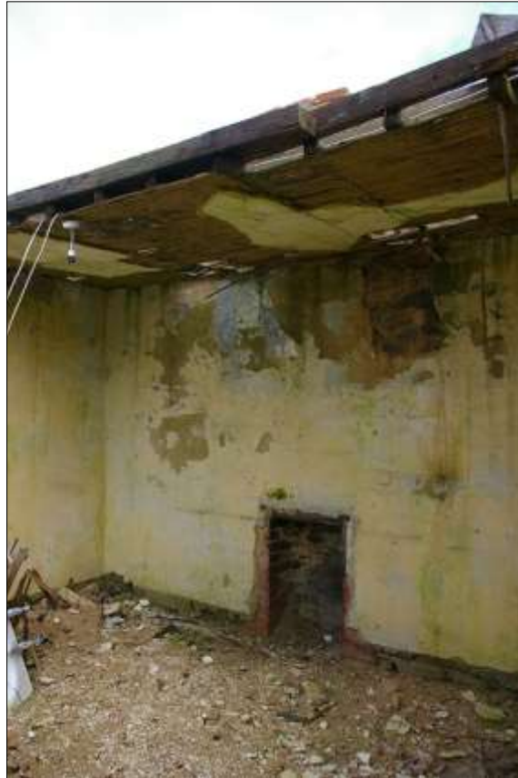
75. THE EAST WALL OF ROOM 11, WITH BRICK LINED HEARTH WITH ROUNDED FIREBACK, QUITE INDICATIVE OF THE 19TH CENTURY; FROM THE SOUTH-WEST.
