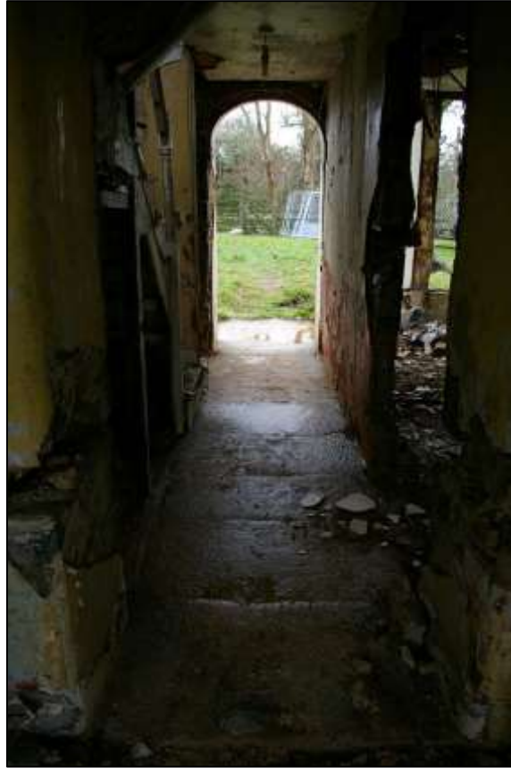
38. THE ENTRANCE HALLWAY, ROOM 2; FROM THE NORTH.
