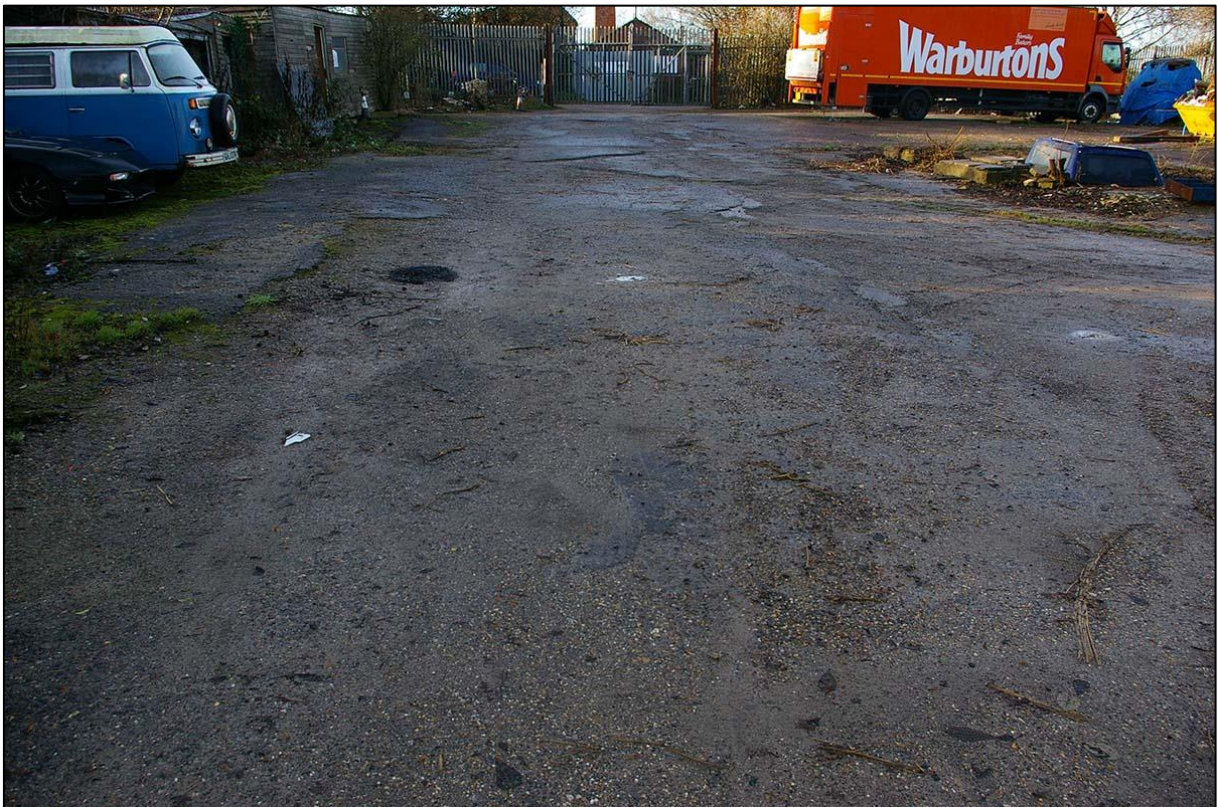
THE HARD CORED GROUND IN THE WESTERN ENCLOSURE, WITH PATCHES OF TARMAC AND CONCRETE, SHOWING SIGNS OF RESURFACING; VIEWED FROM THE EAST.
