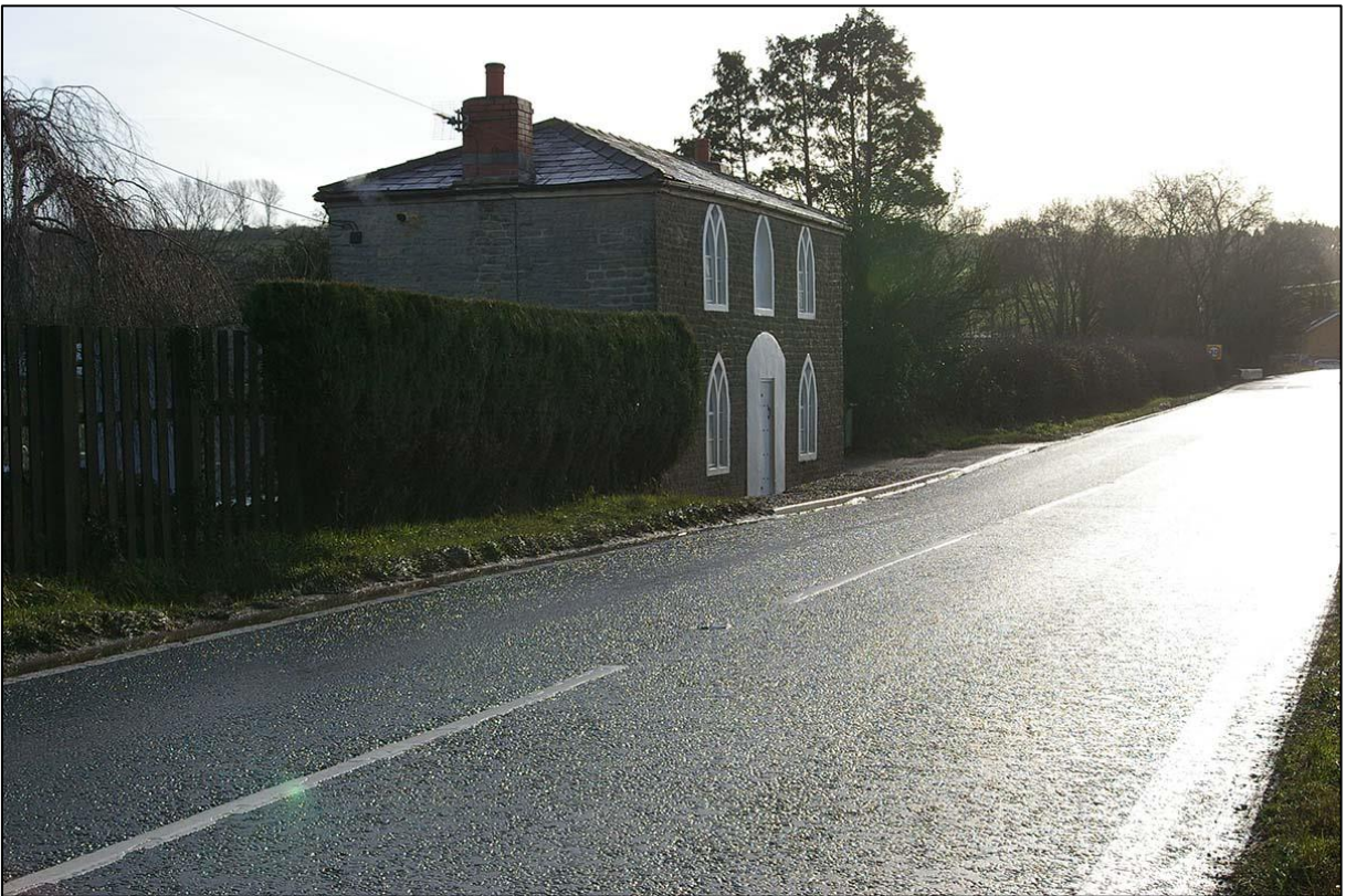
THE LISTED TOLLHOUSE JUST ALONG THE ROAD FROM THE PROPOSED SITE, WITH FINE GOTHIC WINDOWS; VIEWED FROM THE NORTH-WEST.
