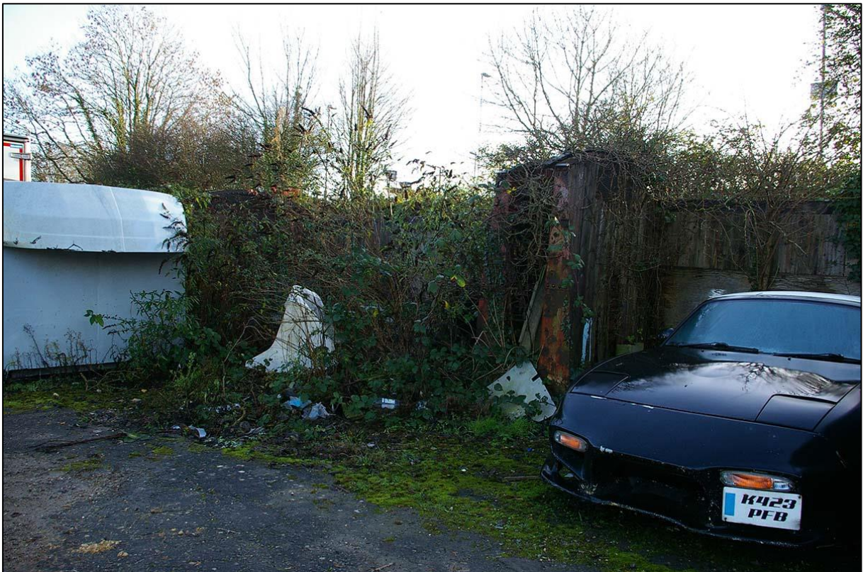
THE TWO CARRIAGES WHICH HAVE LOST THEIR ROOFS; VIEWED FROM THE NORTH-WEST.
