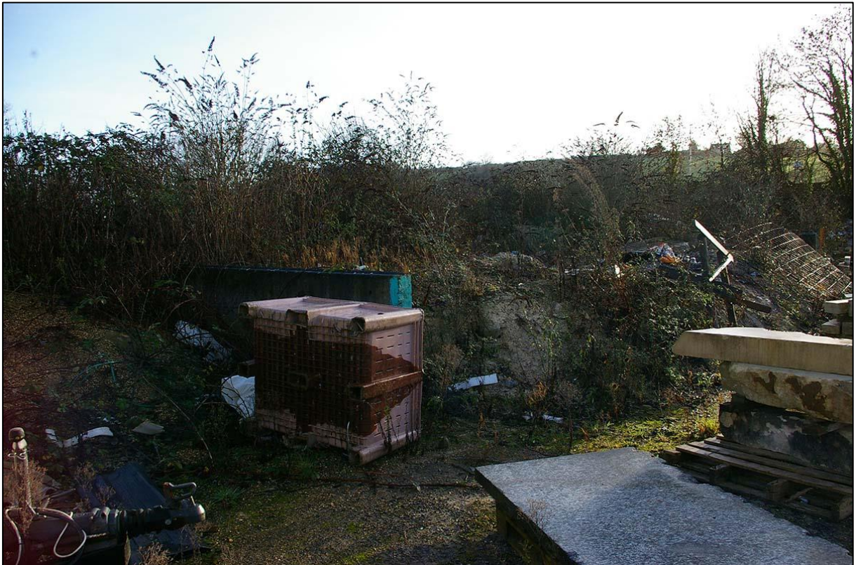
VIEW OF THE CONCRETE 'SILOS' WITH GRIT AND SAND DEPOSITS; VIEWED FROM THE NORTH-WEST.
