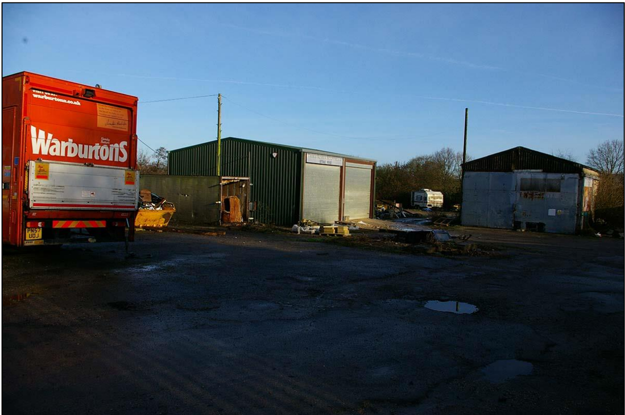
THE BUILDINGS TO THE CENTRE AND NORTH OF THE SITE; VIEWED FROM THE SOUTH-WEST.
