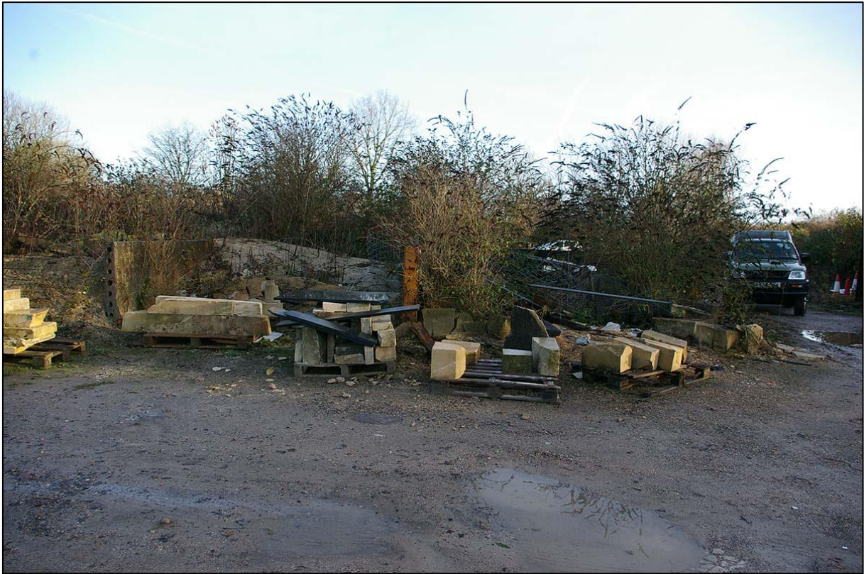
SOME OF THE CONCRETE 'SILOS' HOLDING SAND AND GRIT; VIEWED FROM THE WEST.
