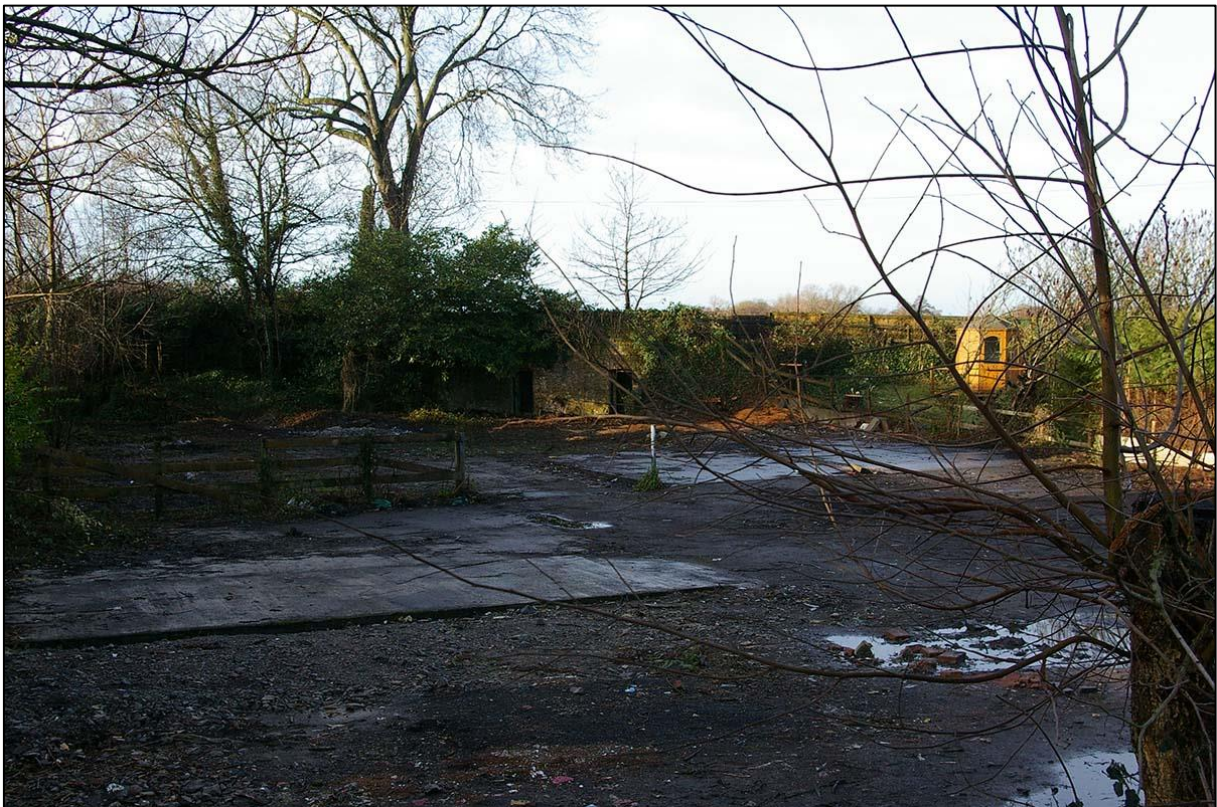
A CLEARED YARD BETWEEN THE RAILWAY COTTAGE AND FACTORY; VIEWED FROM THE EAST.
