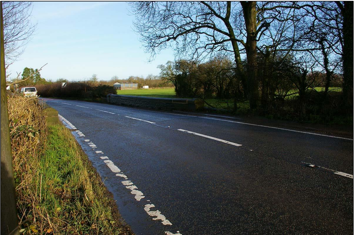
ANSFORD BRIDGE; VIEWED FROM THE SOUTH-WEST.
