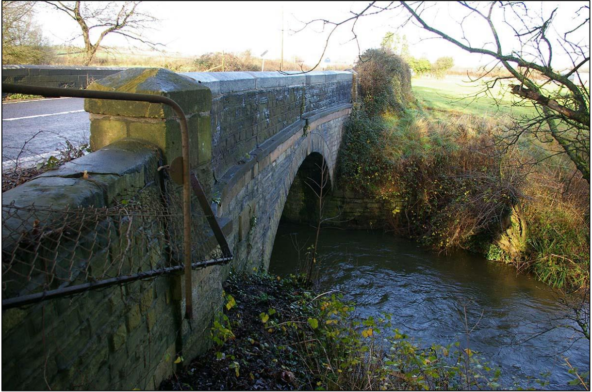
MORE DETAILED VIEW OF ANSFORD BRIDGE; VIEWED FROM THE SOUTH-EAST.
