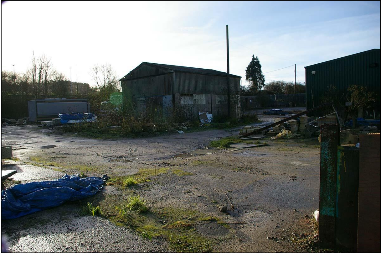
VIEW ACROSS THE WESTERN ENCLOSURE, SHOWING THE CONCRETE AND METAL FRAMED BUILDING AND SMALLER MORE MODERN BUILDING TO THE NORTH; VIEWED FROM THE NORTH-EAST.
