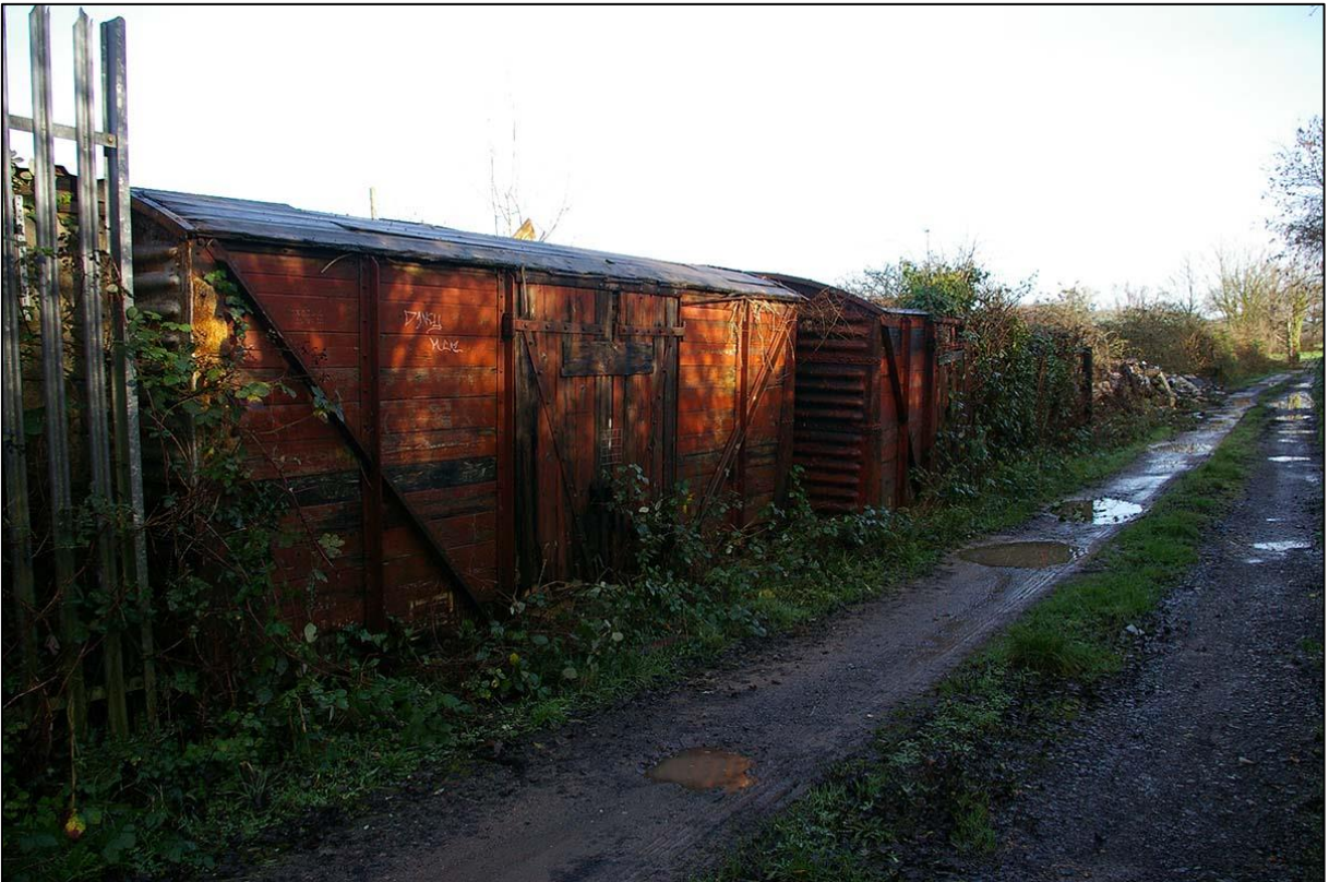
VIEW OF THE THREE HISTORIC WOODEN AND IRON FREIGHT CARRIAGES, WHICH FORM THE SOUTH BOUNDARY OF THE WESTERN PART OF THE SITE; VIEWED FROM THE WEST-SOUTH-WEST.
