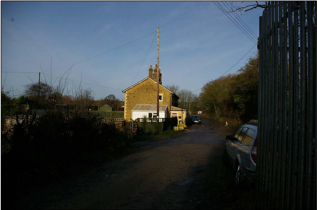
THE RAILWAY COTTAGES; VIEWED FROM THE SOUTH-SOUTH-EAST.
