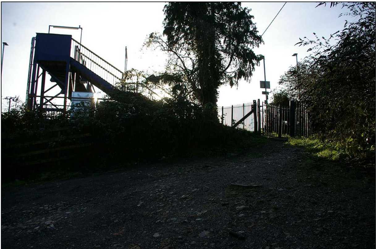
VIEW OF THE BANK, WITH THE GATE TO THE PLATFORM AND THE OVERBRIDGE AT THE STATION; VIEWED FROM THE NORTH.
