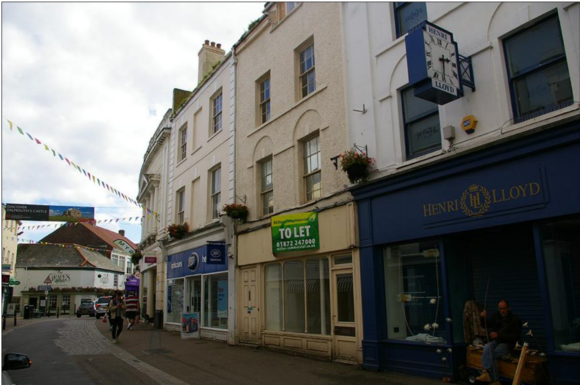
15. VIEW ALONG MARKET STREET SHOWING NOS. 26, 27, AND 27A WHICH BACK ONTO LAND TO THE REAR OF THE SITE; VIEWED FROM THE NORTH-WEST.
