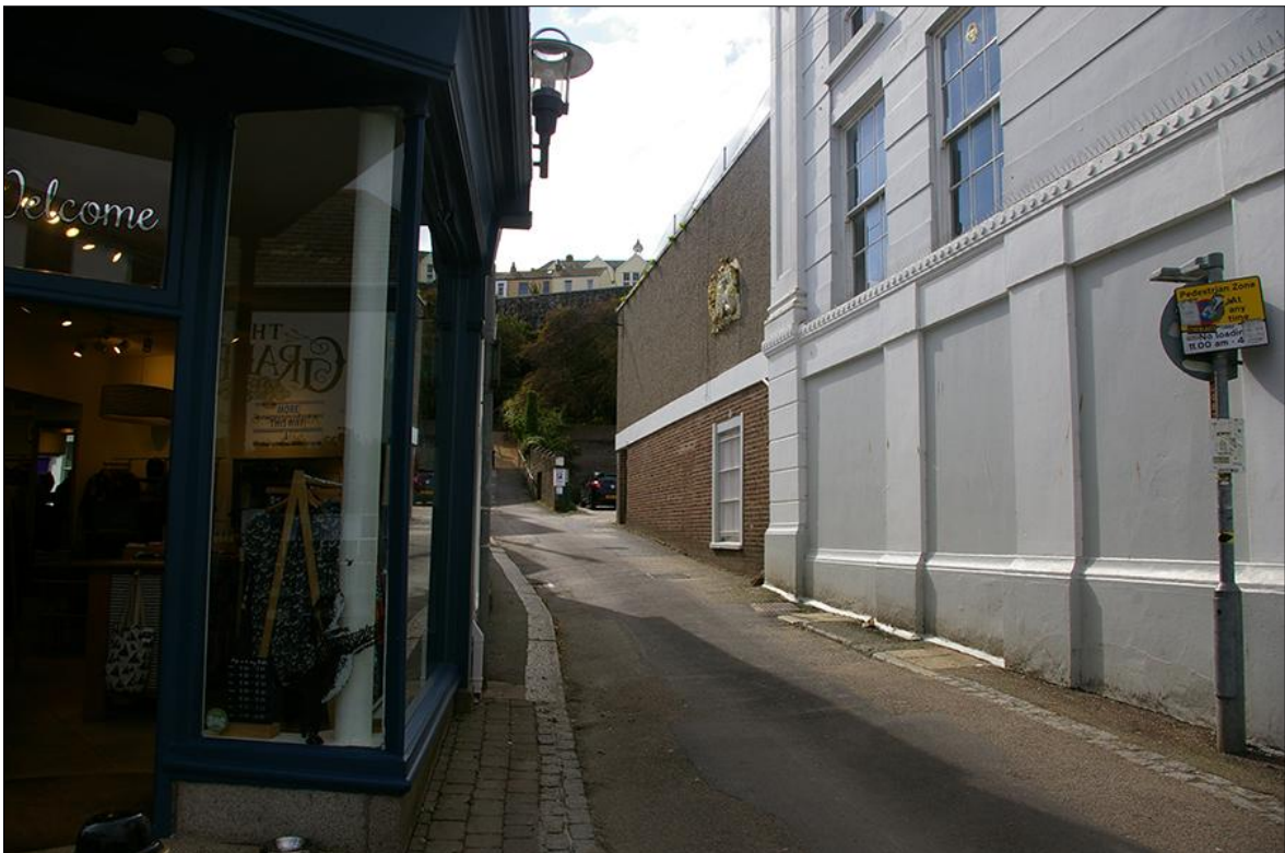
16. VIEW FROM MARKET STREET LOOKING ALONG FISH STRAND HILL, SHOWING SMITHICK HILL TERRACED INTO THE HILL IN THE BACKGROUND, DEMONSTRATING THE EXISTING LOCALISED SCREENING; VIEWED FROM THE NORTH-EAST.
