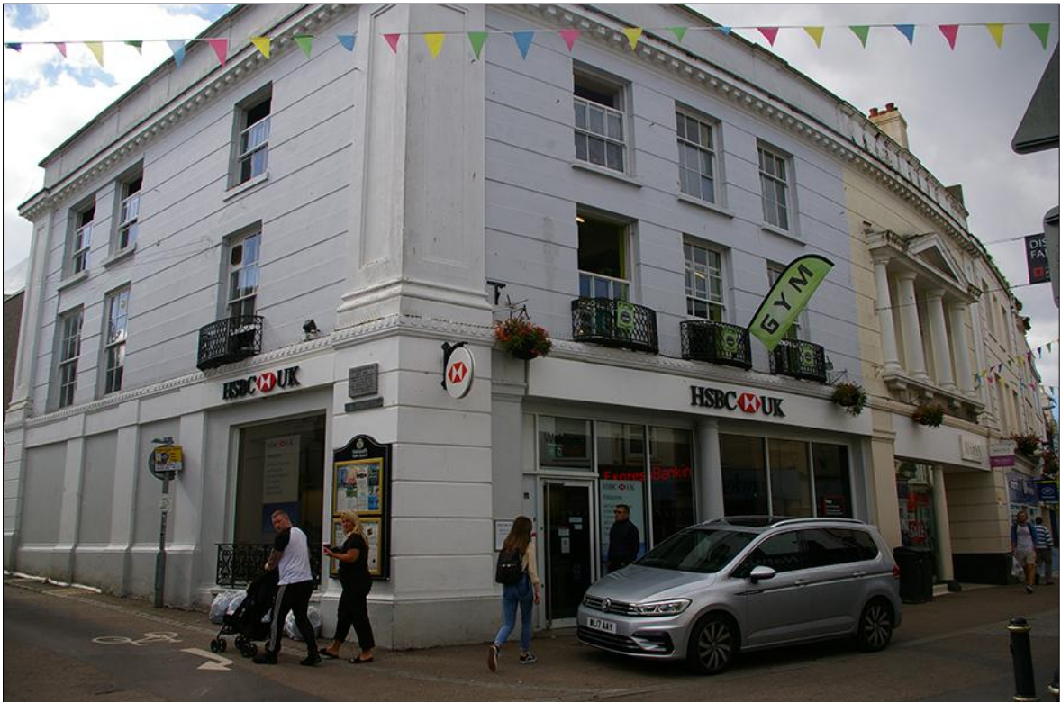
14. VIEW OF THE FORMER ROYAL HOTEL SHOWING IS GRANDIOSE STYLE AND MODERN ALTERATIONS; VIEWED FROM THE NORTH-EAST.
