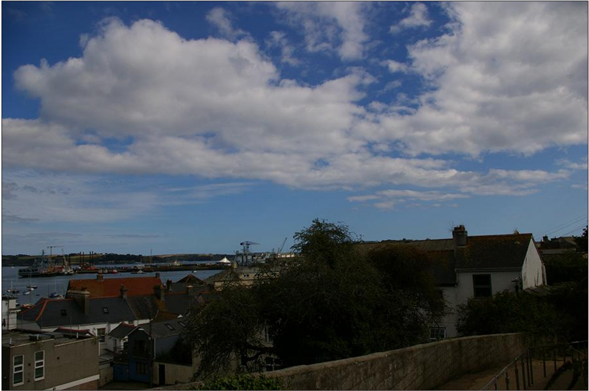
11. VIEW FROM SMITHICK HILL ACROSS FALMOUTH CONSERVATION AREA; VIEWED FROM THE WEST-SOUTH-WEST.
