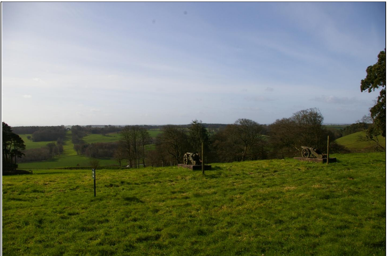
10. VIEW FROM THE SHAM CASTLE, LISTED GRADE II, ALONG THE AVENUE TO THE TRIUMPHAL ARCH. THE SITE IS ON THE RIGHT HAND SIDE, SHOWING THE EFFECTIVE EXISTING SCREENING; FROM THE NORTH-NORTH-EAST.
