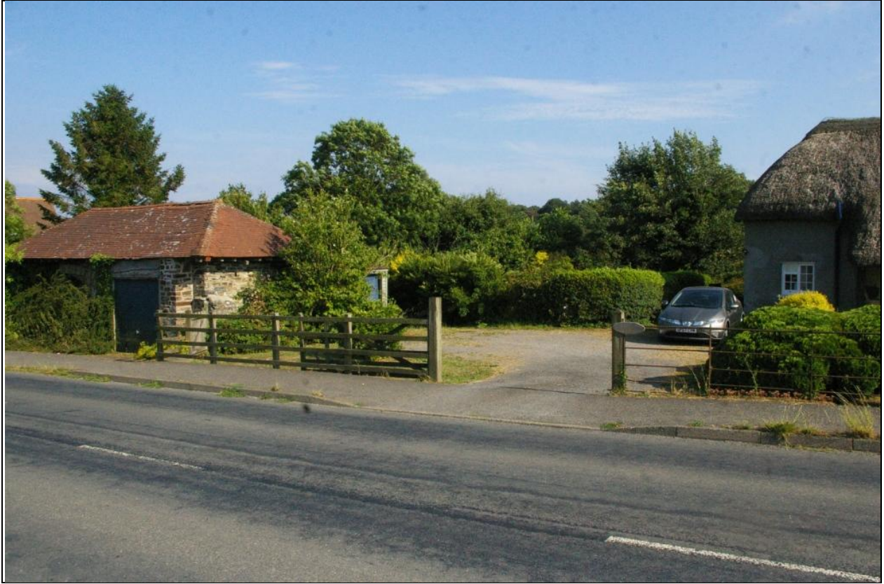
5. SHOT OF CURRENT ACCESS DRIVE TO PAYNES COTTAGES, THE PROPOSED SITE ACCESS, VIEWED FROM THE NORTH.
