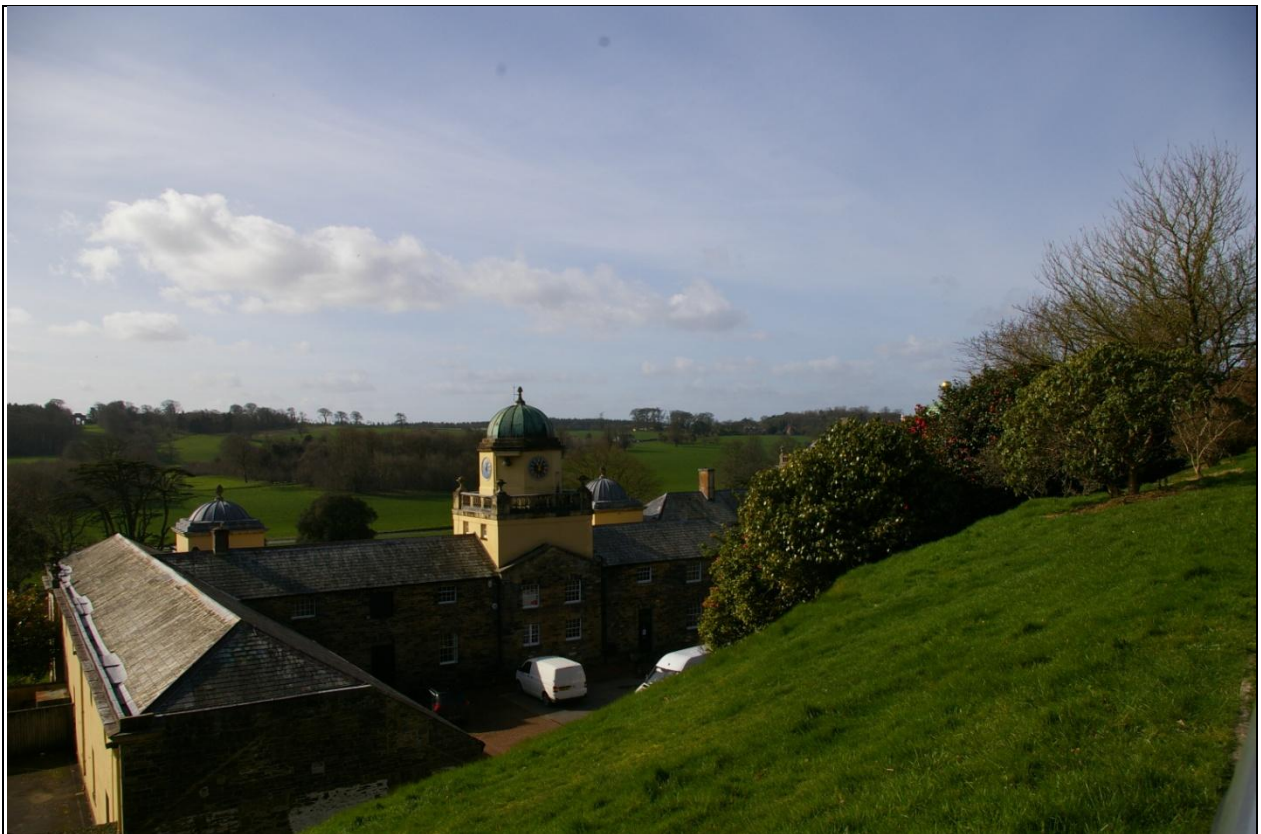
14. VIEW OVER THE ROOF OF CASTLE HILL HOUSE, GRADE II* LISTED ASSET AND STABLES COURTYARD ALSO GRADE II* LISTED IN FOREGROUND; FROM THE NORTH-EAST.
