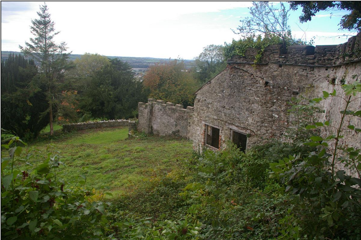
VIEW OF THE KITCHEN GARDEN WALLS TO THE EAST WITH SMALL INTEGRAL SHED AND EVIDENCE OF LOST GLASSHOUSES; FROM THE NORTH-NORTH-EAST.
