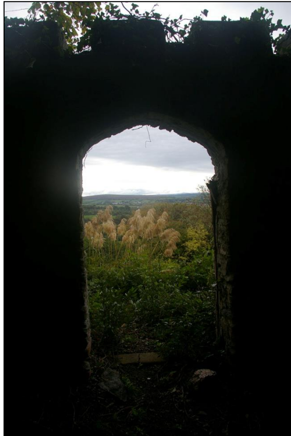
SHALLOW GOTHIC ARCHED DOORWAY INTO THE KITCHEN GARDEN FROM THE REAR PATHWAY; FROM THE NORTH.
