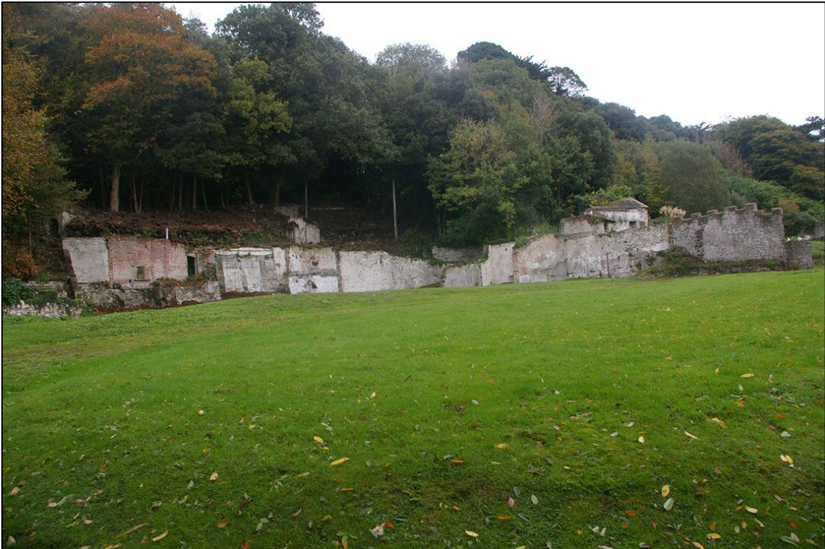
VIEW OF THE FORMER HOUSE'S LOCATION, NOW ALL THAT SURVIVES ARE THE EAST AND NORTH WALLS; FROM THE SOUTH-WEST.
