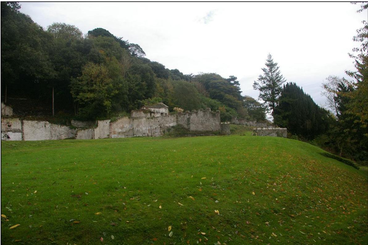
VIEW SHOWING THE CONSIDERABLE TERRACING AND MAN MADE SLOPES ON THE SITE TO ACCOMMODATE THE LARGE HOUSE AND CARRIAGE DRIVES ON A NATURALLY STEEP SLOPE FROM THE SOUTH-WEST.
