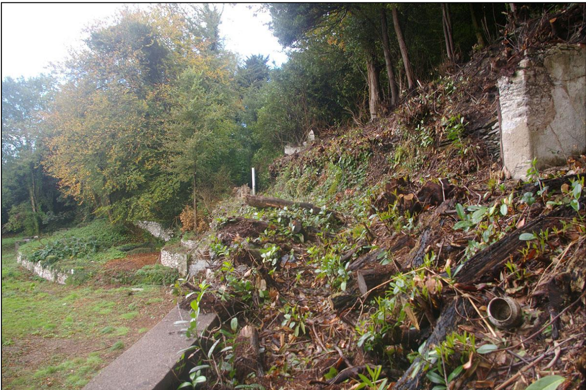
VIEW ALONG THE REAR TERRACE OF THE FORMER HOUSE; FROM THE EAST.
