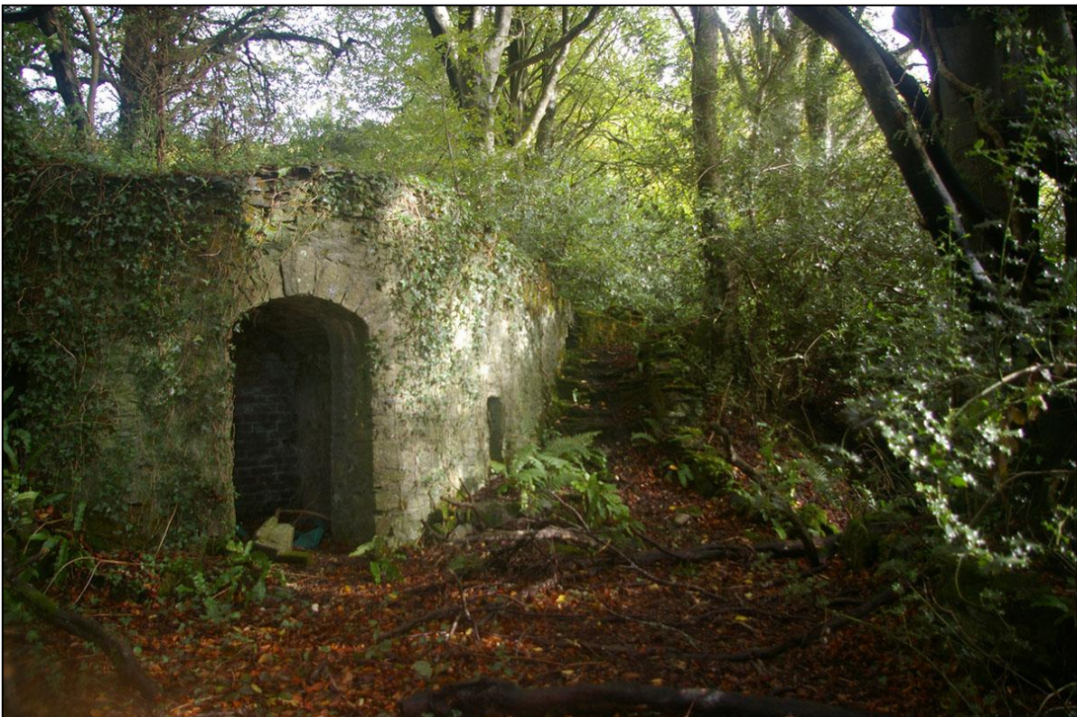
THE SET OF RUSTIC STEPS WHICH RUN DOWN THE SIDE OF THE SUMMERHOUSE AND ACCESS THE WALK UP TO THE FOLLY; FROM THE WEST.
