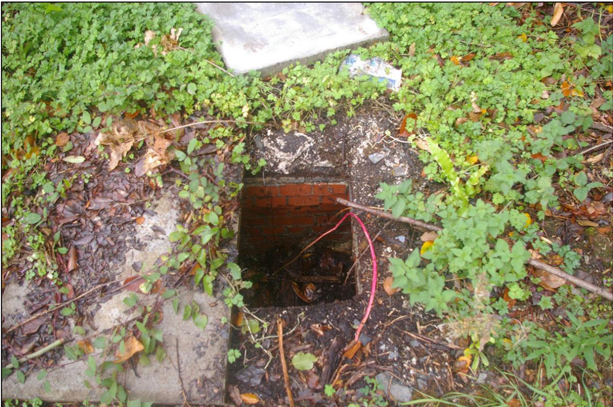
RELATIVELY MODERN BRICK DRAINS, IN QUITE GOOD CONDITION, SUGGESTING THE HOUSE WAS RAZED TO THE GROUND, BUT THAT FOUNDATIONS AND FLOORS COULD SURVIVE; FROM THE EAST.
