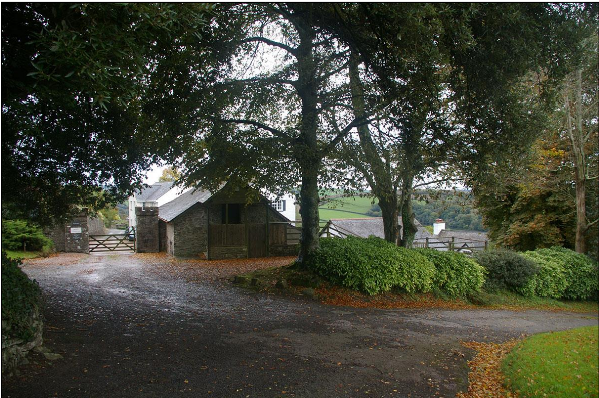
THE FORMER STABLES, COACH HOUSE AND KITCHEN GARDEN COURT, AS WELL AS THE HOME FARM; FROM THE WEST-NORTH-WEST.
