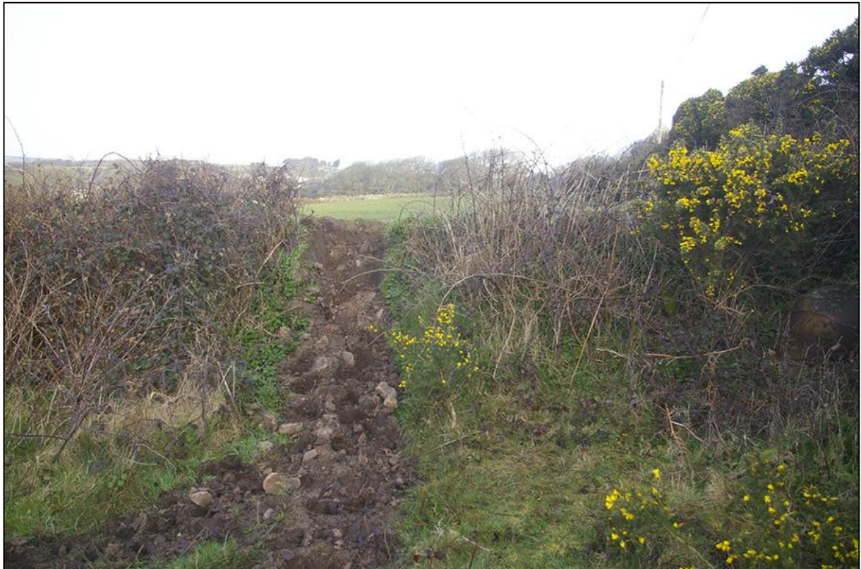
6. ERODED PART OF NORTHERN BOUNDARY AT ITS EAST END, NEAR THE ENTRANCE; VIEWED FROM THE SOUTH (NO SCALE).
