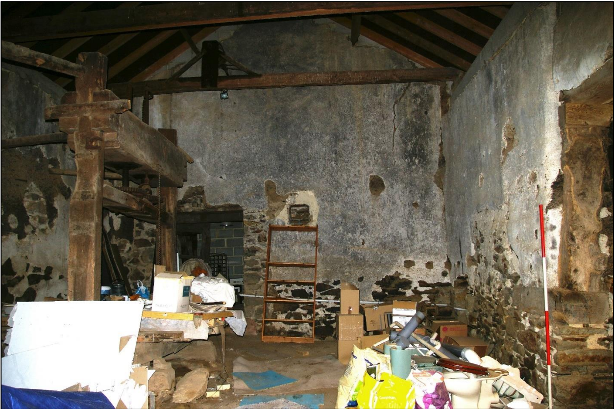
24. EAST END OF CIDER BARN, GENERAL VIEW FROM WEST.
