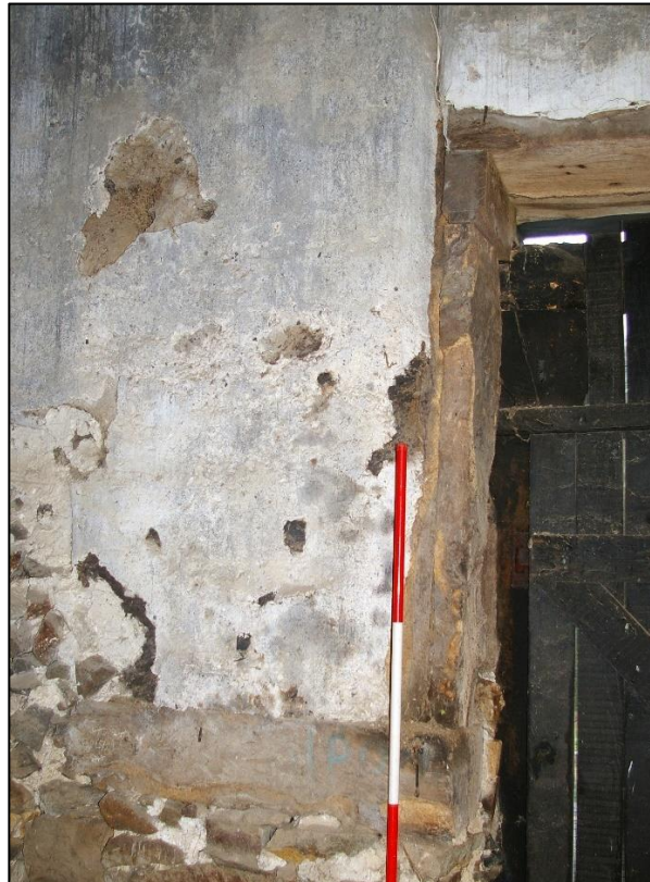
27. DETAIL OF EAST JAMB OF THRESHING DOOR, FROM NORTH.
