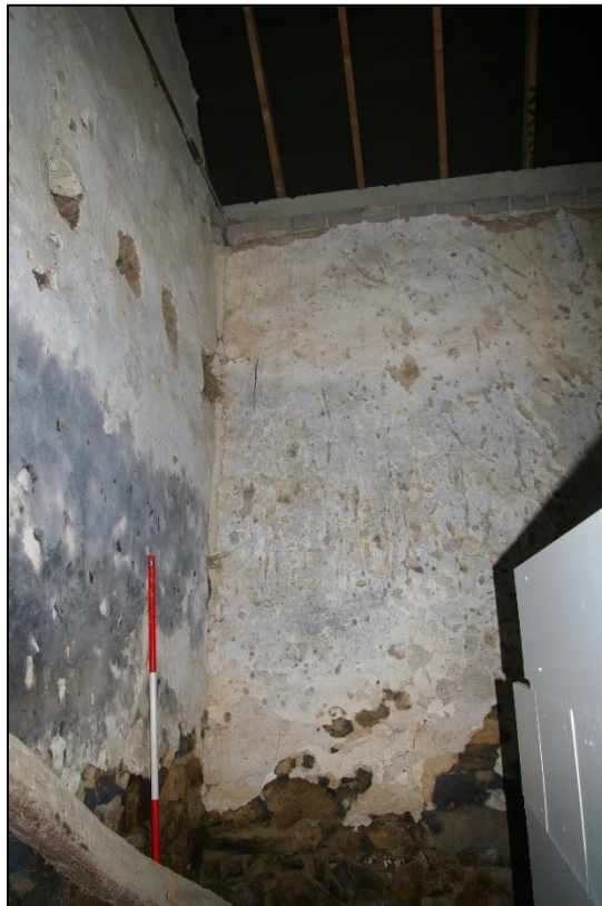
17. WESTERN BAY OF NORTH WALL, FROM SOUTH. NOTE EXTENSIVE PITCHFORK SCARS AND DAISY-WHEEL AT BOTTOM CENTRE.
