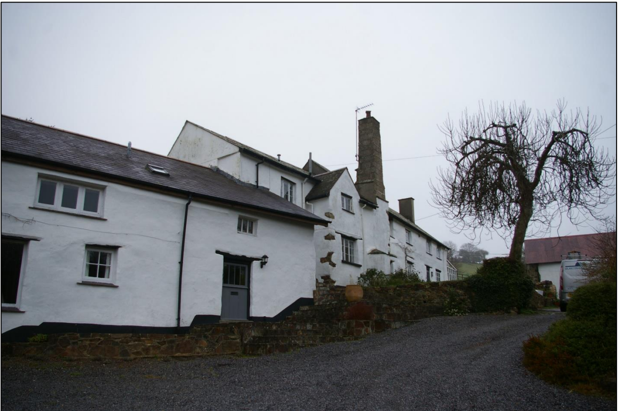
2. RELATIONSHIP OF POUND HOUSE (LEFT) ABUTTING FARM HOUSE AT A HIGHER LEVEL BEYOND. VIEW FROM SOUTH-WEST.
