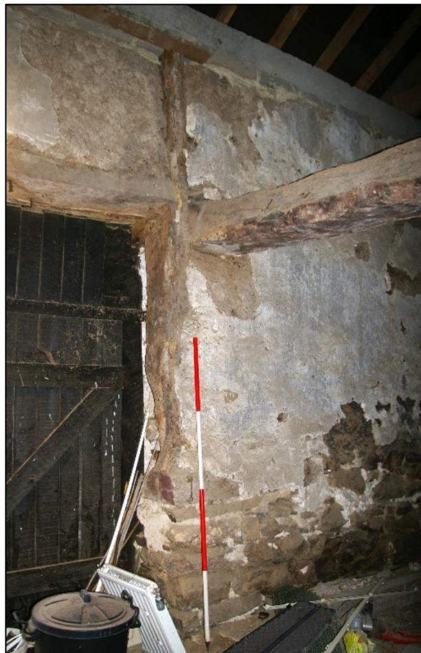
29. WEST JAMB OF THRESHING DOOR IN SOUTH WALL, FROM NORTH-EAST.
