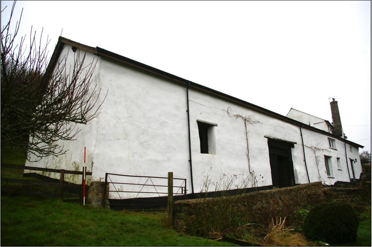
1. FRONT OF CIDER BARN FROM SOUTH-WEST, WITH POUND HOUSE BEYOND; FARM HOUSE RISES BEYOND.
