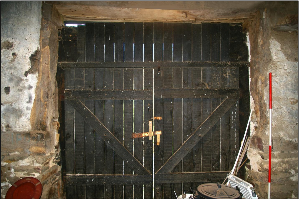
28. WIDE THRESHING DOOR IN SOUTH WALL, FROM NORTH. CHEEK-PIECES PEGGED TO INSIDE FACES OF CRUCK FEET ON EITHER SIDE.
