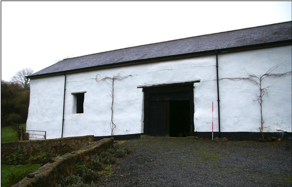
FIGURE 7: THE FRONT ELEVATION OF THE CIDER BARN WITH YARD WALL AND FIELD GATE TO LEFT; FROM THE SOUTH-EAST (2M SCALE).
