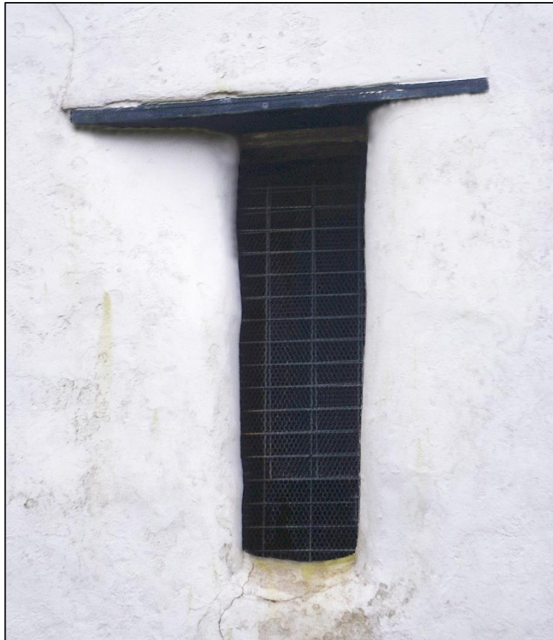
8. C15-C16 VENTILATION SLIT IN WEST GABLE OF BARN. VIEW FROM WEST.
