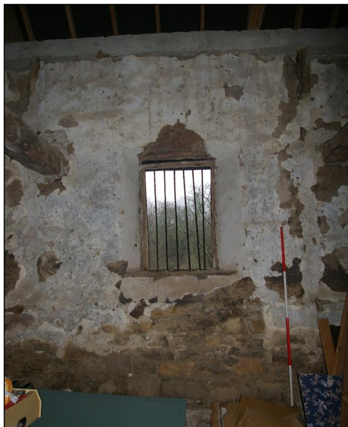
33. FORCED C18 WINDOW IN SOUTH WALL. VIEW FROM NORTH.
