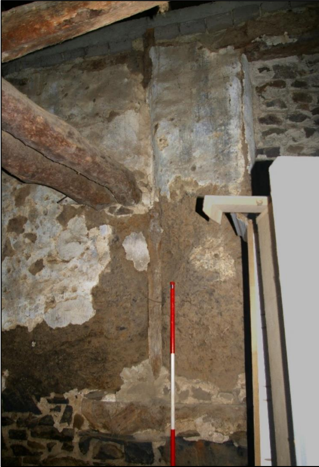
20. WEST JAMB OF NORTH THRESHING DOOR WITH CRUCK FOOT IN COB WALL. VIEW FROM SOUTH-EAST.
