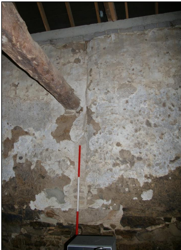
19. SITE OF SECOND CRUCK FROM WEST IN NORTH WALL, WITH LARGE ELM PAD UNDER VERTICAL PLASTERED GROOVE. VIEW FROM SOUTH.
