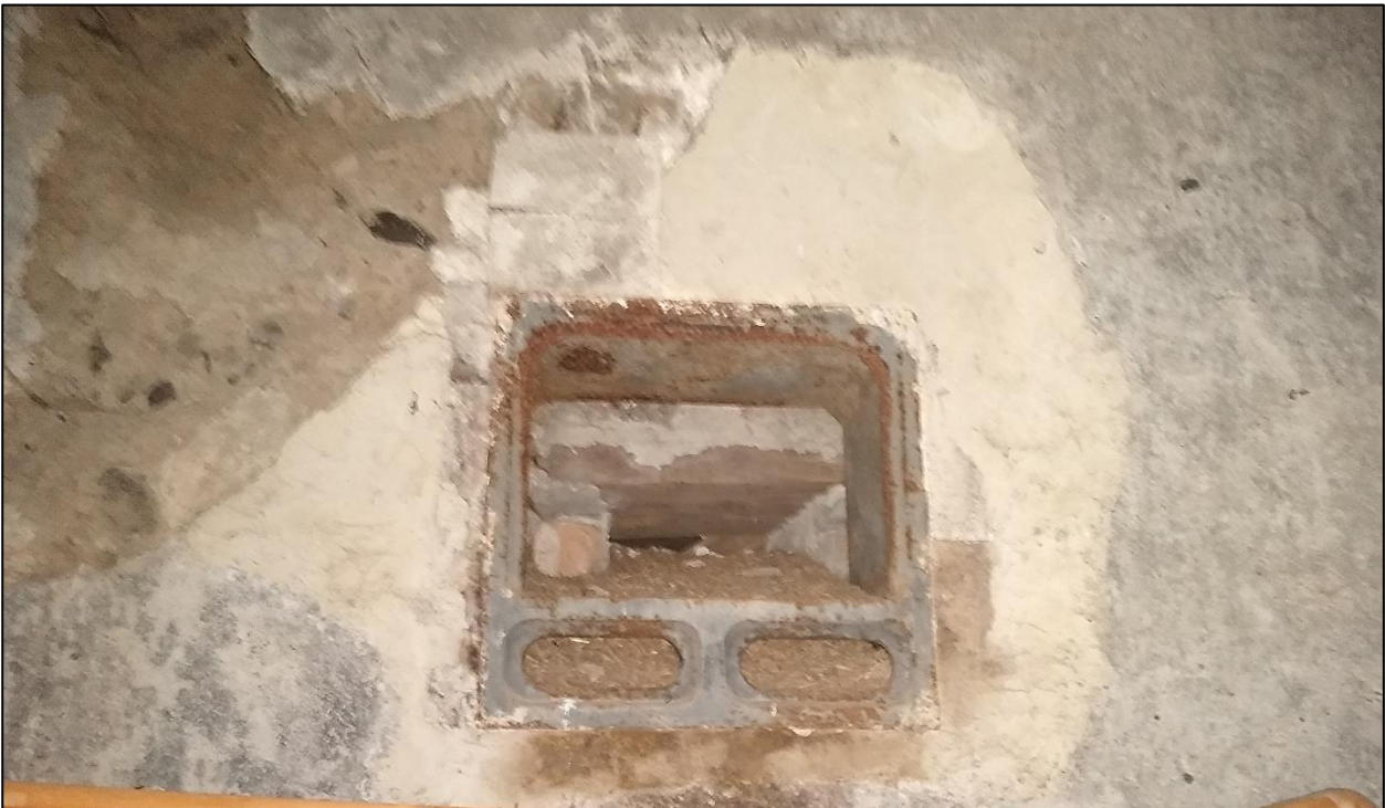
47. CAST IRON BEARING BOX FOR INTERMEDIATE PULLEY ON DRIVE-BELT TRAIN, INSERTED INTO EAST WALL OF BARN IN LATE C19/EARLY C20. NOTE BRICKS AND PALE HARD MORTAR SURROUNDING. VIEW LOOKING UP FROM WEST.
