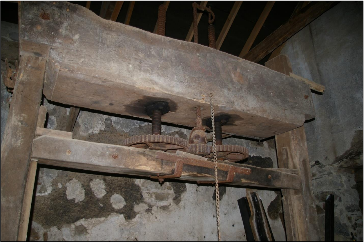
44. UPPER BEAM OF CIDER PRESS, LOOKING UP FROM SOUTH-SOUTH-WEST. THE PURPOSE OF THE LARGE CAPITAL W IS NOT KNOWN.
