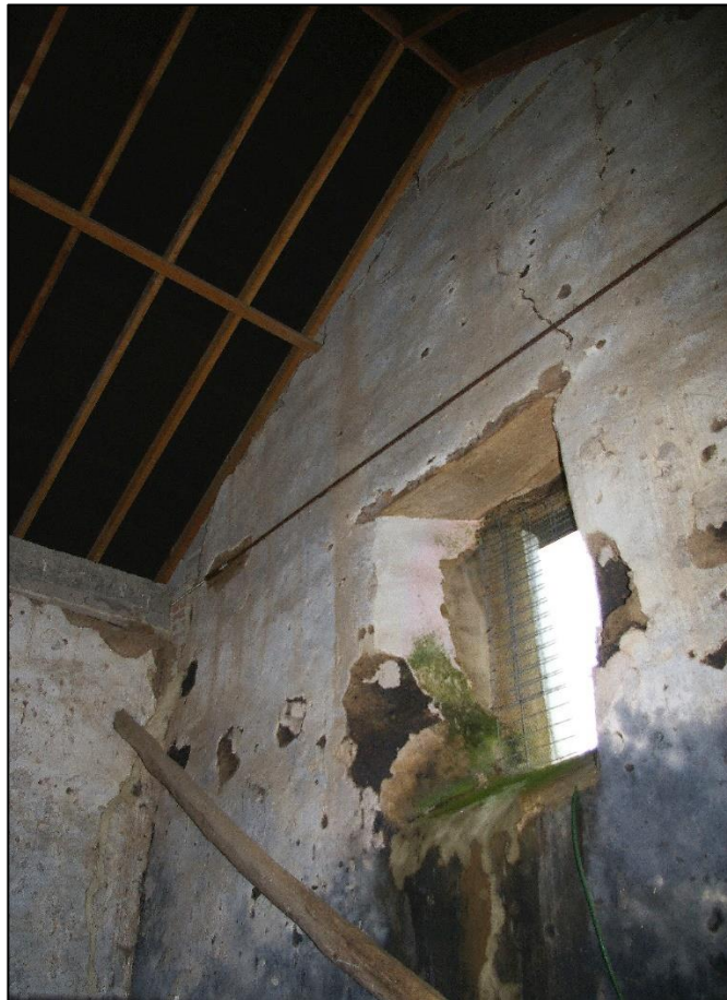
15. WEST GABLE OF CIDER BARN, LOOKING UP FROM NORTH-EAST WITH C15-C16 PRIMARY VENTILATION SLIT. NOTE URINE-BLACKENED COB IN POST-MEDIEVAL JOIST-HOLES UNDER C18 PLASTER.
