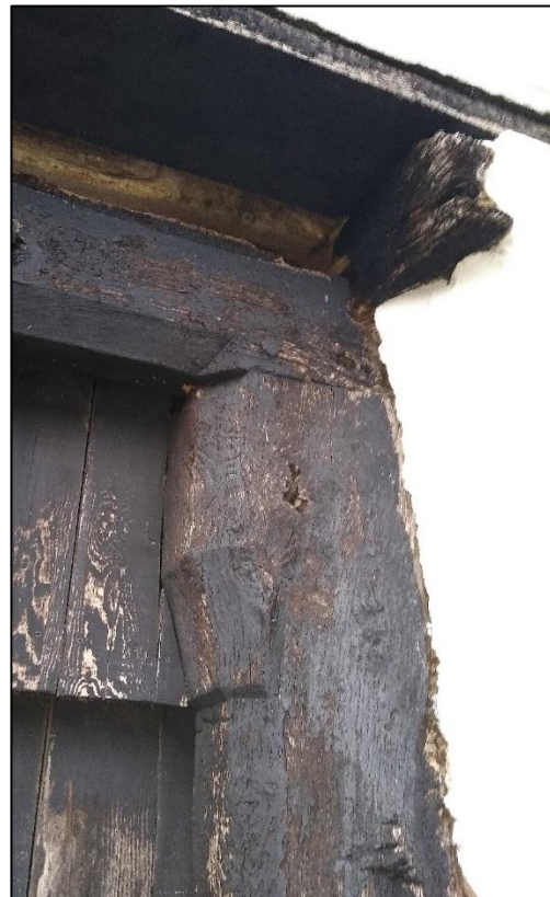
10 & 11. CHAMFERED SHOULDERS OF LEFT AND RIGHT JAMBS OF THRESHING DOOR D1 IN SOUTH WALL. VIEWS FROM SOUTH-EAST AND SOUTH-WEST RESPECTIVELY.
