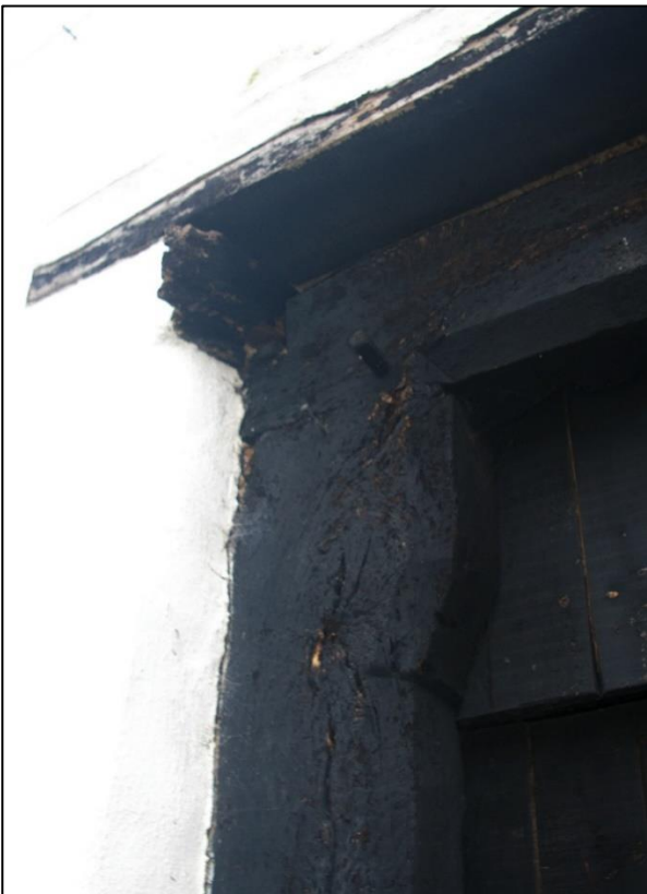
10 & 11. CHAMFERED SHOULDERS OF LEFT AND RIGHT JAMBS OF THRESHING DOOR D1 IN SOUTH WALL. VIEWS FROM SOUTH-EAST AND SOUTH-WEST RESPECTIVELY.
