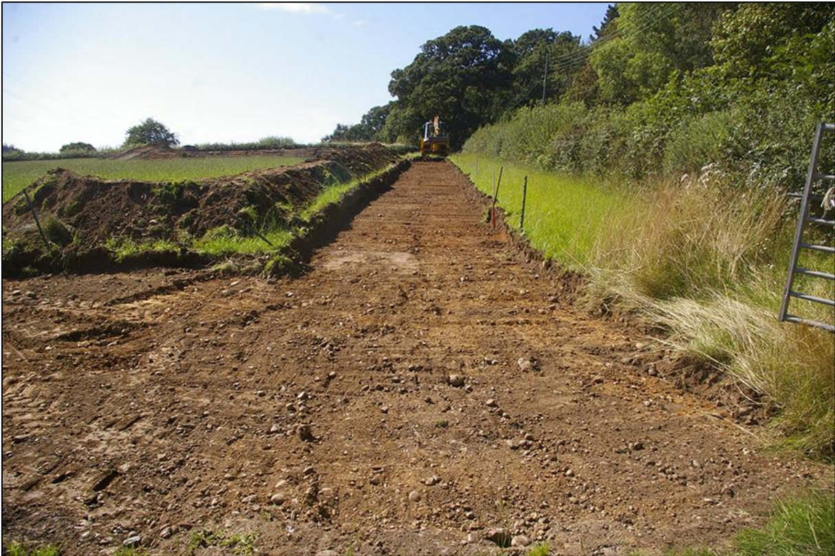
15. ACCESS TRACK, POST-EXCAVATION; VIEWED FROM THE EAST (1M SCALE).
