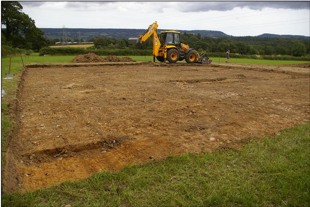
1. SITE SHOT, MID-EXCAVATION; VIEWED FROM THE NORTH-WEST (NO SCALE).
