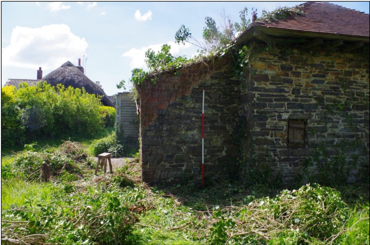
51. EAST ELEVATION FOLLOWING IVY REMOVAL, FROM THE EAST (2M SCALE).
