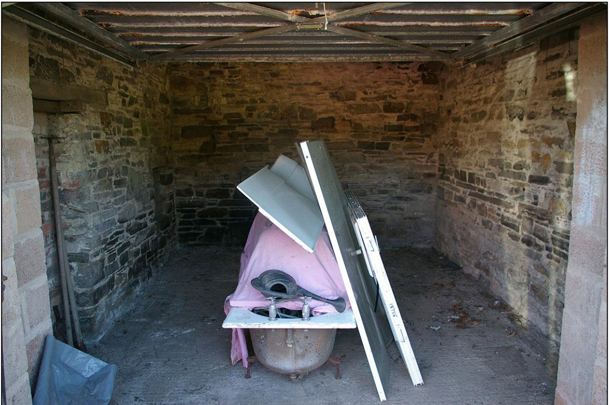
37. ROOM 2; FROM THE EXTERIOR, D2; FROM THE NORTH.
