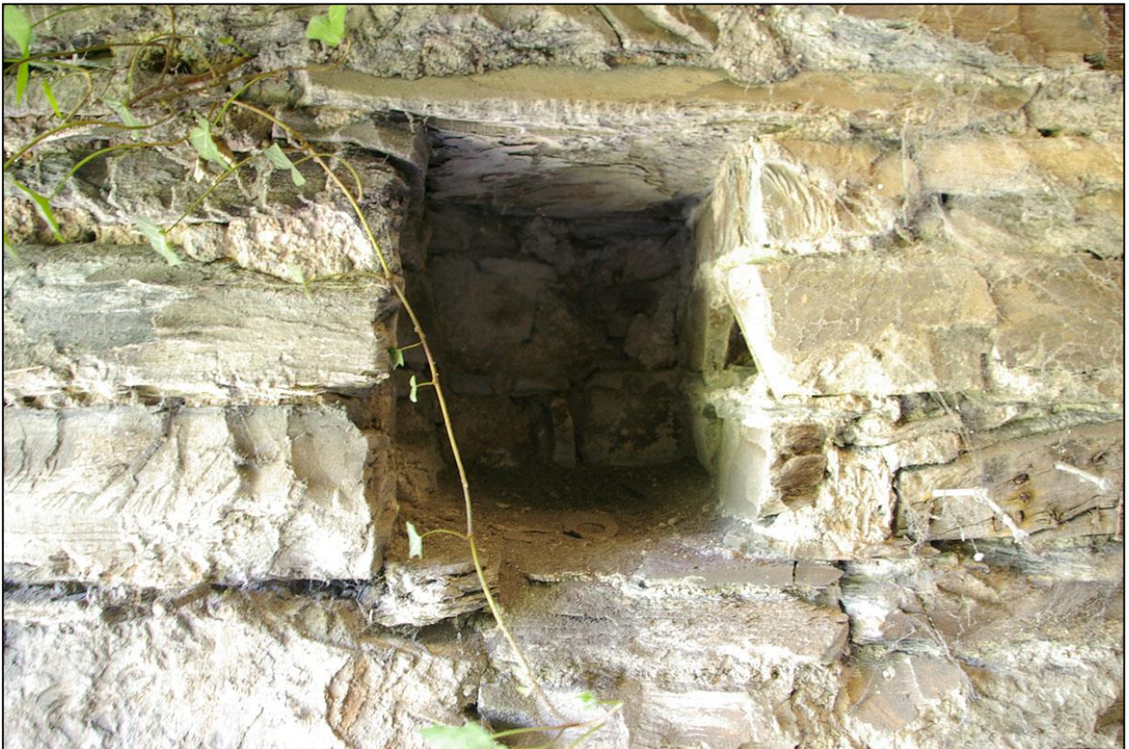
21. THE SMALLER SOCKET, BUILT WITHIN THE STONEWORK; FROM THE EAST.
