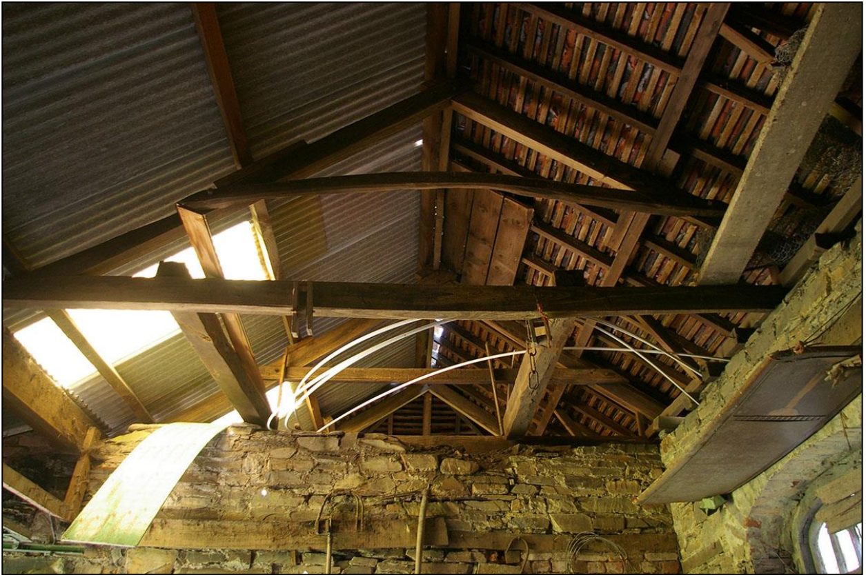
34. THE TRUSS OVER ROOM 1, BETWEEN THE TWO BAYS; FROM THE EAST.
