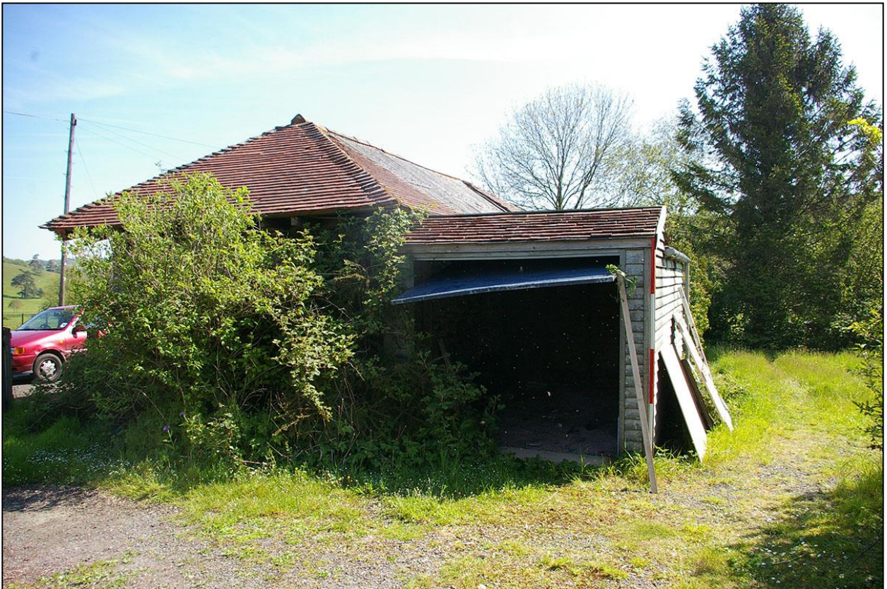
9. THE SMITHY, WITH GARAGE, 2M SCALE; FROM THE SOUTH-WEST.
