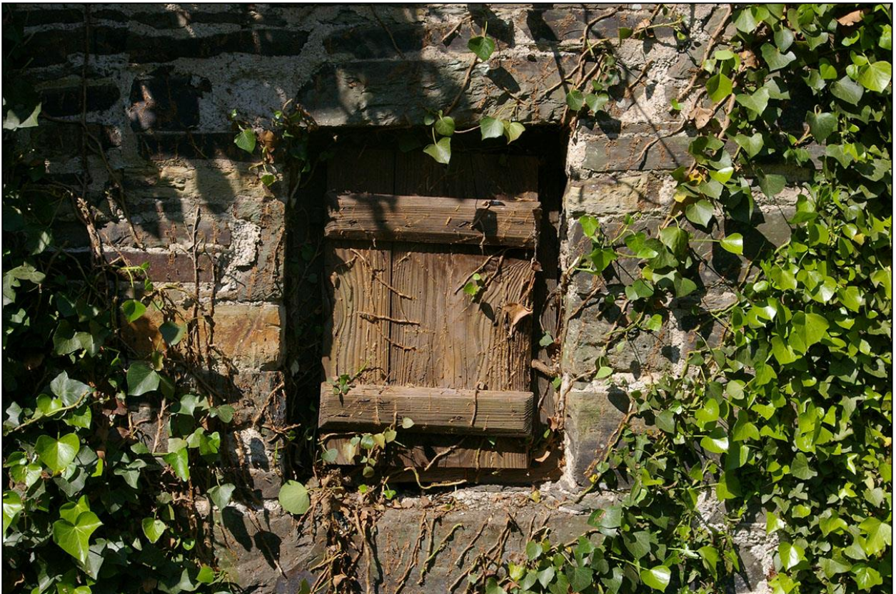
17. BD3 – DOOR/HATCH IN THE EAST ELEVATION; FROM THE EAST.
