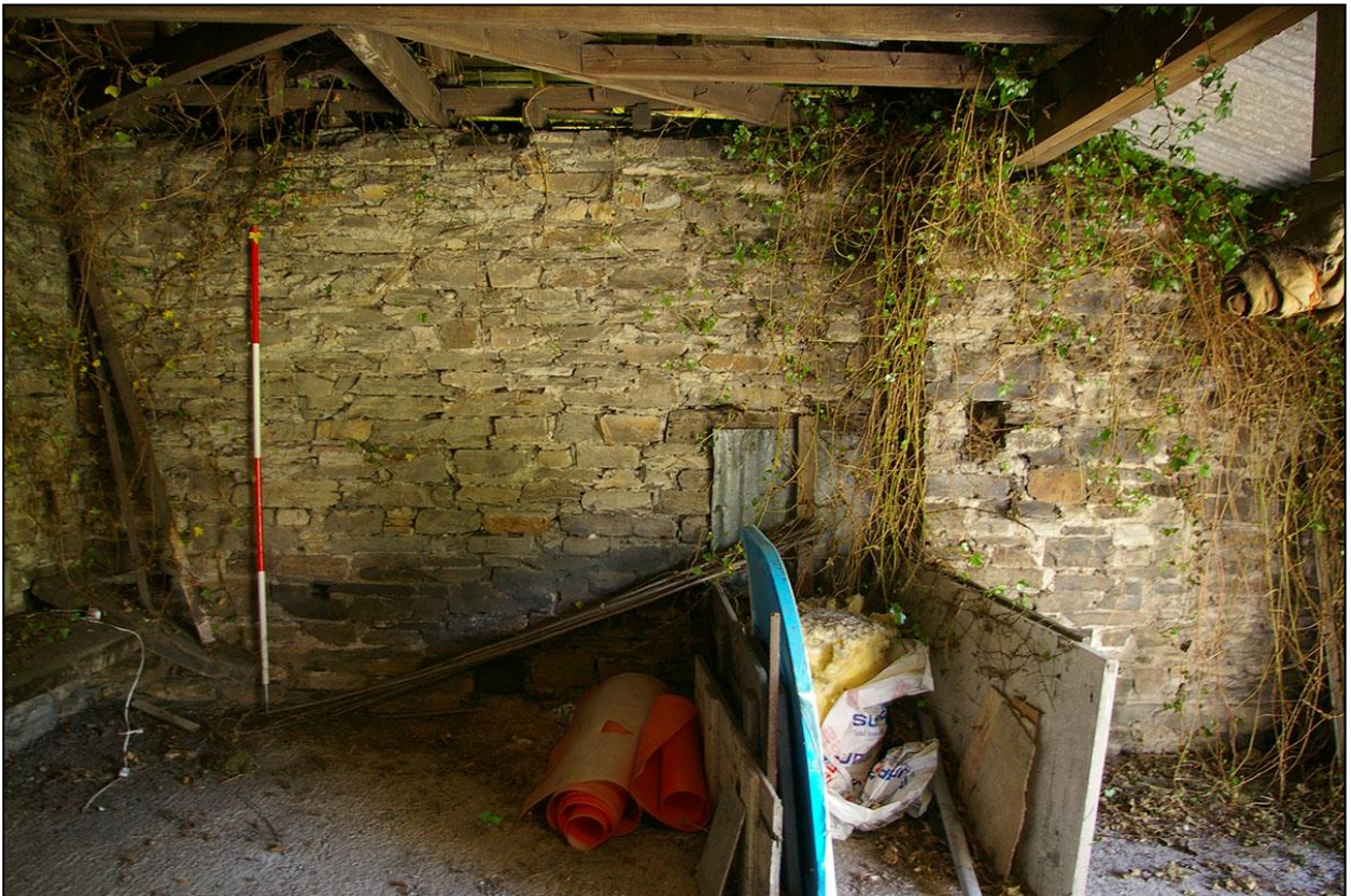
29. THE EAST WALL OF ROOM 1, WITH 2M SCALE; FROM THE WEST.
