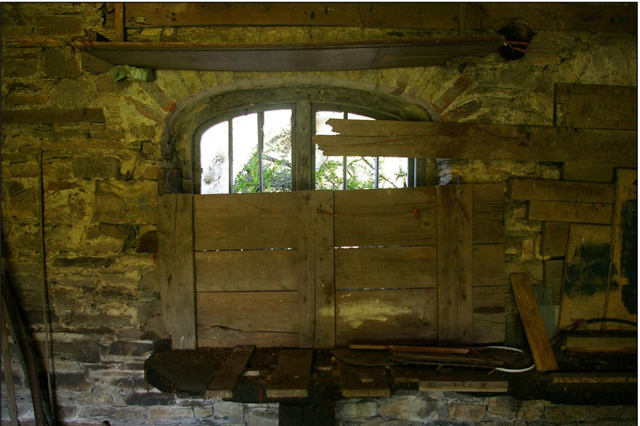
25. W2, SHOWING SOME OF THE BOARDING REMOVED; FROM THE SOUTH.
