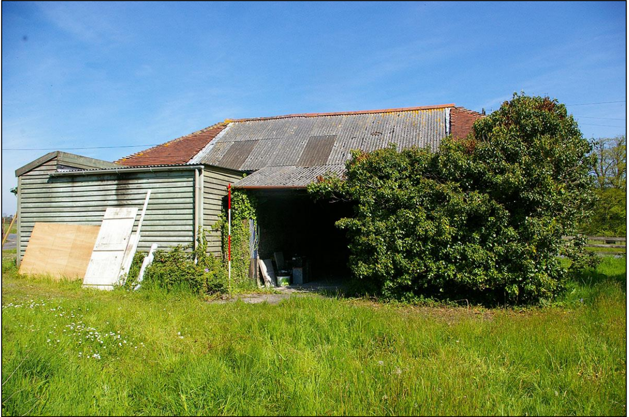
14. WIDE ANGLE OF THE SMITHY, WITH 2M SCALE; FROM THE SOUTH-EAST.
