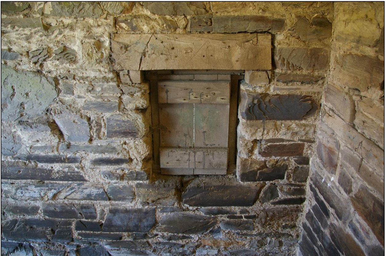
45. BD2 – IN THE EAST WALL OF ROOM 2; FROM THE WEST.
