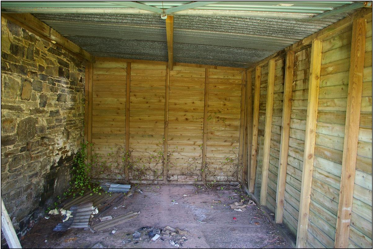
36. ROOM 3; THE TIMBER GARAGE; FROM THE WEST.
