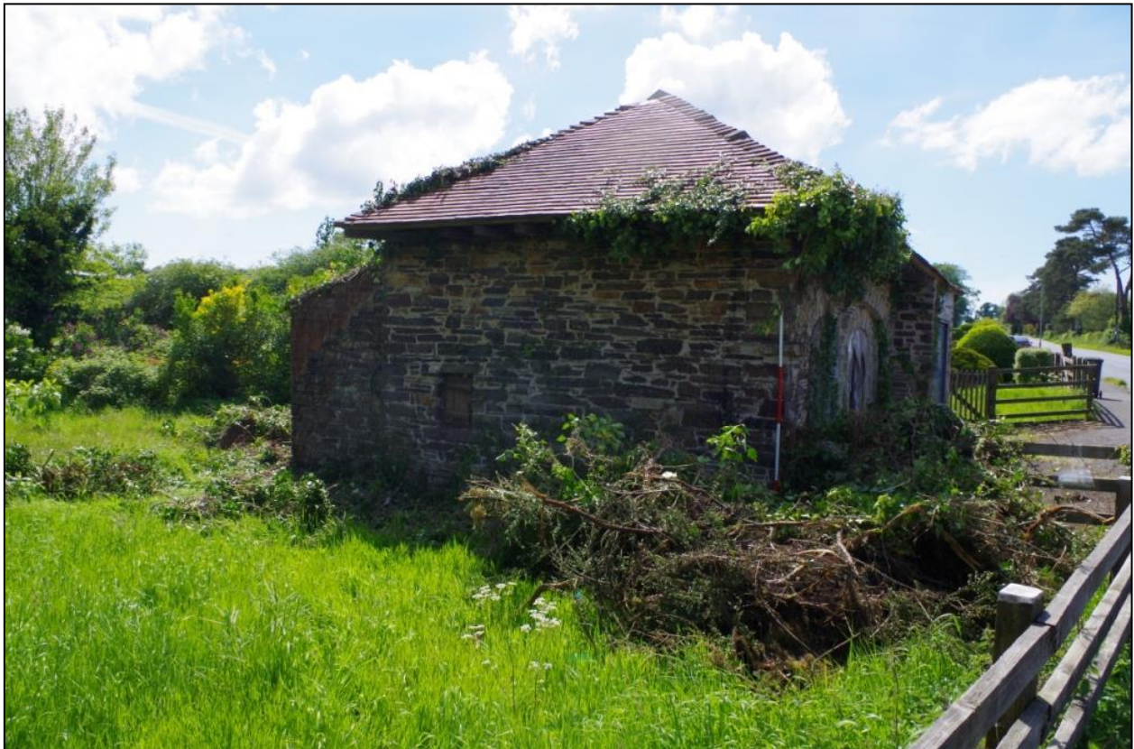
53. AS ABOVE, FROM THE NORTH-EAST (2M SCALE).
