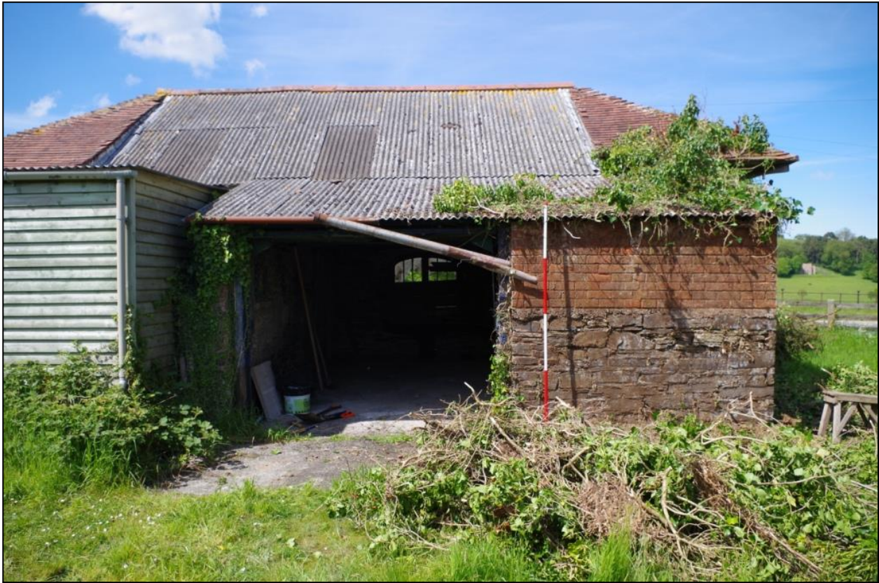
50. SOUTH ELEVATION FOLLOWING IVY REMOVAL, FROM THE SOUTH (2M SCALE).
