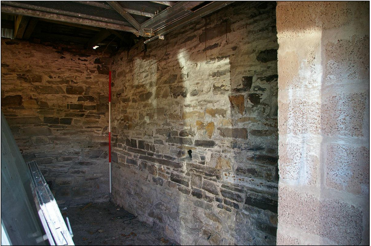
38. THE WEST WALL OF ROOM 2, WITH 2M SCALE; FROM THE NORTH-EAST.
