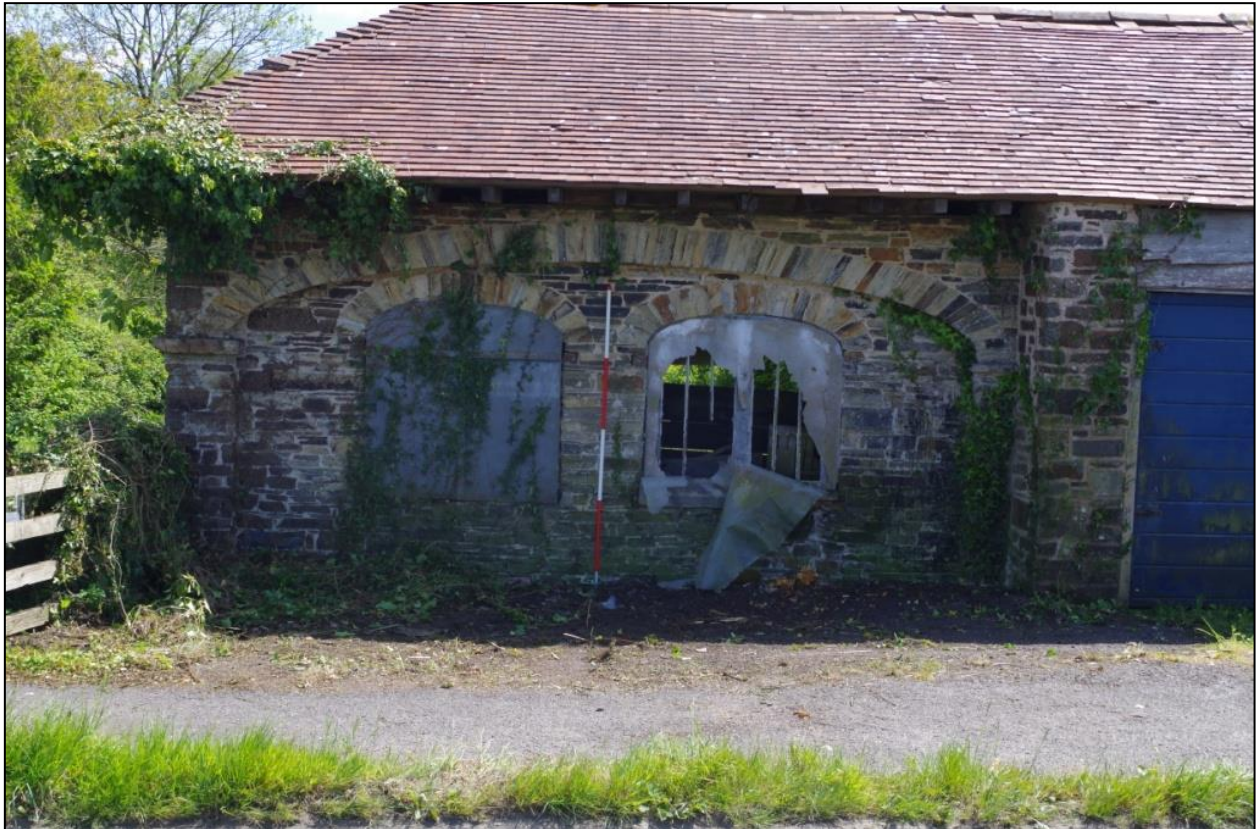
54. NORTH ELEVATION FOLLOWING IVY REMOVAL, FROM THE NORTH (2M SCALE).
