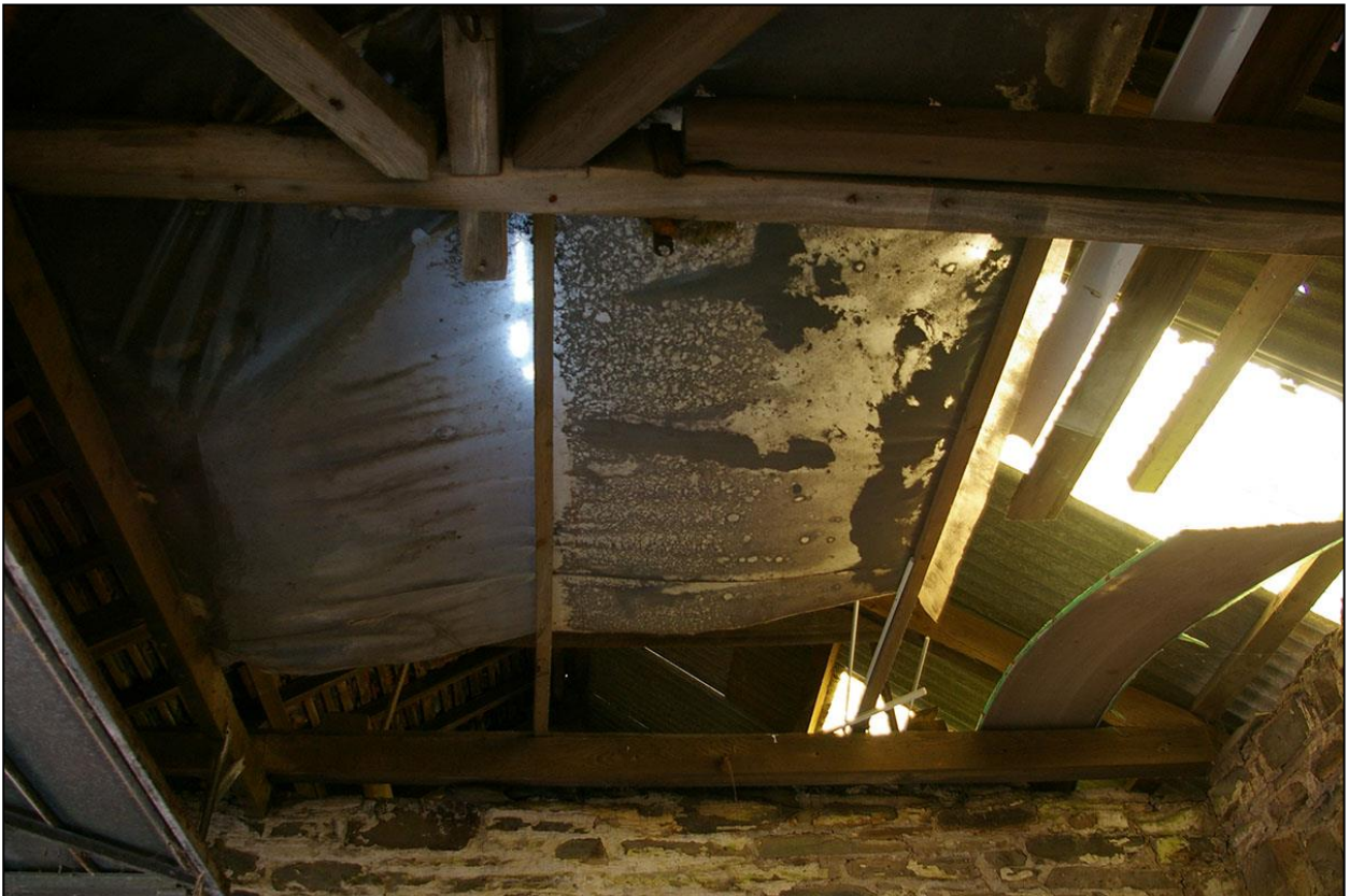
49. THE TRUSS OVER THE PARTY WALL BETWEEN ROOMS 1 & 2; FROM THE WEST.
