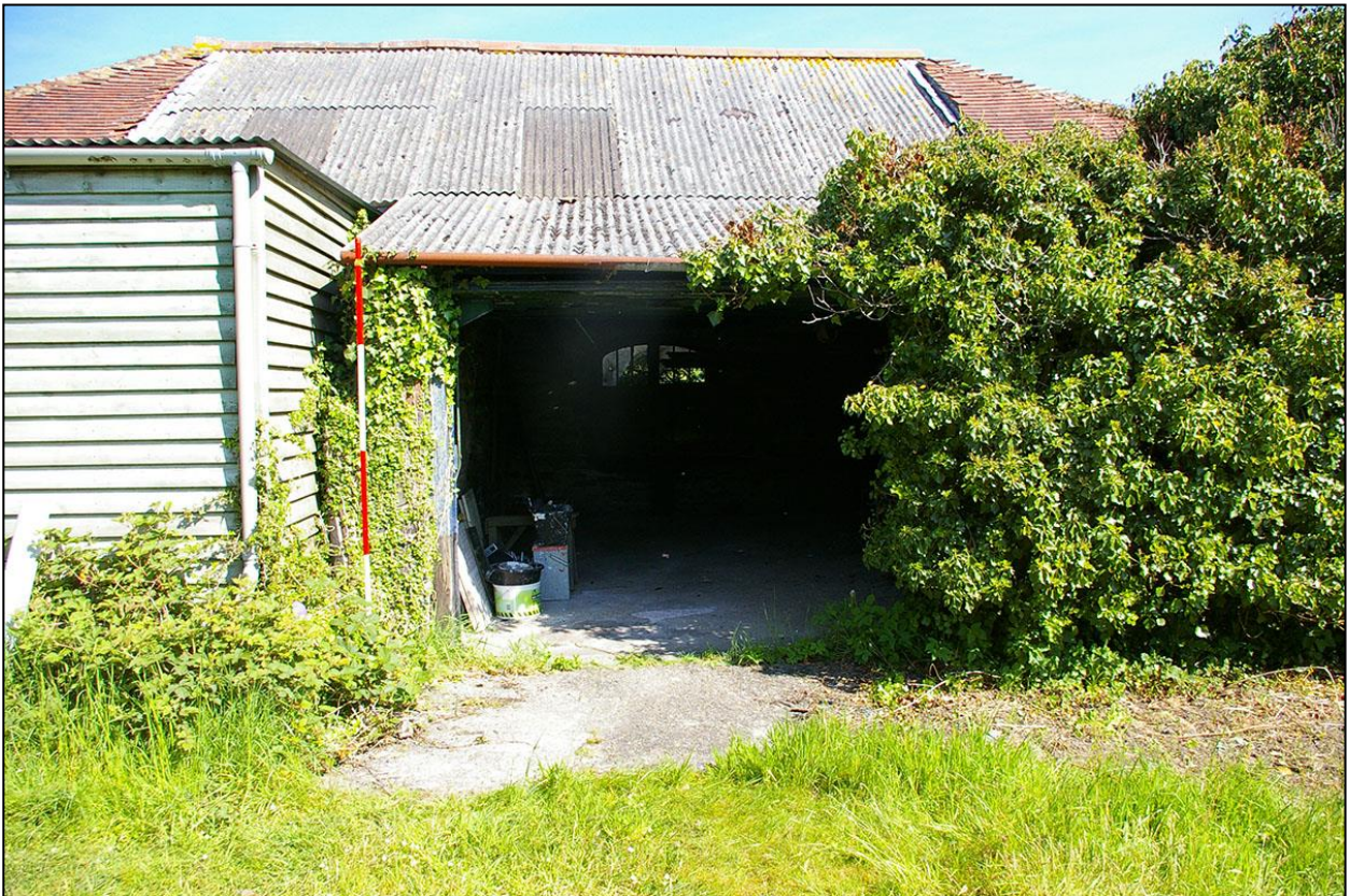
13. D1 THE GARAGE DOOR, LEADING INTO THE INTERIOR OF ROOM 1, WITH 2M SCALE; FROM THE SOUTH.
