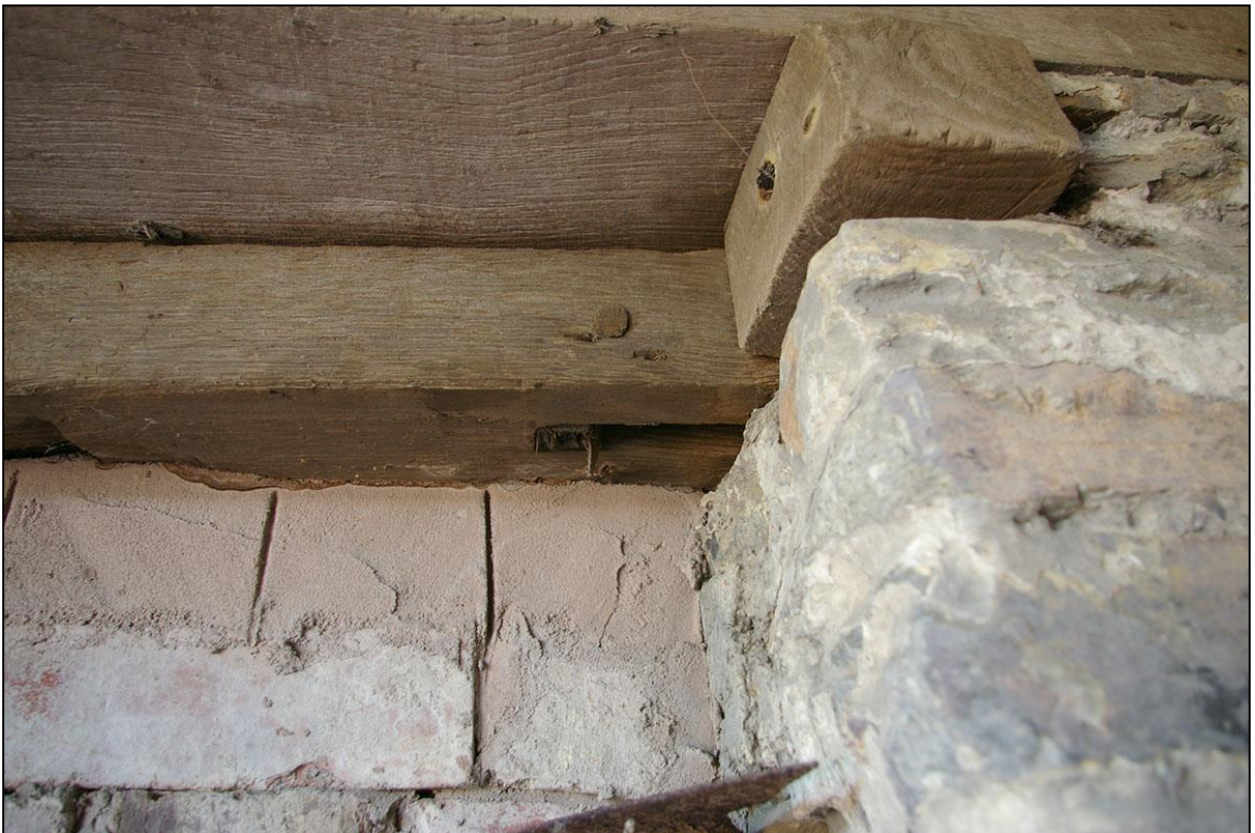
47. BD1 – DETAIL OF THE PEGGED FRAME; FROM THE WEST.
