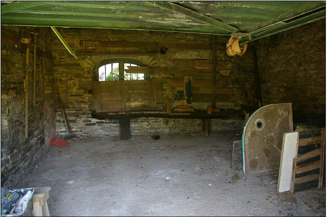
18. ROOM 1, THE MAIN FORMER SMITHY SPACE; FROM THE SOUTH, SOUTH-WEST.
