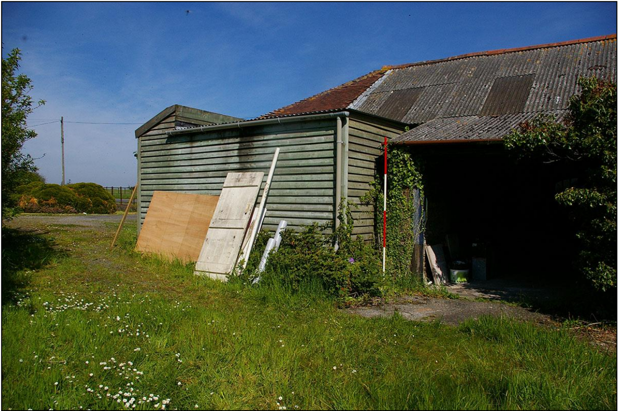
12. THE TIMBER GARAGE, WITH 2M SCALE; FROM THE SOUTH, SOUTH-EAST.
