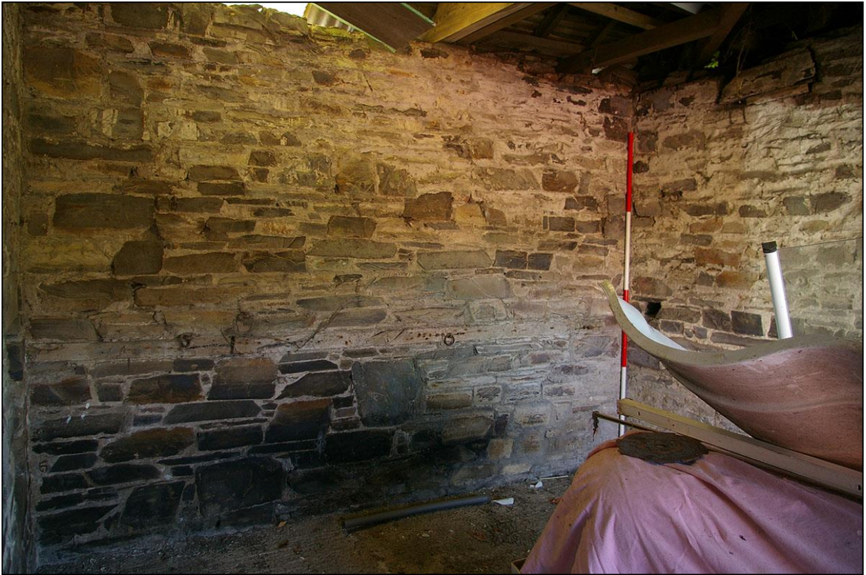
42. THE SOUTH WALL OF ROOM 2, WITH 2M SCALE; FROM THE NORTH-EAST.
