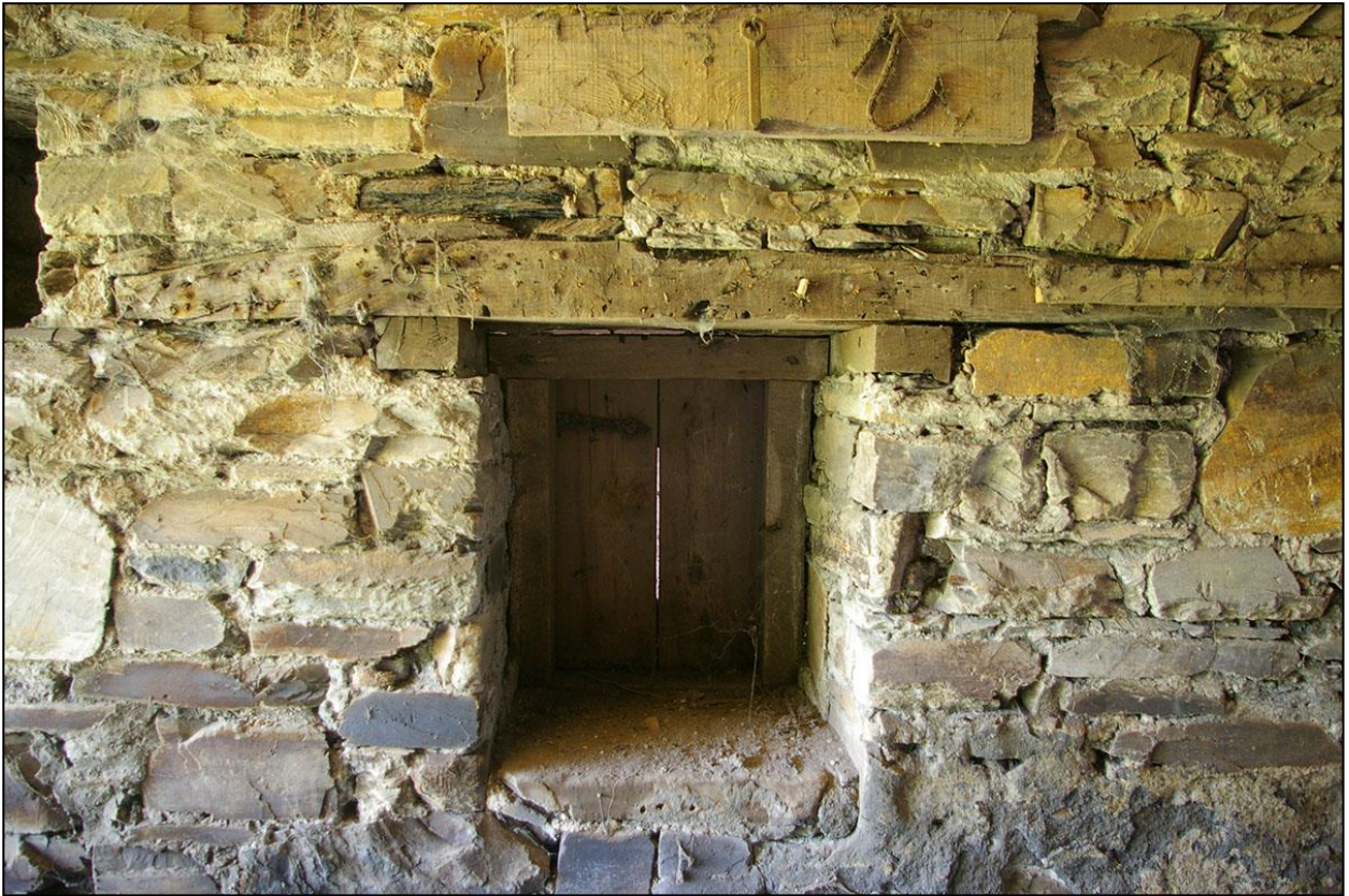
22. BD2 – SMALL RECTANGULAR DOOR/HATCH IN THE PARTY WALL; FROM THE EAST.
