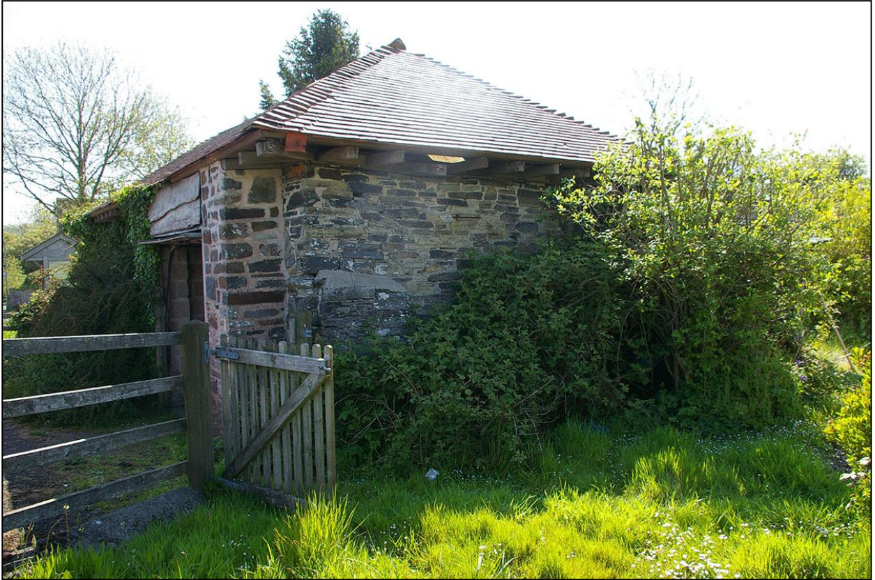
8. THE WEST ELEVATION OF THE BUILDING; FROM THE WEST, NORTH-WEST.
