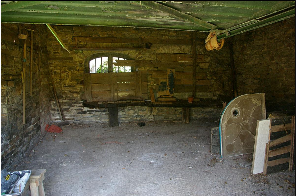
FIGURE 8: ROOM 1, THE MAIN FORMER SMITHY SPACE; FROM THE SOUTH-SOUTH-WEST.
