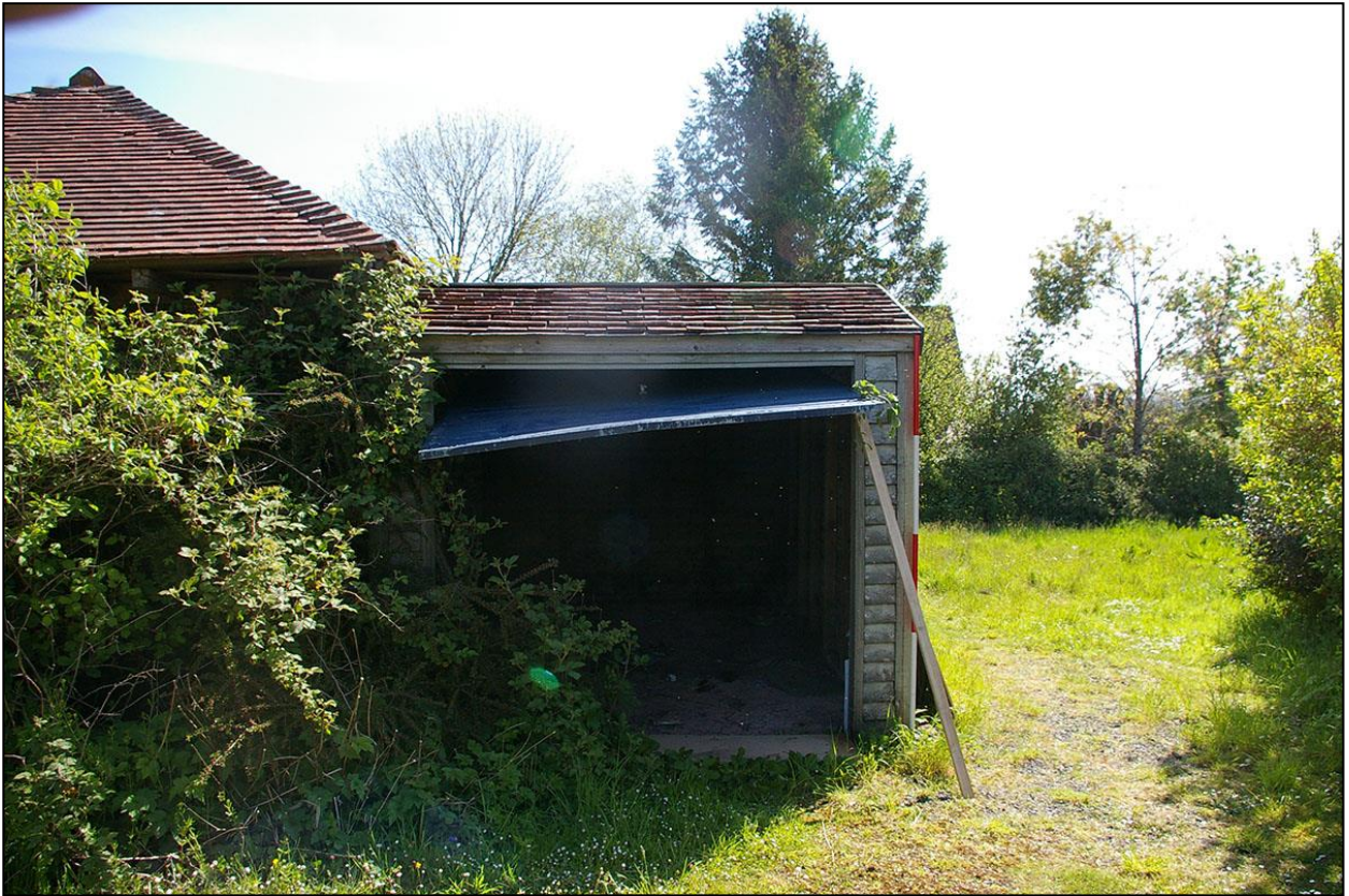
10. THE MODERN TIMBER GARAGE, WITH 2M SCALE AND D3; FROM THE WEST.
