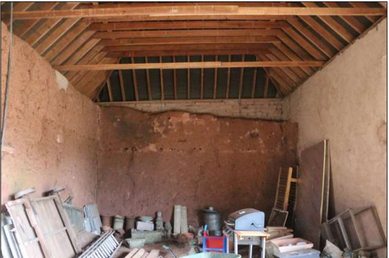
6. THE INTERIOR OF B1; VIEWED FROM THE EAST.
