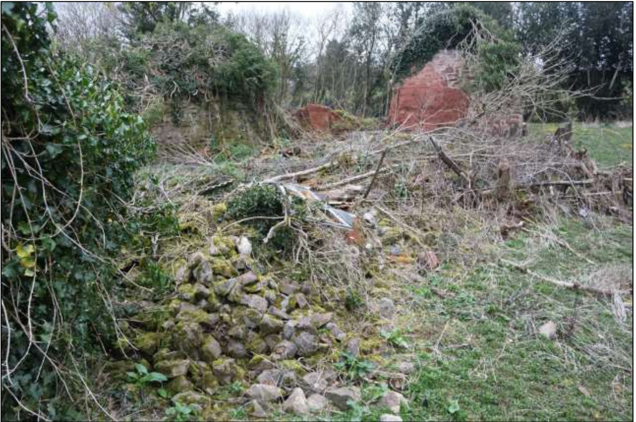
7. THE EAST SIDE OF B2; VIEWED FORM THE SSE.
