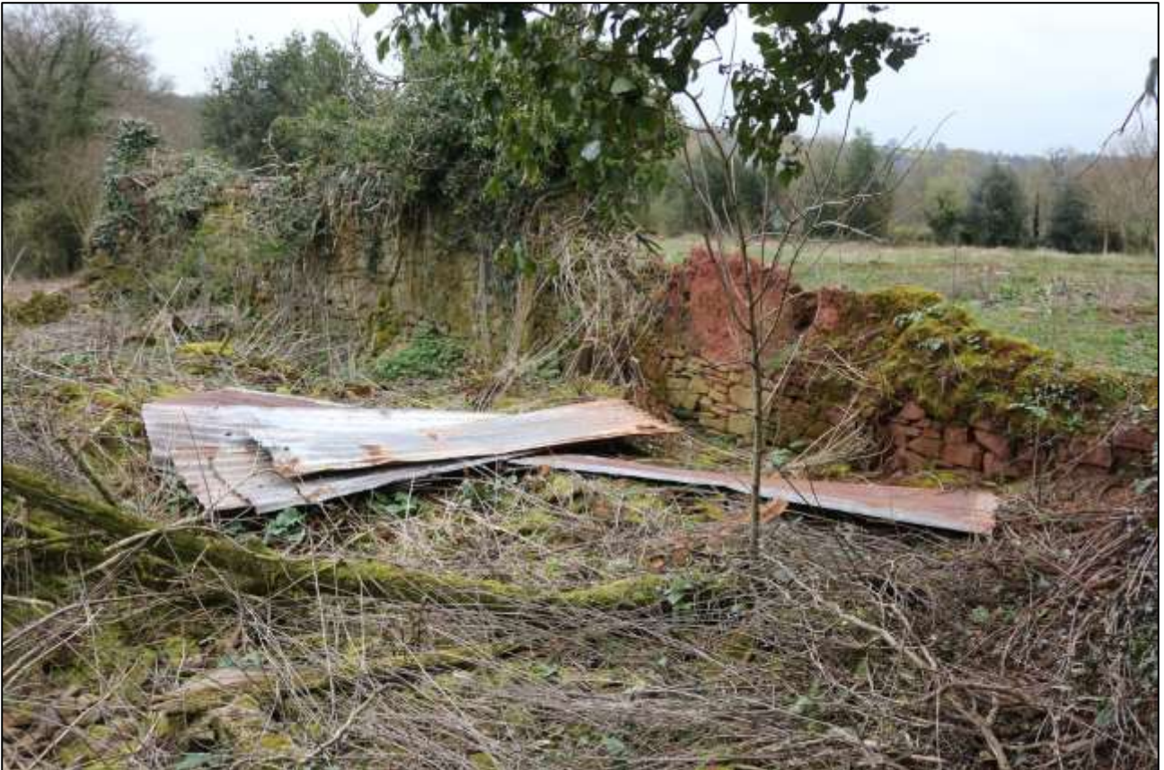
9. THE REAR (WEST) WALL OF B2; VIEWED FROM THE NORTH-EAST.
