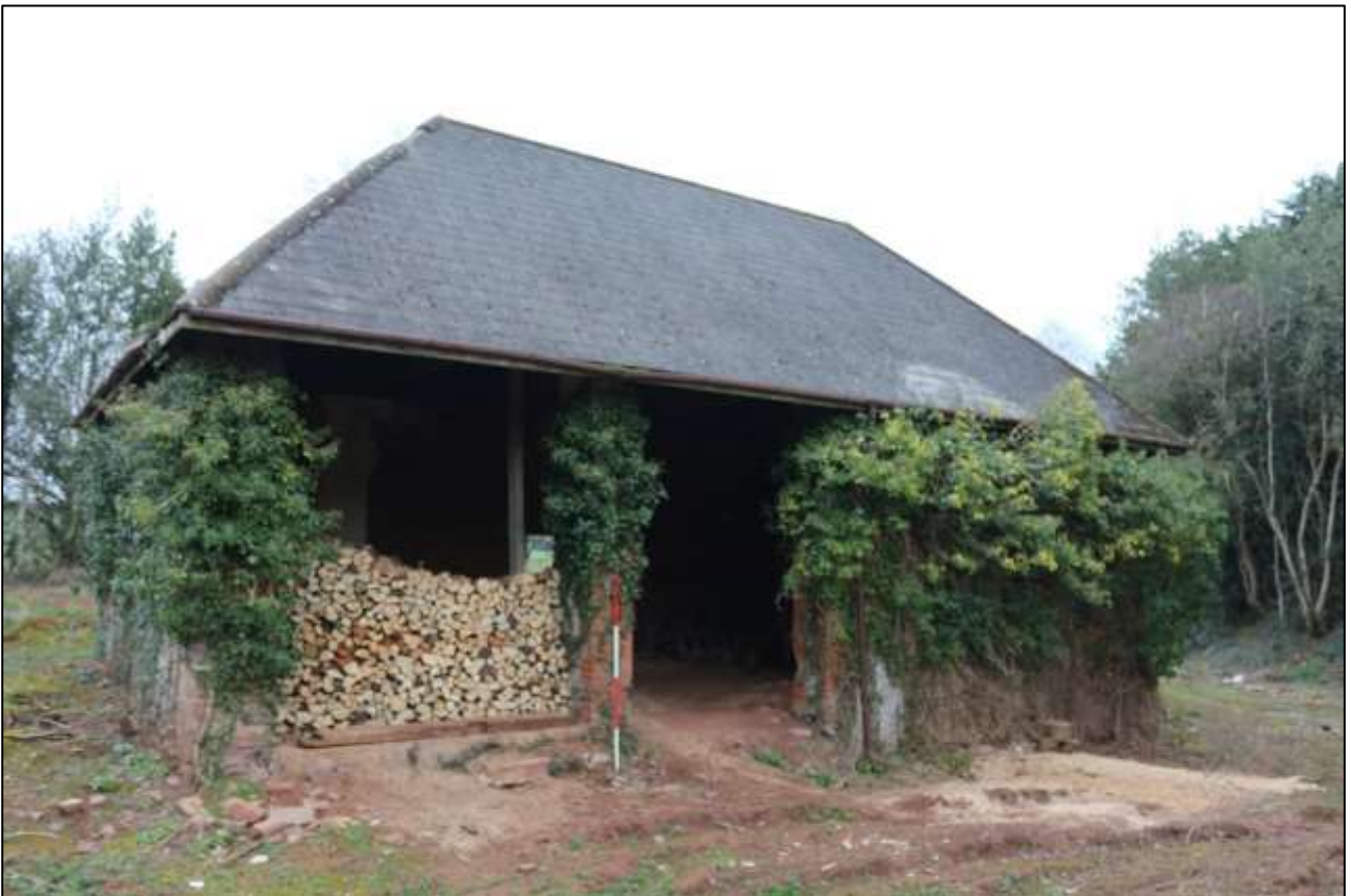
4. THE SOUTH WALL OF B1, SHOWING THE FORCED LINHAY OPENINGS; VIEWED FORM THE SSW (SCALE 2M).
