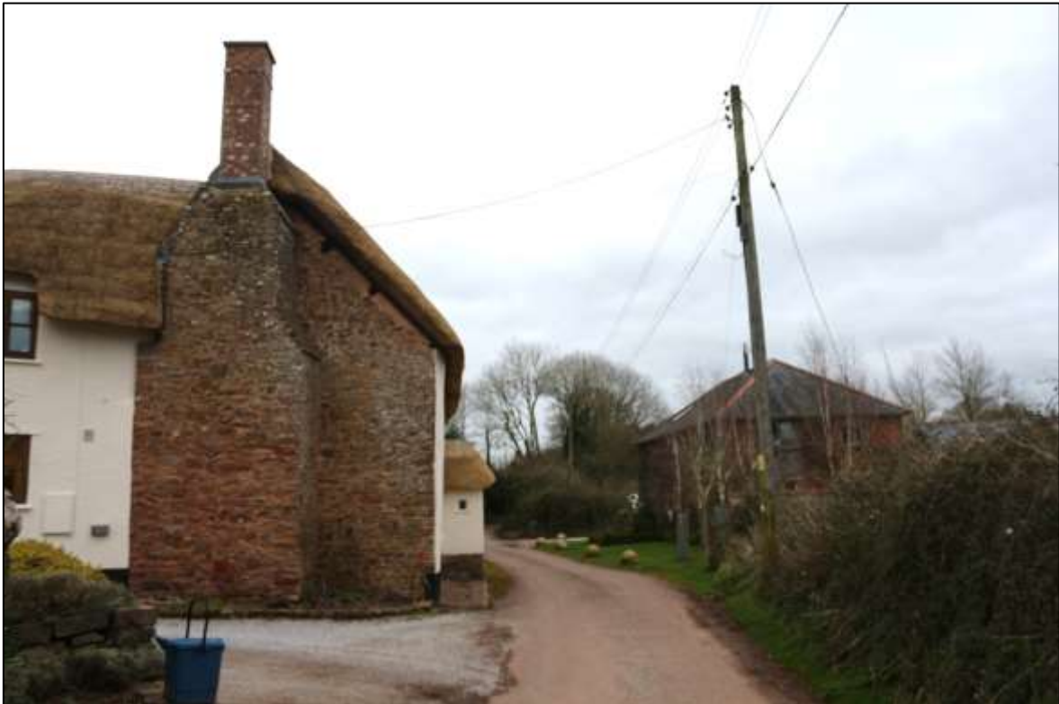
FIGURE 27: VIEW ALONG WEST MANLEY LANE FROM THE WEST, WITH PROWSES TO THE LEFT AND ROSEBARN TO THE RIGHT; VIEWED FROM THE WEST.
