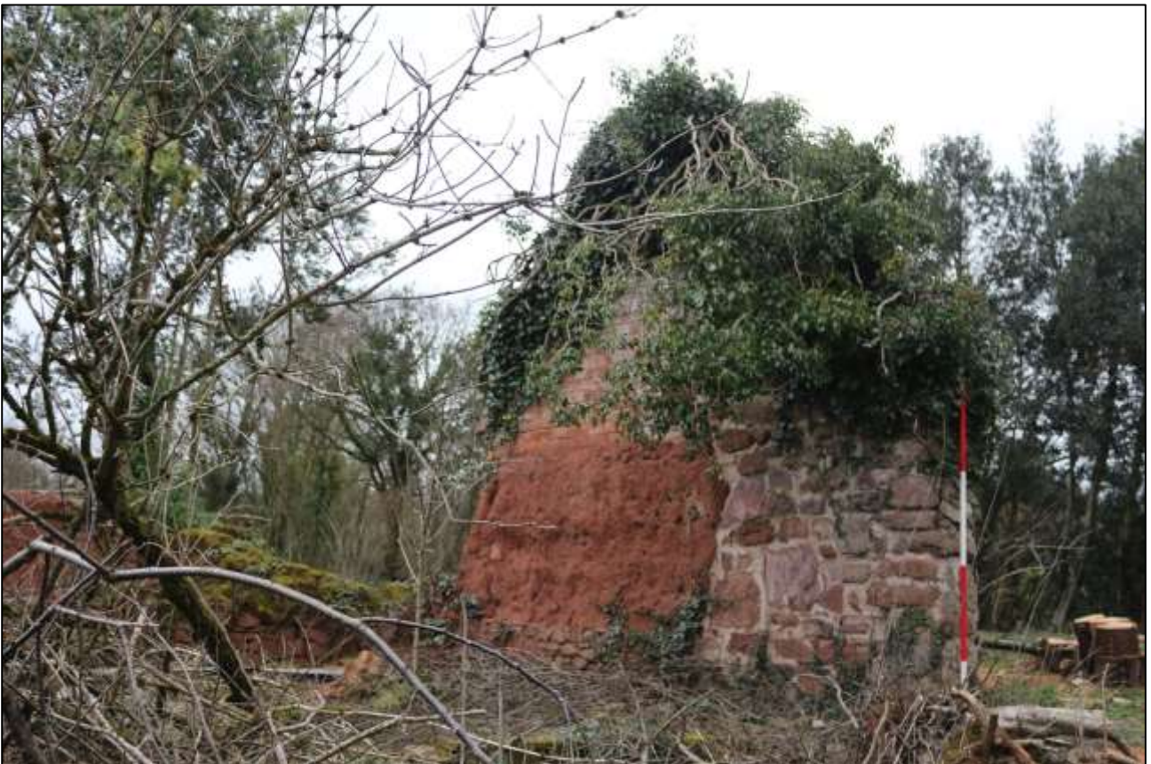
8. THE NORTH GABLE OF B2; VIEWED FROM THE SOUTH-EAST (SCALE 2M).
