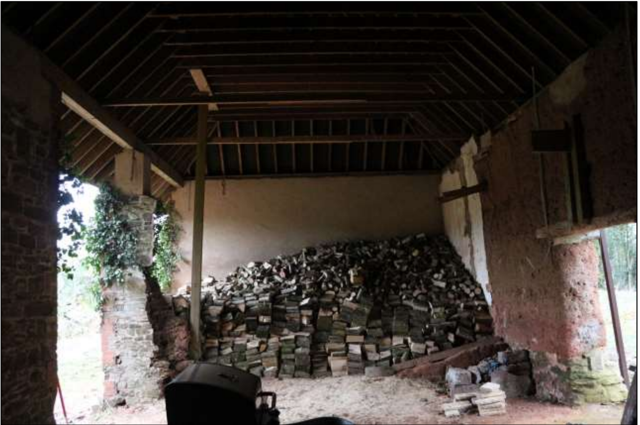
5. THE INTERIOR OF B1; VIEWED FROM THE EAST.
