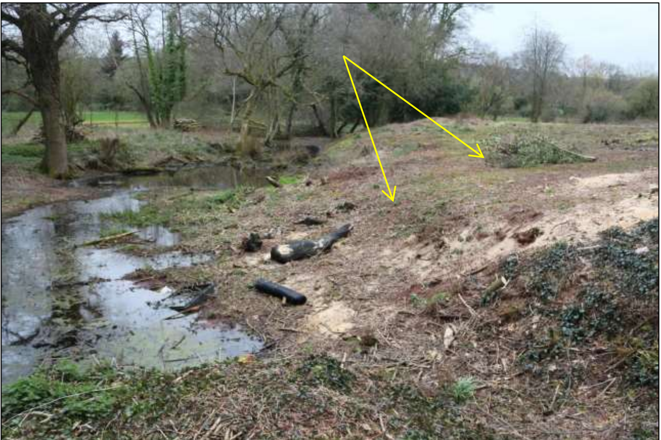
16. THE HOLLOWAY AND THE LOCATION OF FARMHOUSE F1 (INDICATED); VIEWED FROM THE NORTH-EAST.
