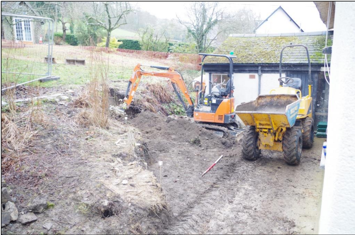
1. START OF WORKS, VIEWED FROM THE NORTH-EAST (1M SCALE).
