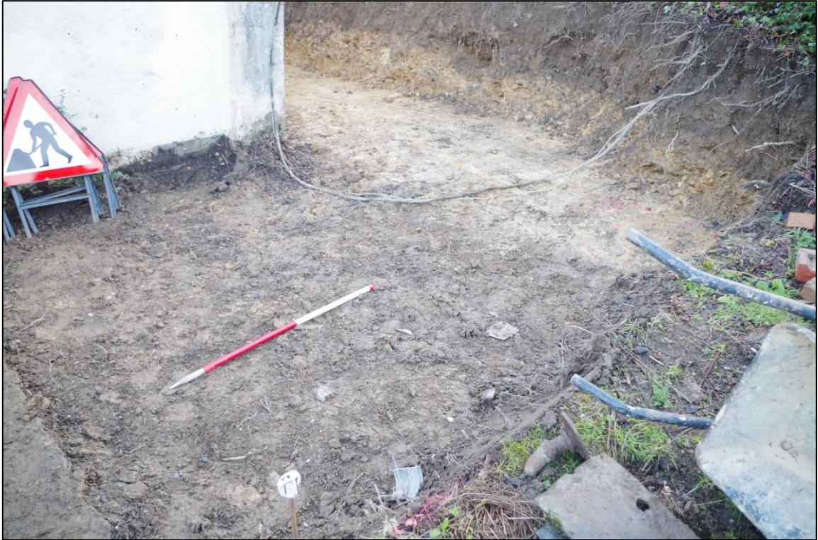
7. THE WESTERN LIMITS OF EXCAVATION, VIEWED FROM THE WEST-NORTH-WEST (1M SCALE).
