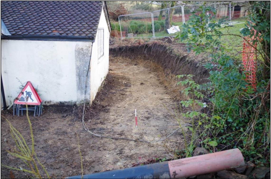
5. LIMITS OF EXCAVATION, VIEWED FROM THE EAST (1M SCALE).
