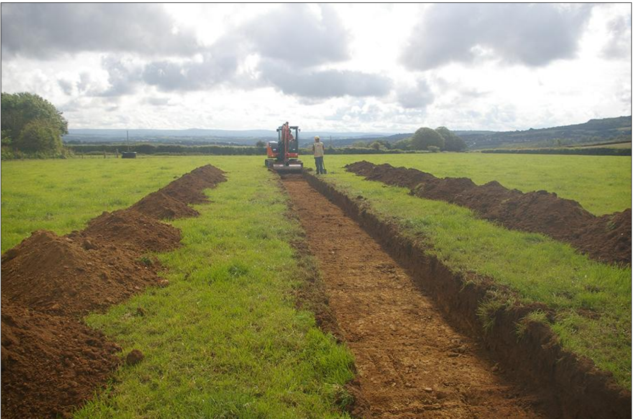
2. WORKING SHOT, TRENCH 01 BEING OPENED; VIEWED FROM THE WEST-NORTH-WEST (NO SCALE).
