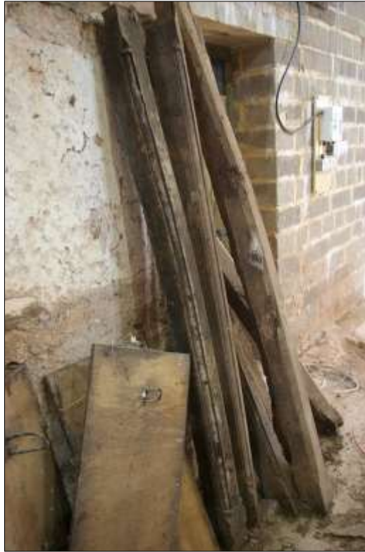
56. DETAIL OF THE EX SITU OVOLO CARVED JOISTS; VIEWED FROM THE NORTH.
