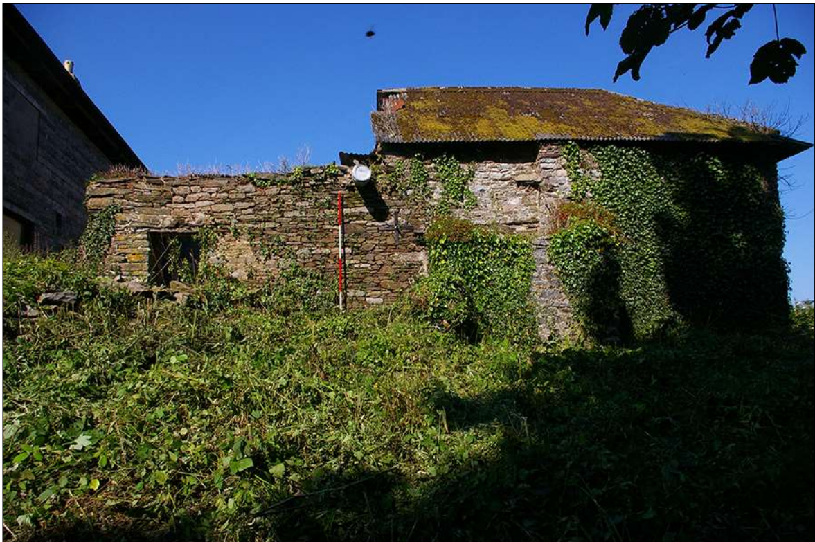
101. THE SOUTH-WEST ELEVATION OF B3; VIEWED FROM THE SOUTH-WEST (2M SCALE).
