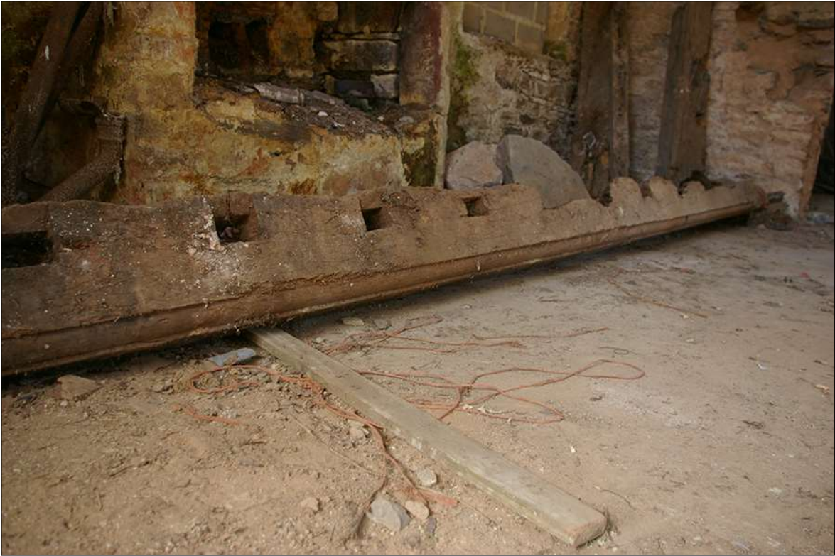
54. DETAIL OF ONE OF THE EX SITU FINE OVOLO CARVED BEAMS WHICH FORMERLY SPANNED THE SOUTH-WEST GROUND-FLOOR ROOM OF B1; VIEWED FROM THE SOUTH.
