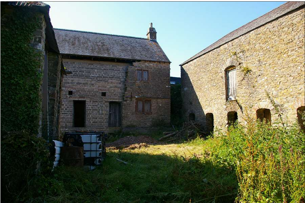
4. THE YARD AREA SURROUND BY B3 (LEFT), B1 (CENTRE), AND B2 (RIGHT); VIEWED FROM THE SOUTH-SOUTH-EAST.
