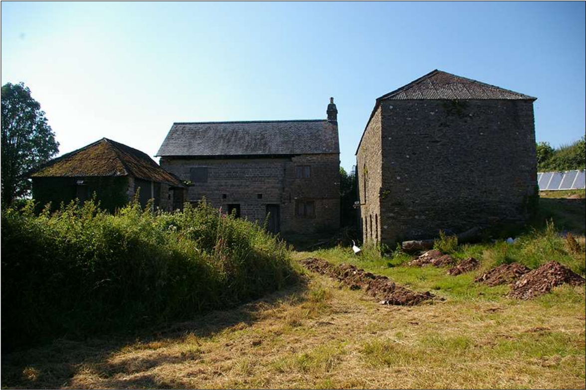
5. VIEW OF THE THREE SURVIVING STRUCTURE (B3 LEFT; B1 CENTRE; B2 RIGHT) AROUND THE CENTRAL YARD; VIEWED FROM THE SOUTH-EAST.
