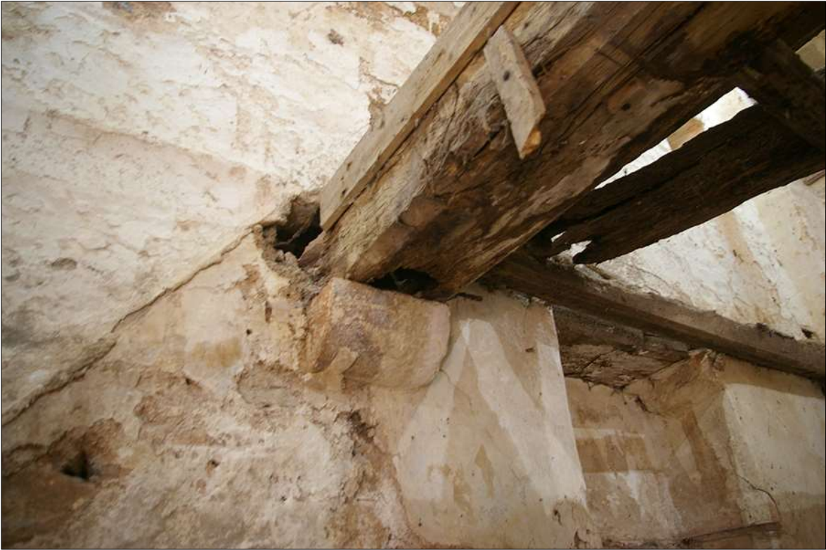
78. DETAIL OF A SURVIVING CEILING BEAM SAT ON A CORBEL; VIEWED FROM THE SOUTH.
