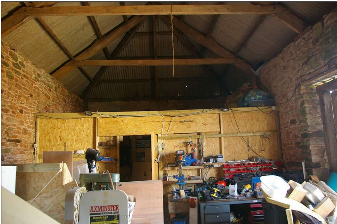
97. THE MODERN PARTITION AND SURFACE MOUNTED WORKSHOP FITMENTS WITHIN B2; VIEWED FROM THE SOUTH-EAST.
