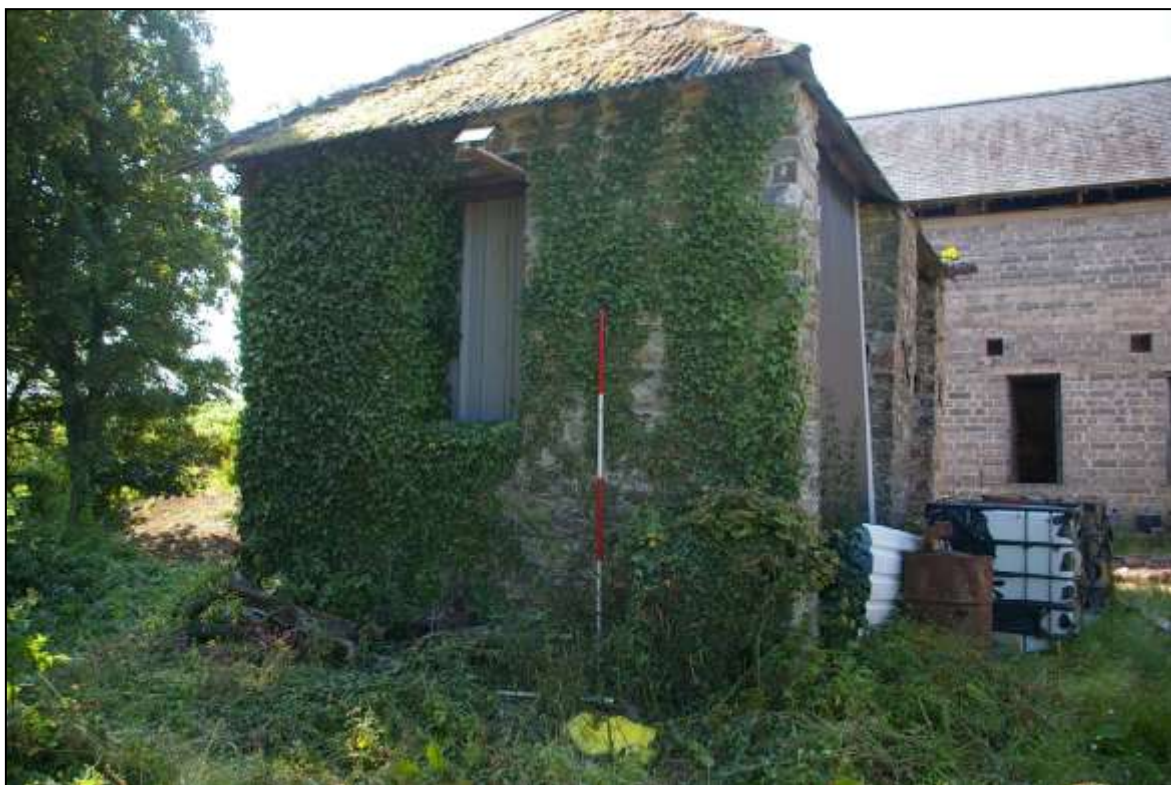
FIGURE 11: SOUTH-EAST ELEVATION OF B3; VIEWED FROM THE EAST (2M SCALE).
