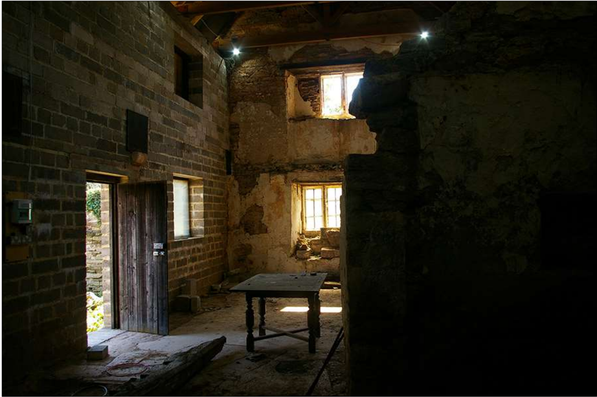
37. VIEW OF THE LARGER SOUTH-WESTERN GROUND-FLOOR ROOM WITHIN B1, DETAILING THE WINDOWS W5 AND W6, AND THE 'RE-SET' WINDOWS W8 AND W10; VIEWED FROM THE NORTH-NORTH-EAST.
