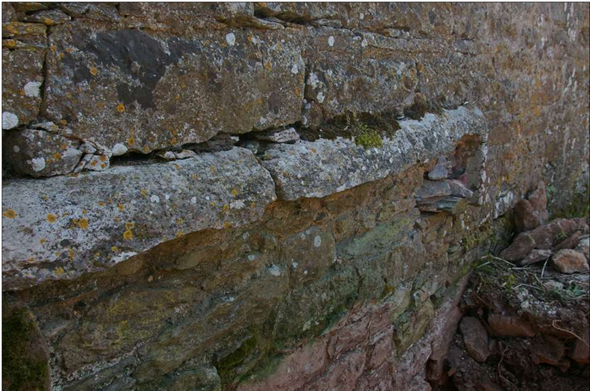
17. DETAIL OF THE CRUDE HOODMOULD OVER W3 WHICH MATCHES THE STRING COURSES TO THE NORTH-EAST AND SOUTH-WEST ELEVATIONS; VIEWED FROM THE NORTH.
