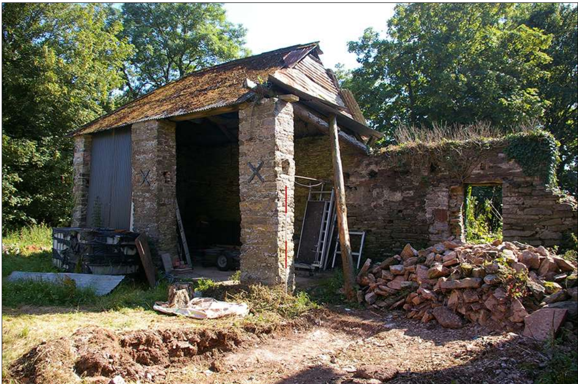
110. THE NORTH-EAST ELEVATION OF B3; VIEWED FROM THE NORTH (2M SCALE).
