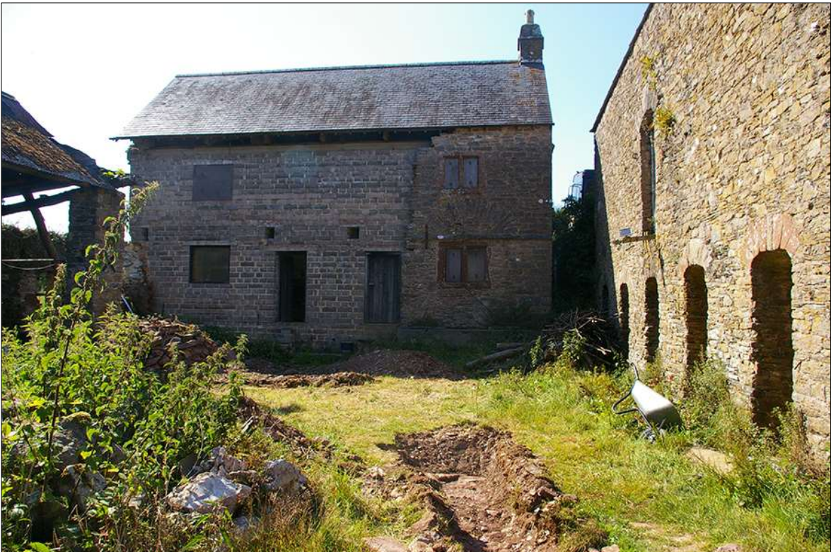
6. THE YARD SURROUNDED BY B3 (LEFT), B1 (CENTRE) AND B2 (RIGHT); VIEWED FROM THE SOUTH-EAST.
