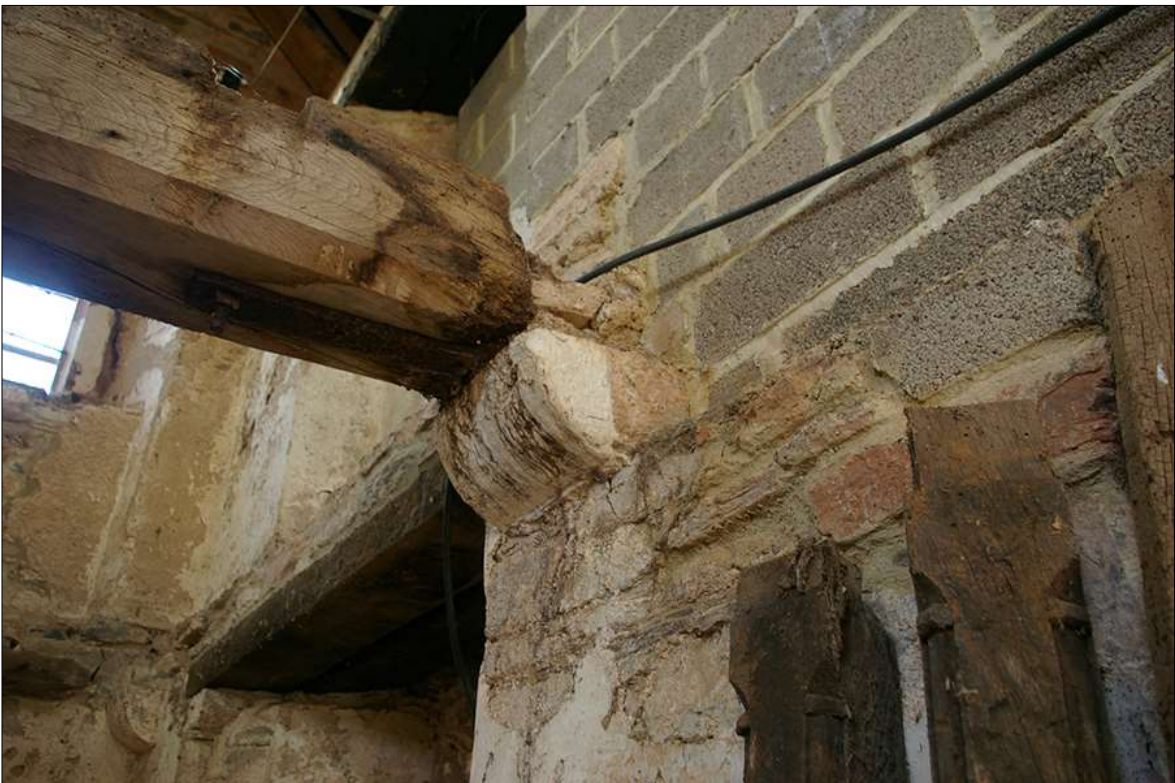
79. DETAIL OF THE SURVIVING CEILING BEAM SAT ON A CORBEL; VIEWED FROM THE WEST.
