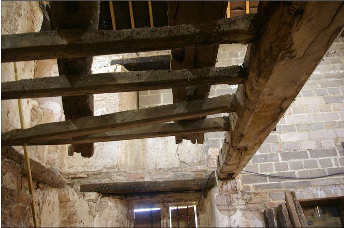
80. DETAIL OF THE CEILING BEAMS TO THE NORTH-EAST GROUND-FLOOR ROOM WITHIN B1, SHOWING THAT THE JOISTS ARE ALSO CHAMFERED WITH CUT STOPS; VIEWED FROM THE NORTH-WEST.
