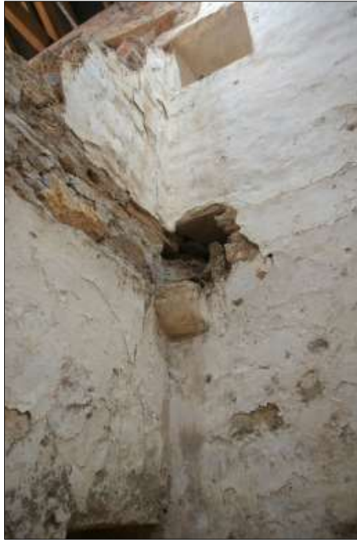
74. (LEFT) DETAIL OF THE CROSS-WALL, SHOWING HOW IT IS CRUDELY BUILT OVER THE CORBEL AND NOT WELL TIED INTO THE NORTH-WEST WALL OF B1; VIEWED FROM THE EAST.
