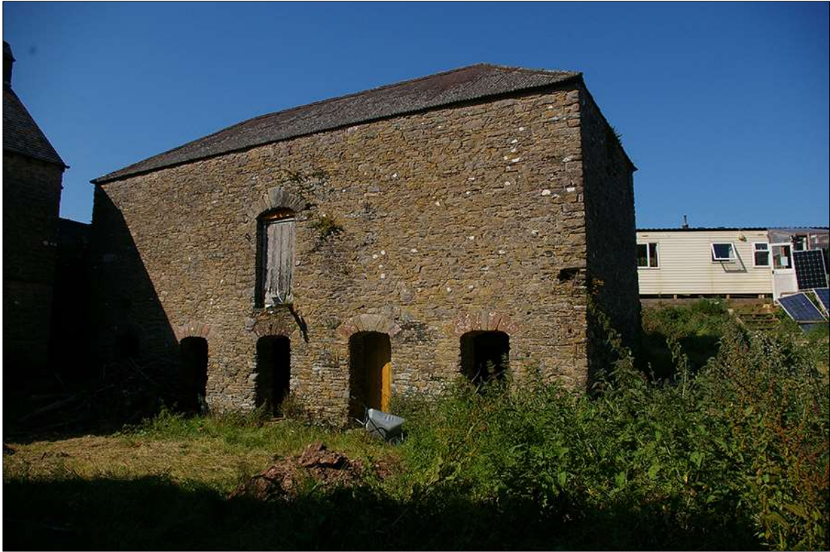
86. THE SOUTH-WEST ELEVATION OF B2; VIEWED FROM THE SOUTH-SOUTH-EAST.
