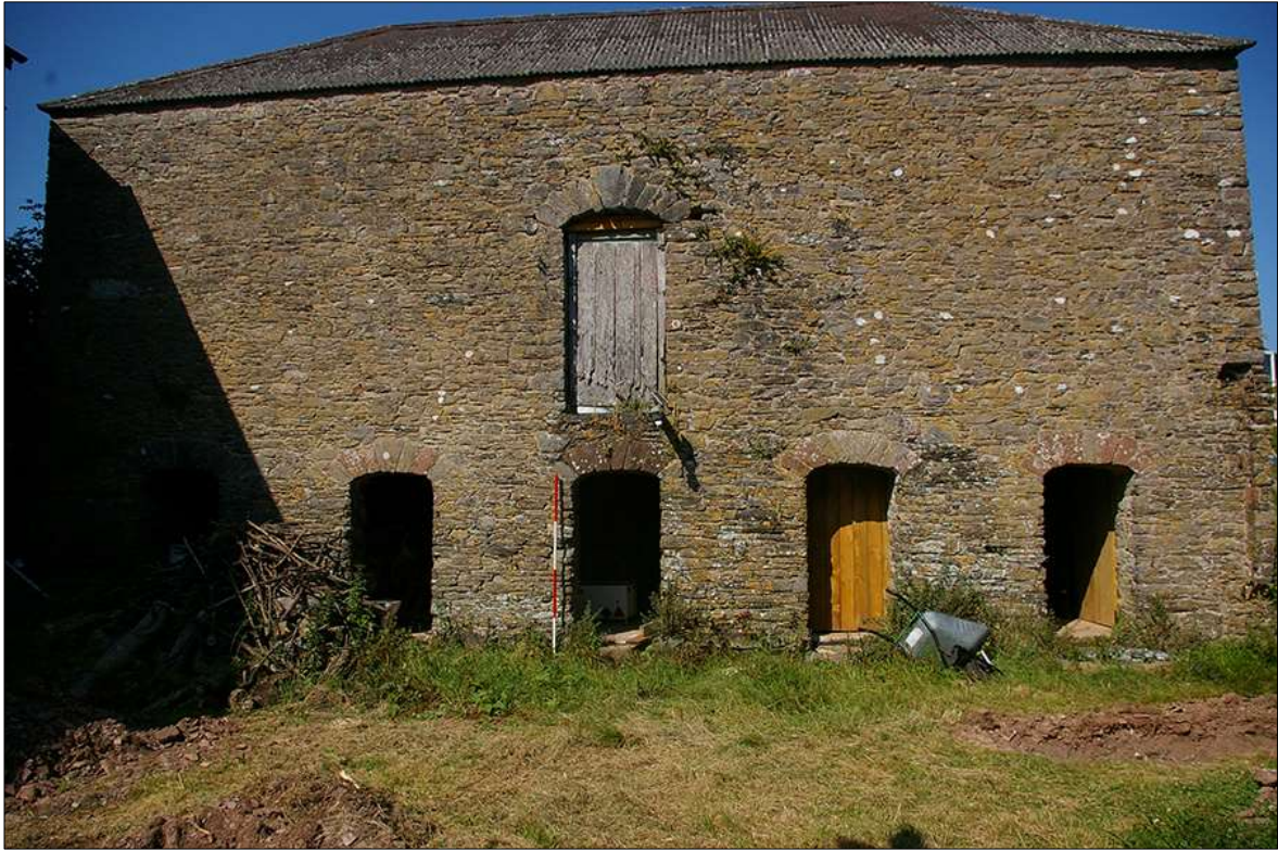
89. THE SOUTH-WEST ELEVATION OF B2; VIEWED FROM THE SOUTH-WEST (2M SCALE).
