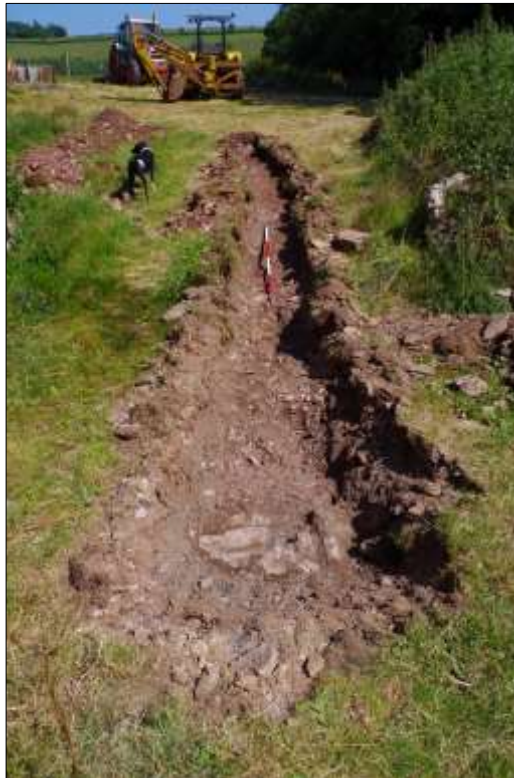
6. TRENCH 03, POST-EXCAVATION; VIEWED FROM THE NORTH-WEST (2M SCALE).
