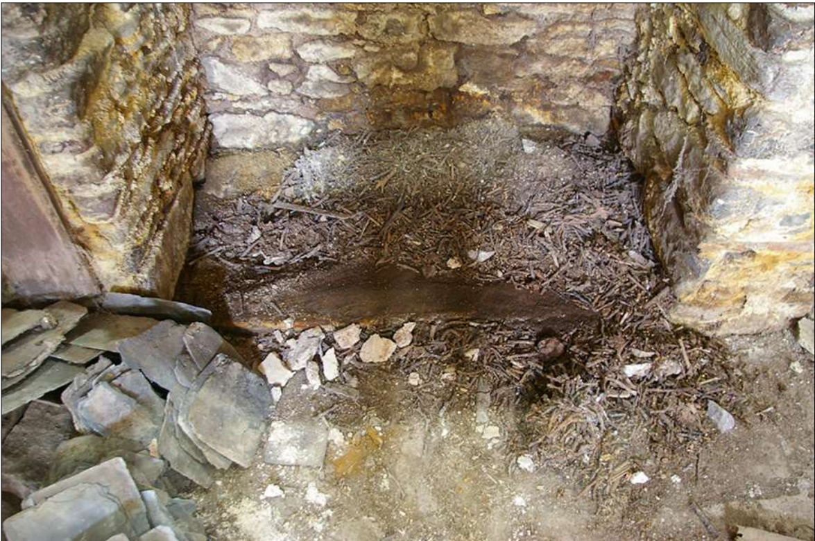
66. DETAIL OF THE LIME MORTARED BRICK HEARTH OF FP2; VIEWED FROM THE SOUTH-WEST.
