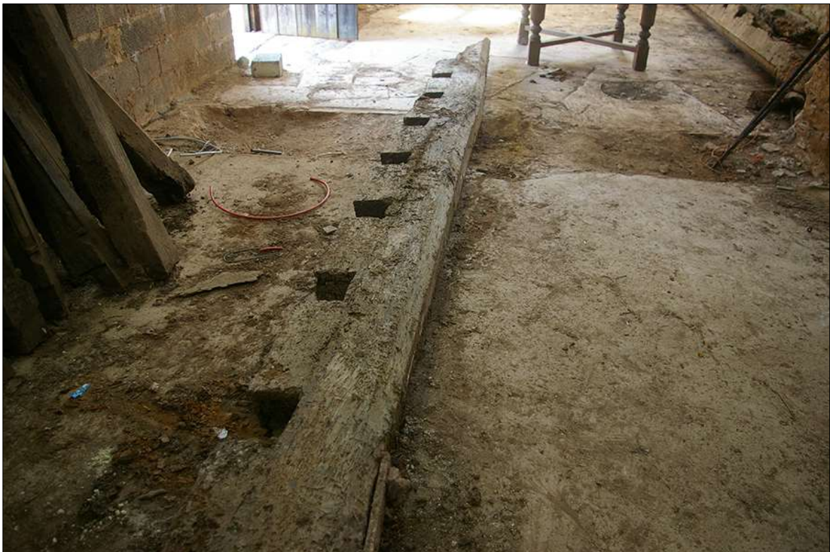
57. DETAIL OF ONE OF THE EX SITU PLAIN CHAMFERED BEAMS; VIEWED FROM THE NORTH-EAST.
