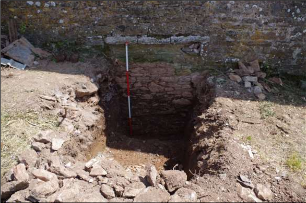
3. BLOCKING OF WINDOW W3 IN THE NORTH-WEST ELEVATION OF B1, AS SEEN WITHIN TRENCH 01; VIEWED FROM THE NORTH-WEST (2M SCALE).
