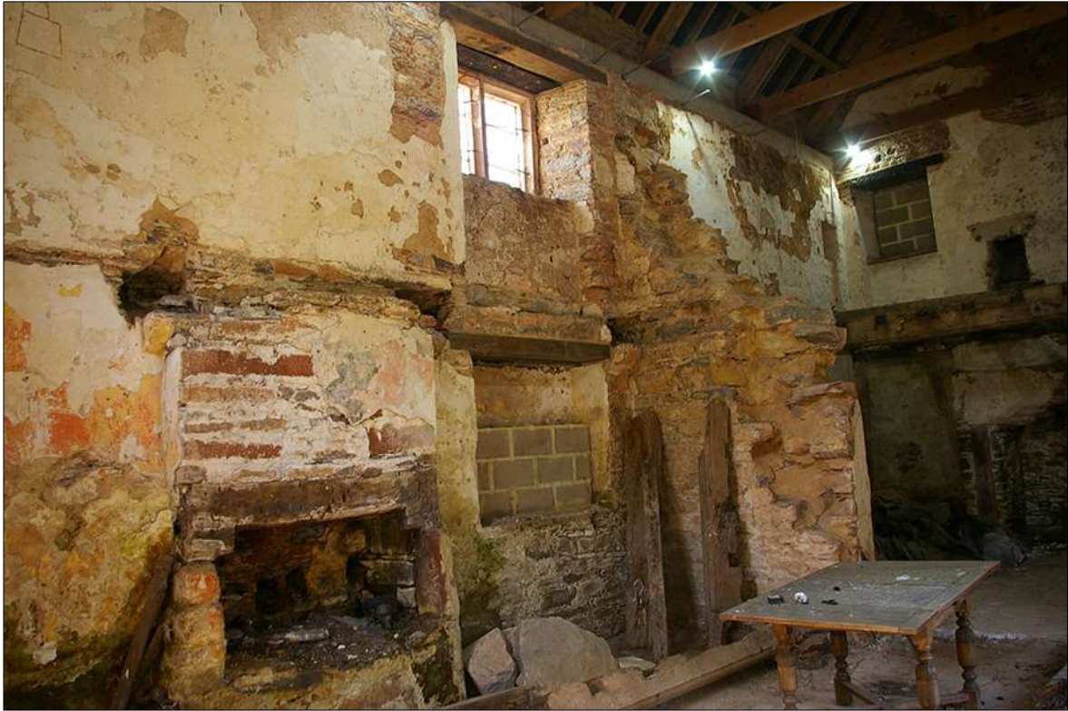
29. THE INTERIOR FACE OF THE NORTH-WEST WALL OF B1, MID, SHOWING FIREPLACE FP1, BLOCKED WINDOWS W3 AND W4 AND THE CROSS-WALL; VIEWED FROM THE SOUTH.
