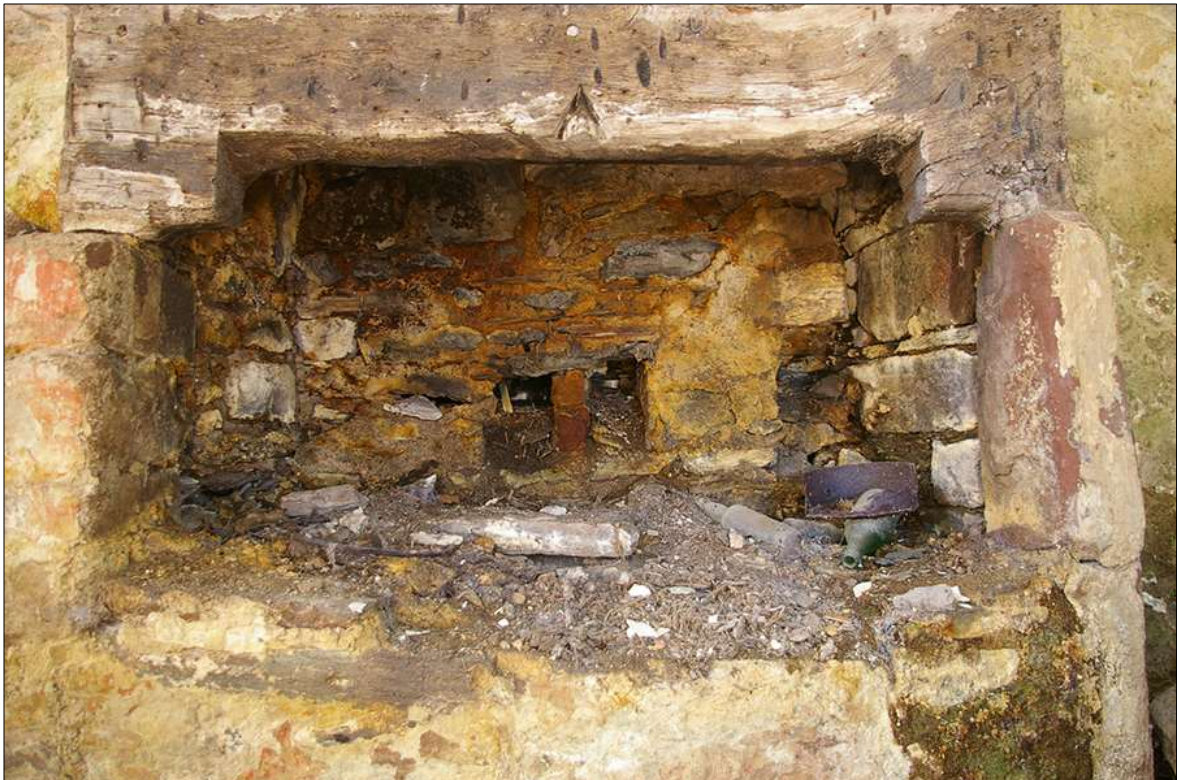
47. DETAIL OF THE HEARTH OF FIREPLACE FP1; VIEWED FROM THE SOUTH-EAST.
