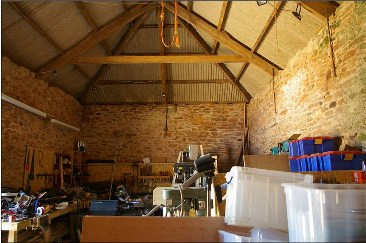
100. DETAIL OF THE ROOF STRUCTURE OF B2; VIEWED FROM THE NORTH-WEST.
