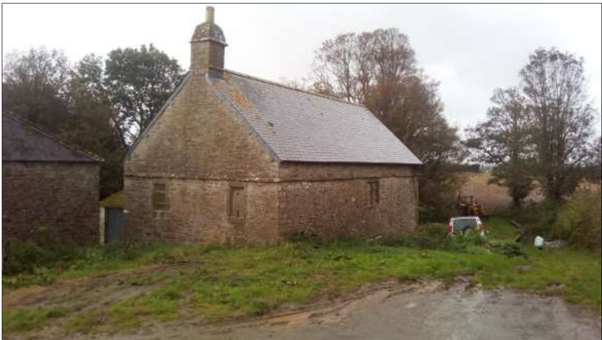
2. VIEW TOWARDS WEEK (B1 & B2) AT THE END OF THE HEDGE-LINED APPROACH; VIEWED FROM THE NORTH.
