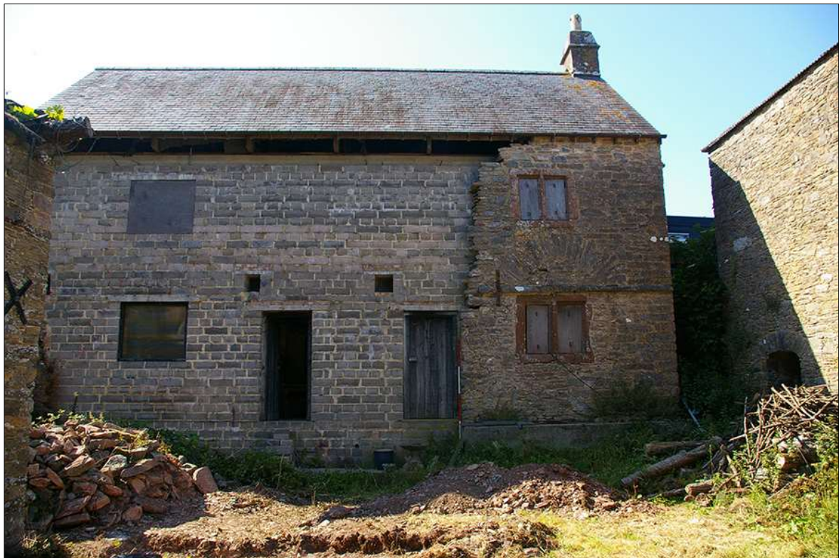
24. THE SOUTH-EAST ELEVATION OF B1; VIEWED FROM THE SOUTH-EAST (2M SCALE).
