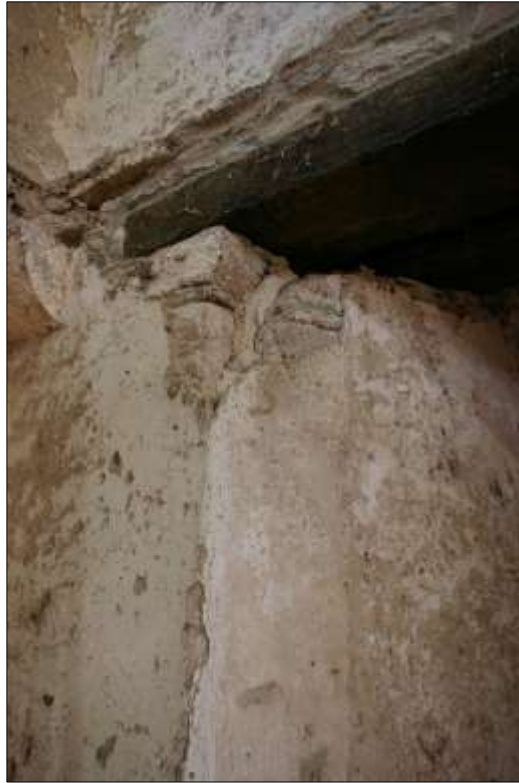
69. DETAIL OF THE RUBBLE INFILL OF THE BLOCKED DOORWAY BUILT OVER THE EARLIER HAIR COB AND LIME PLASTER TO CREATE WINDOW W7; VIEWED FROM THE WEST-SOUTH-WEST.
