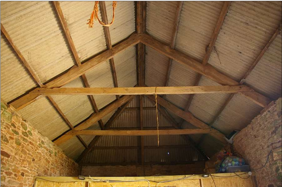
99. THE A-FRAME TRUSS ROOF STRUCTURE OF B2; VIEWED FROM THE SOUTH-EAST.
