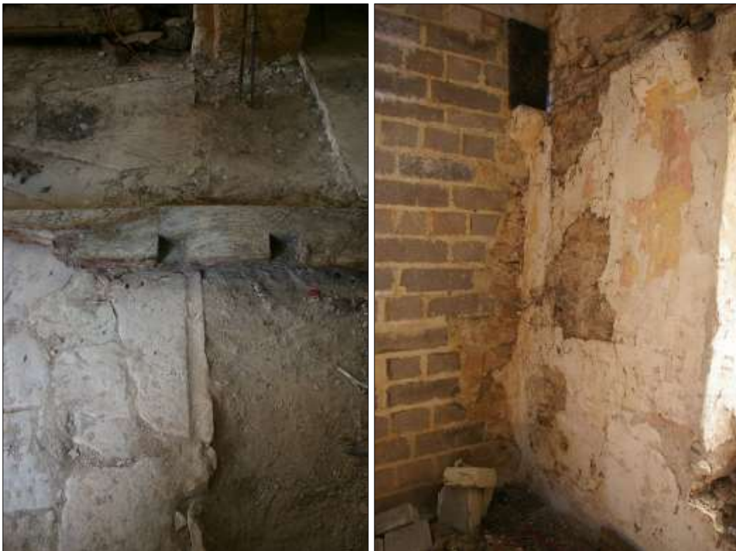
40. (LEFT) DETAIL OF THE REBATE IN THE FLAGSTONE FLOOR OF THE SOUTH-WEST GROUND-FLOOR ROOM OF B1, SUGGESTING THE POSITION OF AN EARLIER SCREEN DIVISION; VIEWED FROM THE SOUTH-EAST.
