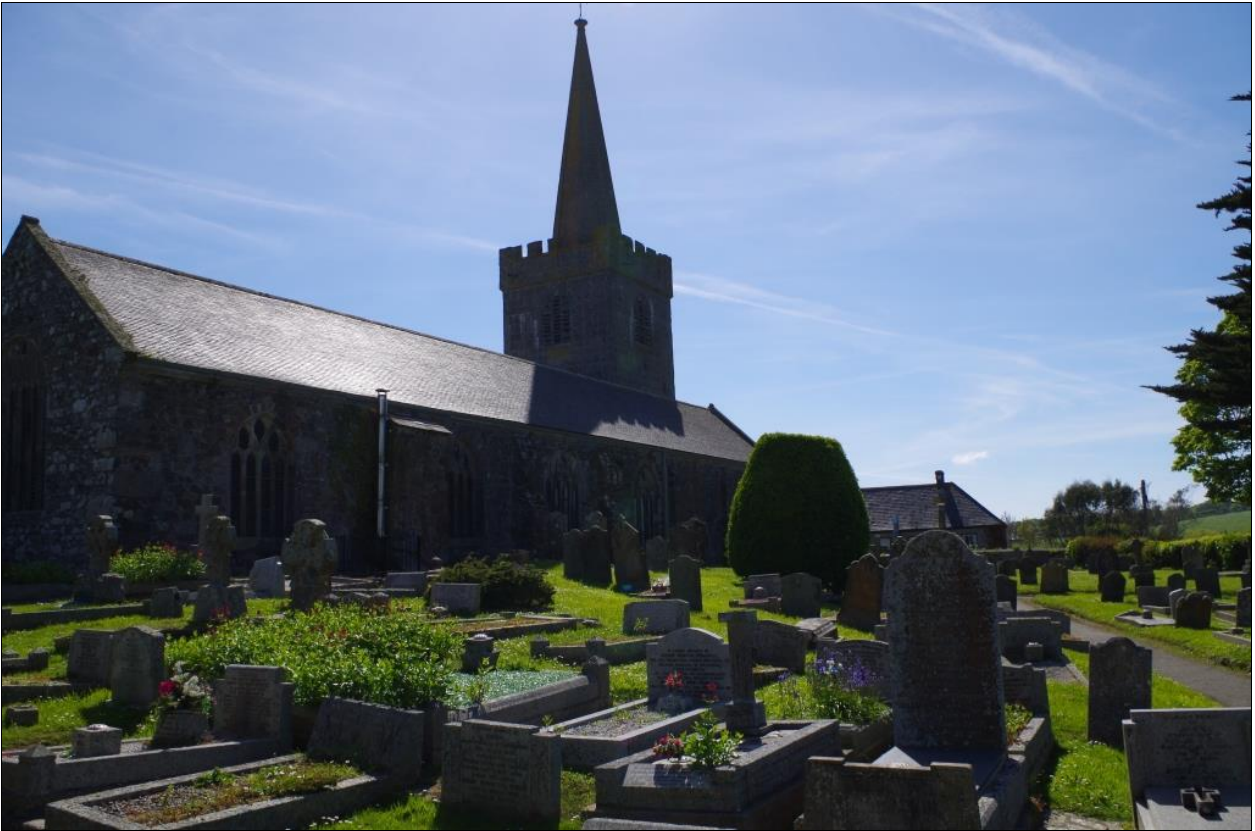
PHOTO 9: VIEW OF ST KEVERNE CHURCH, VIEWED FROM THE NORTH-EAST.
