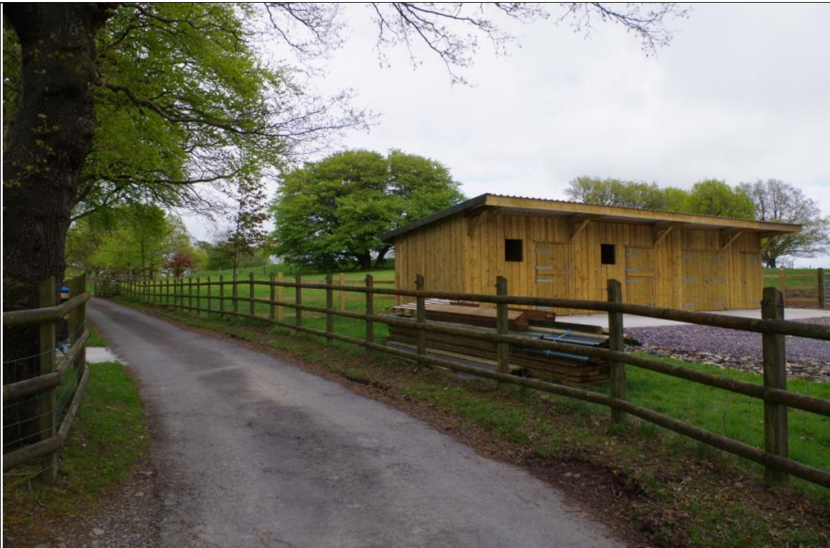
FIGURE 6: AS ABOVE, FROM THE WEST-NORTH-WEST.
