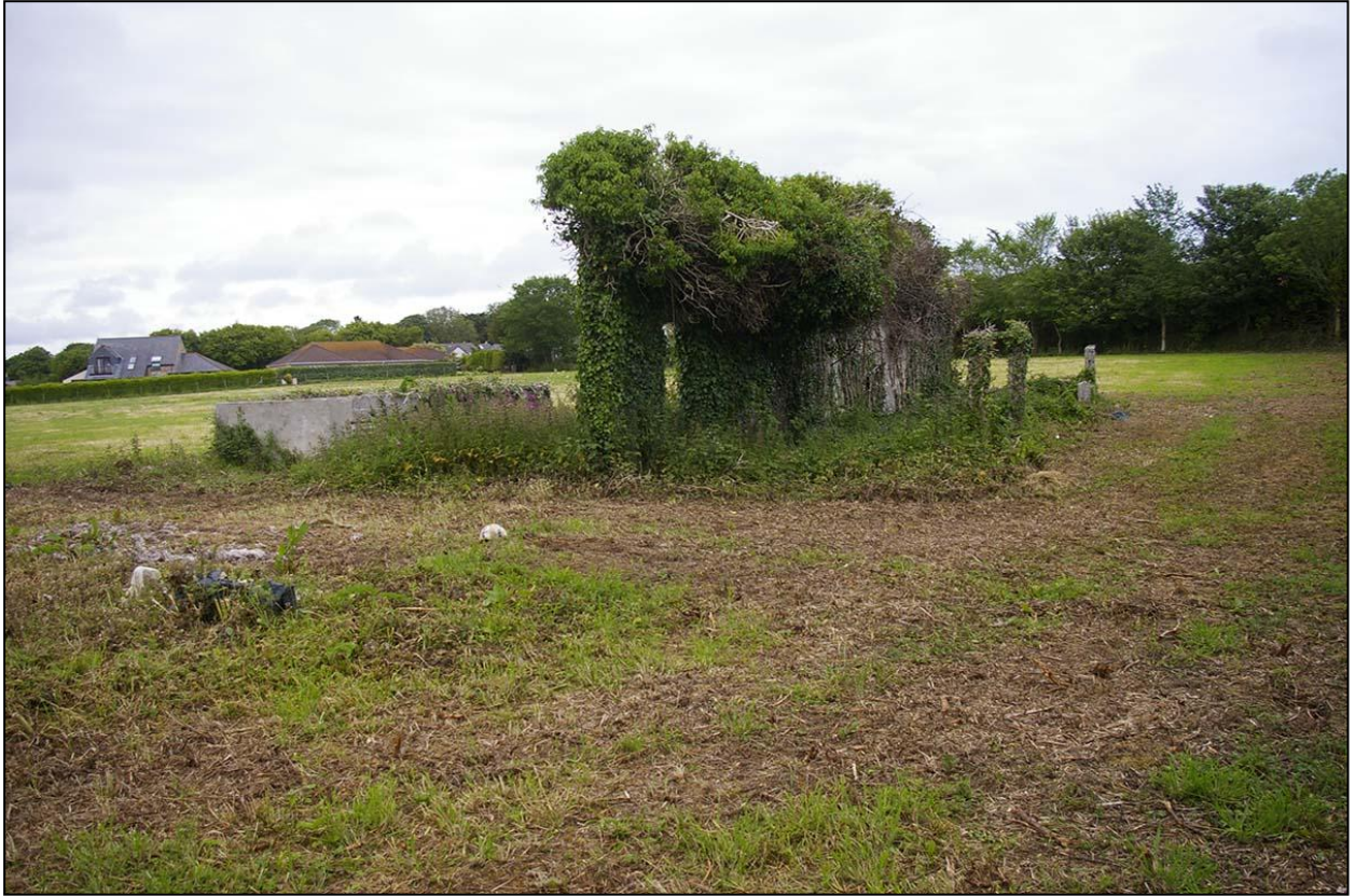
DETAIL OF THE 20 TH CENTURY STRUCTURE; VIEWED FROM THE WEST.
