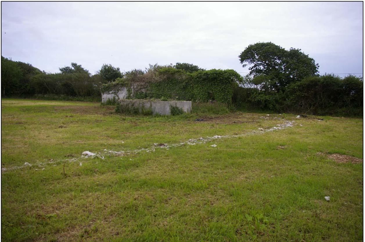
DETAIL OF THE REMAINS OF THE 20 TH CENTURY STRUCTURE; VIEWED FROM THE NORTH.
