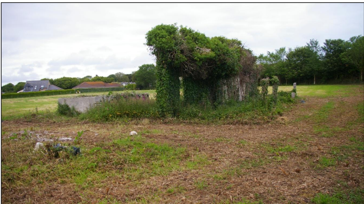
FIGURE 7: DETAIL OF THE CONCRETE-BLOCK STRUCTURE; VIEWED FROM THE SOUTH-WEST.
