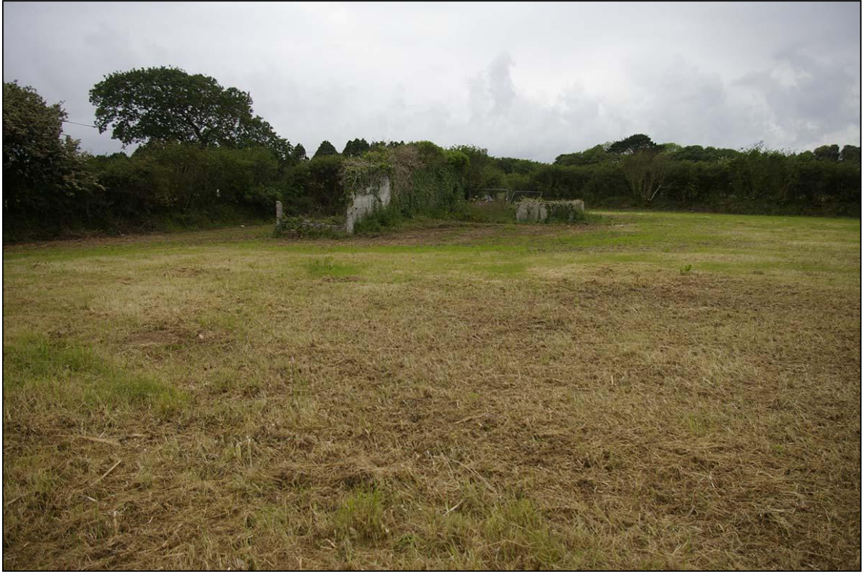
DETAIL OF THE 20 TH CENTURY STRUCTURE AT THE SOUTHERN END OF THE SITE; VIEWED FROM THE EAST.
