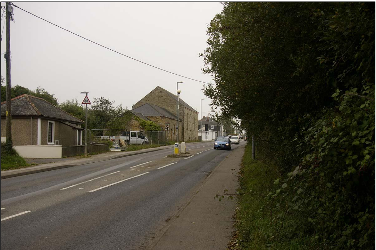
VIEW OF THE CHURCH FROM THE ROAD PARALLEL TO FIELD 1; VIEWED FROM THE NORTH.
