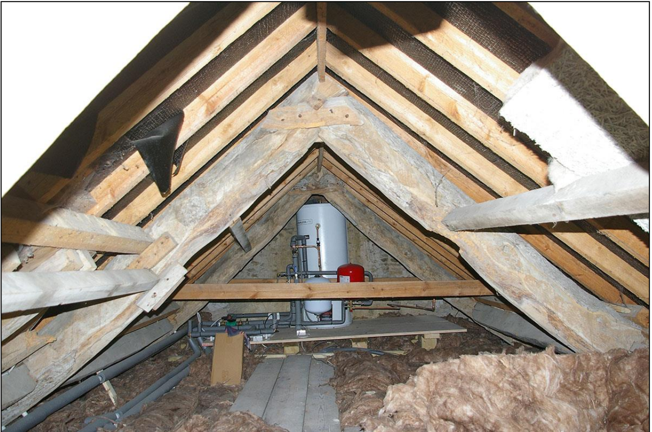
R17, THE LOFT SPACE SHOWING TWO TRUSSES AND LOOKING THROUGH THE THIRD; VIEWED FROM THE WEST.
