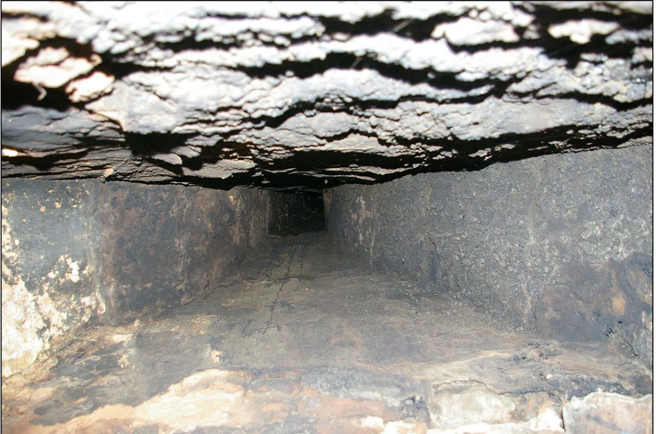
R2, VIEW UP THE FLUE; VIEWED FROM BELOW.
