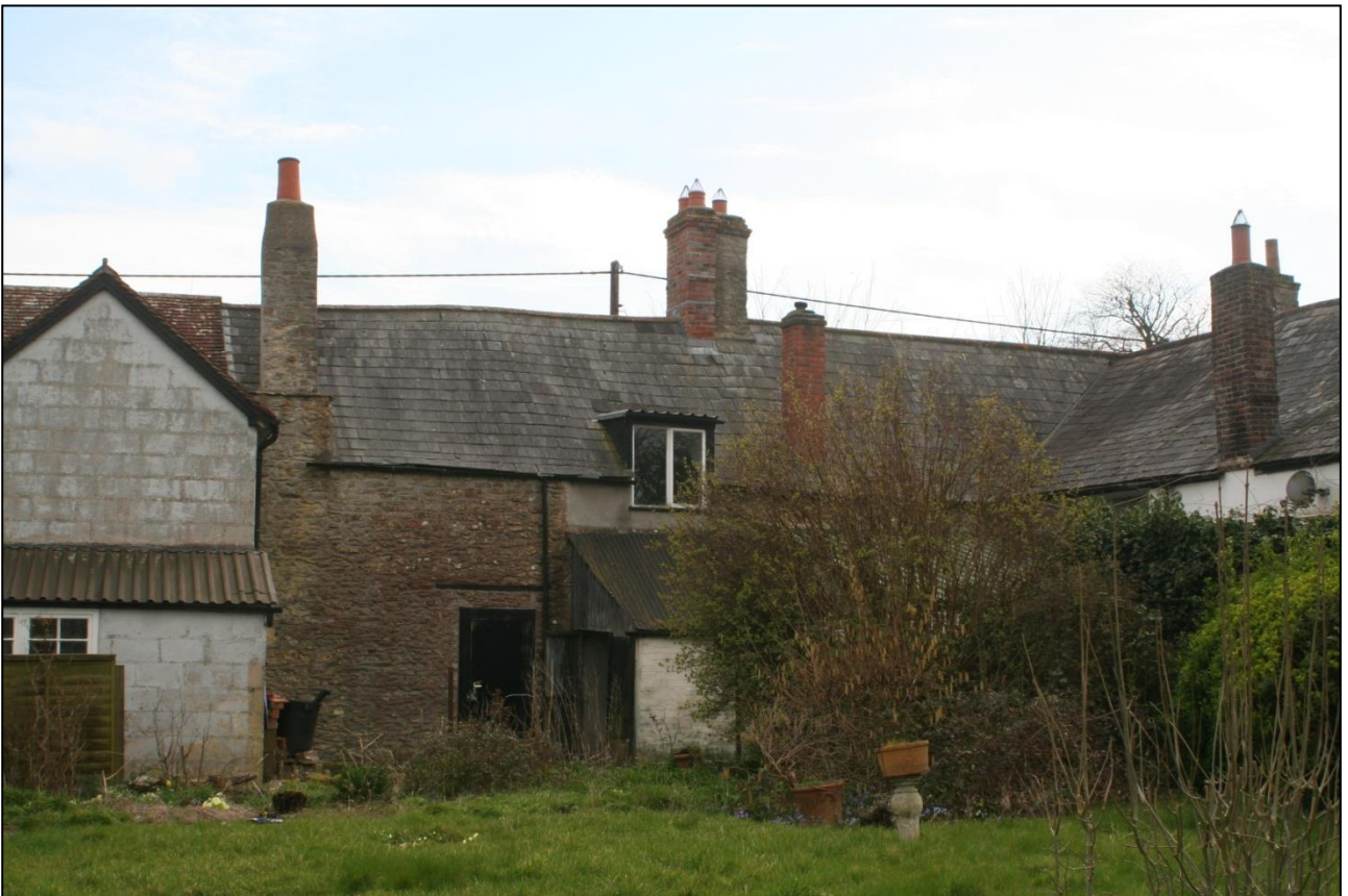
THE NORTH ELEVATION WHERE IT ADJOINS THE OLD BAKEHOUSE; VIEWED FROM THE NORTH-EAST; SUPPLIED BY CLIENT.
