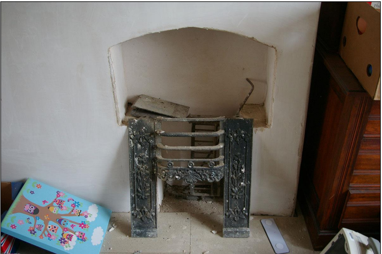
R15, THE FINE SMALL LATE 18 TH CENTURY OR EARLY 19 TH CENTURY HOB GRATE; VIEWED FROM THE EAST.
