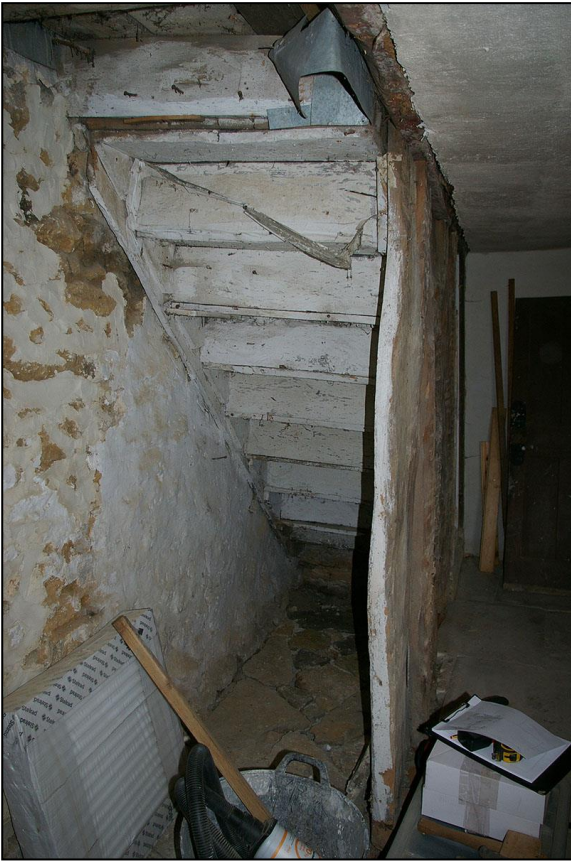
LEFT: R2, THE STAIRS (R14) SUPPORTED AND ENCLOSED BY A HEAVY RUSTIC SCREEN, WITH LOOSER RANDOM STONE PAVING BENEATH; VIEWED FROM THE SOUTH-SOUTH-EAST.
