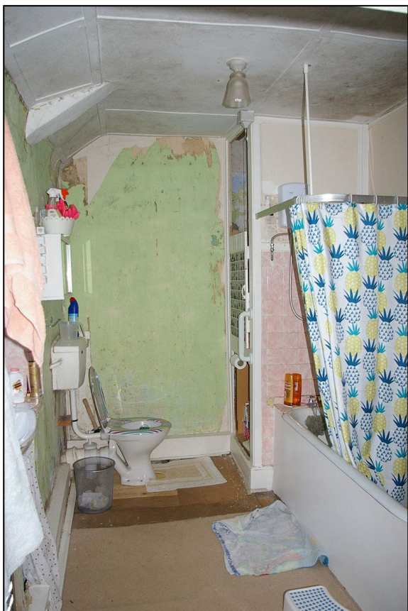
LEFT: R12; VIEWED FROM THE WEST.
