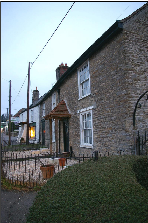
VIEW ALONG THE FRONT ELEVATION OF THE LONG RANGE, SHOWING THE DIFFERENCE IN ALIGNMENT THAT IDENTIFIES THESE AS SEPARATE STRUCTURES; VIEWED FROM THE EAST.
