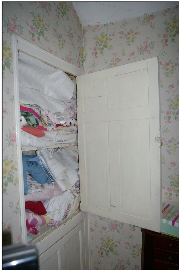
LEFT: R11, THE 18 TH CENTURY PANELLED CUPBOARD SET INTO AN ALCOVE AGAINST THE STACK, AND THE SMALL EDWARDIAN GRATE INSERTED INTO THE FIREPLACE, LIKELY BLOCKING A LARGER OPENING; VIEWED FROM THE WEST-SOUTH-WEST.
