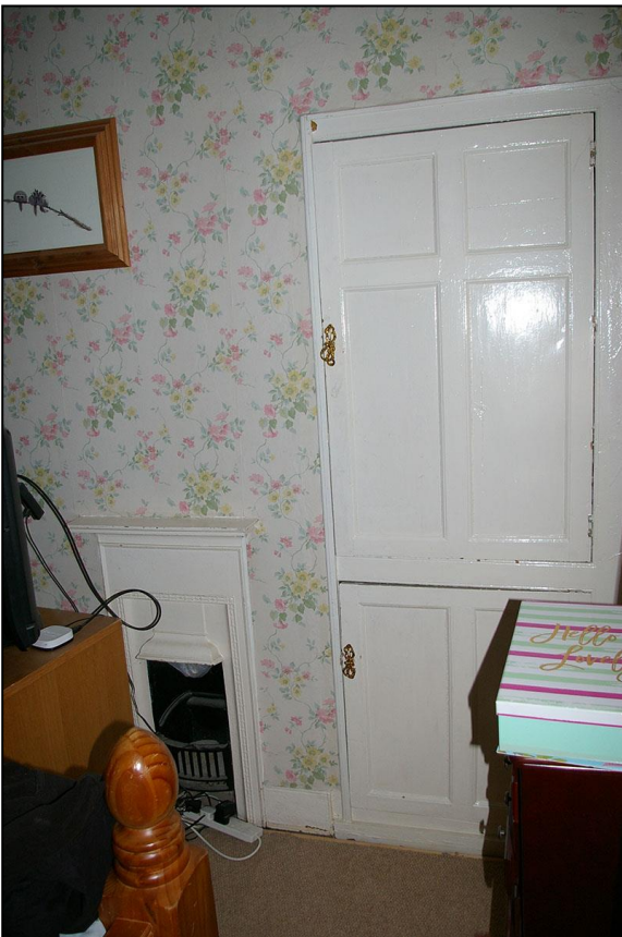
LEFT: R11, THE 18 TH CENTURY PANELLED CUPBOARD SET INTO AN ALCOVE AGAINST THE STACK, AND THE SMALL EDWARDIAN GRATE INSERTED INTO THE FIREPLACE, LIKELY BLOCKING A LARGER OPENING; VIEWED FROM THE WEST-SOUTH-WEST.
