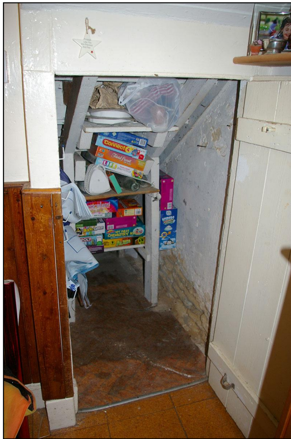
RIGHT: R5, THE UNDERSTAIR CUPBOARD, SHOWING THE CHUNKY PLANK AND TREAD RISERS CARRIED ON CARRIAGE BRACES, A TYPICAL 18 TH CENTURY FORM OF STAIR CONSTRUCTION; VIEWED FROM THE NORTH-NORTH-EAST.
