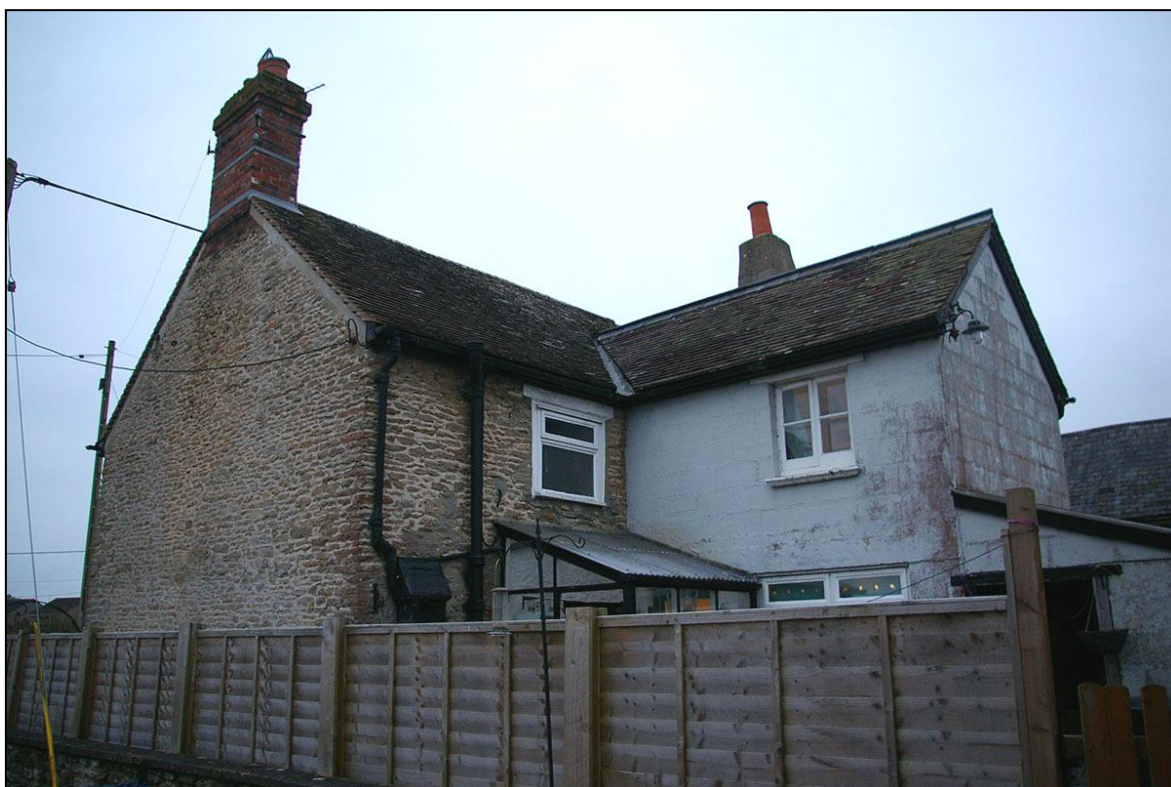
FIGURE 7: THE EAST GABLE AND REAR BLOCKWORK EXTENSION; VIEWED FROM THE NORTH-EAST.
