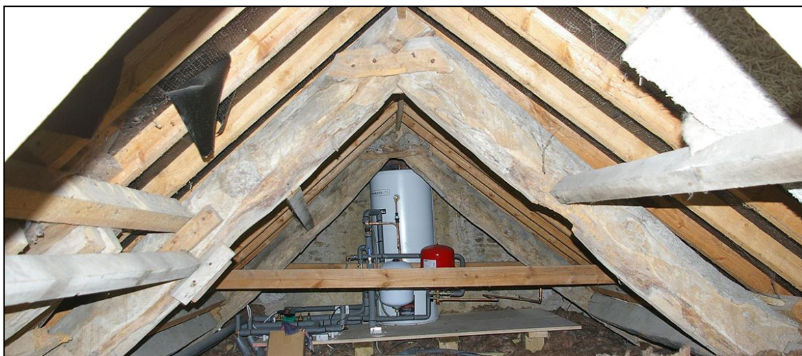
FIGURE 16: THE EASTERN ROOF TRUSSES IN R17; VIEWED FROM THE WEST.
