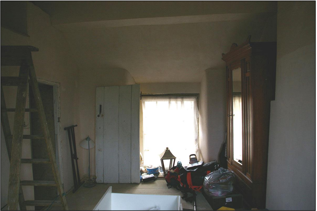
R15, THE SOUTH WALL; VIEWED FROM THE NORTH.
