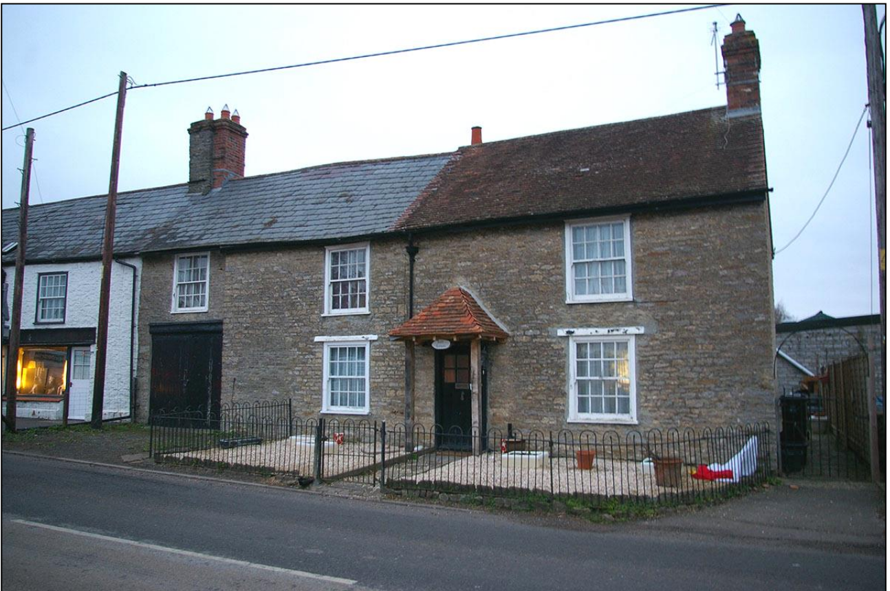
THE SOUTH ELEVATION OF ASH HOUSE; VIEWED FROM THE SOUTH-EAST.
