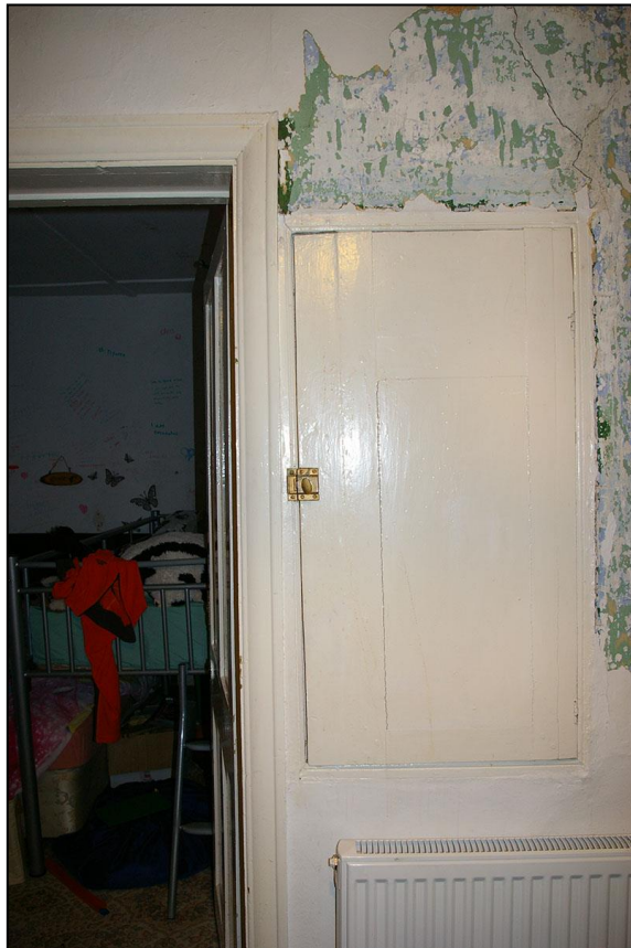
RIGHT: R9, THE SMALL CUPBOARD WITH MOULDED FRAME AND UNEVEN PLANK DOOR SET INTO THE SIDE OF THE LATERAL STACK; VIEWED FROM THE EAST.
