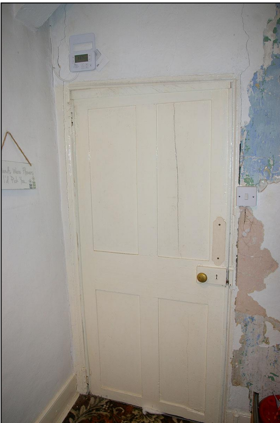
LEFT: R9, FINE 18 TH CENTURY RAISED AND FIELDED PANELLED DOOR ON LH HINGES TO R12, NOW A BATHROOM; VIEWED FROM THE WEST. RIGHT: R9, THE PANELLED SIDE OF THE DOOR TO R12; VIEWED FROM THE WEST.
