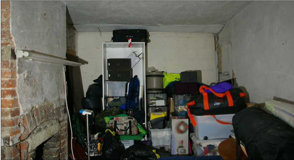
FIGURE 12: THE GARAGE, ROOM 3, SHOWING THE BRICK STACK ADDED AGAINST THE ADJACENT HOUSES' GABLE END WALL; FROM THE SOUTH.
