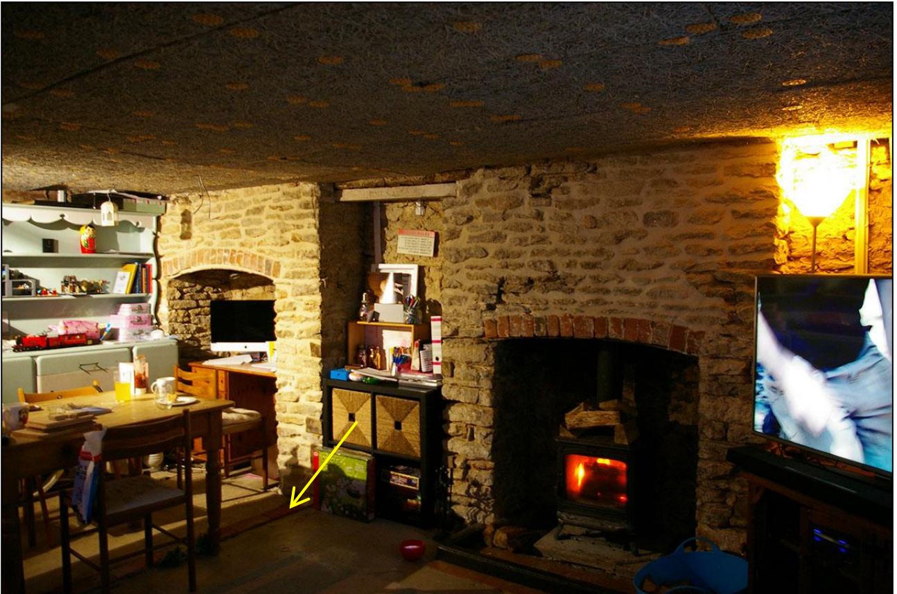
R4, FORMED BY THE REMOVAL OF A BRICK PARTITION (INDICATED), WITH TWO STONE STACKS; VIEWED FROM THE SOUTH-WEST.
