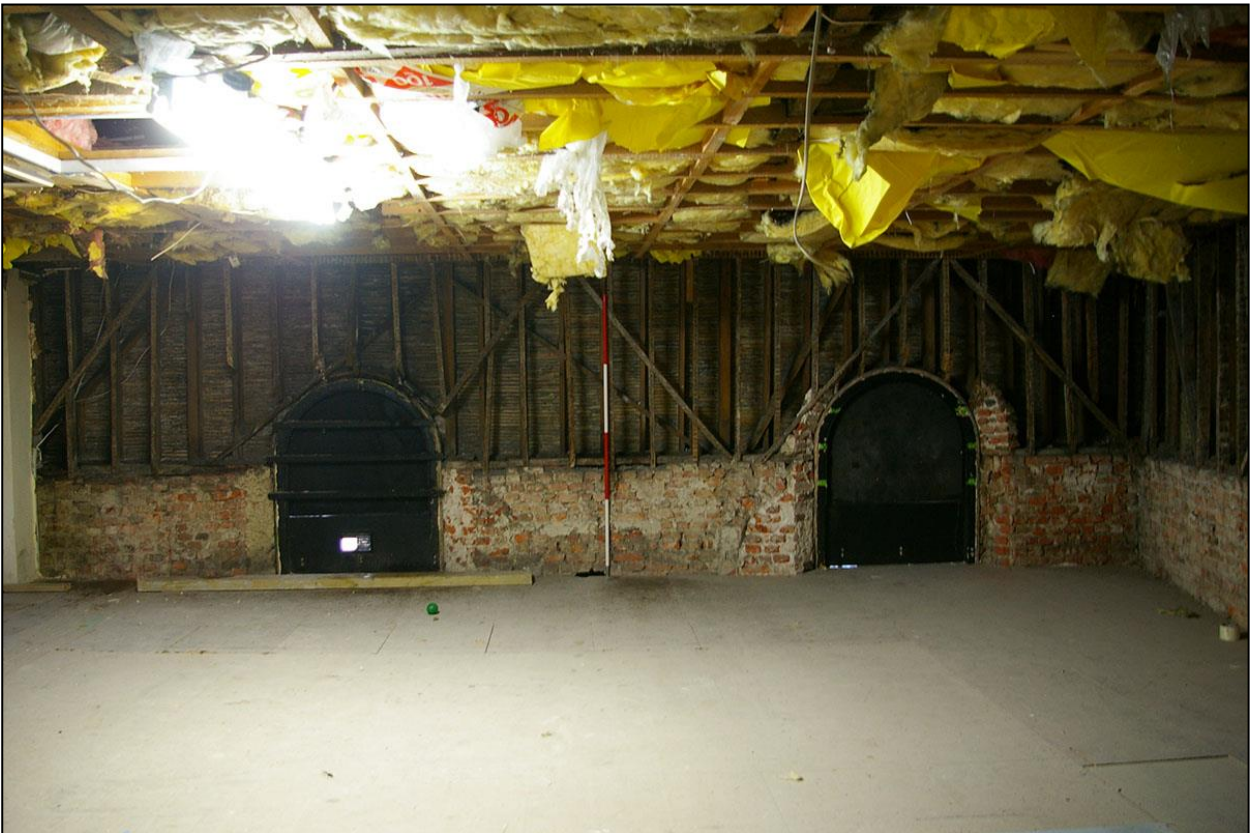
THE TOP OF THE EAST WALL OF THE SYNAGOGUE, ROOM 9, SHOWING THE TOP OF THE ROUND ARCHED PAIR OF WINDOWS AND THE RAISE IN STUDWORK ABOVE; FROM THE WEST (2M SCALE).
