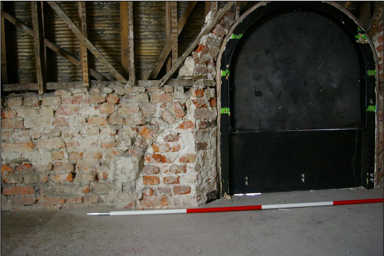
DETAILED VIEW SHOWING THE EARLIER, LOWER AND NARROWER ROUND ARCHED WINDOWS, FROM THE FIRST SYNAGOGUE, RAISED BY THE STUDWORK AND ENLARGED IN THE 19 TH CENTURY; FROM THE WEST (2M SCALE).
