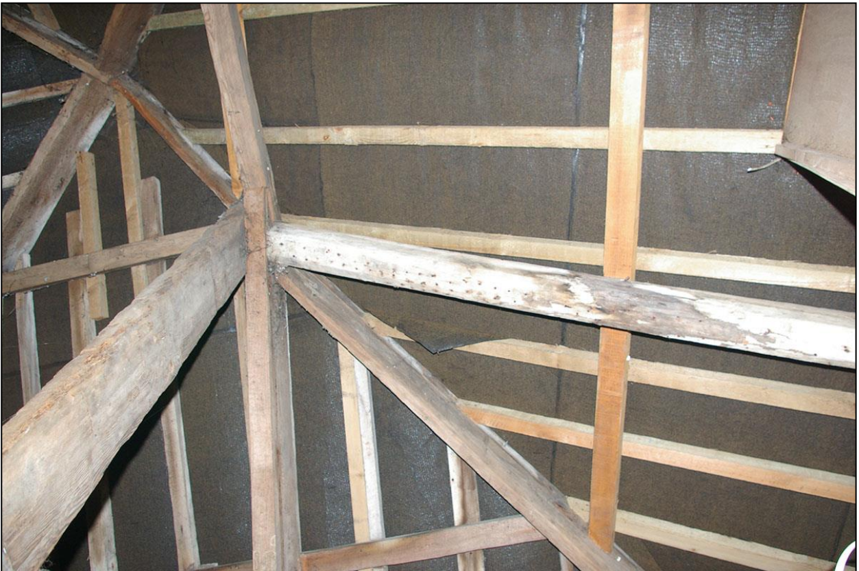
THE COMPOSITE TIMBER ROOF STRUCTURE ABOVE THE SYNAGOGUE.
