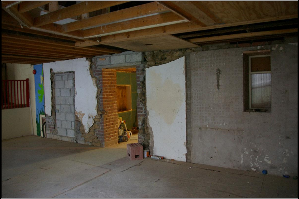
THE FORCED OPENING IN THE EAST WALL LEADING TO THE CONCRETE LINKING STRUCTURE; FROM THE SOUTH-WEST.
