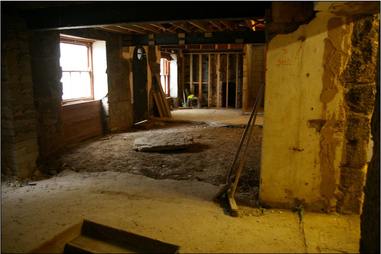
VIEW FROM ROOM 1, INTO ROOM 6; FROM THE SOUTH-EAST.
