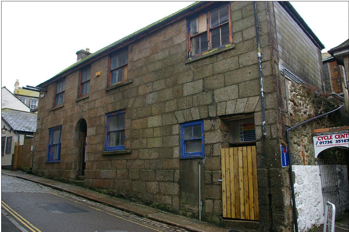
FIGURE 2: THE WEST, ASHLAR FRONTAGE OF 1 NEW STREET; FROM THE WEST-SOUTH-WEST.
