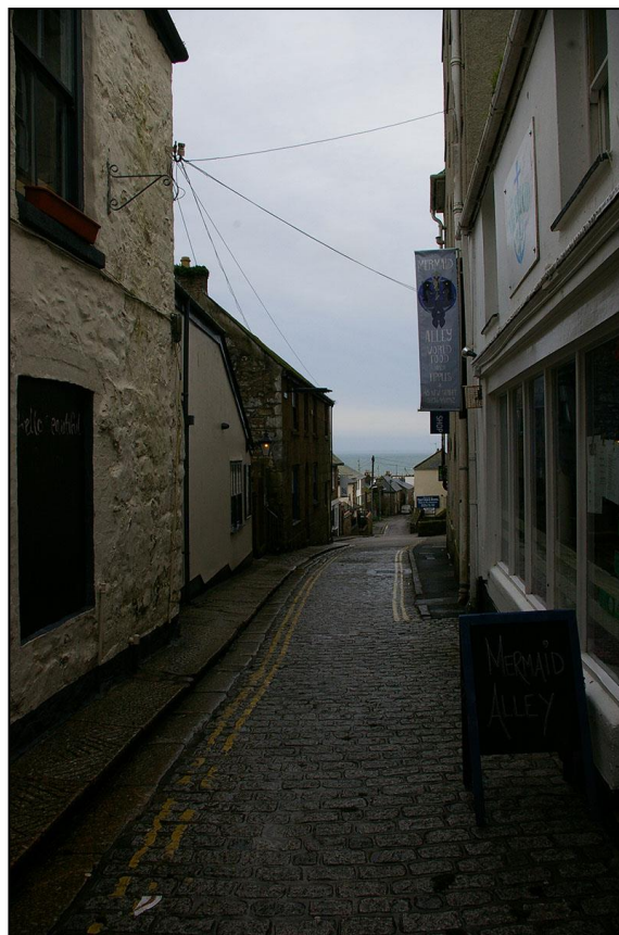
VIEW OF NEW STREET SHOWING HOW IMPORTANT NO.1 IS TO THE STREETScape WITH ITS ASHLAR FACADE; FROM THE NORTH.
