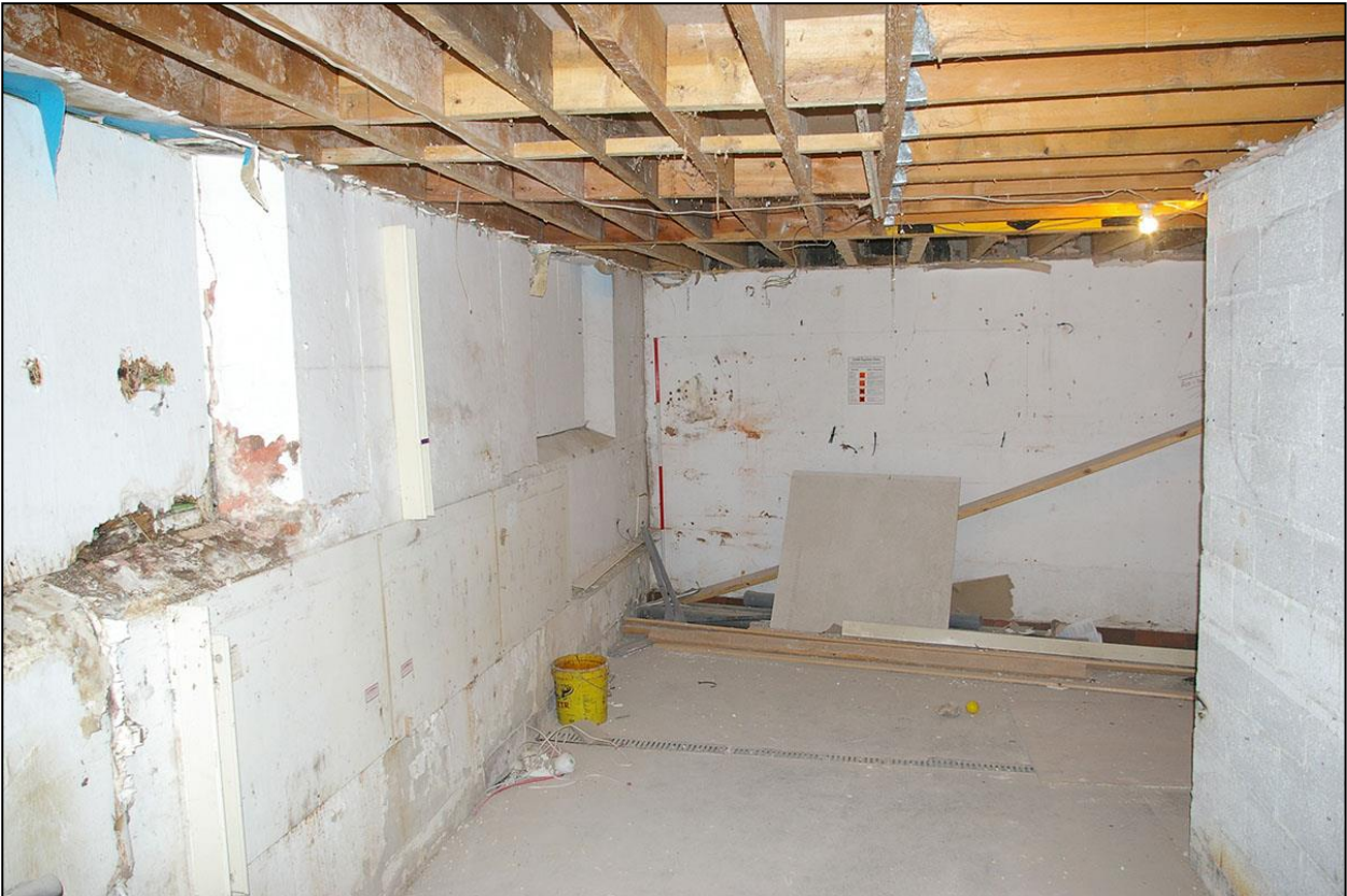
THE EAST AND SOUTH PLASTERED BRICKWORK WALLS OF THE SYNAGOGUE, WITH FLASH; FROM THE NORTH (2M SCALE).
