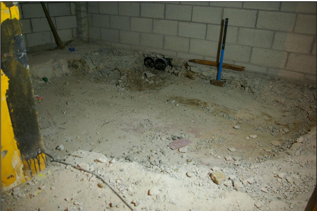
THE CONCRETE BLOCK EXTENSION ON THE NORTH OF ROOM 5, WITH RAISED CONCRETE FLOOR SHOWING DEEP MODERN LAYERS, WITH A MID 20 TH CENTURY LINO SURFACE BURIED BEHIND MORE RECENT CONCRETE; FROM THE SOUTH-EAST.
