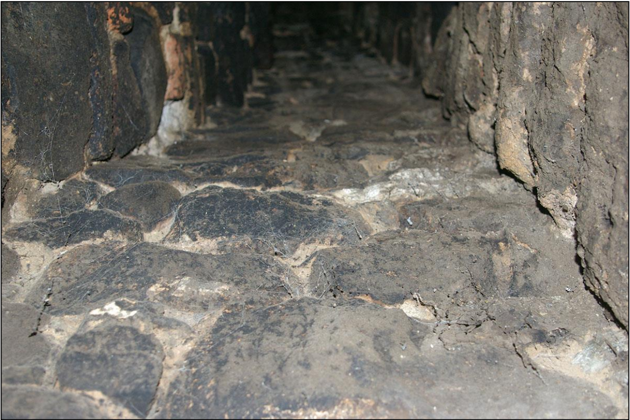
VIEW UP THE SMOKE-BLACKENED, TAPERED STACK; FROM BELOW.
