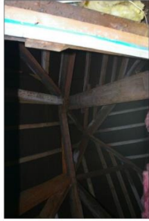
Roof structure to be removed to allow for new roof structure.
