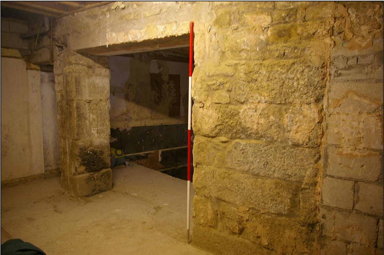
THE COURSED MASSIVE GRANITE SLAB STONEWORK OF THE EXTENSION TO THE SOUTH END OF NO.1 NEW STREET, SEEN IN ROOM 2, INFILL BEHIND THE HISTORIC BUILDING, A FORMER OPEN YARD; FROM THE NORTH-EAST (2M SCALE).
