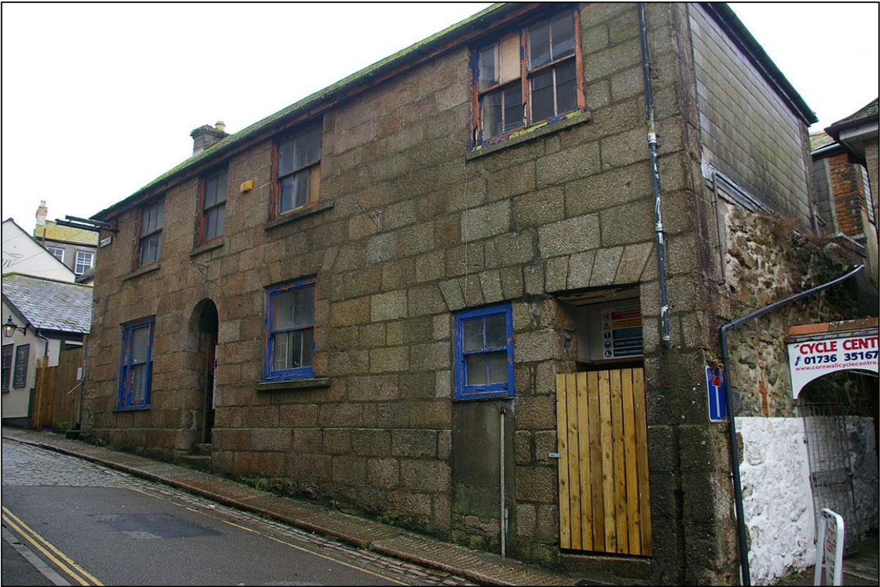
NO.1 NEW STREET, WITH SYMMETRICAL DOOR AND WINDOW TO THE NORTH AND WINDOW AND BLOCKED CARRIAGE ARCH TO THE SOUTH END; FROM THE WEST, SOUTH-WEST.
