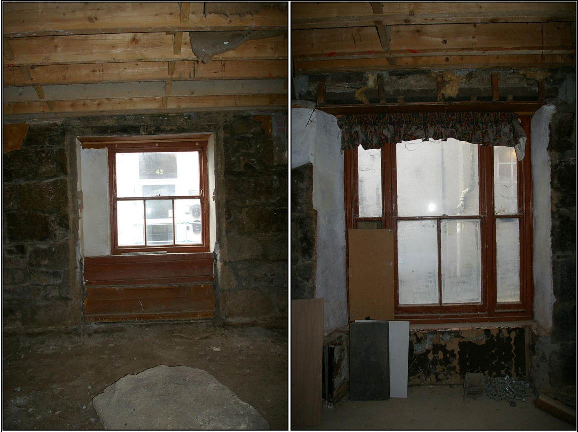
LEFT: THE WINDOW TO THE SOUTH, SET WITHIN A PARTIALLY BLOCKED OPENING, THIS PHASING NOT VISIBLE ON THE ASHLAR FRONTAGE; FROM THE EAST.
