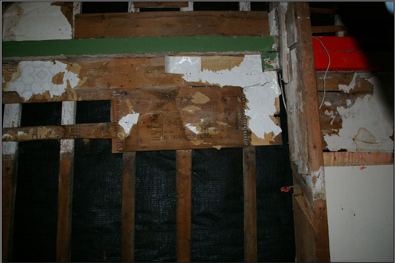
19 TH CENTURY LYLES SUGAR BOX, NAILED TO THE ROOF TIMBERS, FORMING SARK BOARDING; FROM THE EAST.
