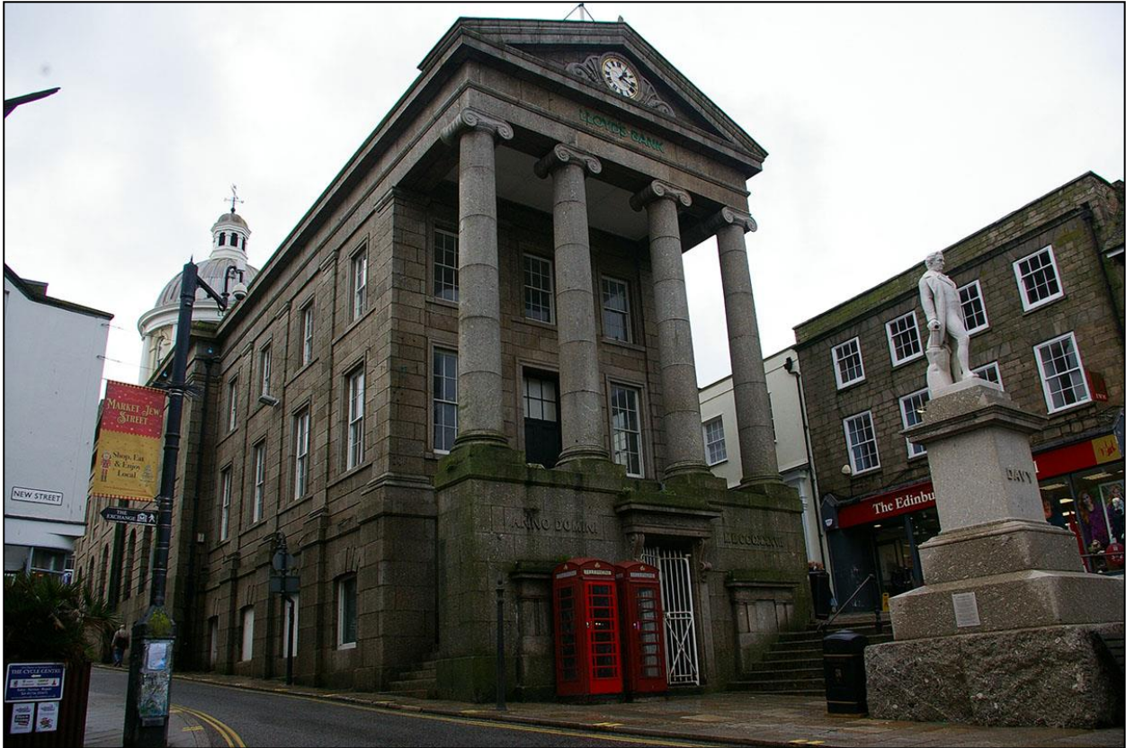
THE MARKET HALL, ON MARKET JEW STREET, A GRADE I LISTED 19 TH CENTURY, OPPOSITE THE STAR INN; FROM THE EAST, SOUTH-EAST.
