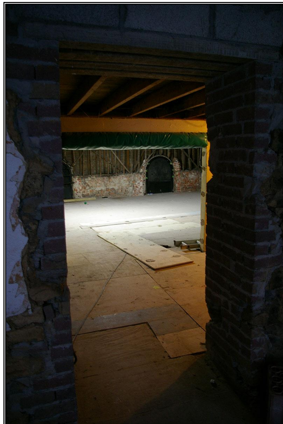
VIEW THROUGH THE OPENING IN THE EAST WALL OF ROOM 7, THROUGH ROOM 8 TO ROOM 9, THE FORMER SYNAGOGUE; FROM THE WEST.
