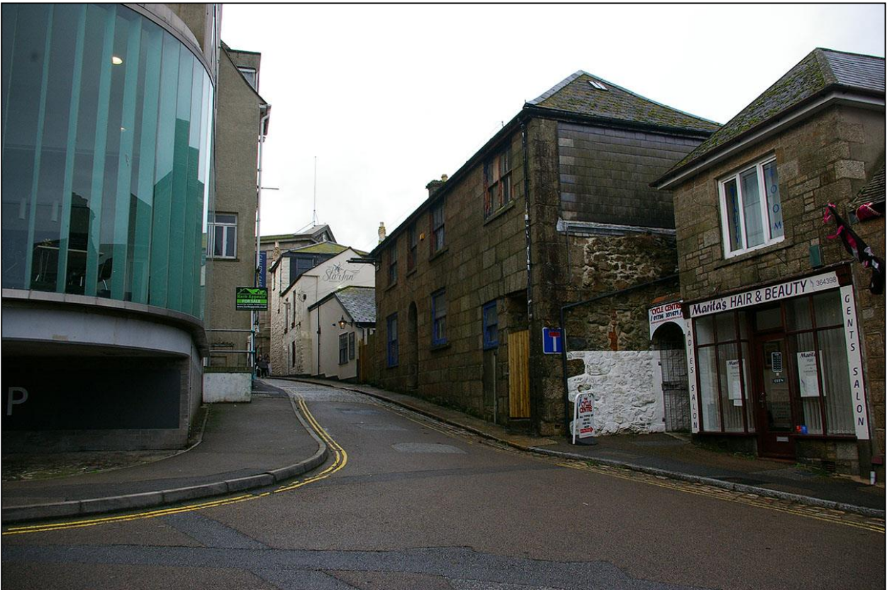
VIEW OF NO.1 NEW STREET FROM THE JUNCTION WITH PRINCES STREET; FROM THE SOUTH-WEST.
