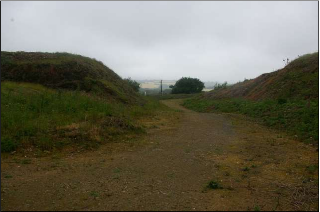
41. VIEW OUT OF THE MAIN NORTHERN QUARRY PIT, SHOWING THE PRESENT BUT LIMITED VIEW OUT TO THE LANDSCAPE TO THE WEST; FROM THE EAST.
