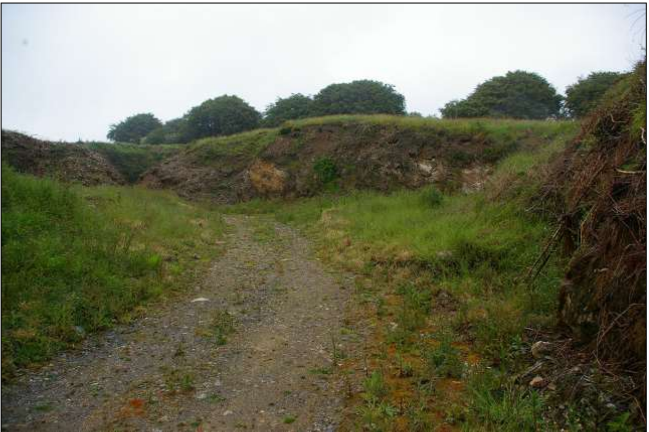
42. VIEW OF THE SMALLER SOUTHERN OF THE TWO MAIN QUARRY PITS AND THE CUT THROUGH LINK TO THE MAIN AREA; FROM THE WEST.
