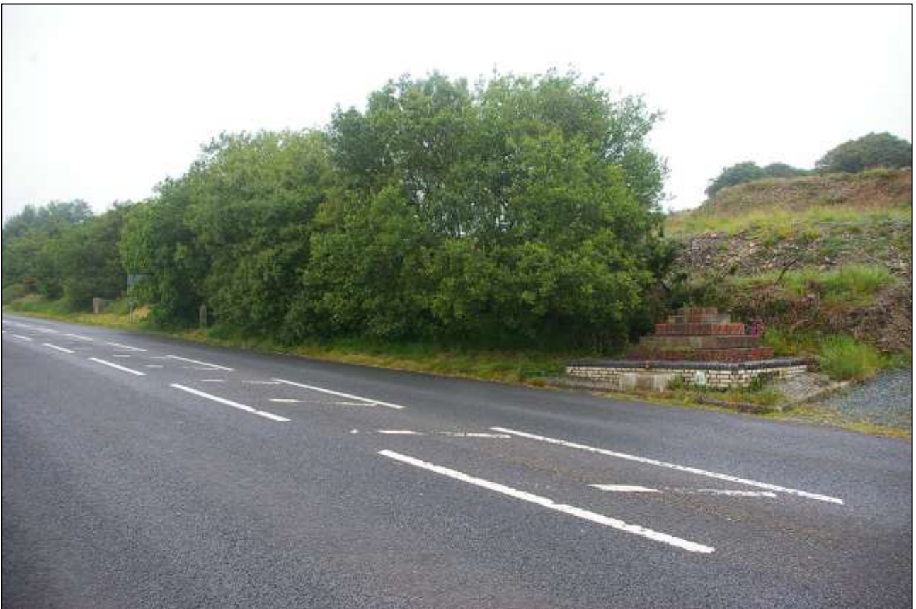
12. VIEW OF THE FOUNTAIN AND LISTED MILESTONE, DEMONSTRATING THEIR ROADSIDE SETTING ON THE WEST BOUNDARY OF THE QUARRY; FROM THE SOUTH-WEST.
