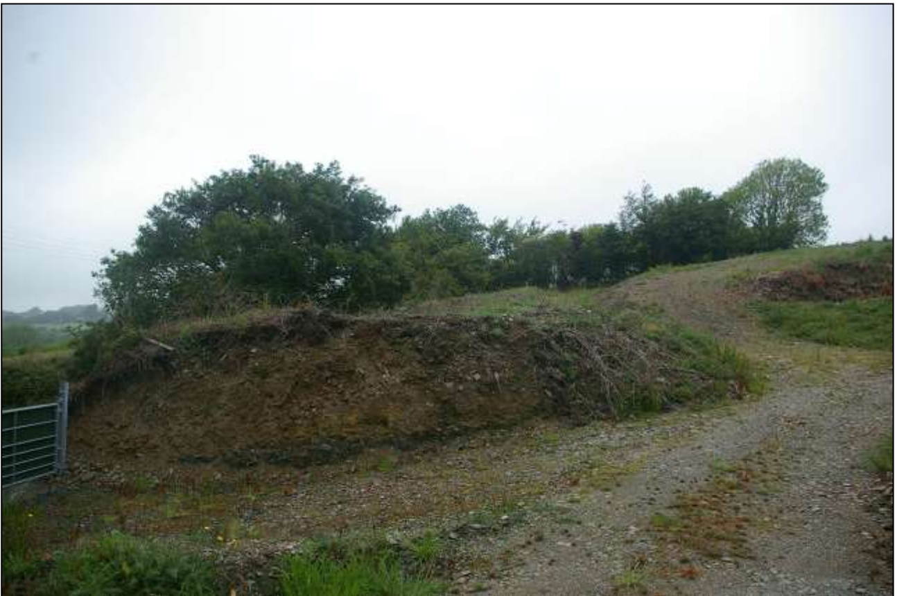
18. DETAIL OF THE SLUMPS OF QUARRY WASTE AGAINST THE HISTORIC BOUNDARY BANK IN THE NORTH-WEST CORNER OF THE SITE; FROM THE SOUTH.
