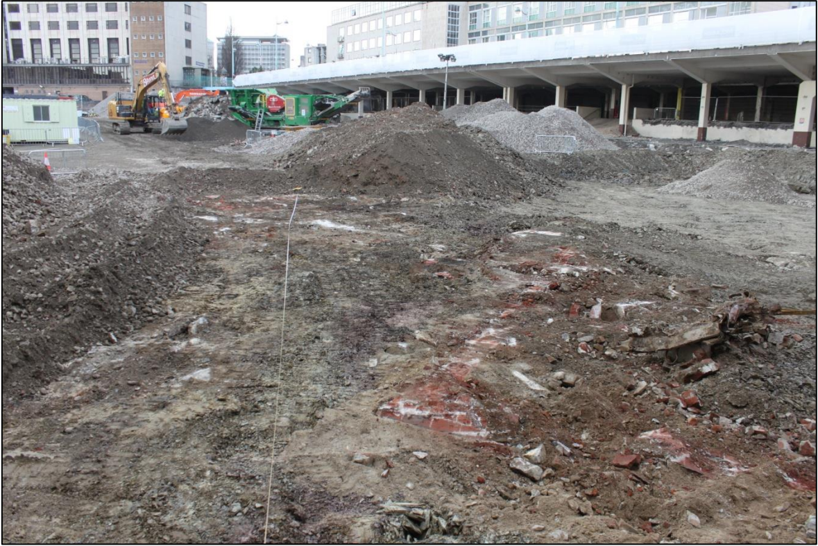
WALLS {142}; VIEWED FROM THE NORTH-EAST (NO SCALE).
