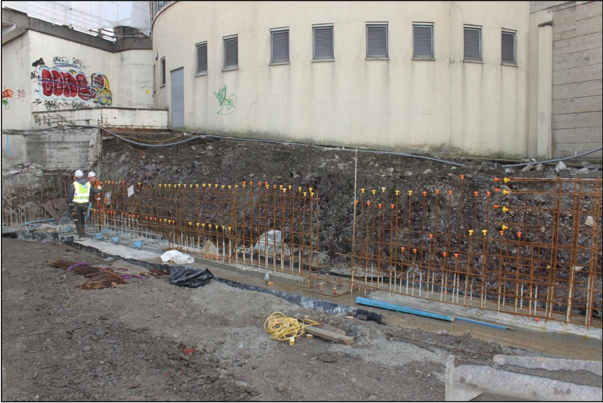
GENERAL SITE SHOT DURING GROUNDWORKS; VIEWED FROM THE SOUTH (NO SCALE).
