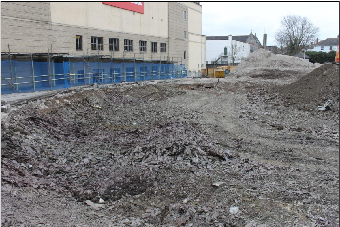
GENERAL SITE SHOT DURING GROUNDWORKS; VIEWED FROM THE NORTH (NO SCALE).
