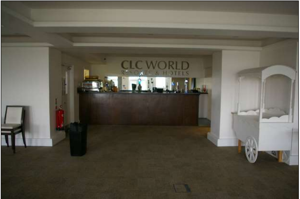
THE FORMER FRONT OF THE HOUSE, BETWEEN THE BAY WINDOWS, WHERE THE WALL OF THE HISTORIC BASEMENT HAS BEEN FORCED TO PROVIDE ACCESS BETWEEN THE OLD AND NEW SECTION UNDER THE UPPER TERRACE; FROM THE WEST.
