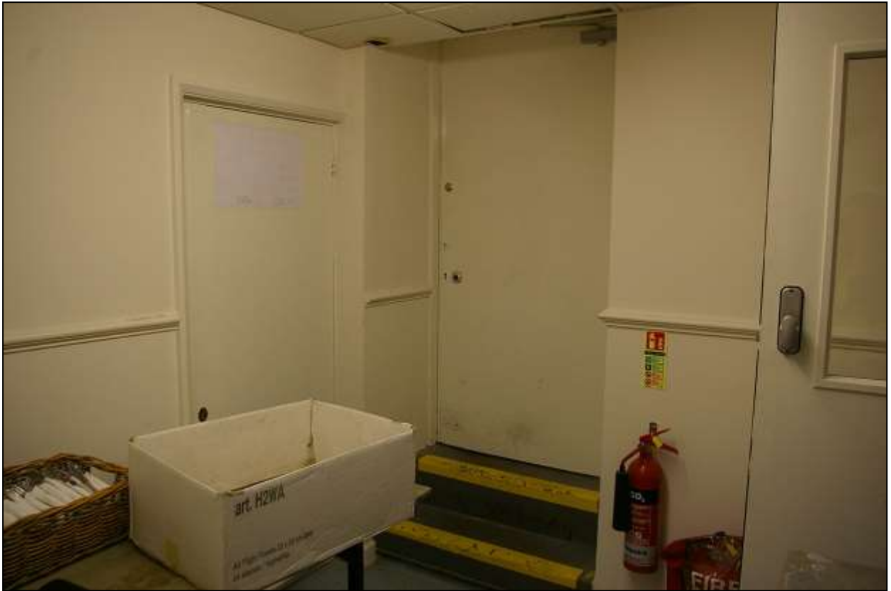
THE SMALL BAR SERVICE ROOM FORMED BY MODERN PARTITIONS AT THE BASE OF THE BASEMENT STAIRS; FROM THE SOUTH-WEST.
