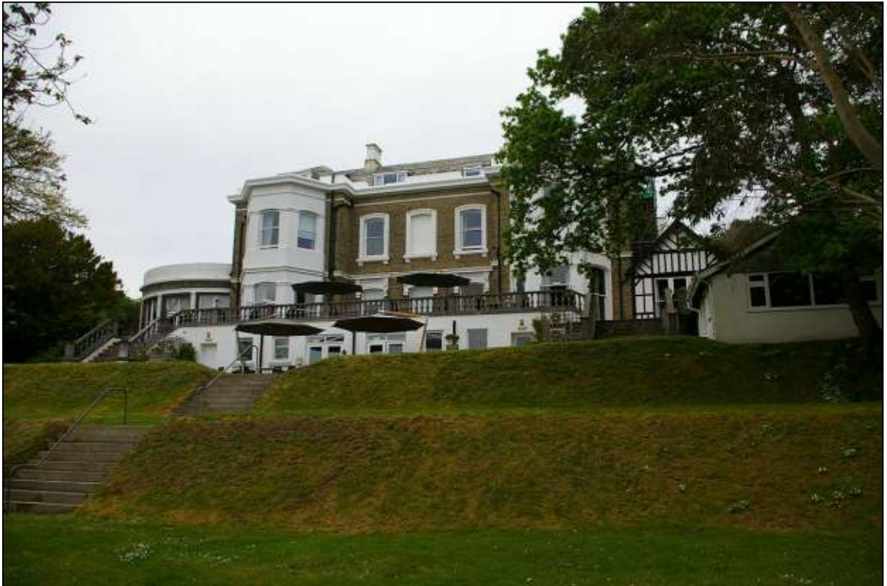
MORE DETAILED VIEW OF THE HOUSE AND ITS TERRACE, WITH THE VARIOUS DISPARATE EXTENSIONS TO NORTH AND SOUTH, ONE A ROUNDED CONSERVATORY, THE OTHER A TUDOR STYLE SERVICE WING; FROM THE SOUTH-WEST.
