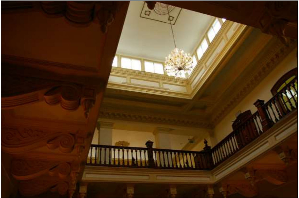
THE GLASS LANTERN OVER THE LOBBY OF THE HOTEL; FROM THE WEST, NORTH-WEST.
