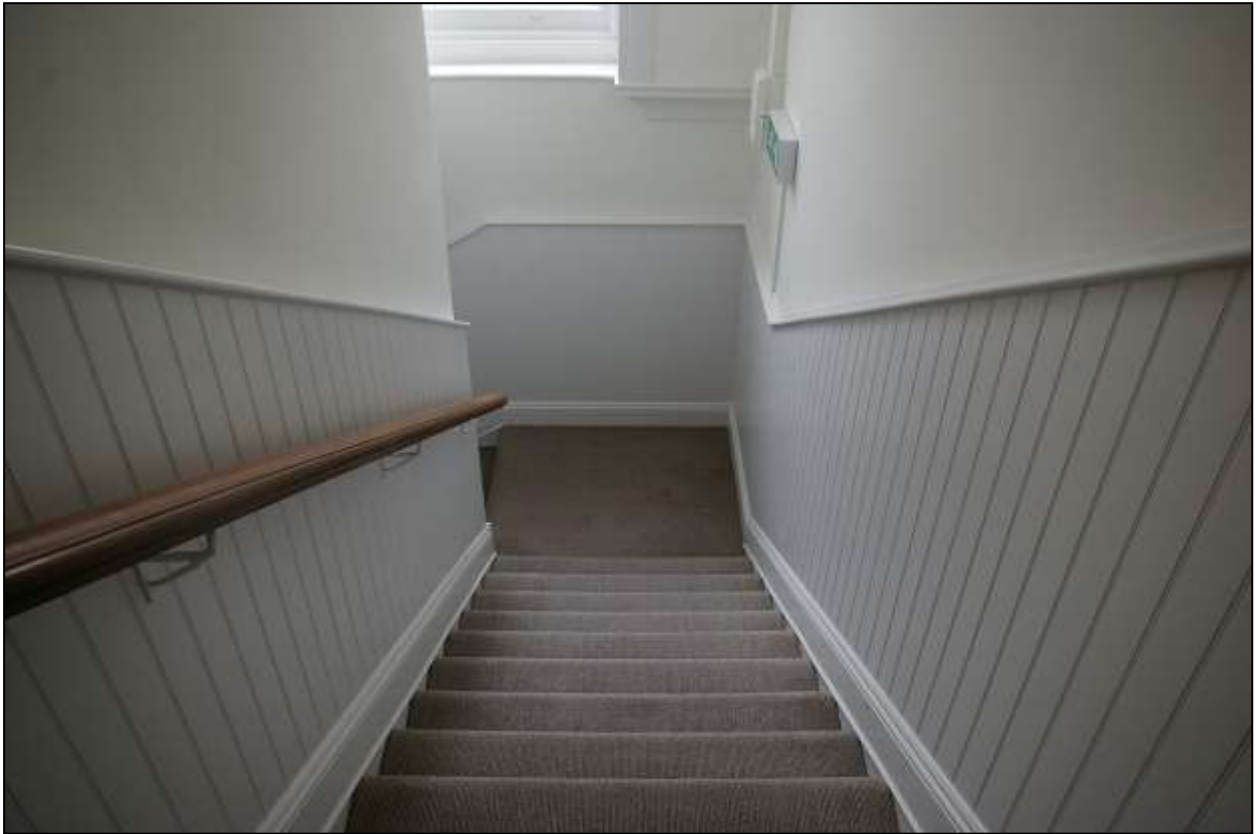
VIEW DOWN THE CARPETED STAIRS TOWARDS THE BASEMENT; FROM THE EAST.
