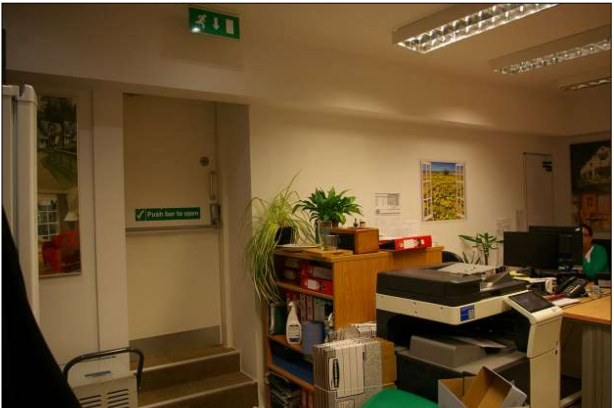
THE DOOR AND SET OF STEPS ACCESSING THE REST OF THE HISTORIC BASEMENT FROM THE MUCH MODERNISED OFFICE SPACE; FROM THE NORTH-WEST.
