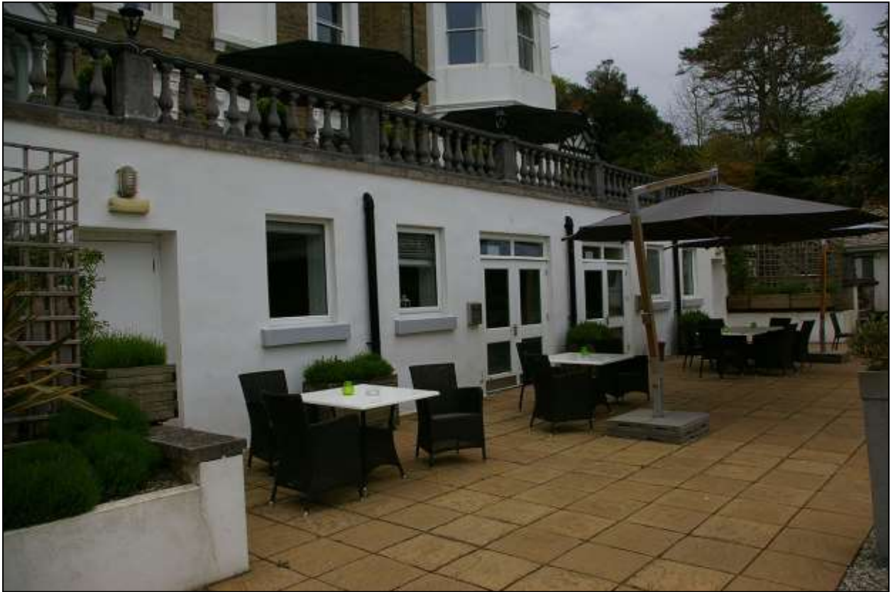
THE FRONT OF THE RELATIVELY MODERN UPPER TERRACE, WITH MODERN DOORS AND WINDOWS SET INTO THE WALL UNDER THE BALUSTRADE, SHOWING THE MODERN CHARACTER OF THIS AREA; FROM THE NORTH-WEST.
