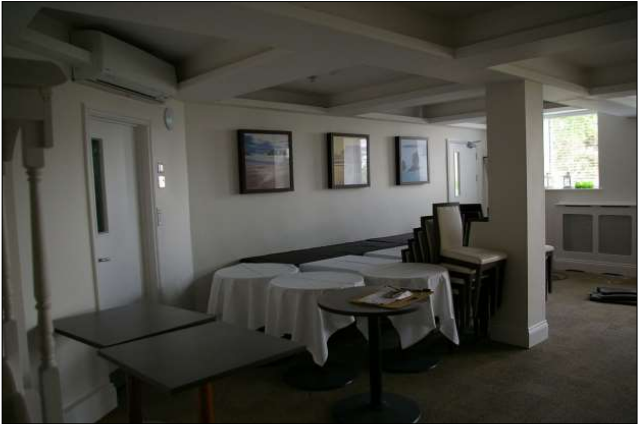
THE SOUTH BAY WINDOW AND MODERN PARTITION WALL OF THE BASEMENT, WHICH FORMS A CUPBOARD AGAINST THE WALL; FROM THE NORTH, NORTH-EAST.
