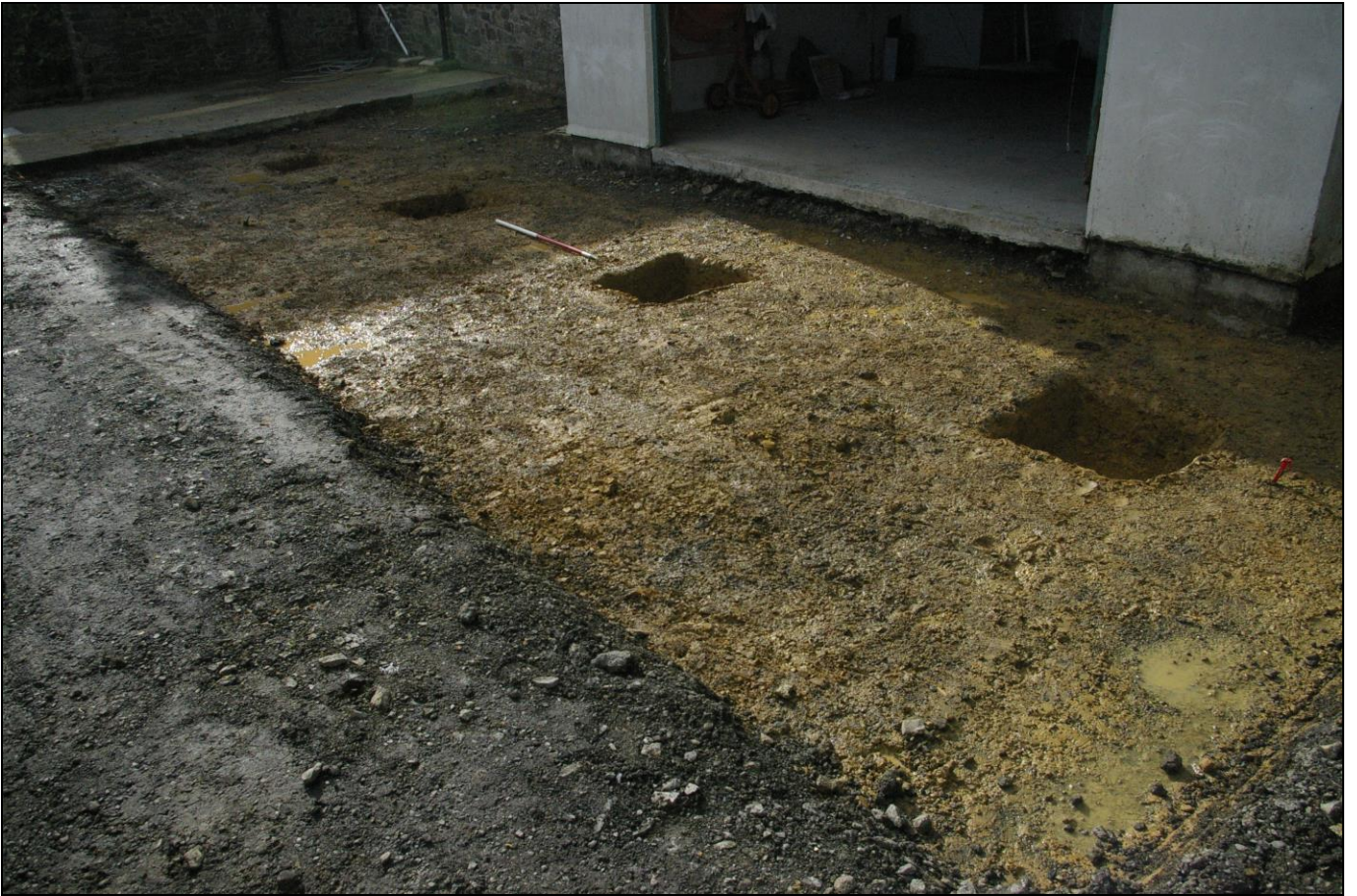
FIGURE 2: PITS 1-4 VIEWED FROM THE NORTH-EAST (1M SCALE).
