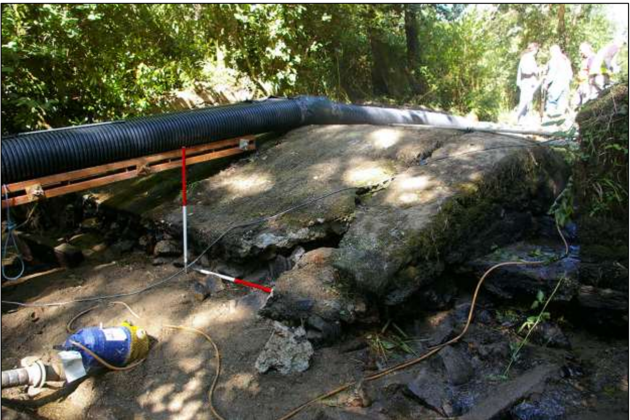
31. THE EXPOSED WEIR DURING DRAINAGE WORKS; FROM THE NORTH-EAST (1M SCALES).
