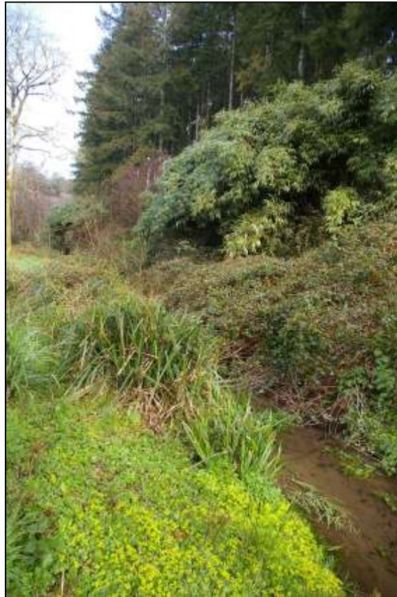
26. VIEW OF THE LEAT AT IT RUNS NORTH TOWARDS THE WEIR, WHERE IT BECOMES MORE SILTED UP AND OVERGROWN; FROM THE SOUTH, SOUTH-WEST.
