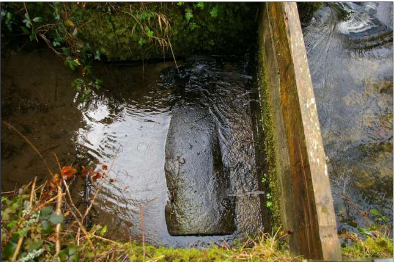
10. DETAIL OF A HEAVY CARVED STONE SLAB IN THE BASE OF THE LEAT, JUST PAST THE SLUICE GATE, EVIDENCE OF AN EARLIER SLUICE GATE OR SIMILAR? FROM THE NORTH.
