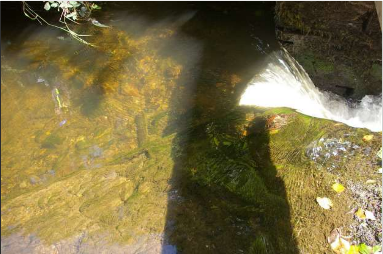
42. DETAIL OF THE SLATE SLAB EDGING TO THE CHANNEL ABOVE THE FISH PASS; FROM THE SOUTH-WEST.
