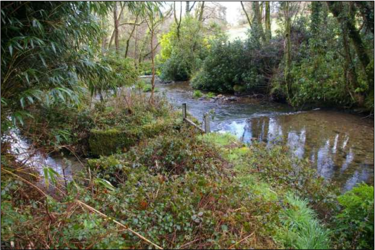
28. THE SLUICE WITH AND LEAT LOOKING SOUTH DOWN THE RIVER.
