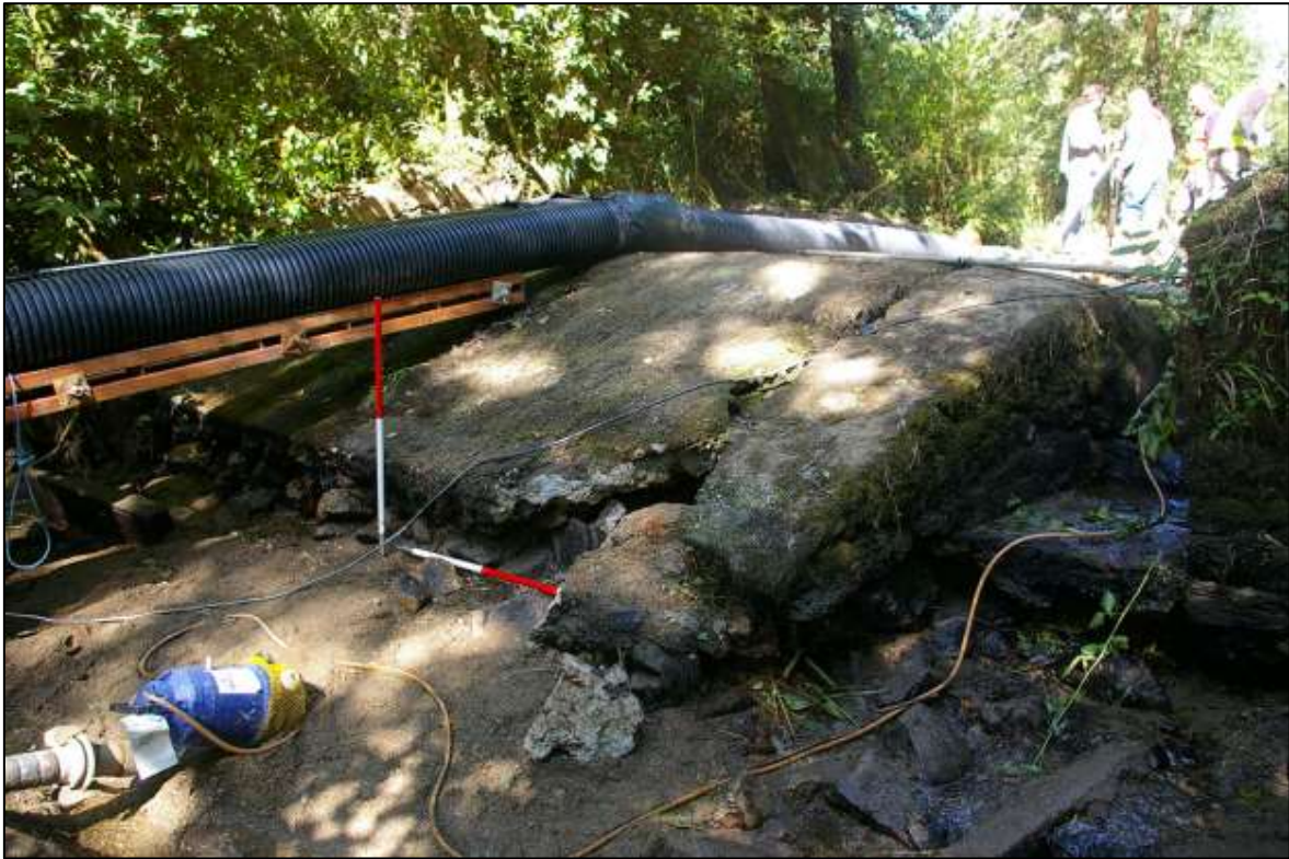
FIGURE 6: THE EXPOSED WEIR; FROM THE EAST-SOUTH-EAST (1M SCALES).
