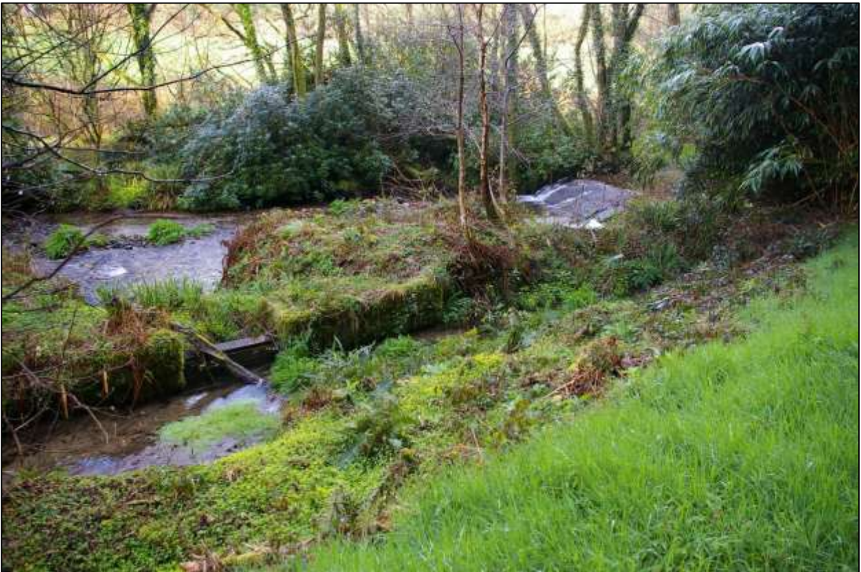
29. THE SLUICE, LEAT AND WEIR; FROM THE EAST.
