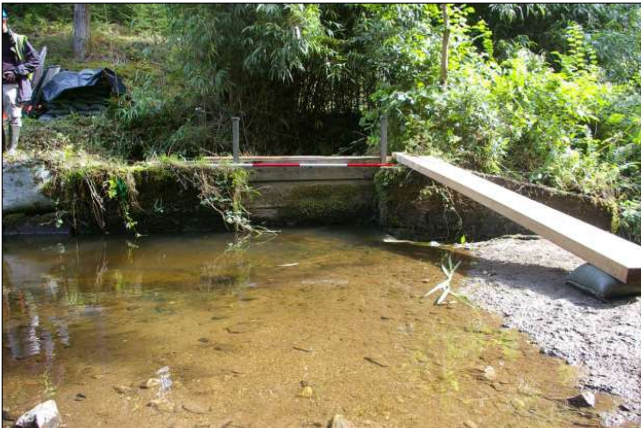
41. THE MODERNISED SLUICE GATE, WITH 2M SCALE; FROM THE WEST-SOUTH-WEST.
