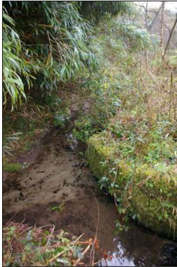
11. THE ANGLED CURVE WHICH CARRIES THE LEAT AWAY FROM THE RIVER AND THEN CORRECTS TO RUN SOUTH WITHIN THE VALLEY, SHOWING DEEP BUILT UP OF SANDY SILT IN THE BASE OF THE LEAT; FROM THE NORTH, NORTH-WEST.
