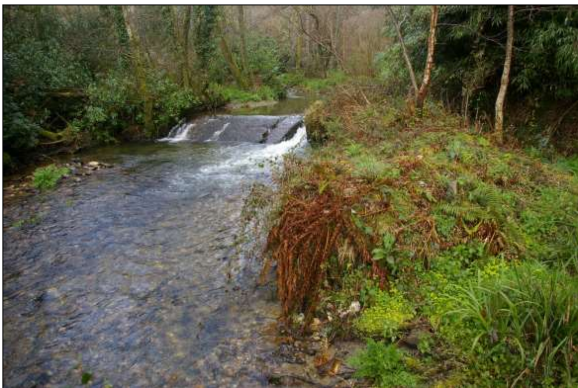
FIGURE 5: THE WEIR IN ITS SETTING, AS VIEWED FROM THE SOUTH-SOUTH-EAST (NO SCALES).
