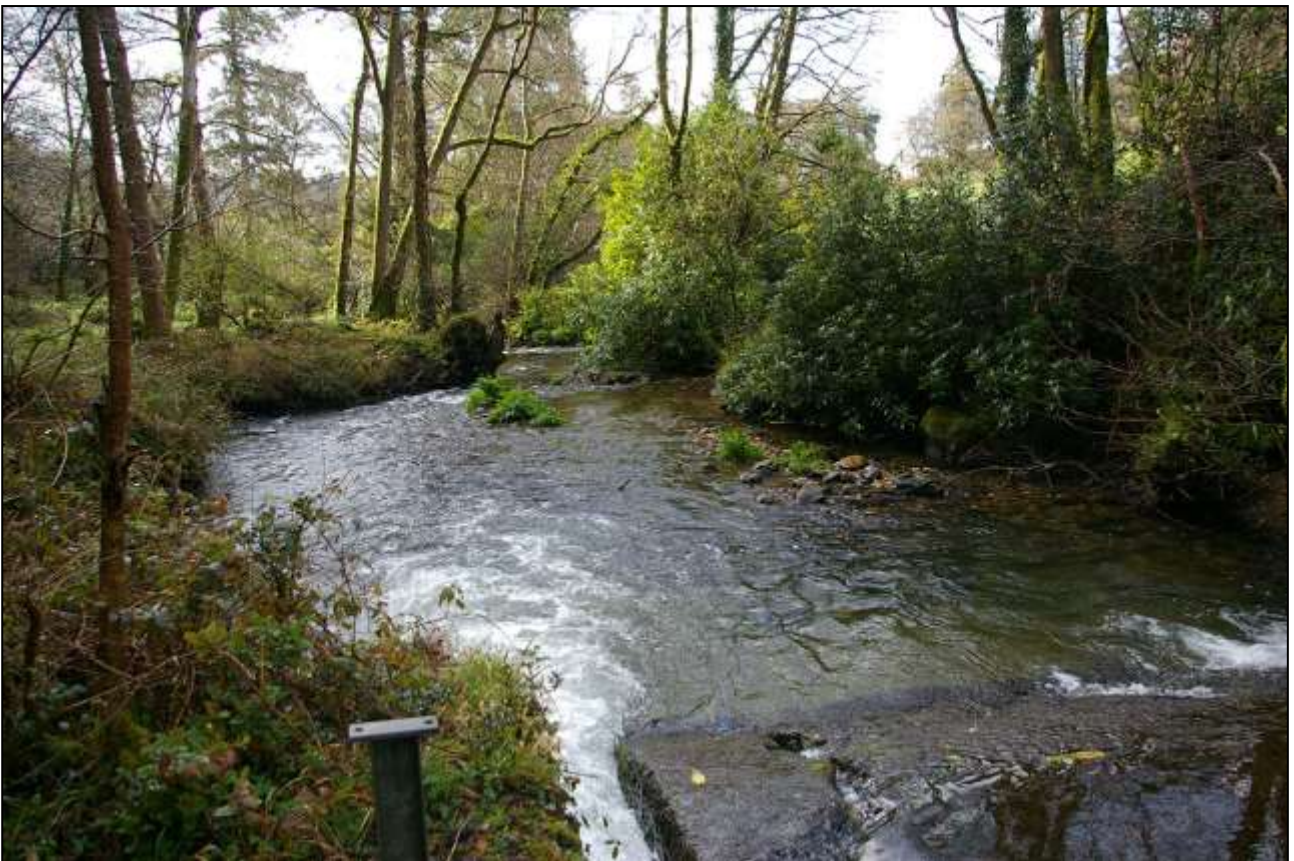
8. VIEW OF THE RIVER BELOW THE WEIR, SHOWING A WIDE ANGLED EXTENSION ON THE EAST BANK, FLANKED BY ABUTMENT WALLS, WHICH IS AN OVERFLOW FROM THE WORKING LEAT; FROM THE NORTH, NORTH-EAST.
