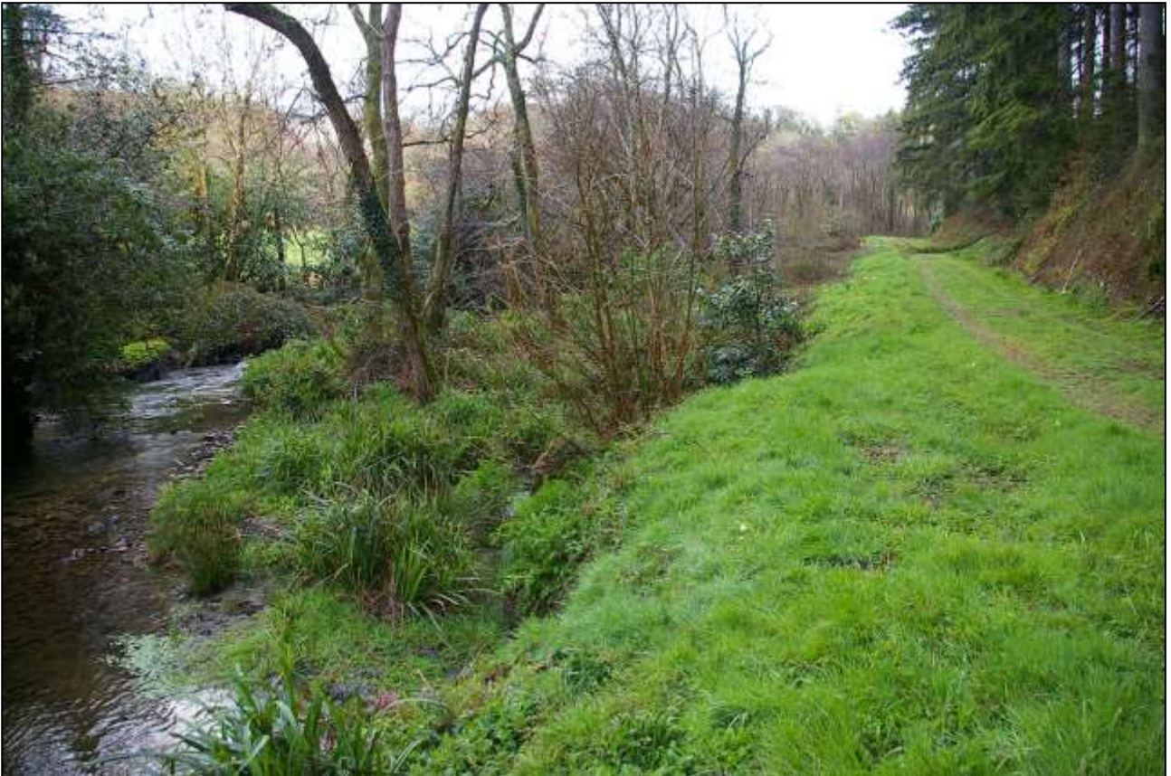
3. VIEW OF WHERE THE SILTED UP LEAT ADJOINS THE RIVER, JUST ABOVE THE WEIR; FROM THE SOUTH-EAST.
