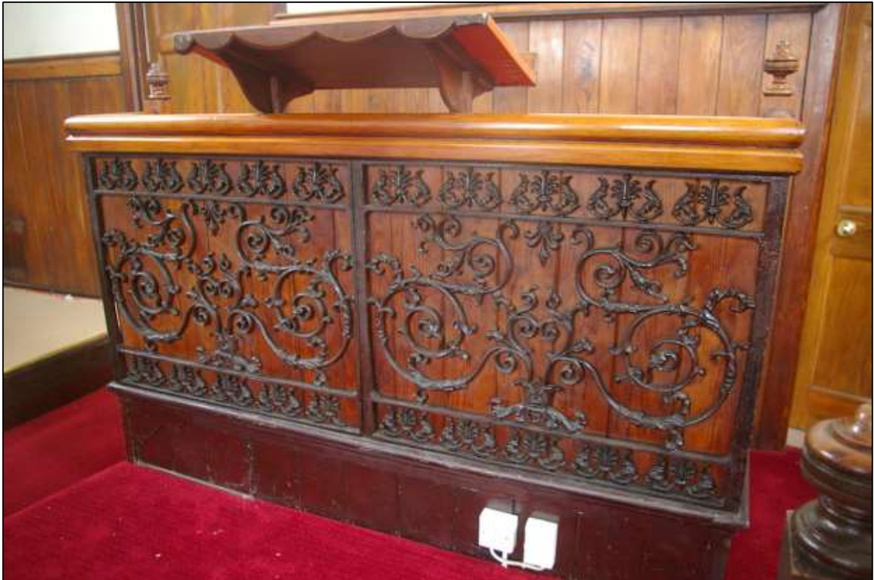
52. CAST IRON PULPIT FRAME, A LATER EDITION ENCLOSING THE PLAIN PLANK UPRIGHTS, LIKELY AN 1896 ADDITION; FROM THE SOUTH-EAST.
