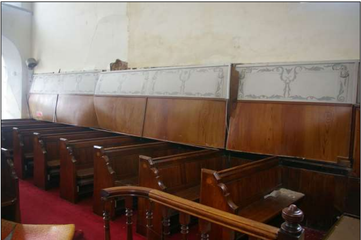
35. THE WOOD VENEER AND PAINTED MODERN PANELLING TREATMENT TO THE LOWER PART OF THE CHAPEL WALLS; FROM THE NORTH-EAST.
