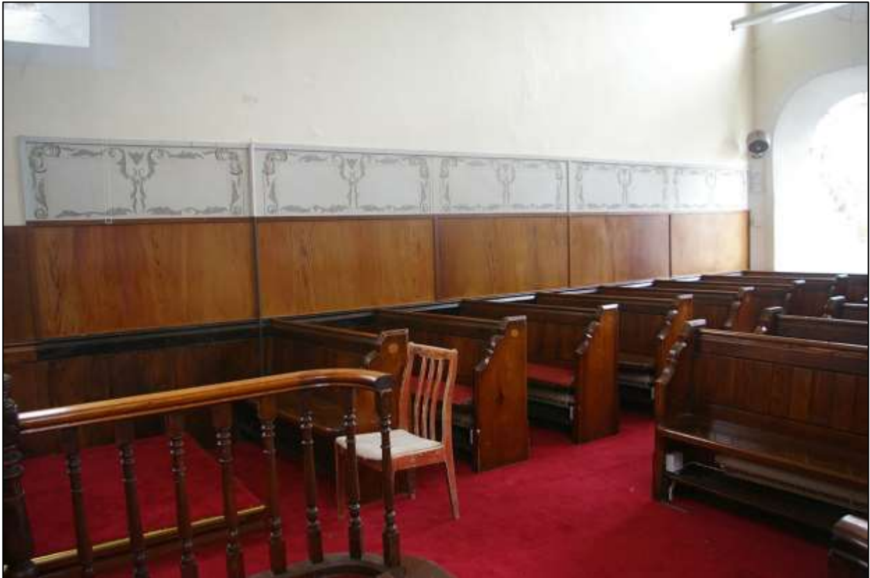
40. THE WOOD VENEER AND PAINTED MODERN PANELLING TREATMENT TO THE LOWER PART OF THE CHAPEL WALLS; FROM THE NORTH-WEST.
