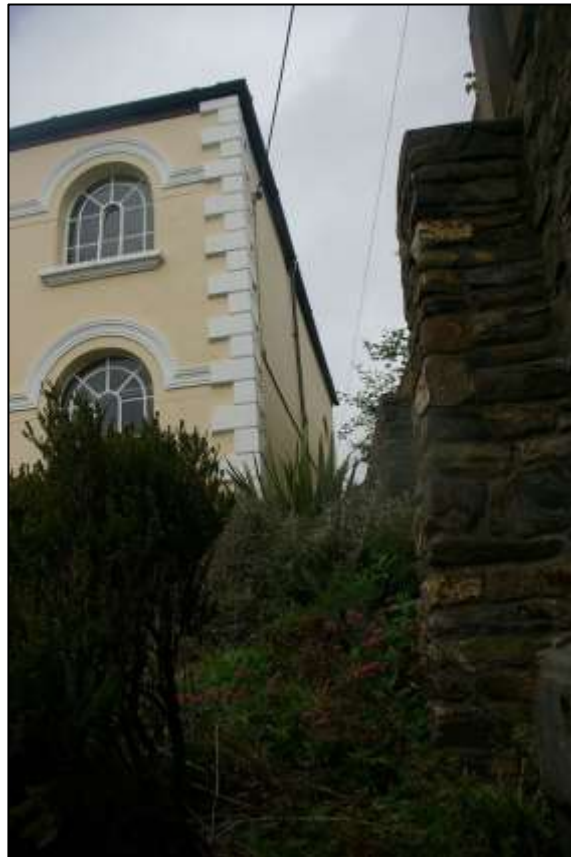
4. THE EAST ELEVATION OF THE CHAPEL BUILDING; FROM THE SOUTH.
