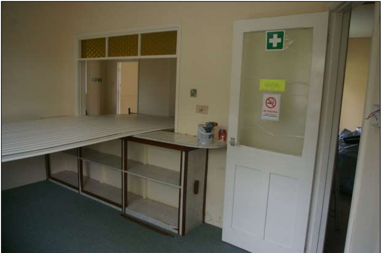
66. THE SERVING HATCH AND SHELVES; FROM THE SOUTH-WEST.
