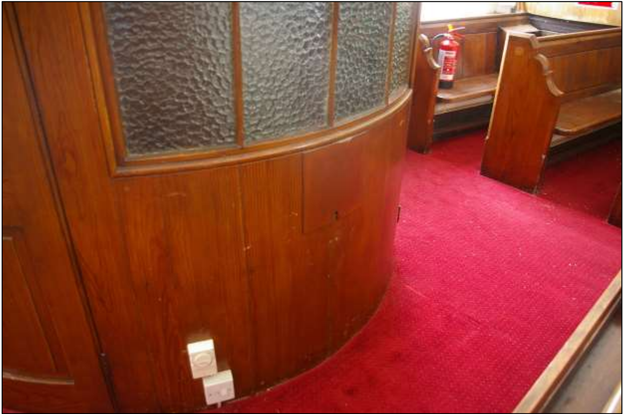
28. THE REAR SIDE OF THE COLLECTION BOX, NOW BOARDED OVER, A METAL BOX OR CASE OR SIMILAR LIKELY REMOVED; FROM THE NORTH-EAST.
