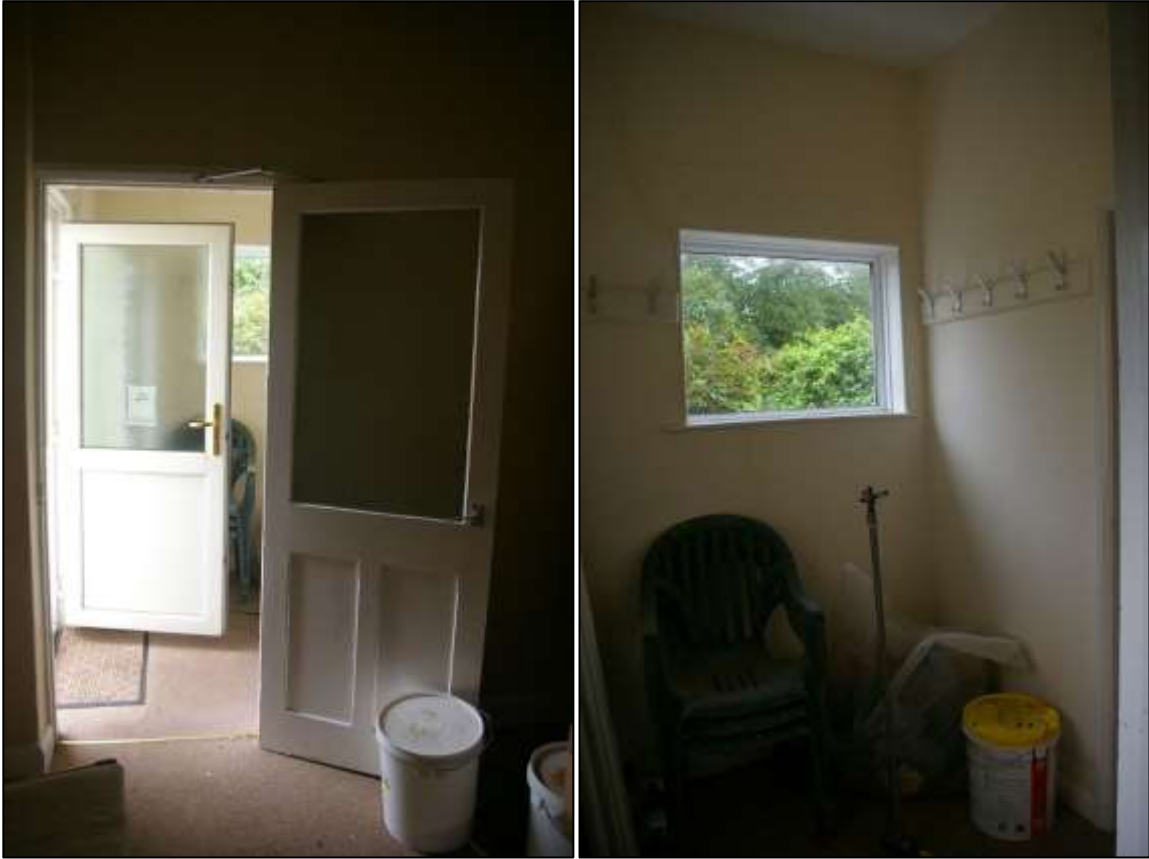
61. LEFT: THE DOOR TO THE REAR ENTRANCE, TO THE WEST YARD, D6 AND D8; FROM THE EAST. 62. RIGHT: THE REAR ENTRANCE TO THE COMMUNITY HALL; FROM THE EAST, SOUTH-EAST.
