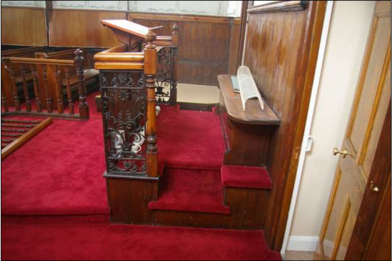
47. THE RAISED PLANK BOARDED PULPIT STEPPED STRUCTURE; FROM THE EAST.
