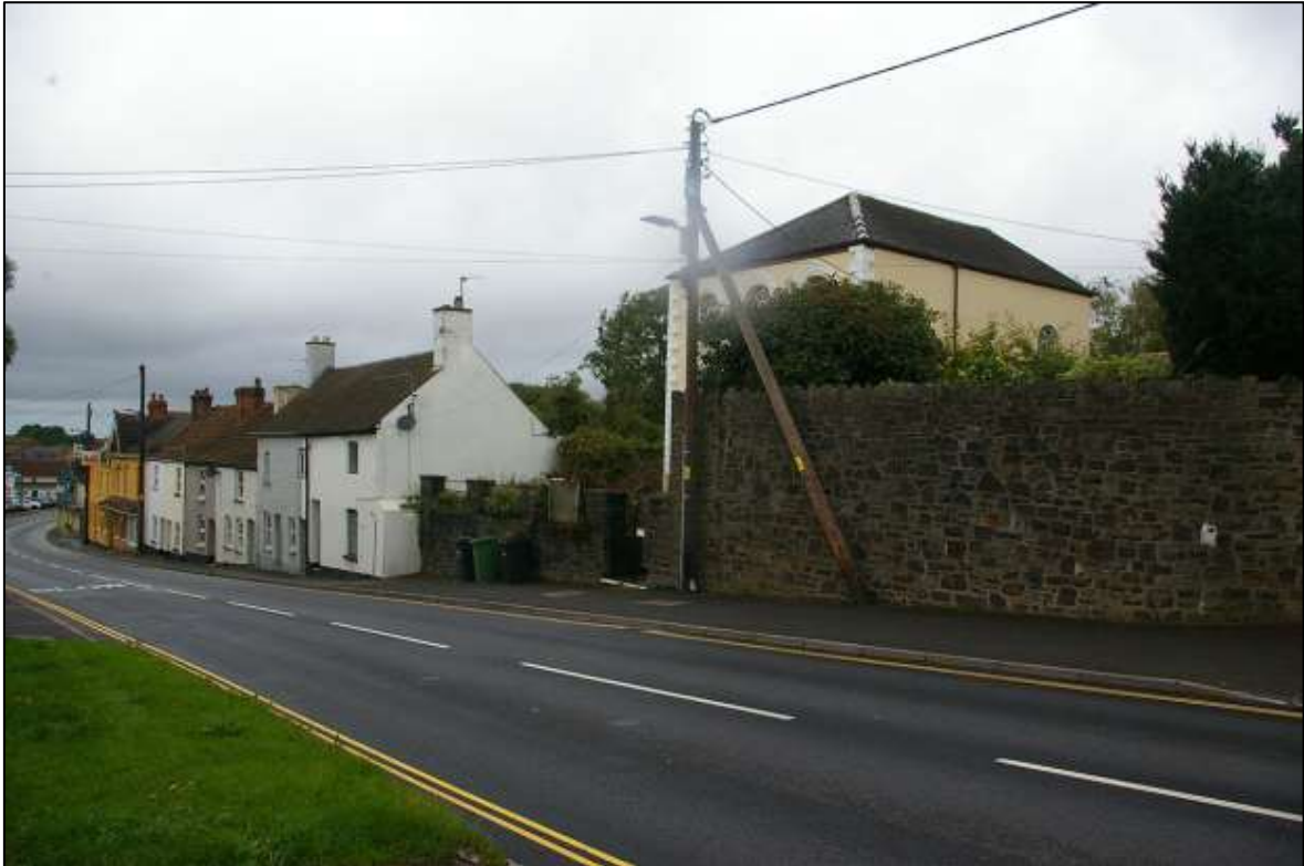
FIGURE 2: THE CHAPEL SETTING, ON BICKINGTON ROAD; FROM THE EAST, SOUTH-EAST.
