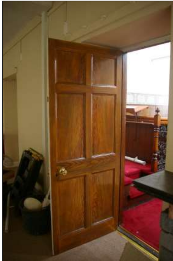
57. THE SIX PANEL D5, A REPLACEMENT DOOR; FROM THE NORTH-WEST.
