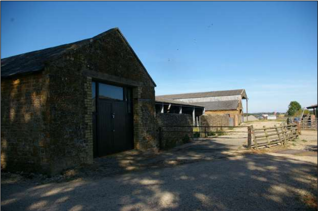
THE U-SHAPED RANGE WITH ENCLOSED COURTYARD TO FRONT, WITH LOW WALL; VIEWED FROM THE WEST-SOUTH-WEST.
