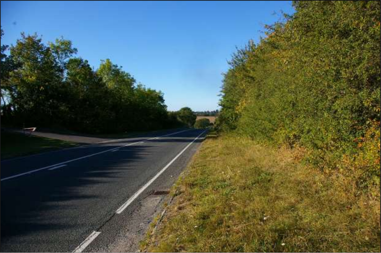
VIEW OF THE MODERN ROAD SET DOWN INTO A CUTTING WITH BANKING AND TREE PLANTING, TRUNCATING THE LANDSCAPE AND DIVIDING DANE HILL FARM FROM THE REST OF THE VALLEY; VIEWED FROM THE SOUTH-SOUTH-EAST.
