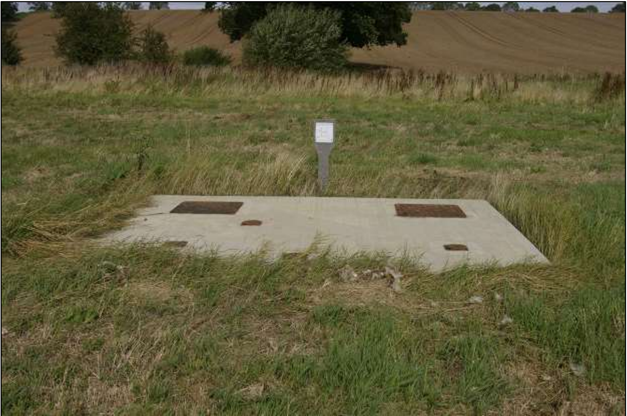
VIEW OF THE PUMPING MAIN INSPECTION HATCH; VIEWED FROM THE SOUTH.
