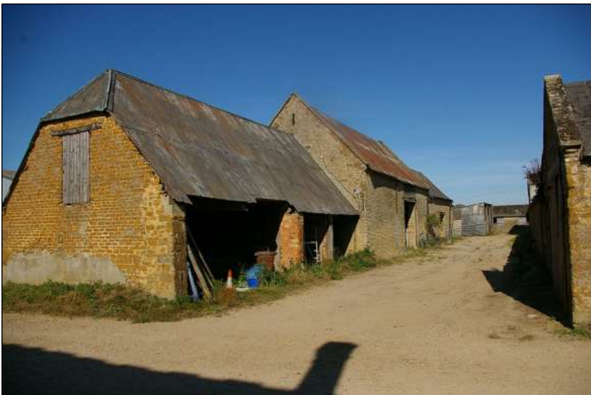
FIGURE 29: VIEW ALONG THE FRONT OF THE HISTORIC LINEAR RANGE AT HILL FARM, WITH BARN, MIDDLE THRESHING BARN AND IN THE FOREGROUND AN OPEN-FRONTED CART SHED/LINHAY; VIEWED FROM THE WEST-SOUTH-WEST.
