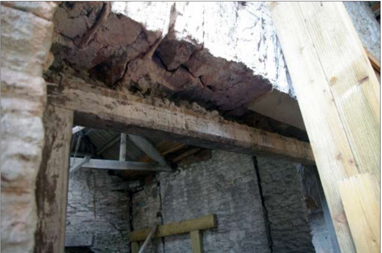
72. B1 FF R1, DETAIL OF THE CHAMFERED DOORFRAME TO D19; VIEWED FROM THE SOUTH-WEST.
