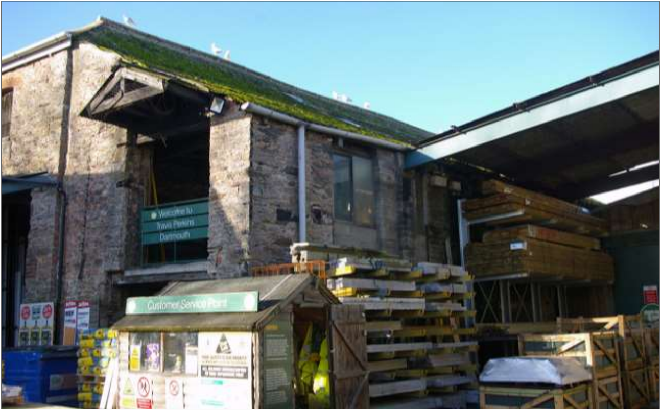
138. THE SOUTH AND EAST ELEVATIONS OF B3; VIEWED FROM THE SOUTH-EAST.
