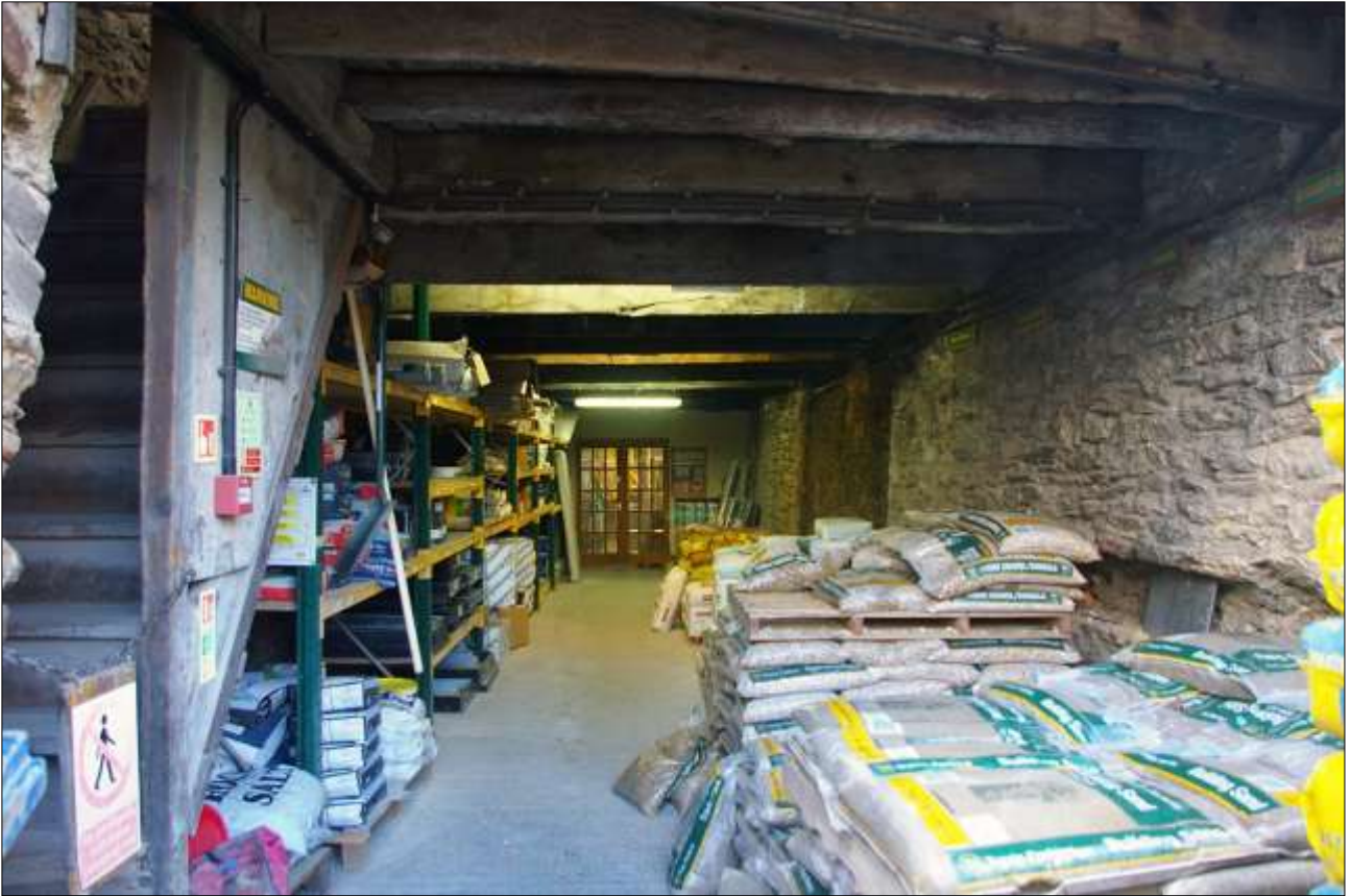
147. THE GF INTERIOR OF B3; VIEWED FROM THE SOUTH.
