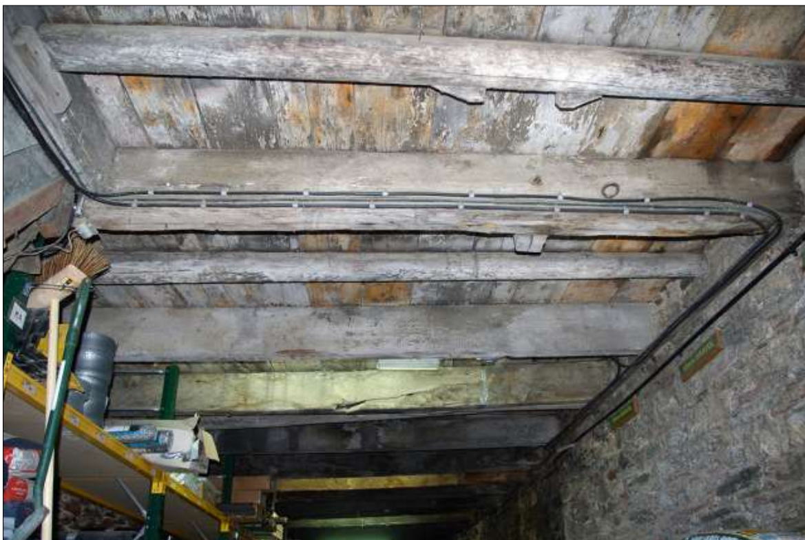
FIGURE 30: SOME OF THE JOISTS IN B3, SHOWING THE REUSE OF SHIPS TIMBERS; VIEWED FROM THE SOUTH.
