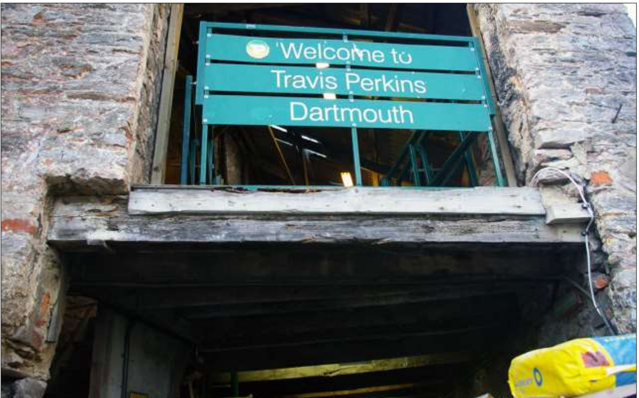
142. THE SOUTH ELEVATION OF B3, SHOWING THE LINTEL OVER D13; VIEWED FROM THE SOUTH.
