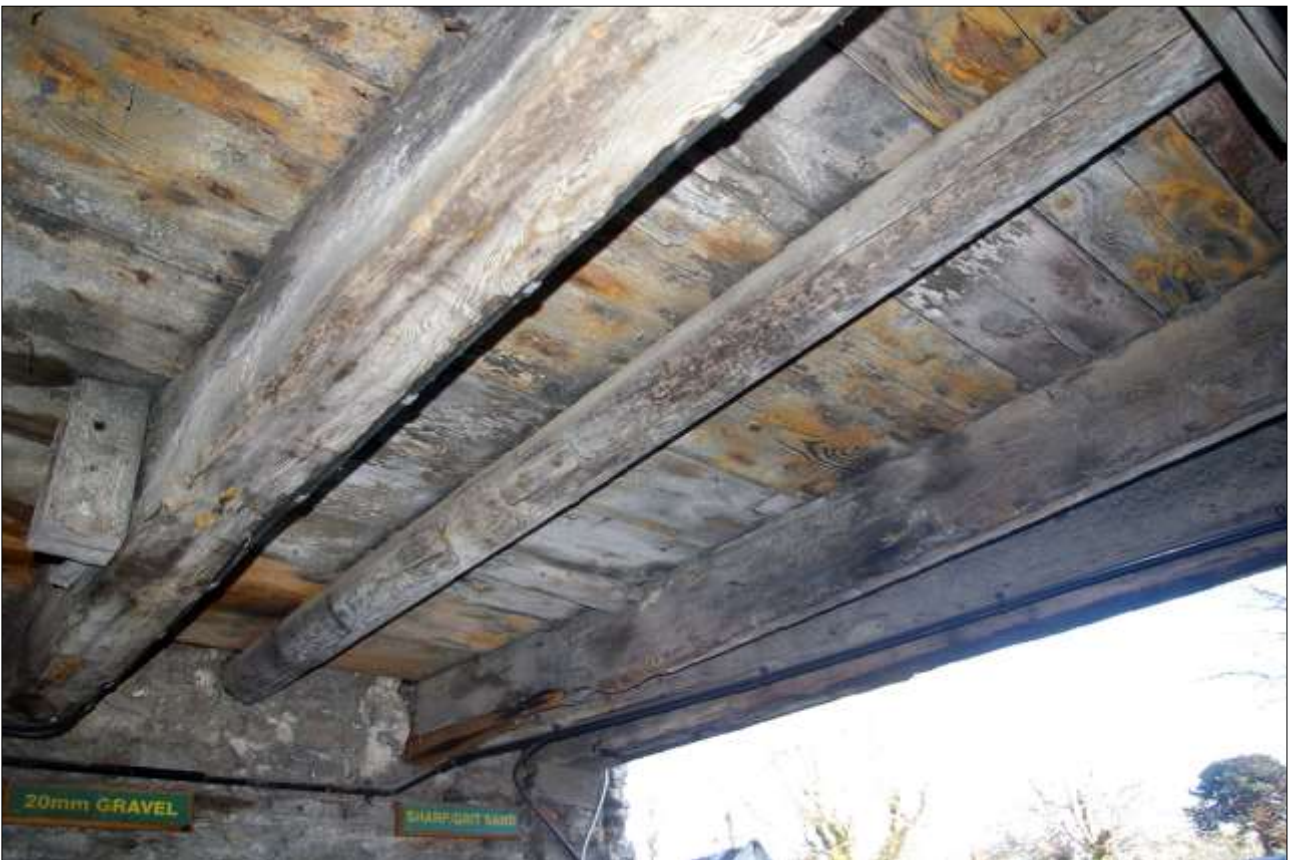
156. AS ABOVE, AT THE ENTRANCE (D13); VIEWED FROM THE WNW.
