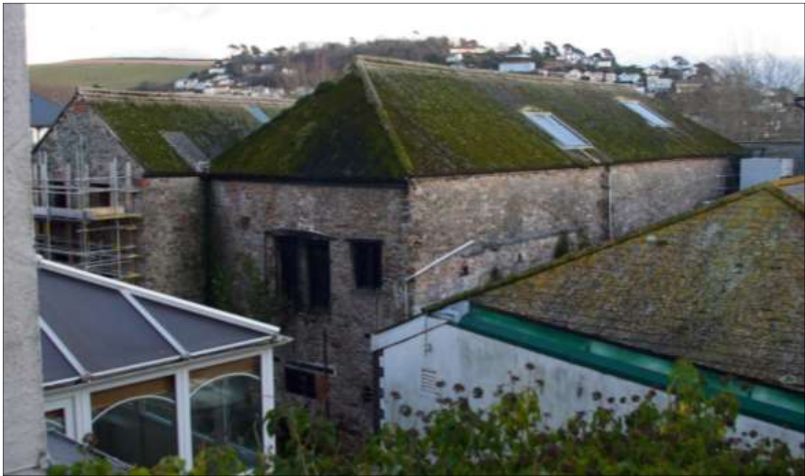
FIGURE 19: THE NORTH AND WEST WALLS OF B1, VIEWED FROM THE NORTH-WEST.
