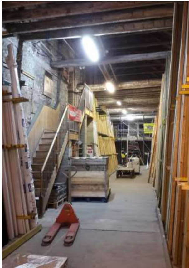
97. THE STRIPPED-OUT INTERIOR OF B2; VIEWED FROM THE SOUTH.
