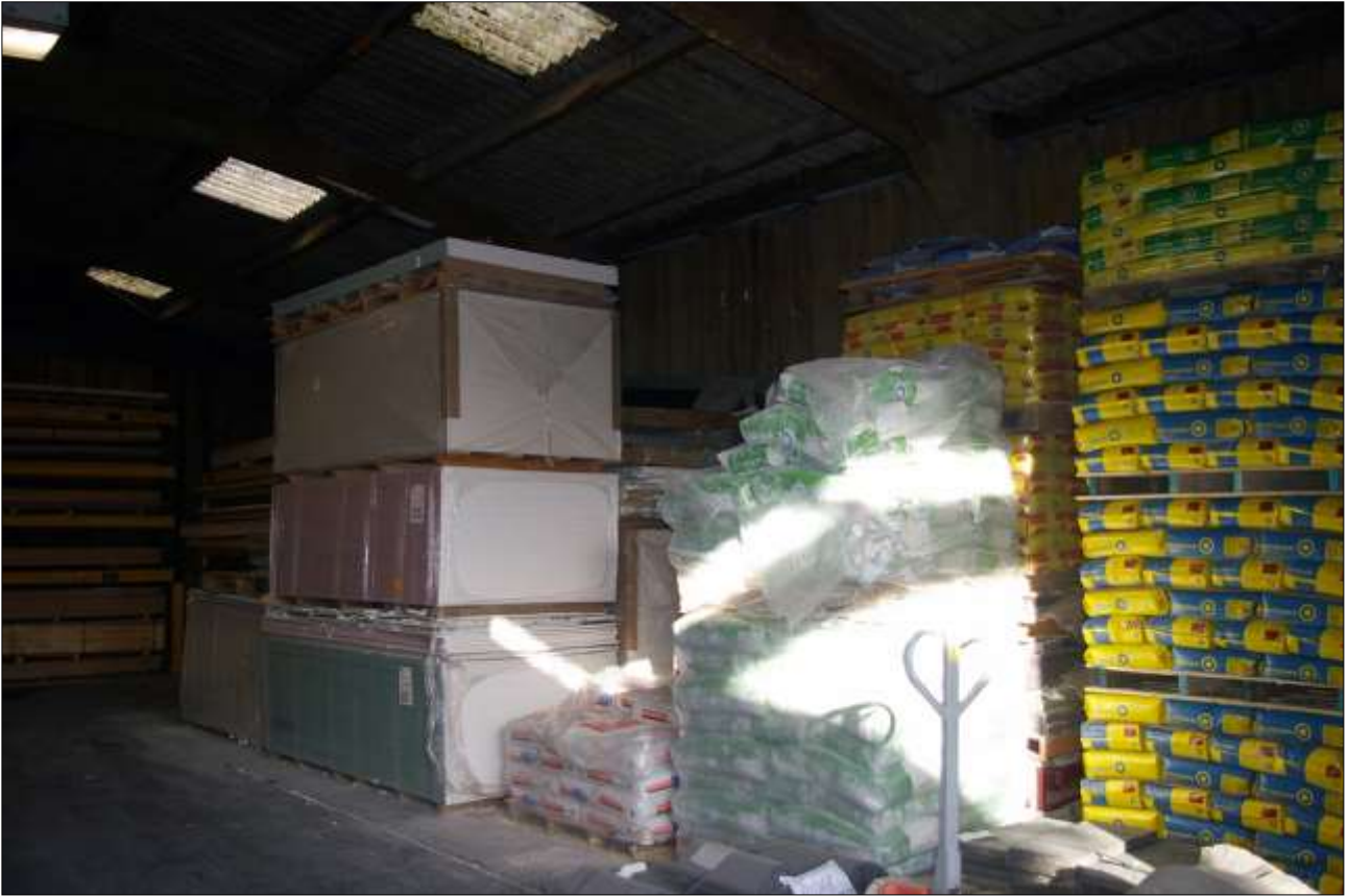
196. AS ABOVE, THE CONCEALED EAST WALL OF B4 (WALL OF THE ADJOINING PROPERTY); VIEWED FROM THE SOUTH-WEST.
