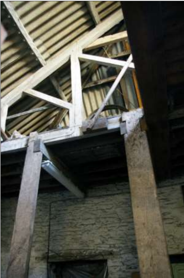
B1 FF R1, DETAIL OF THE YOKED LINTEL OVER W9; VIEWED FROM THE NORTH.
