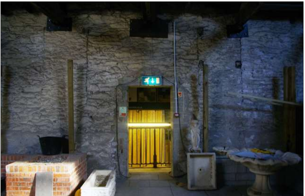
44. B1 FF ROOM 1 (R1), SHOWING FORCED DOORWAY D18 IN BO37; VIEWED FROM THE WEST.
