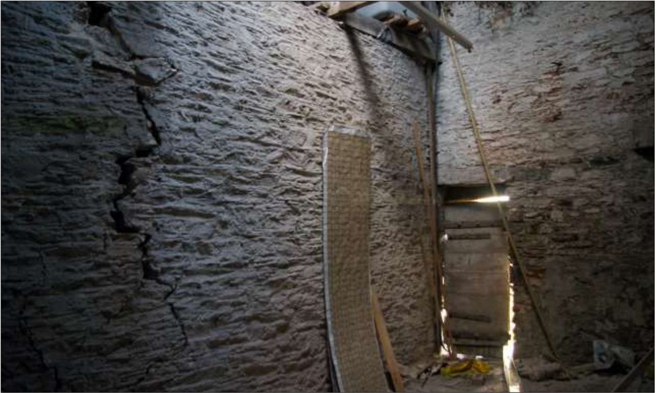
74. B1 FF R2, VIEW OF THE STRUCTURAL CRACK IN THE WEST WALL, AND D22 IN THE NORTH WALL; VIEWED FROM THE SSE.
