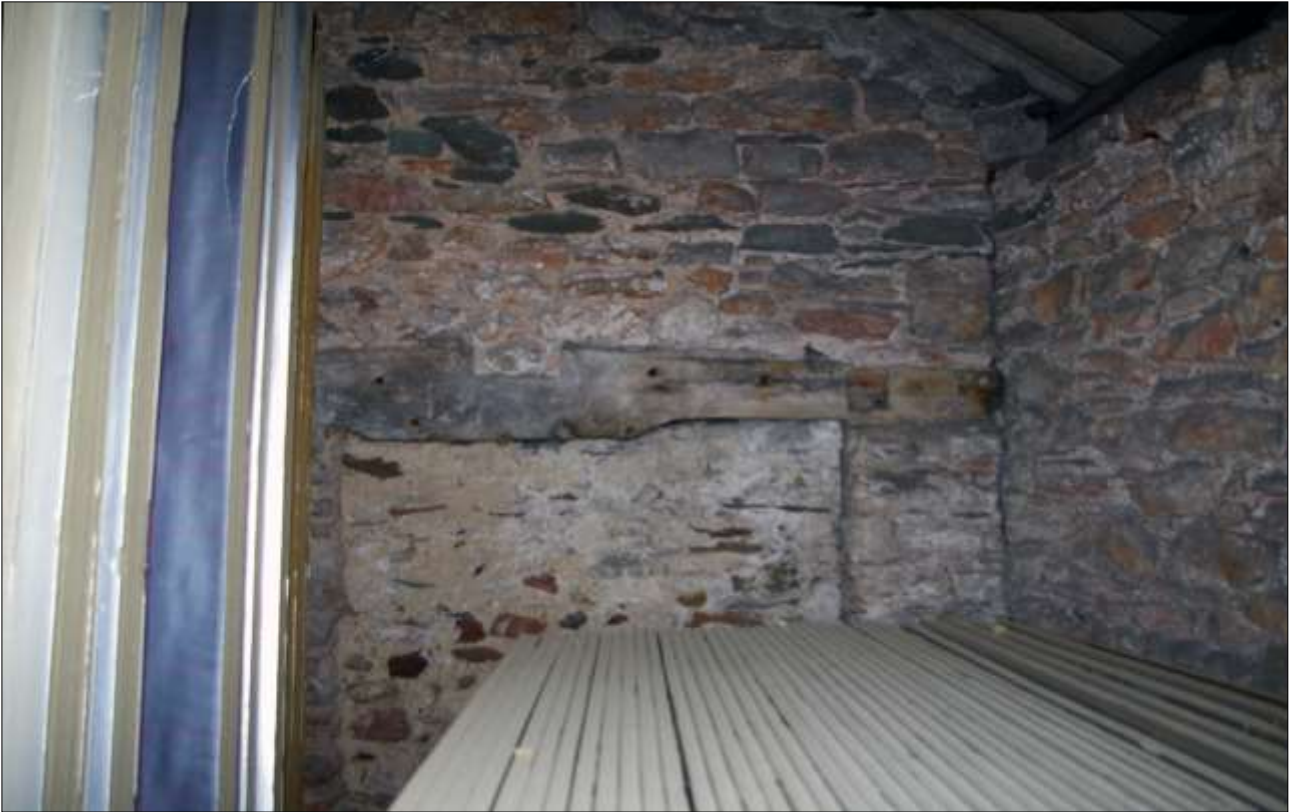
189. B3 FF INTERIOR, THE NORTH WALL SHOWING BO46 WITH UPSIDE-DOWN YOKED LINTEL; VIEWED FROM THE SOUTH.
