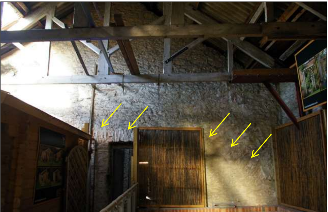
68. B1 FF R1, THE NORTH WALL SHOWING D19 BELOW THE WIDE RELIEVING ARCH (INDICATED); VIEWED FROM THE SOUTH.
