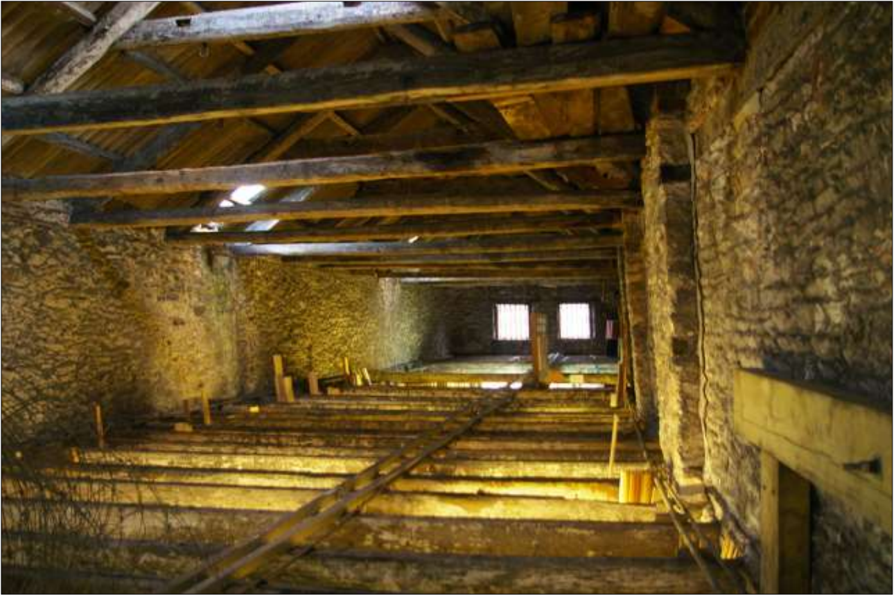
119. AS ABOVE; VIEWED FROM THE NNW.
