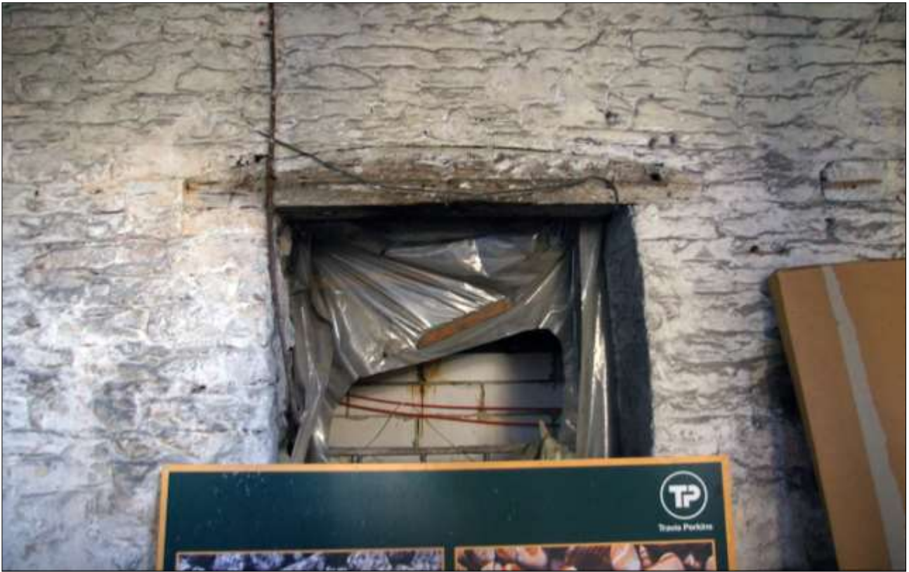
B1 FF R1, DETAIL OF THE YOKED LINTEL OVER W9; VIEWED FROM THE NORTH.
