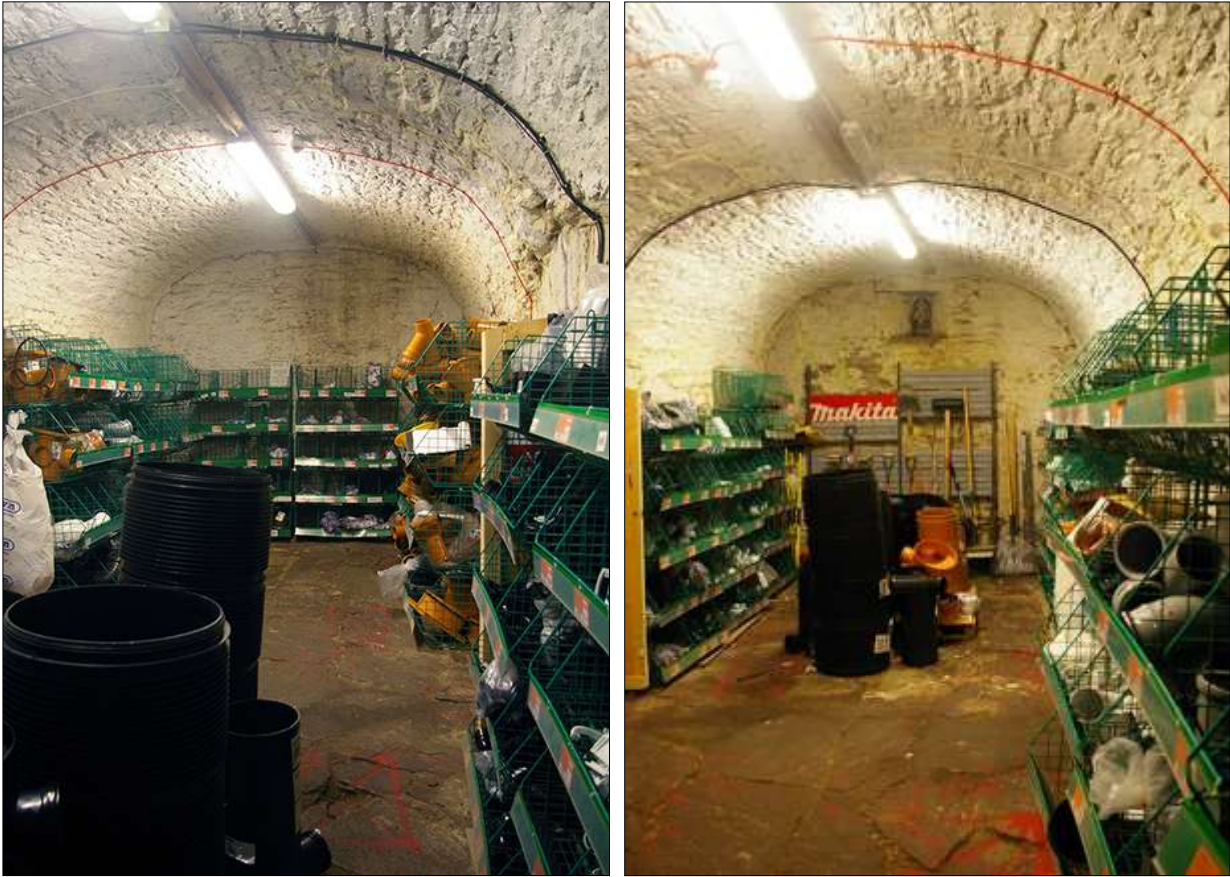
28. LEFT: B1 GF V2; VIEWED FROM THE WEST.
