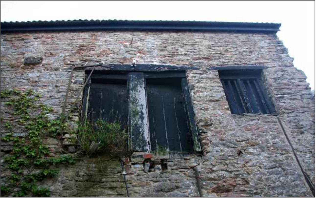
4. THE NORTH ELEVATION OF B1, SHOWING W11 AND FF DOOR 21 (D21) AND DOOR 22 (D22); VIEWED FROM THE NORTH.
