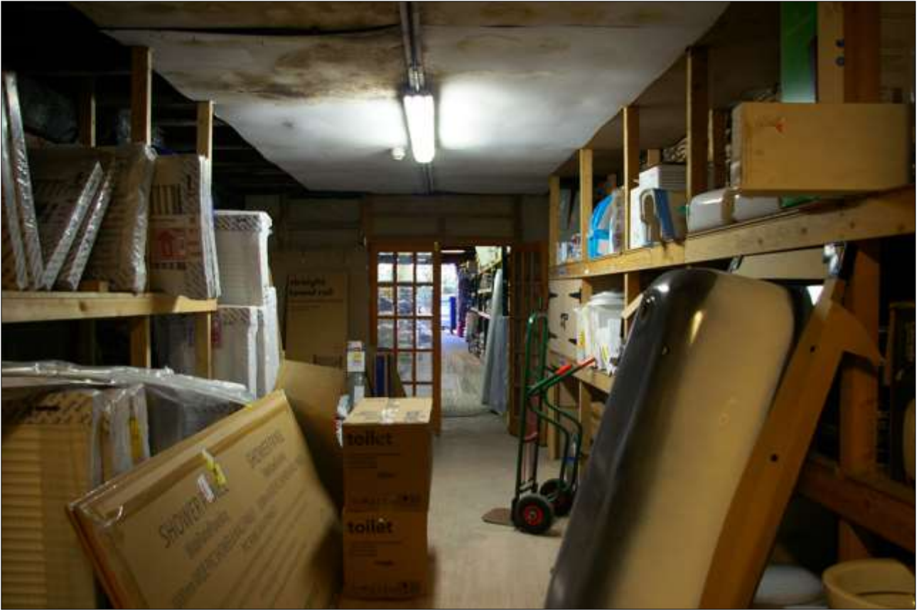
161. B3 GF INTERIOR, THE NORTHERN END; VIEWED FROM THE NORTH.
