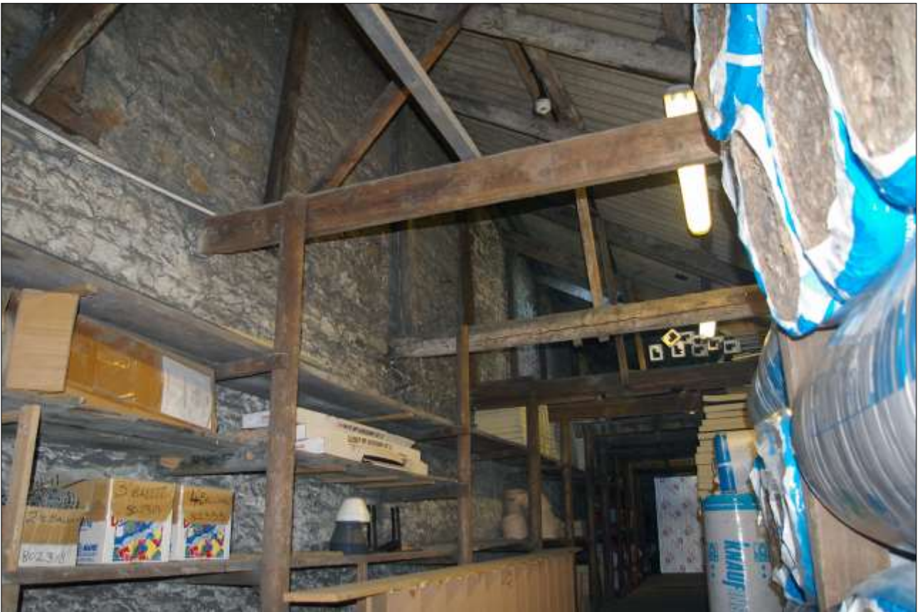
182. B3 FF INTERIOR, SHOWING THE ROOF STRUCTURE; VIEWED FROM THE SSE.
