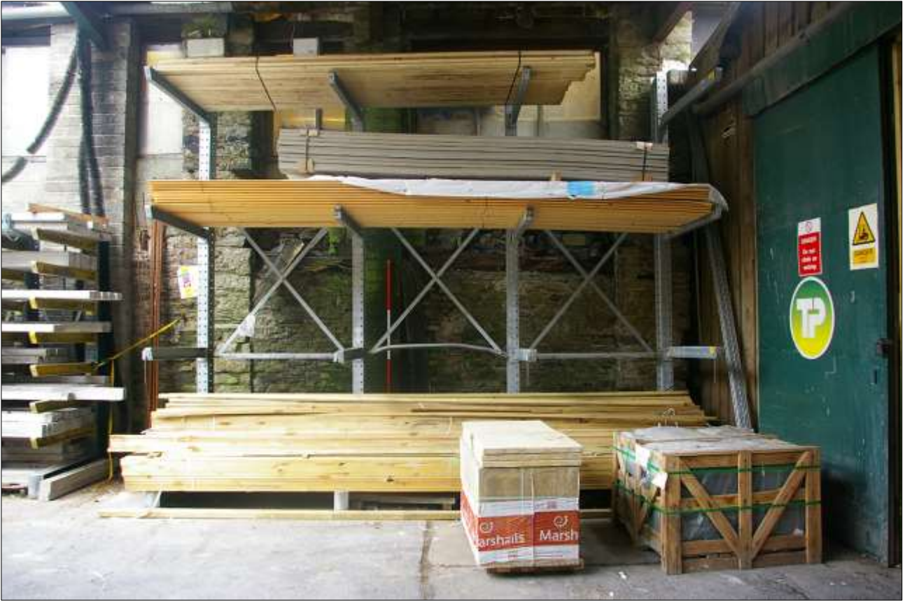
143. THE EAST ELEVATION OF B3 TO THE SOUTH OF B4; VIEWED FROM THE EAST (SCALE 2M).
