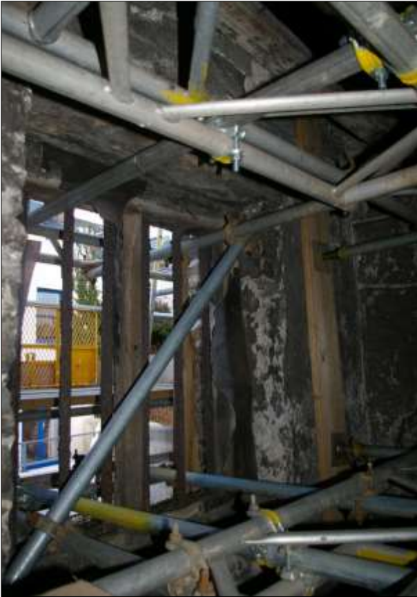
130. B2 SF INTERIOR, NORTH WALL, SHOWING W21; VIEWED FROM THE SOUTH-WEST.
