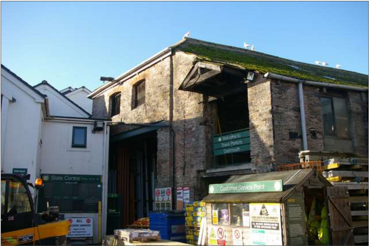
93. THE SOUTH ELEVATION OF B2 AND B3; VIEWED FROM THE SOUTH-EAST.
