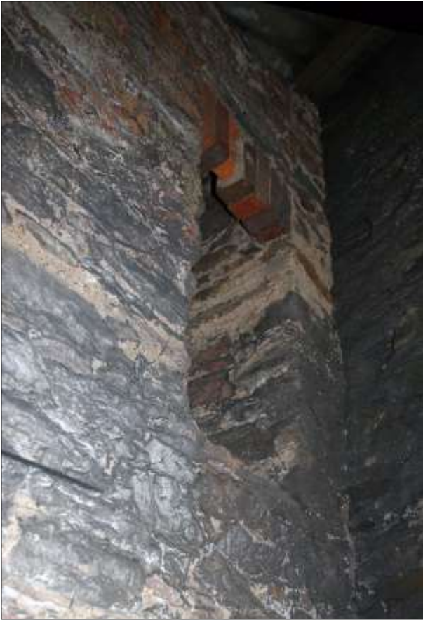
174. B3 SF INTERIOR, DETAIL OF FP4 ABOVE THE STAIRS; VIEWED FROM THE NORTH-EAST.
