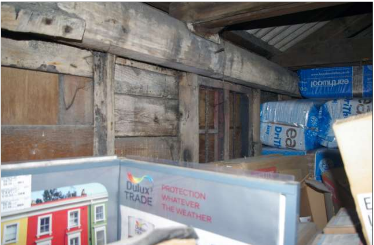
188. AS ABOVE; VIEWED FROM THE NORTH-WEST.
