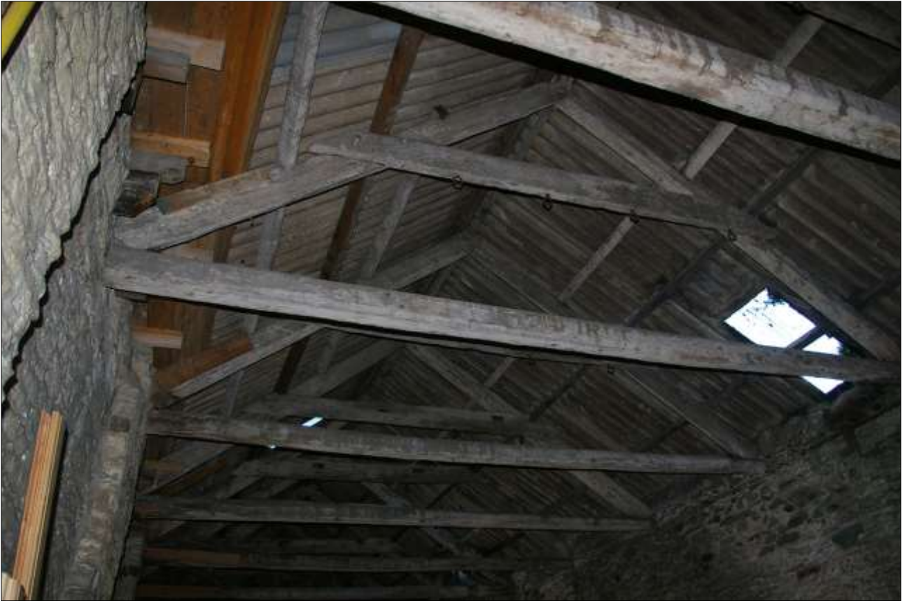
132. AS ABOVE, THE NORTHERN HALF OF THE ROOF; VIEWED FROM THE SOUTH.
