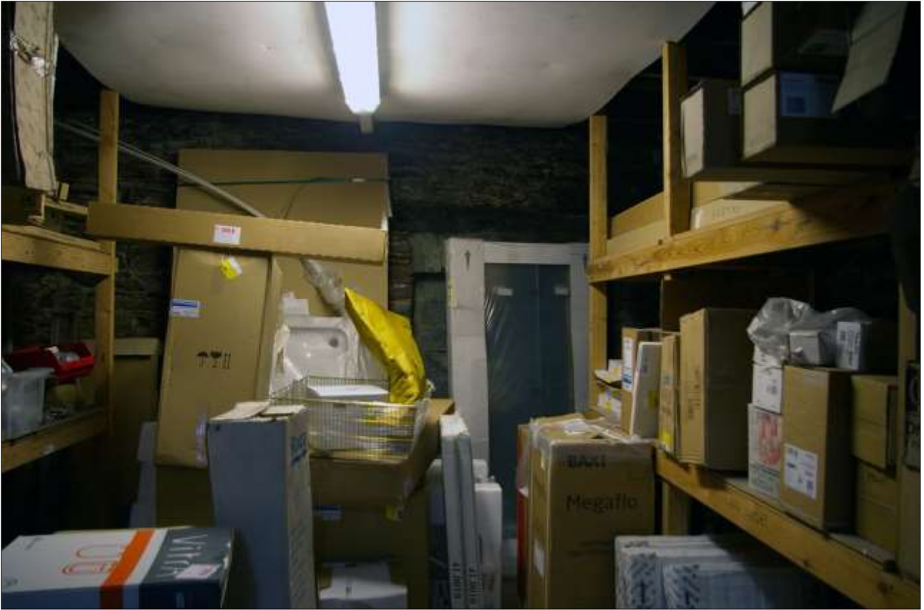
165. B3 GF INTERIOR, THE NORTH WALL WITH BO34; VIEWED FROM THE SOUTH.
