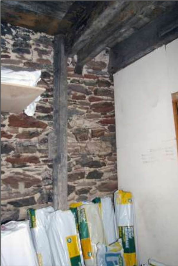
153. AS ABOVE, NEXT TO THE MODERN PARTITION; VIEWED FROM THE EAST.
