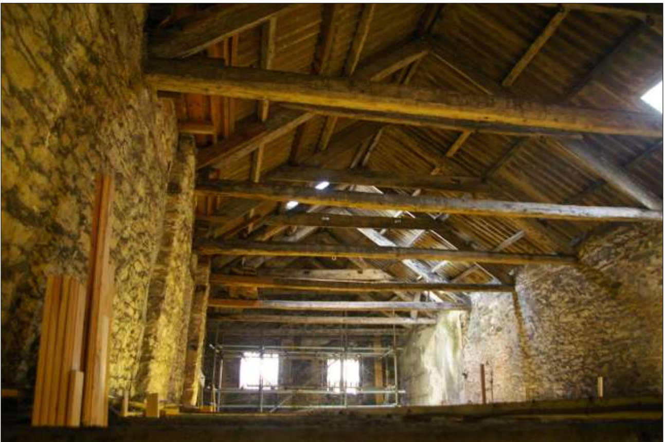
122. B2 SF INTERIOR; THE ROOF STRUCTURE OVER THE NORTHERN END OF B2, W20 AND W21; VIEWED FROM THE SSW.
