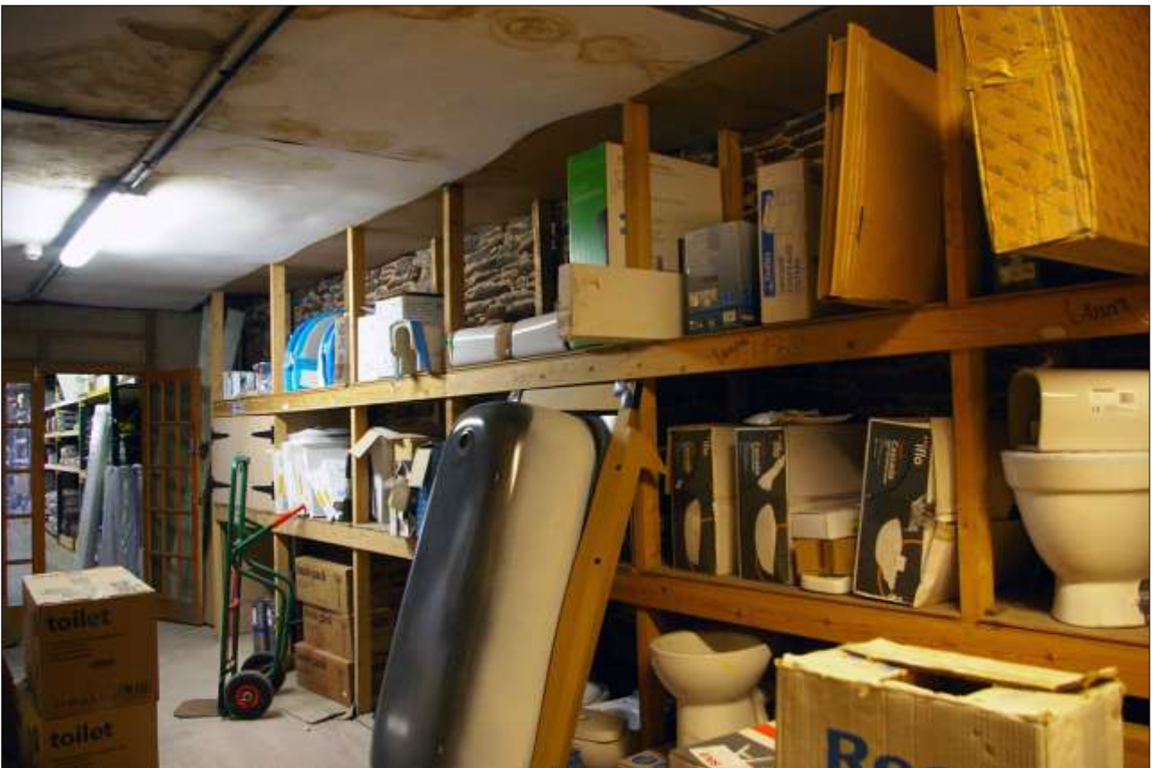
164. B3 GF INTERIOR, THE NORTHERN END, SHOWING THE EAST WALL OF B2; VIEWED FROM THE ENE.
