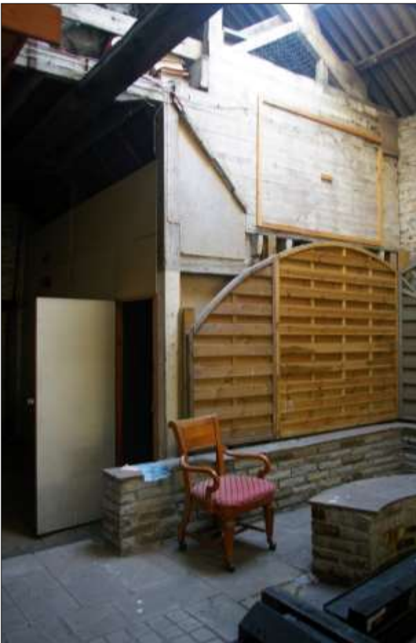
53. LEFT: AS ABOVE; VIEWED FROM THE NORTH-EAST.
