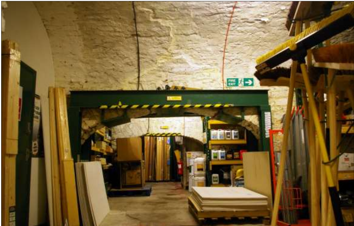
FIGURE 20: THE VAULTS ON THE GROUND-FLOOR LEVEL OF B1, LOOKING THROUGH ARCHWAY D4 TO D7, IN VAULTS V3-V5; VIEWED FROM THE SOUTH.
