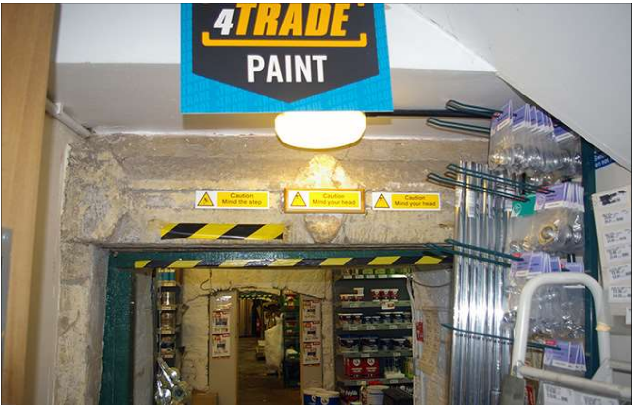
19. AS ABOVE, DETAIL OF THE RE-USED DRESSED STONE LINTEL; VIEWED FROM THE SOUTH.
