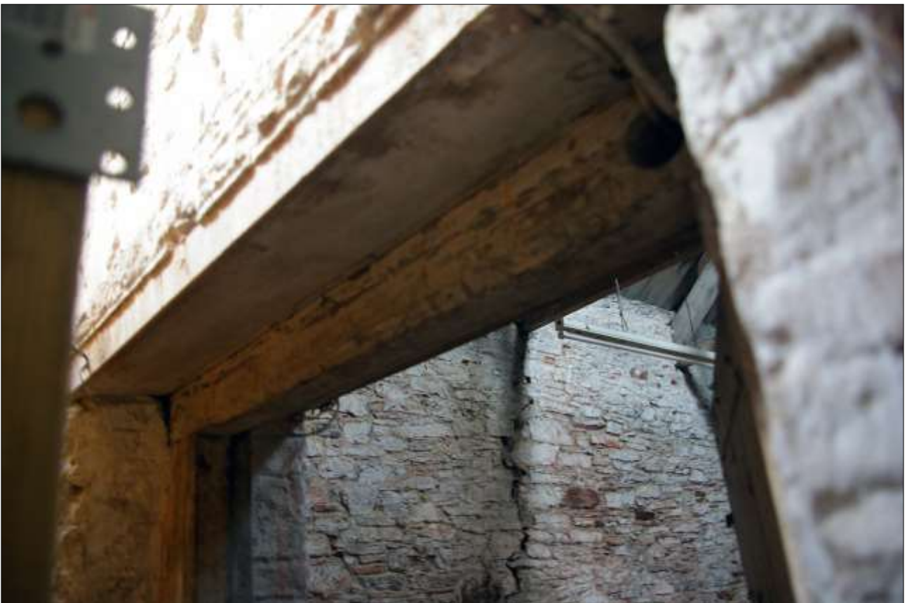
73. B1 FF R1, DETAIL OF THE DOORFRAME TO D20; VIEWED FROM THE SOUTH-EAST.
