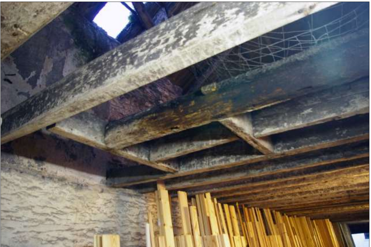
116. AS ABOVE, AS VIEWED FROM THE NORTH-WEST AND SHOWING HATCH OPENING (S21).
