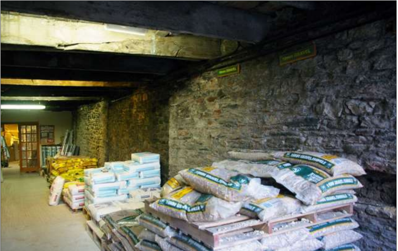
149. B3 GF INTERIOR, THE EAST WALL; VIEWED FROM THE SSW.
