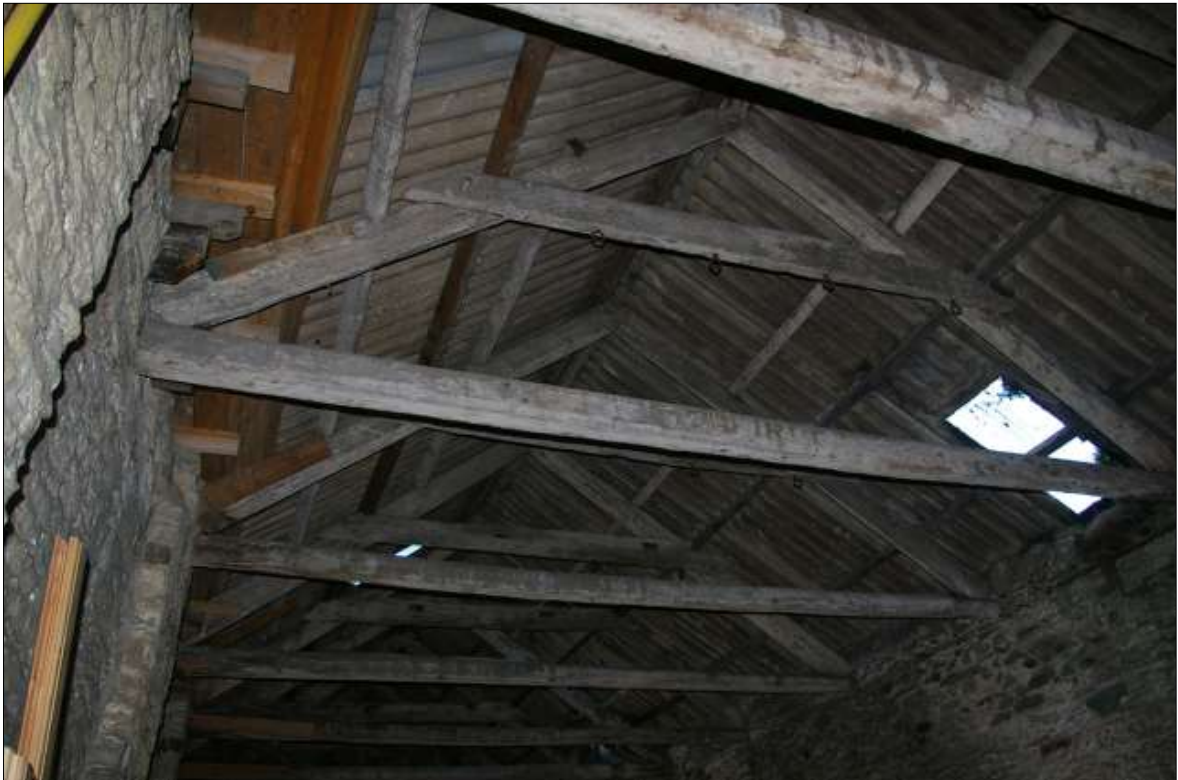
FIGURE 28: THE ROOF STRUCTURE IN B2; VIEWED FROM THE SOUTH.
