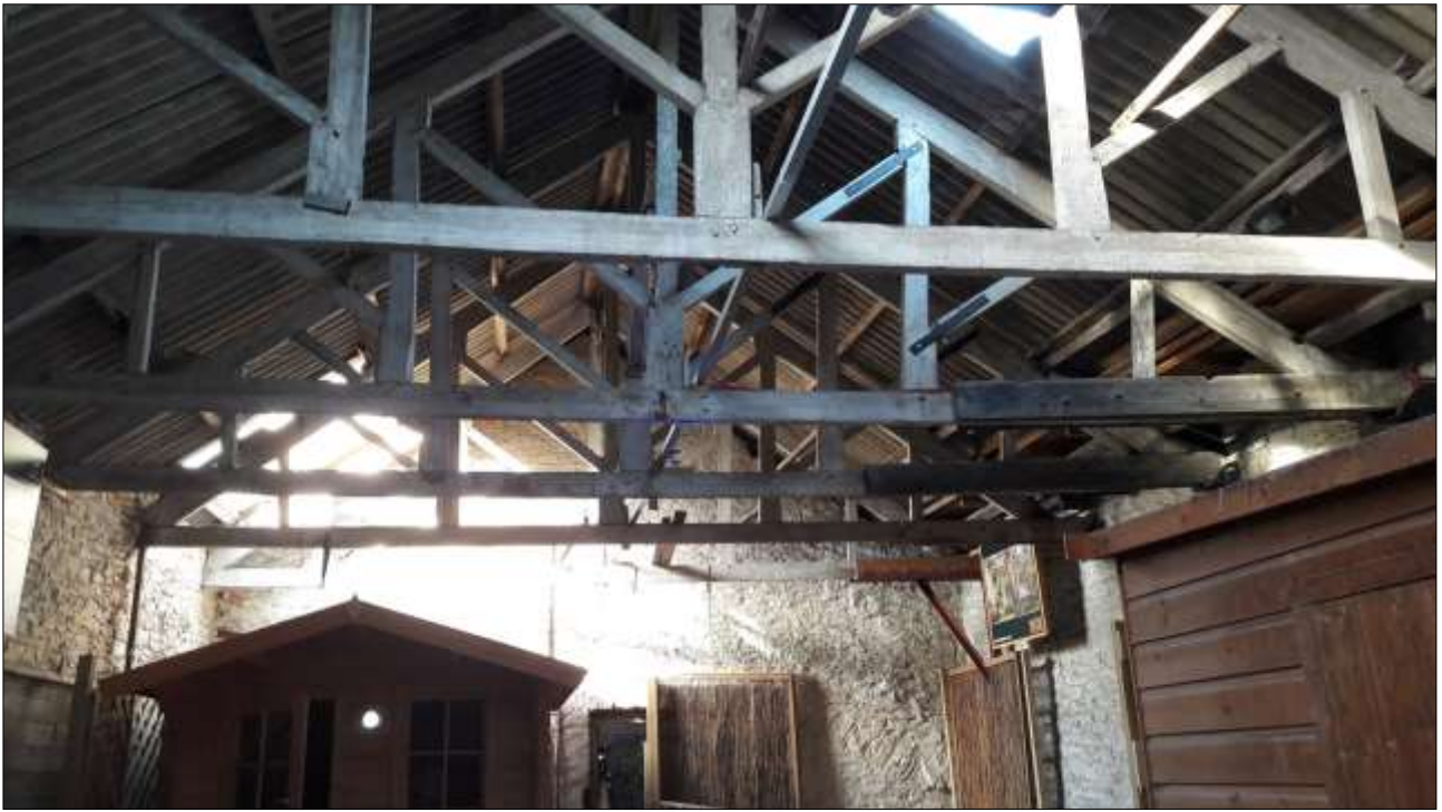
65. B1 FF, DETAIL OF THE ROOF STRUCTURE; VIEWED FROM THE SOUTH.
