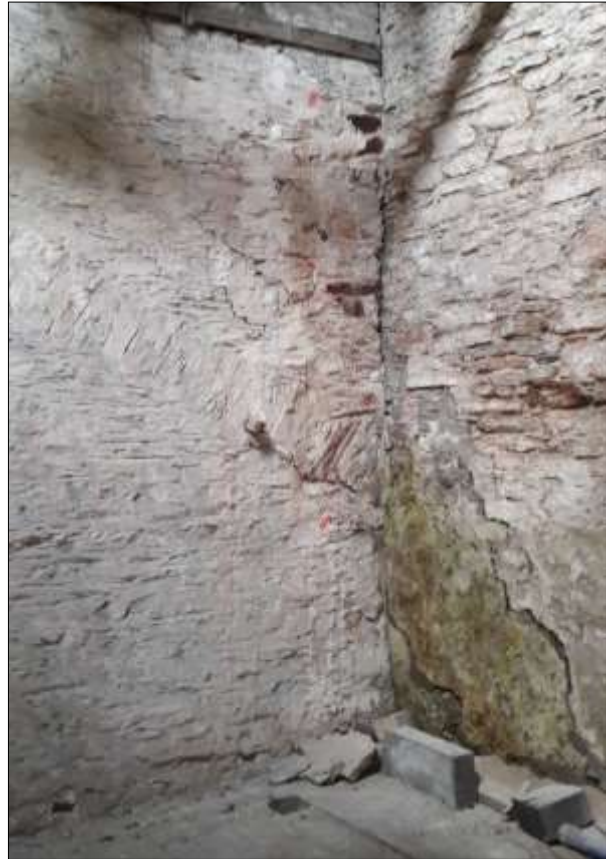
81. RIGHT: B1 FF R3, VIEW OF THE PARTY WALL WITH R1 SHOWING THE RELIEVING ARCH; VIEWED FROM THE NNE.
