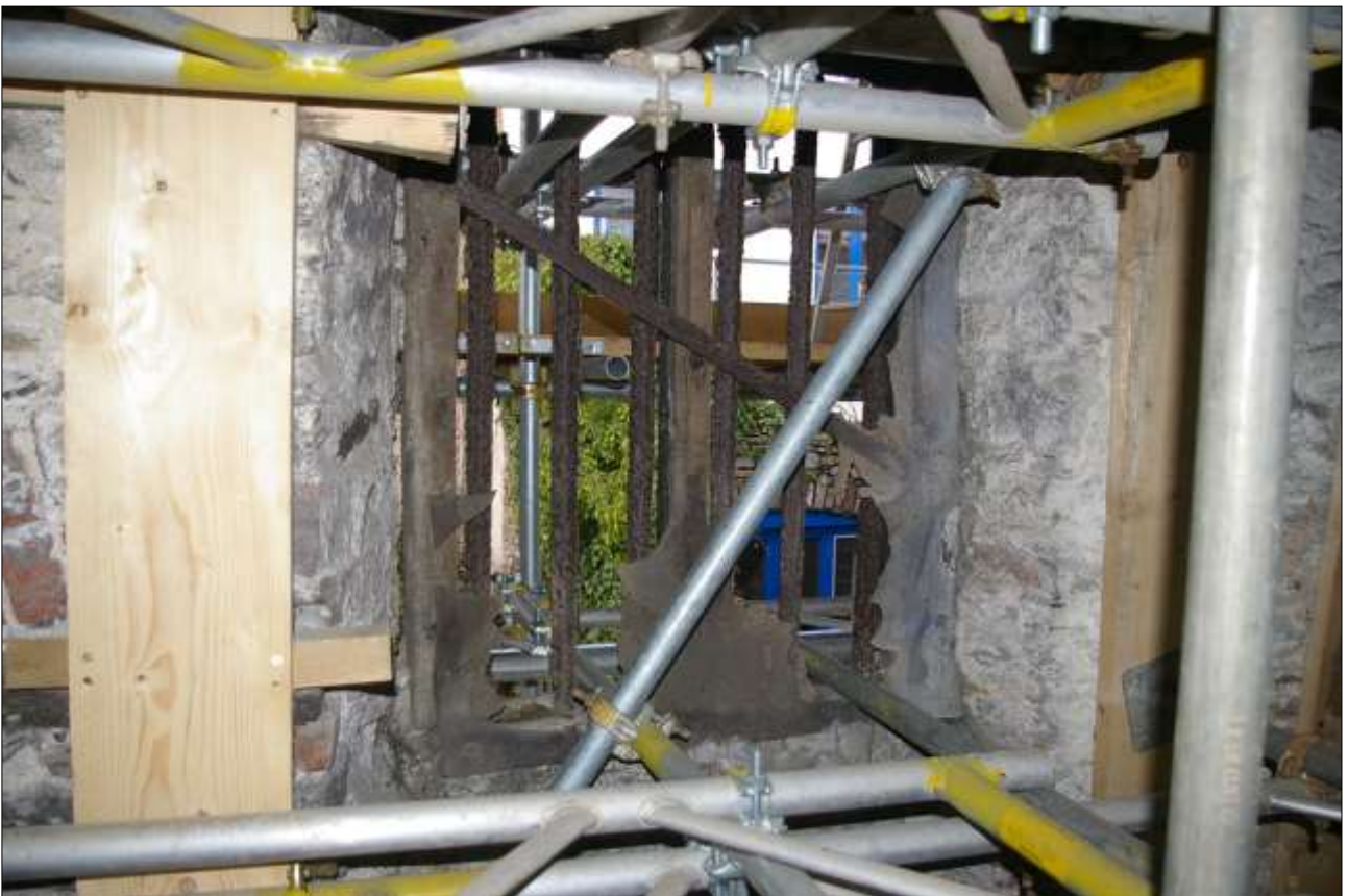
114. B2 FF INTERIOR, NORTH WALL, SHOWING W13; VIEWED FROM THE SOUTH.
