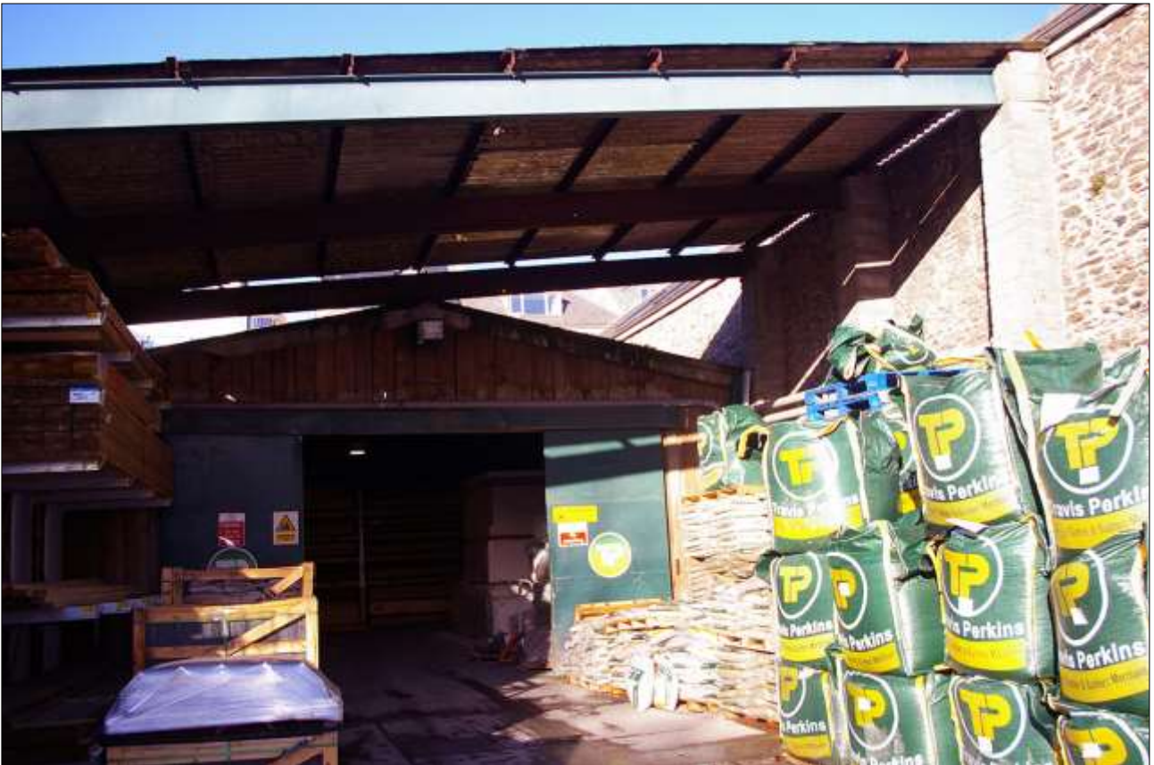
193. B4; VIEWED FROM THE SOUTH.
