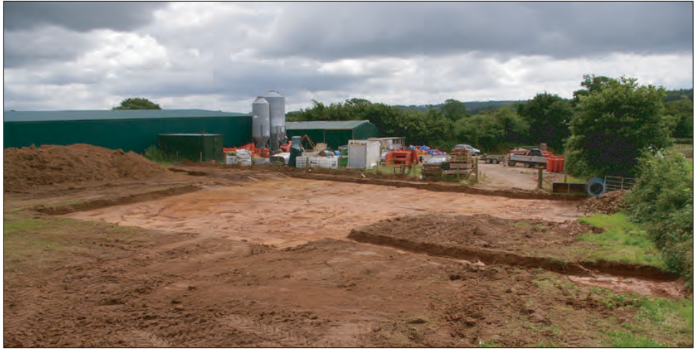
Plate 1: Hurdles Farm, Upton Pyne: the excavated area from the north-west.
