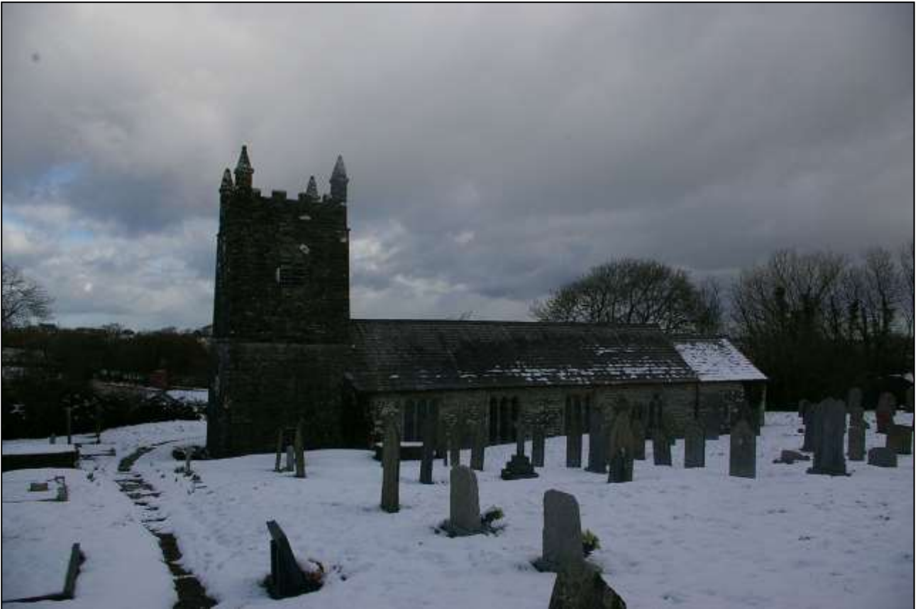
THE CHURCH WITHIN ITS CHURCHYARD; FROM THE SOUTH-WEST.
