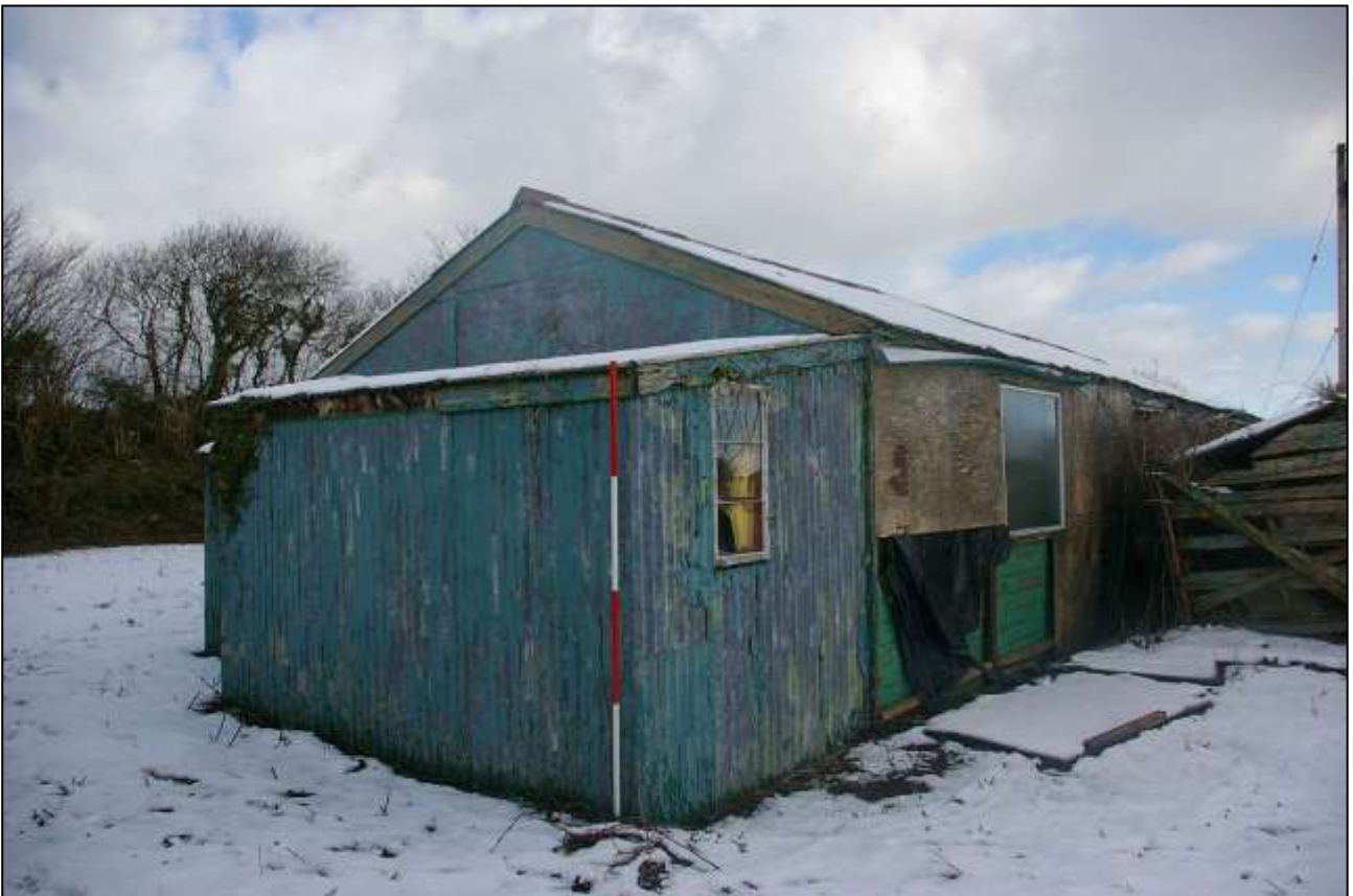
THE LEAN-TO SHEDS, OF CORRUGATED SHEETING TO THE WEST, WITH 2M SCALE; FROM THE SOUTH-WEST.
