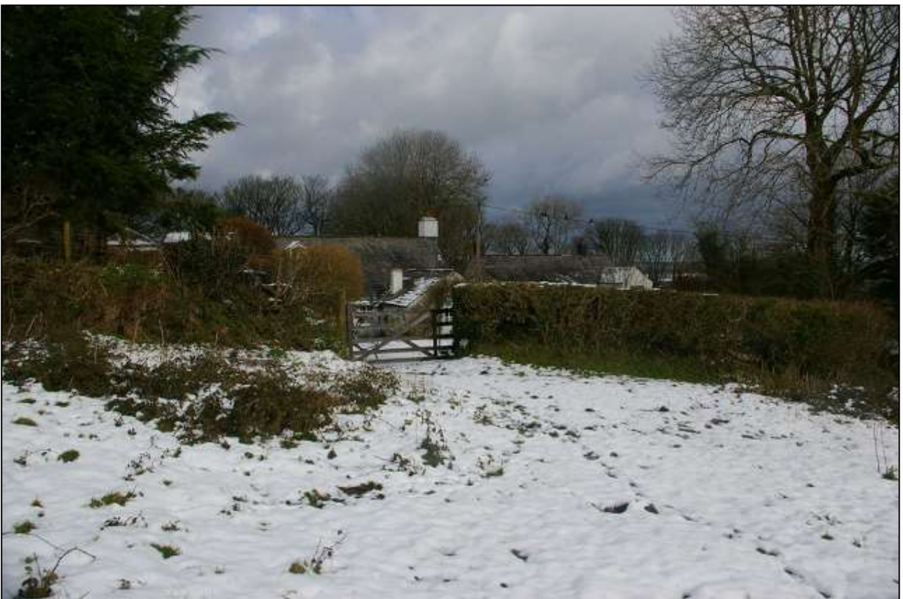
VIEW FROM THE COMMON TO THE LISTED BUILDINGS, SHOWING SCREENING FROM GARDEN AND HEDGE TO THE COTTAGE AND THE LOW LYING LOCATION OF THE MANOR BEYOND; FROM THE SOUTH-WEST.
