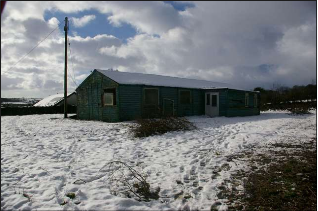
THE SITE AND ITS CURRENT BUILDING; FROM THE NORTH-EASTERN ENTRANCE GATEWAY.
