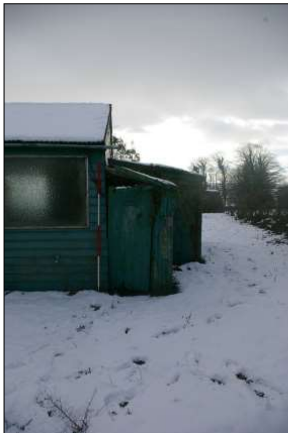
THE CORRUGATED SHEDS TO THE NORTH OF THE MAIN BUILDING, WITH 2M SCALE; FROM THE NORTH.
