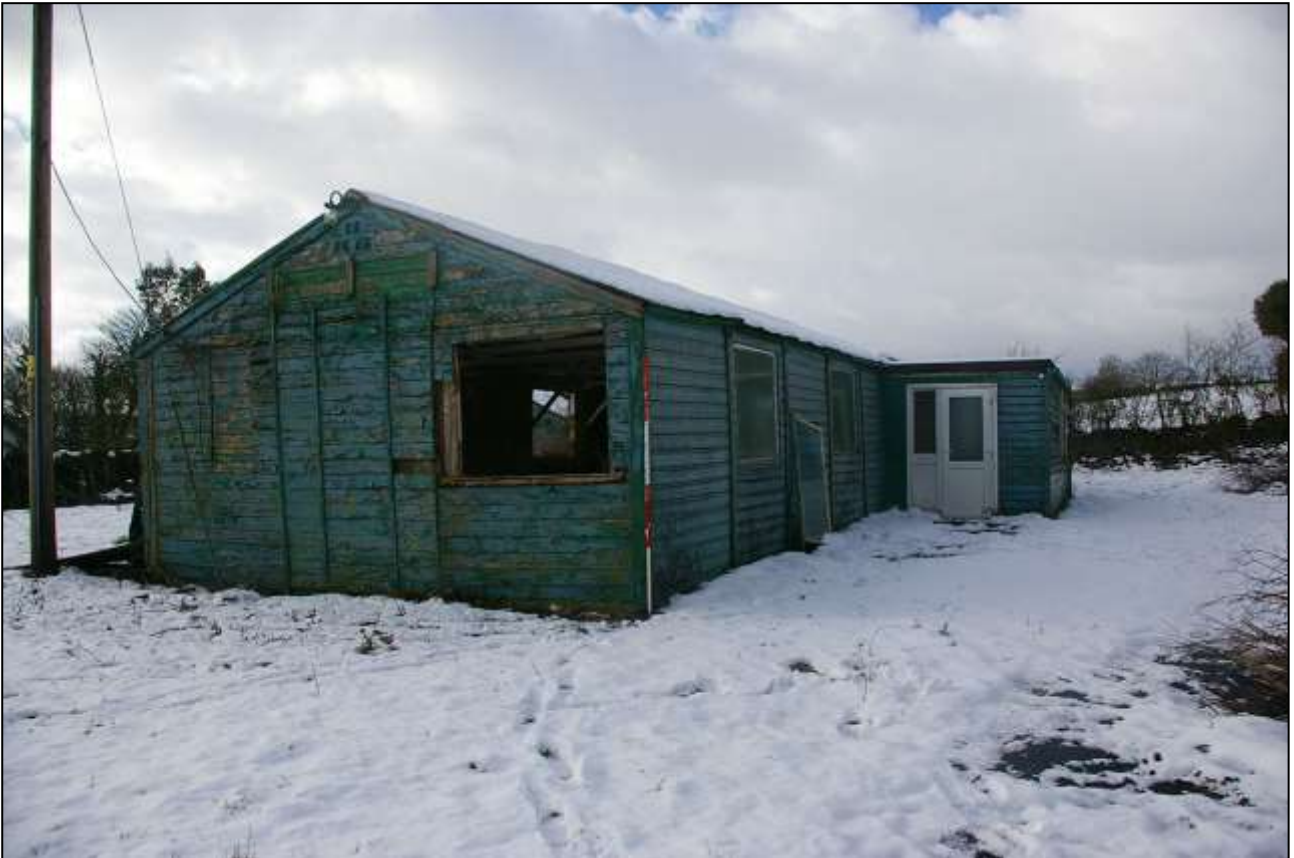
THE SOUTH-EAST CORNER OF THE BUILDING AND ENTRANCE TO THE PORCH, WITH 2M SCALE; FROM THE NORTH-EAST.
