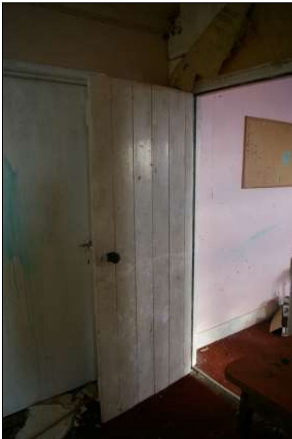
LEFT: BOARDED PLANK DOOR BETWEEN THE TWO ROOMS IN THE BUILDING; FROM THE WEST, SOUTH-WEST.
