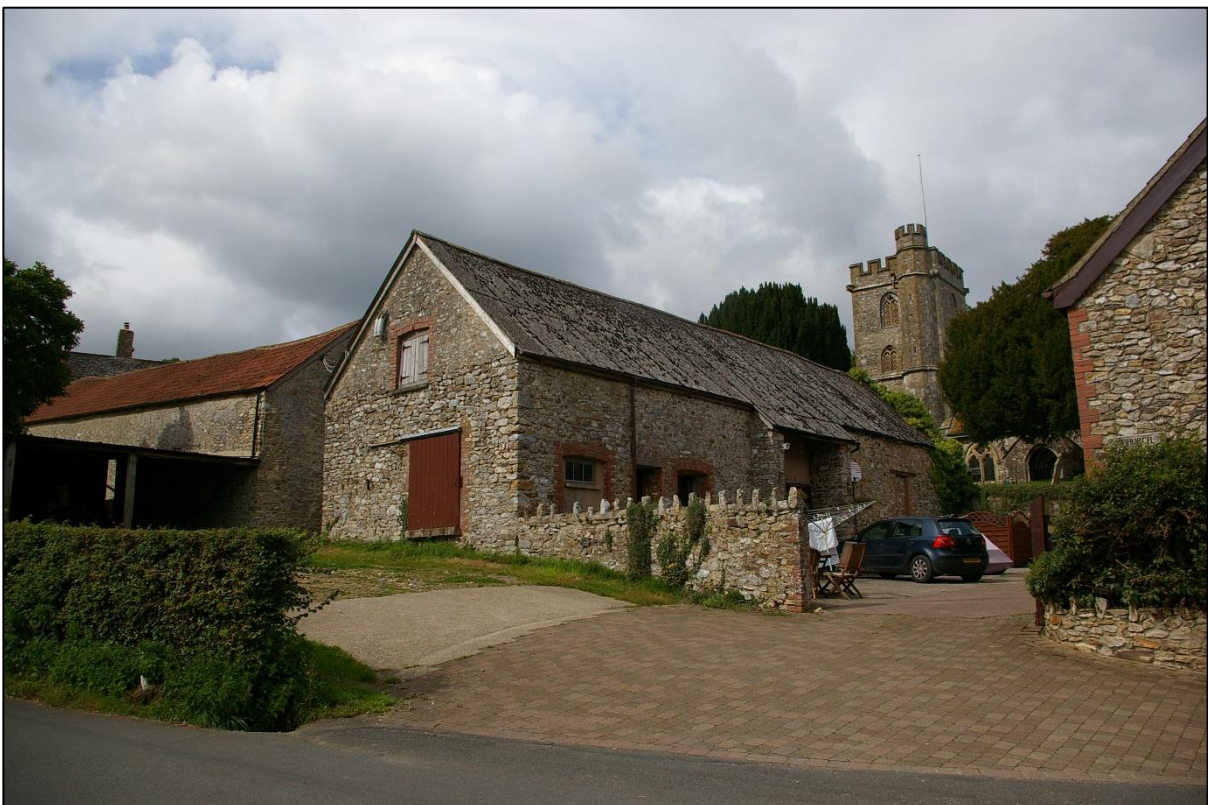
Figure 3: View of the church, from the lane, showing it enclosed and framed by the historic barns of Churchstyle Farm; from the south-south-east. [distance c.65m]
