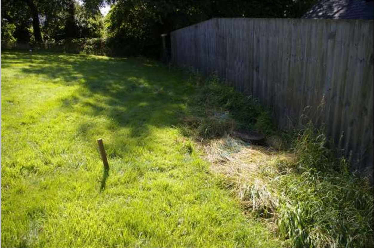
3. THE WESTERN BOUNDARY OF THE SITE, SHOWING THE MANHOLE COVER; VIEWED FROM THE NORTH (NO SCALE).
