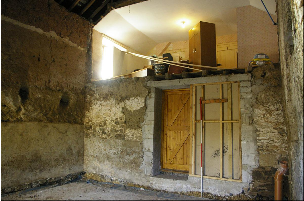
FIGURE 4: THE WEST PARTITION WALL; VIEWED FROM THE NORTH-EAST (2M SCALE).
