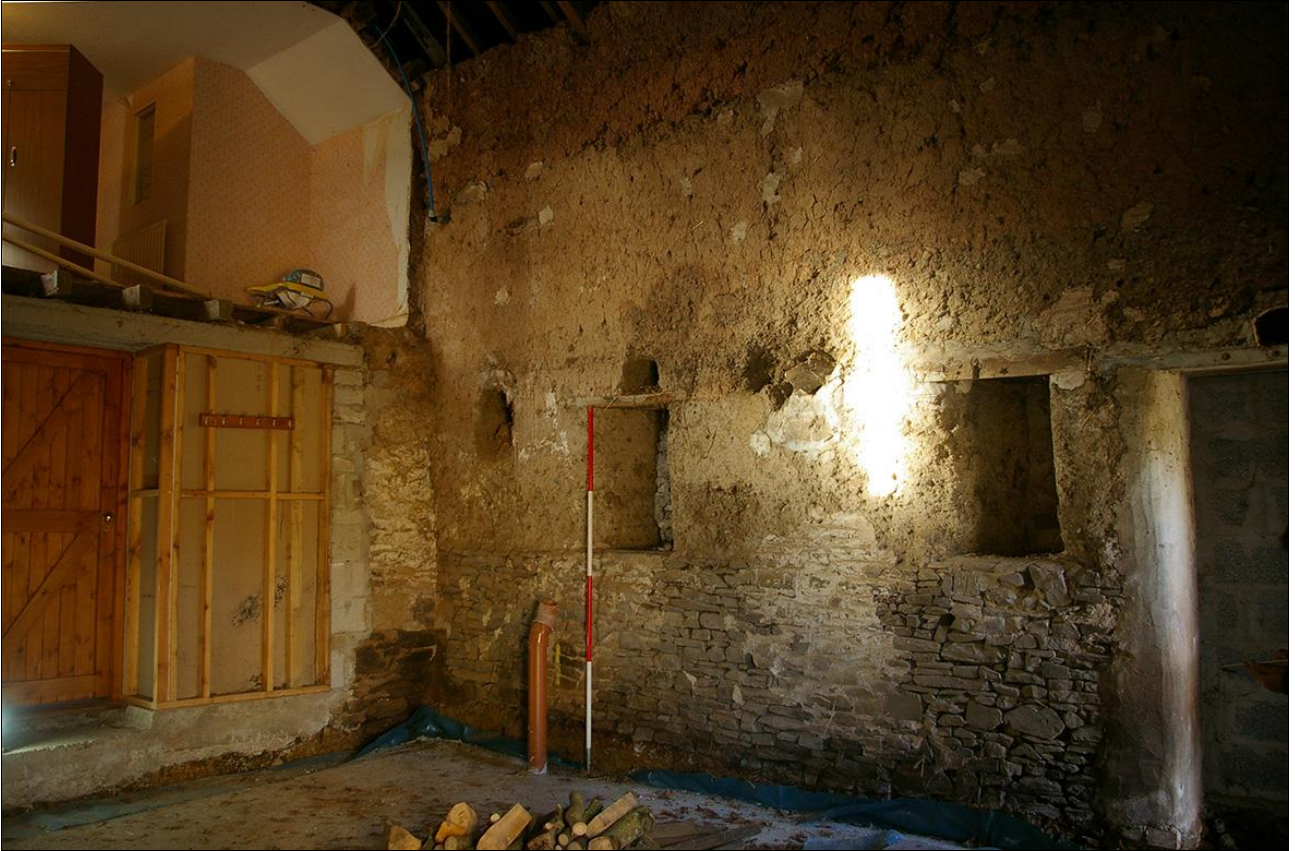
9. THE INTERIOR, NORTH WALL; VIEWED FROM THE SOUTH-EAST (SCALE 2M).
