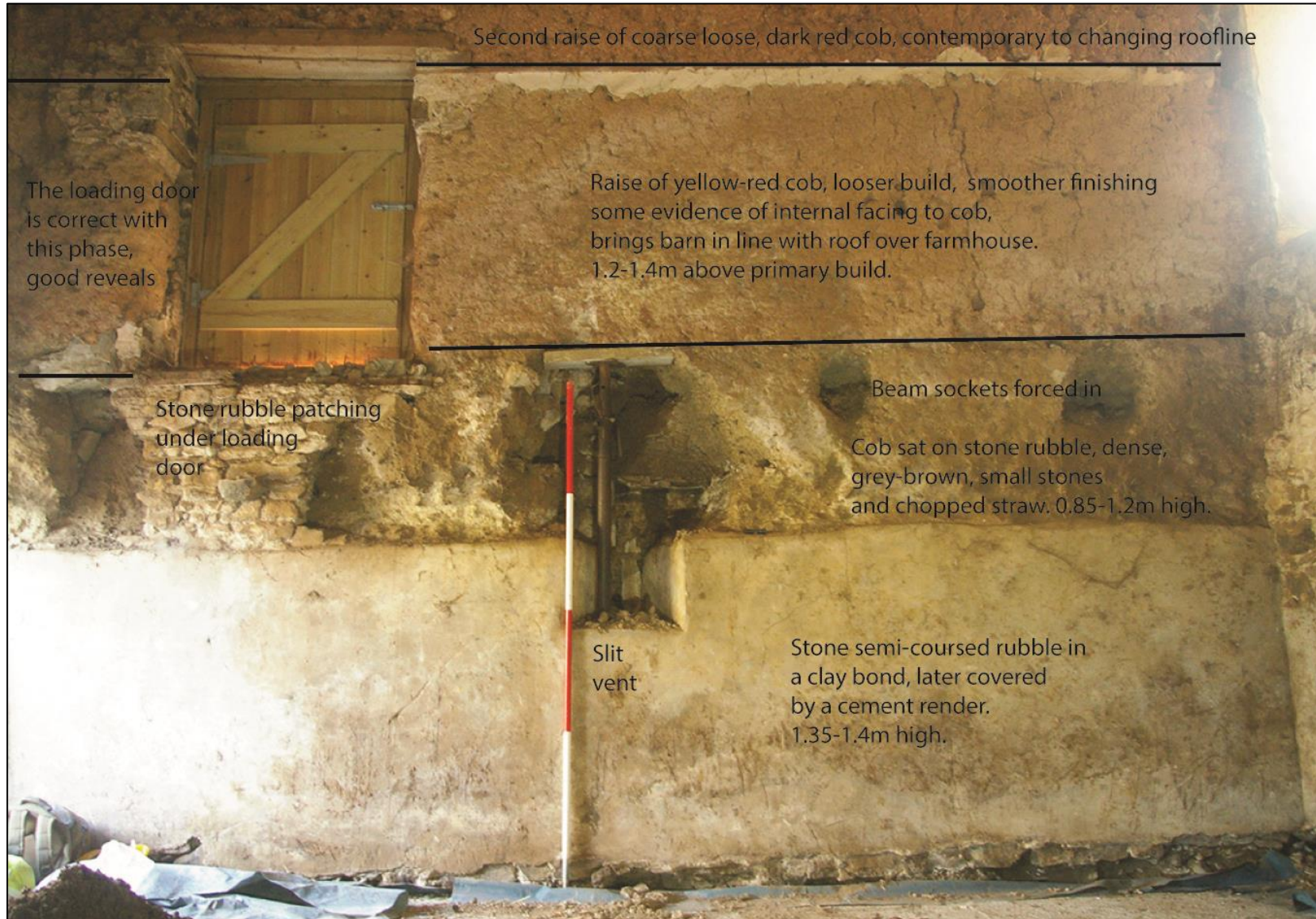
1. SOUTH WALL OF BRITTONS FARM SHIPPON, WITH 2M SCALE; WITH ANNOTATIONS AND NOTES ON STRUCTURAL PHASING.
