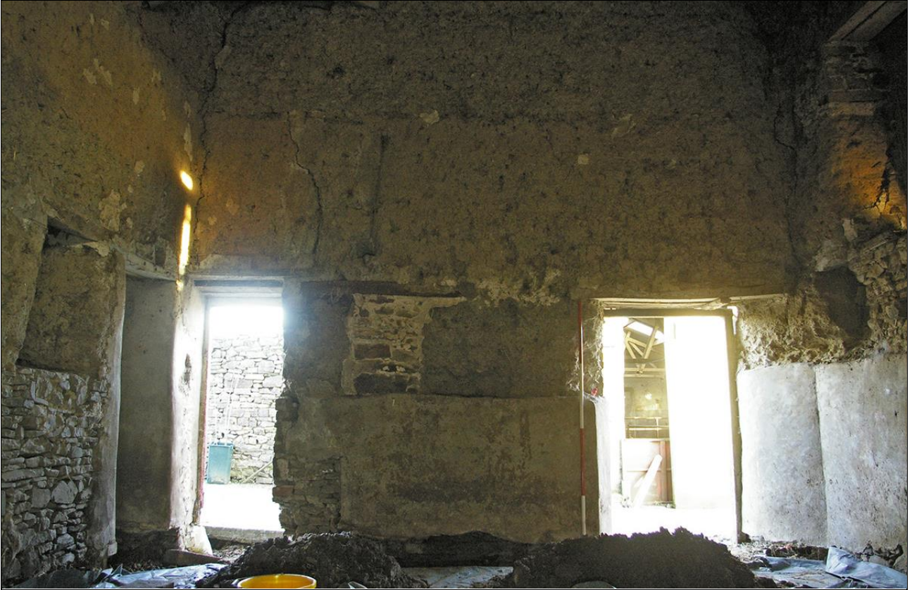
19. THE GABLE OF THE BARN; VIEWED FROM THE WEST (2M SCALE).
