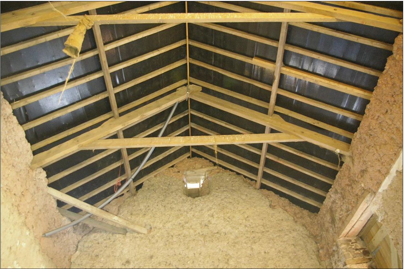
21. THE CURRENT ROOF OF THE BARN; VIEWED FROM THE WEST.
