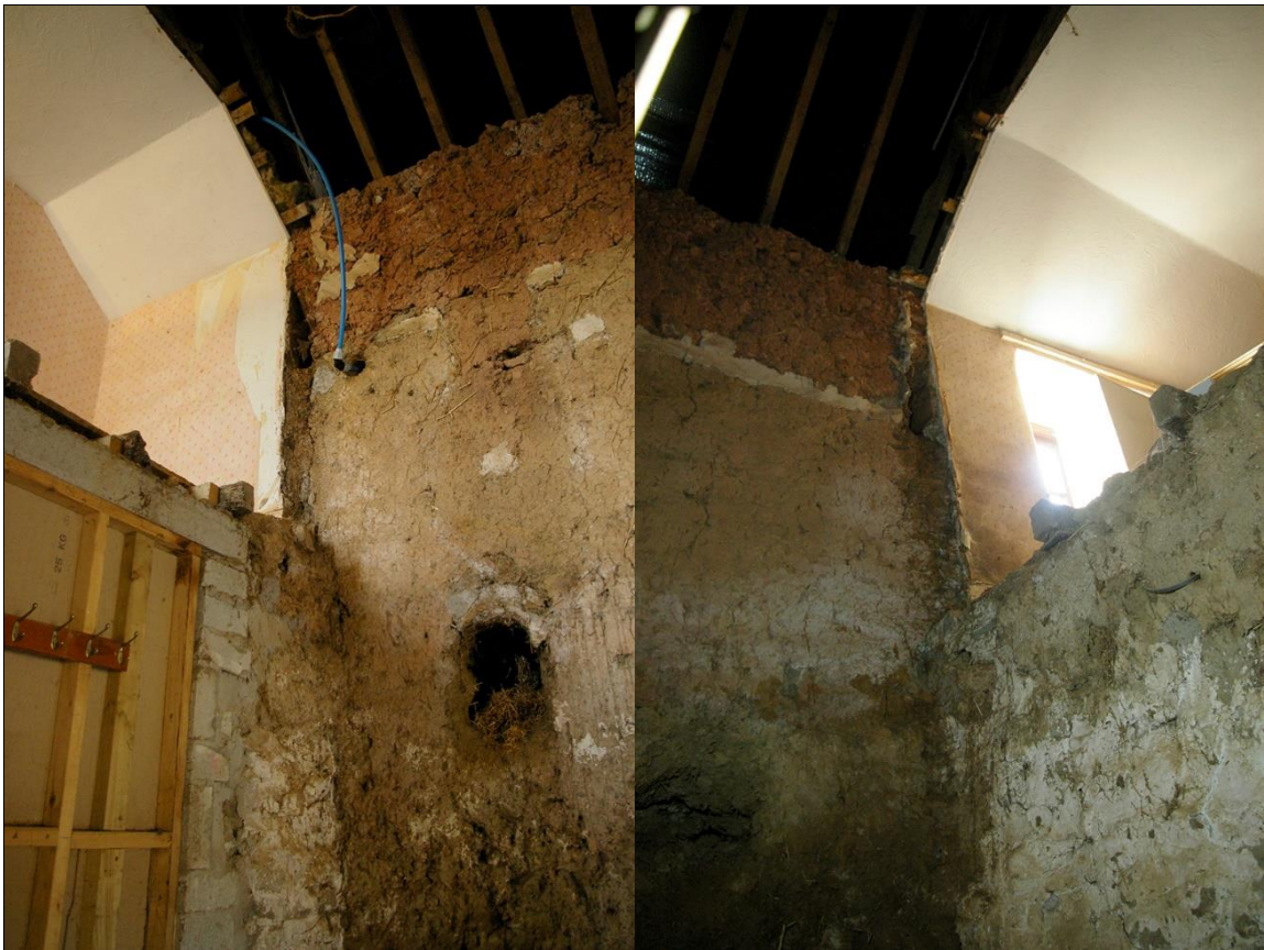
13. LEFT: THE NORTH-WEST CORNER OF THE BARN, SHOWING A LARGE EMPTY SOCKET AND POSSIBLE INFILLED SLOT BELOW; VIEWED FROM THE SOUTH-EAST. 14. RIGHT: THE SOUTH-WEST CORNER OF THE BARN, SHOWING A LARGE EMPTY SOCKET WITH POSSIBLE INFILLED SLOT BELOW; VIEWED FROM THE NORTH-EAST.
