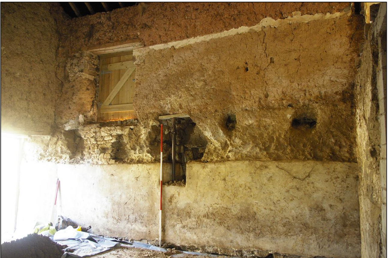
16. THE SOUTH WALL, INTERIOR FACE; VIEWED FROM THE NORTH-WEST (2M SCALE).
