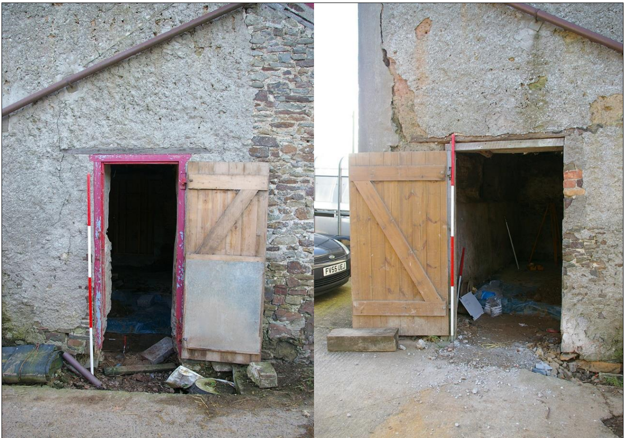
7. LEFT: THE NORTHERN OF THE TWO DOORWAYS IN THE EAST ELEVATION, WITH REUSED FRAME; VIEWED FROM THE ENE (2M SCALE).
