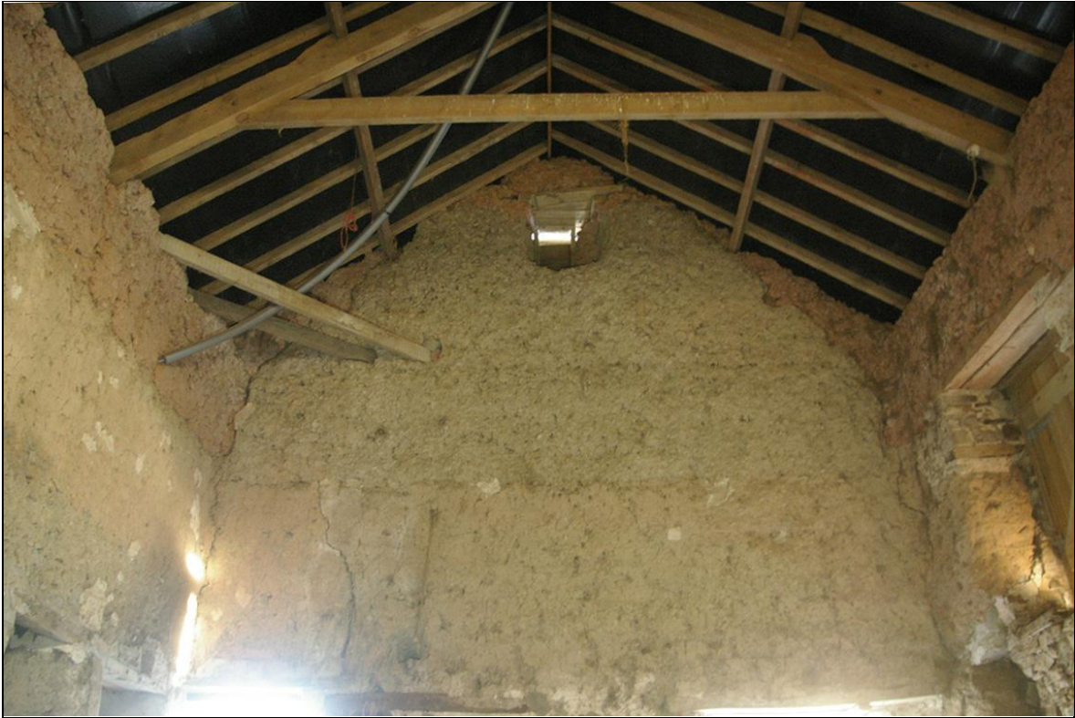
FIGURE 6: THE APEX OF THE EAST GABLE; VIEWED FROM THE WEST.
