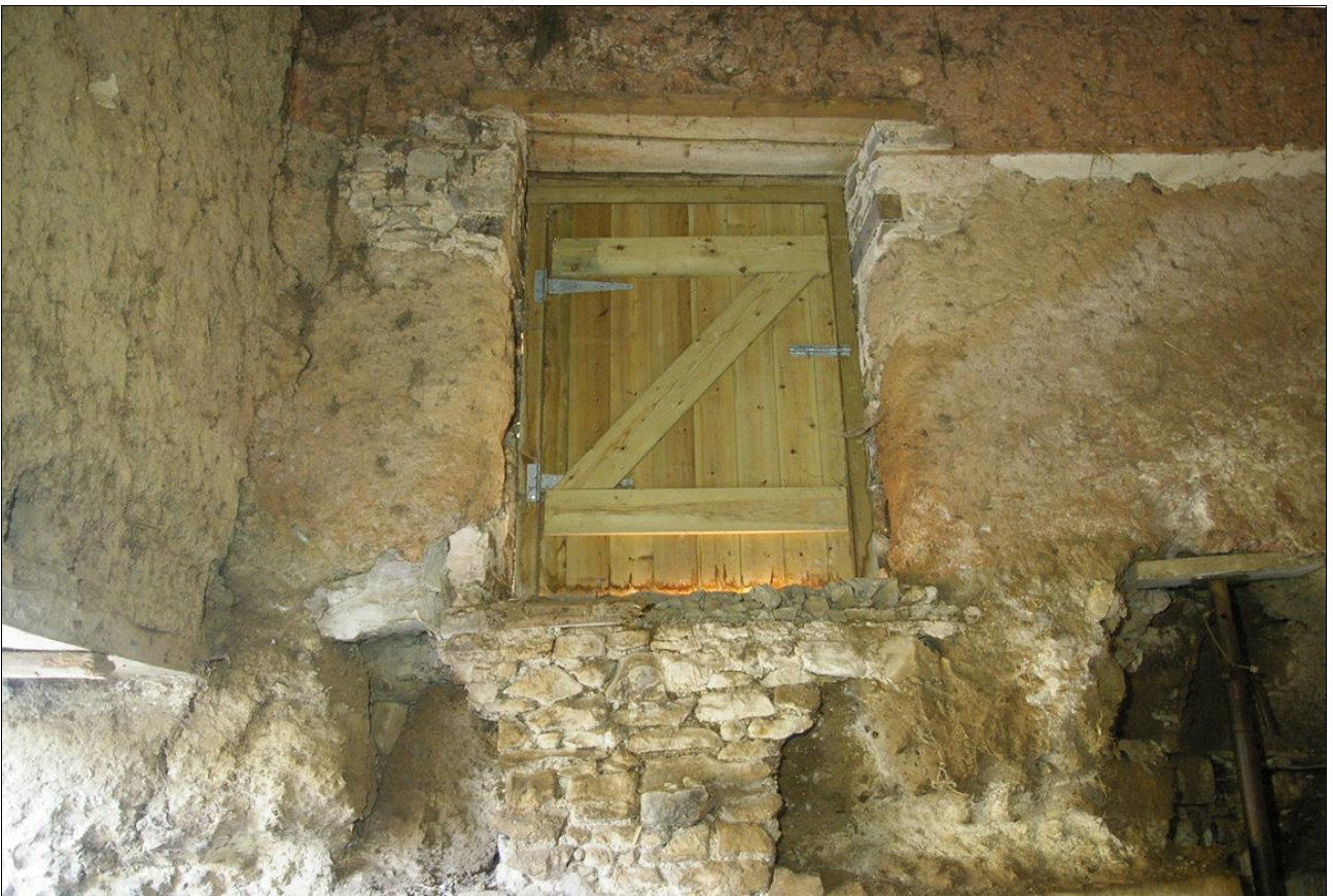
18. THE LOADING DOOR IN THE SOUTH WALL; VIEWED FROM THE NORTH.
