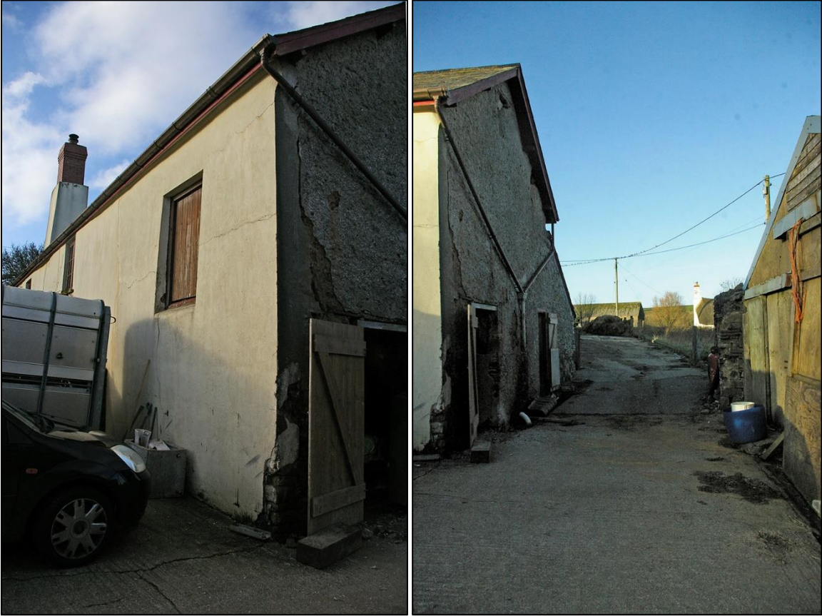
3. LEFT: THE SOUTH ELEVATION OF THE 'SHIPPON'; VIEWED FROM THE ESE.
