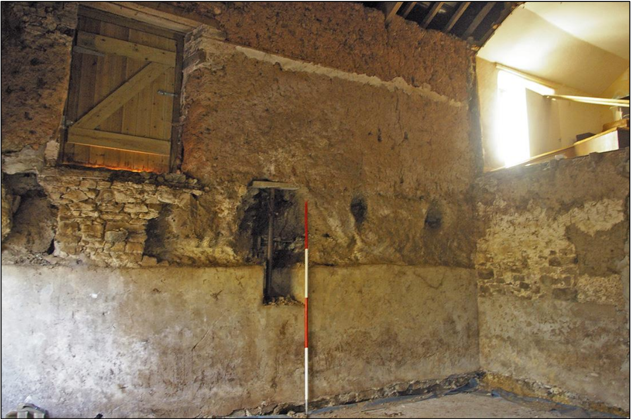
15. THE SOUTH WALL, INTERIOR FACE; VIEWED FROM THE NORTH-EAST (2M SCALE).
