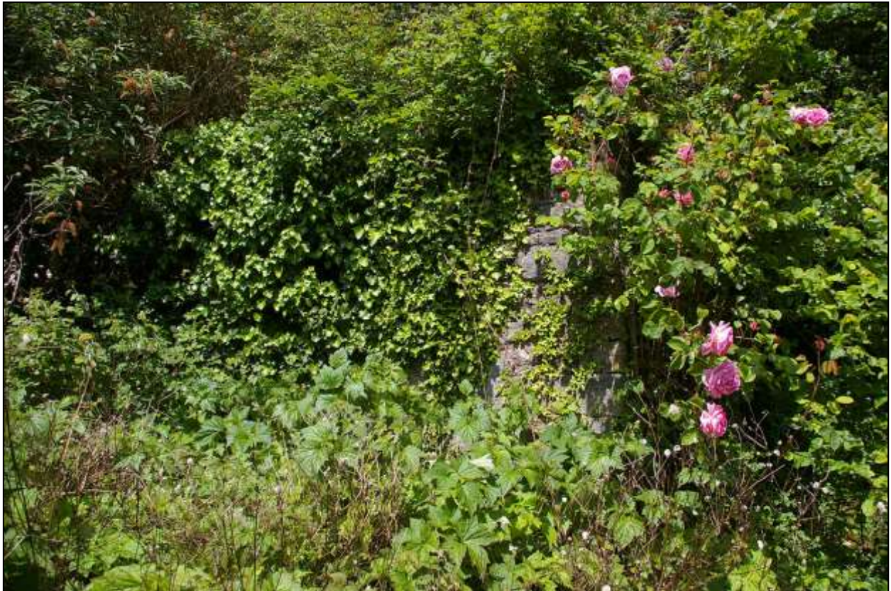
THE SOUTH-EAST CORNER OF THE SQUARE BLOCK, SHOWING ITS GOOD SHAPED BLOCK QUOINS; FROM THE SOUTH-EAST.
