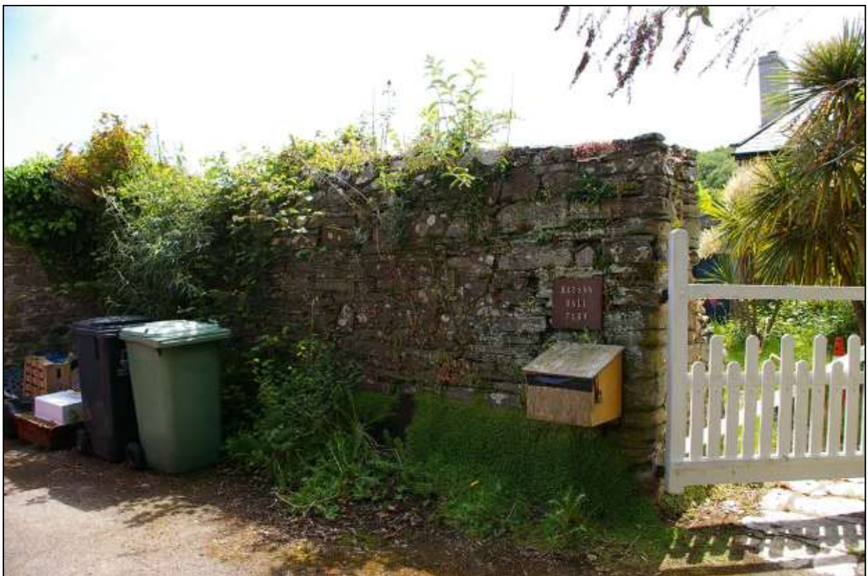
THE NORTH OUTER FACE OF THE HEAVY SLATESTONE WALL, WHICH IS THE FORMER GABLE END OF AN EARLY BUILDING; FROM THE NORTH-WEST.
