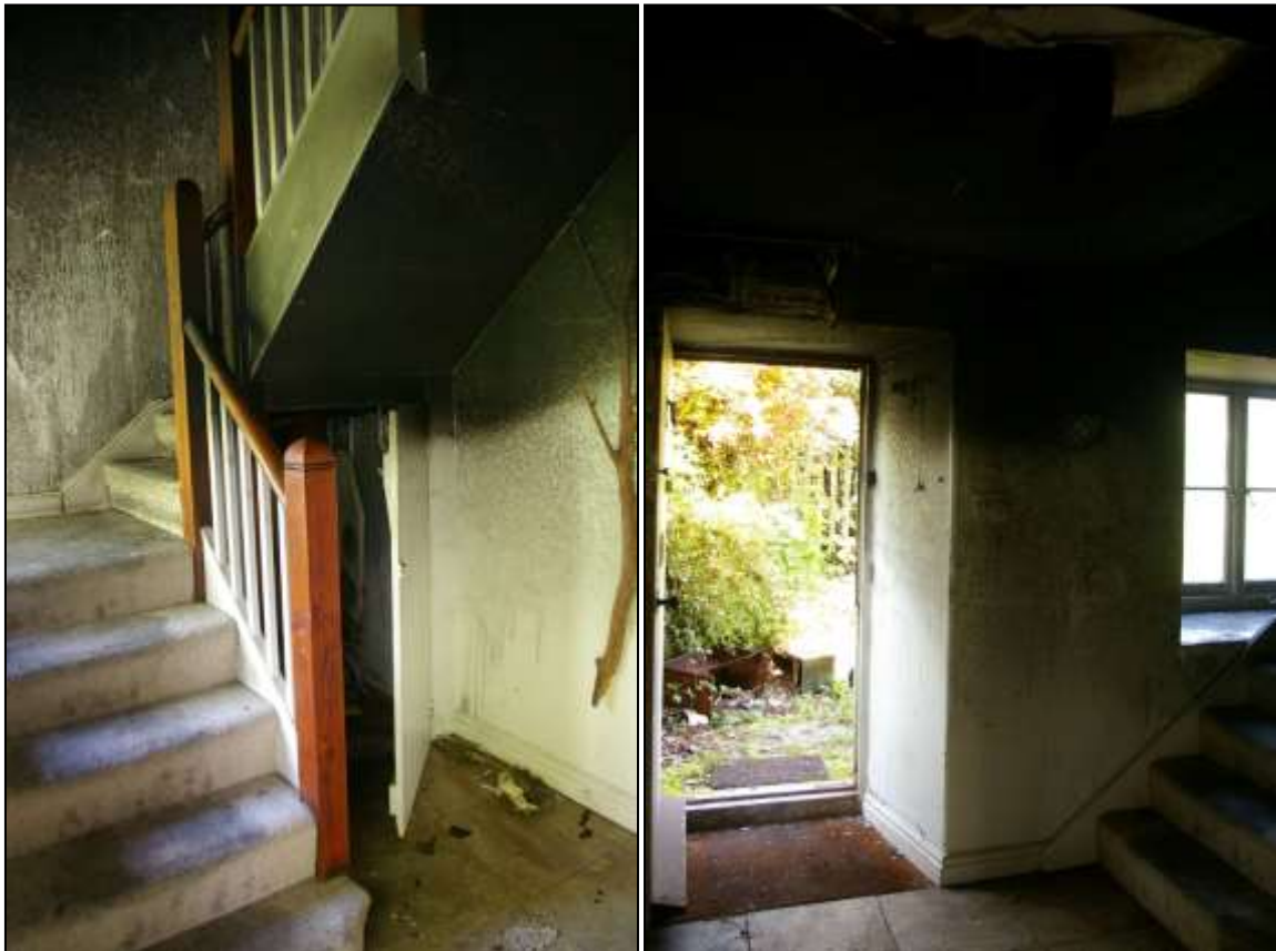
LEFT: VIEW OF THE LATE 20 TH CENTURY TIMBER STAIRCASE, HEAVILY SMOKE BLACKENED; FROM THE NORTH-WEST.
