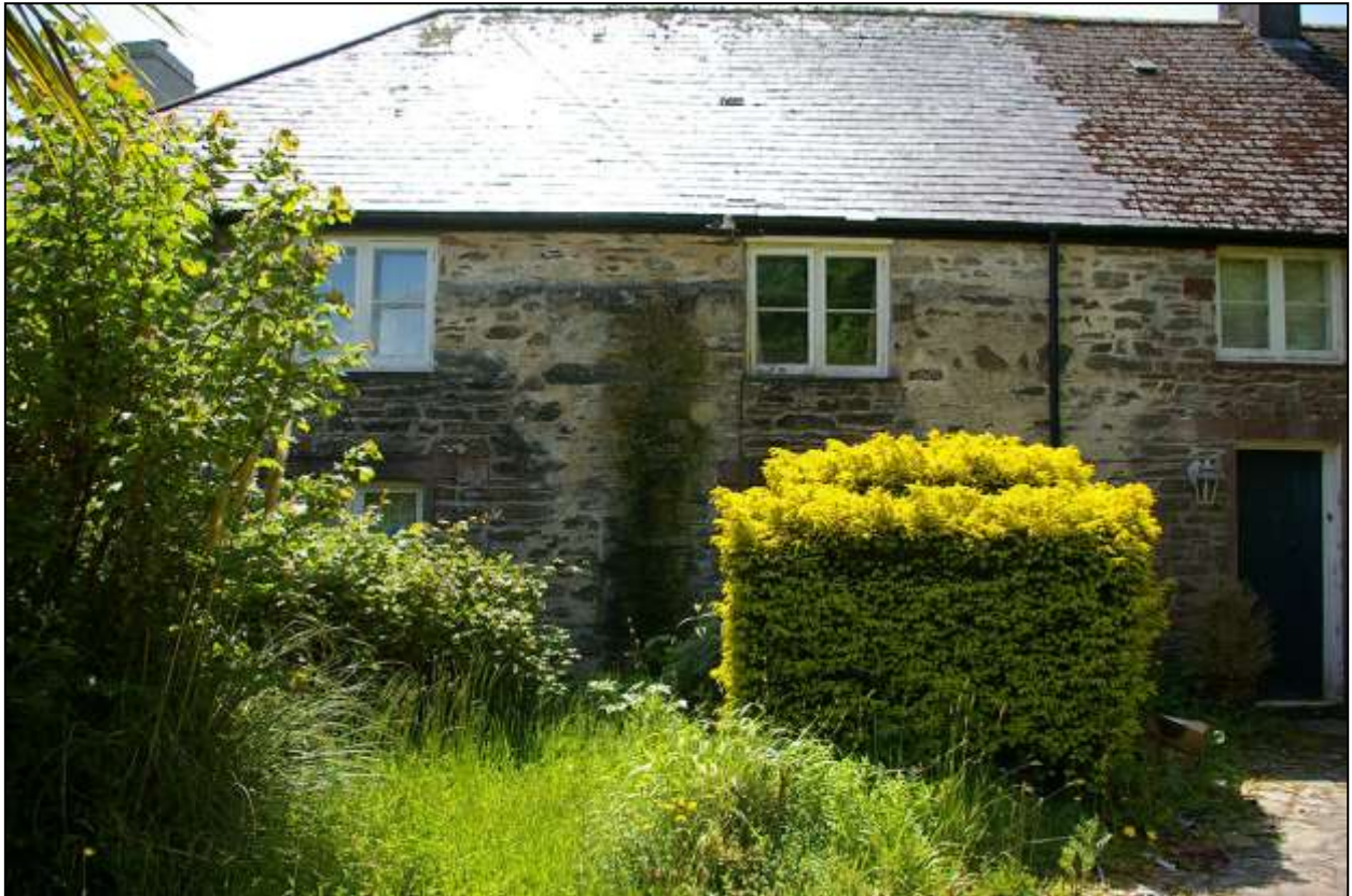
DETAILED VIEW OF THE THICKER LOWER SECTION OF WALLING WHICH DOMINATES THE NORTH FRONT OF THE FARMHOUSE, AT THE EAST END, THE REMAINS OF A RUINED EARLIER BUILDING; FROM THE NORTH.
