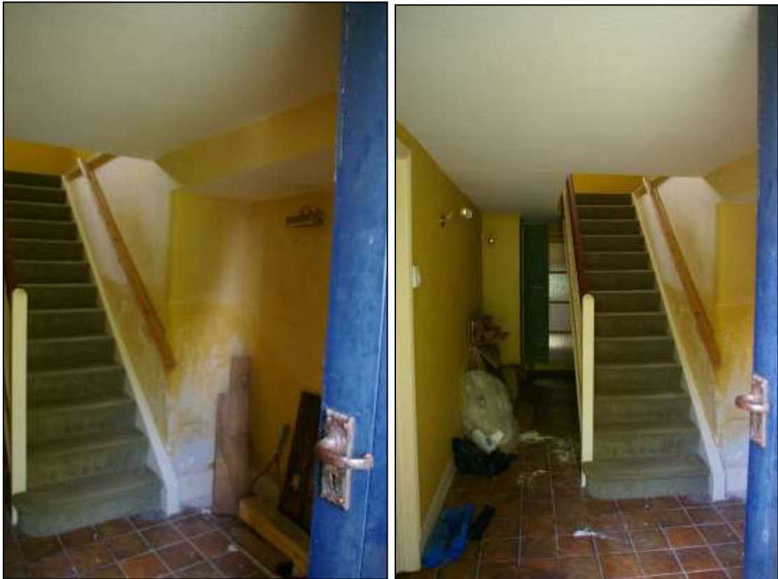
LEFT: INTO THE ENTRANCE HALLWAY AND STAIRS, ROOM 1, SHOWING HOW THIS DOOR HAS BEEN FORCED UP AGAINST THE PARTY WALL TO THE COTTAGE, WHICH HAS A LARGE BLOCKED DOORWAY WITHIN IT; FROM THE NORTH-EAST.
