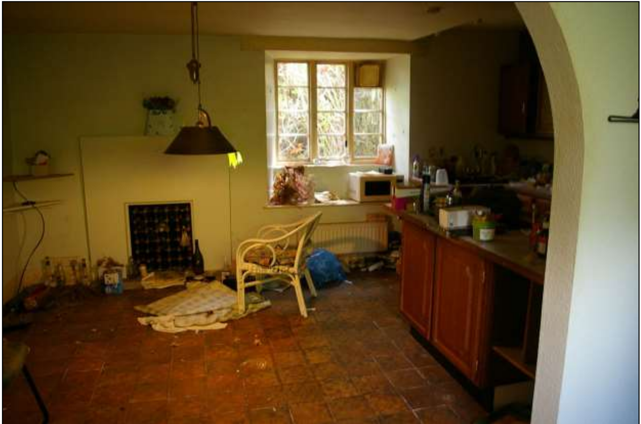
THE FITTED KITCHEN, WITH THE THREE LIGHT 19 TH CENTURY CASEMENT AND WINDOW SEAT, BLOCKED FIREPLACE ON THE REAR WALL, MODERN QUARRY TILED FLOOR, BOARDED OUT CEILING WHICH OBSCURES A CHANGE IN CEILING HEIGHT; FROM THE NORTH, NORTH-EAST.
