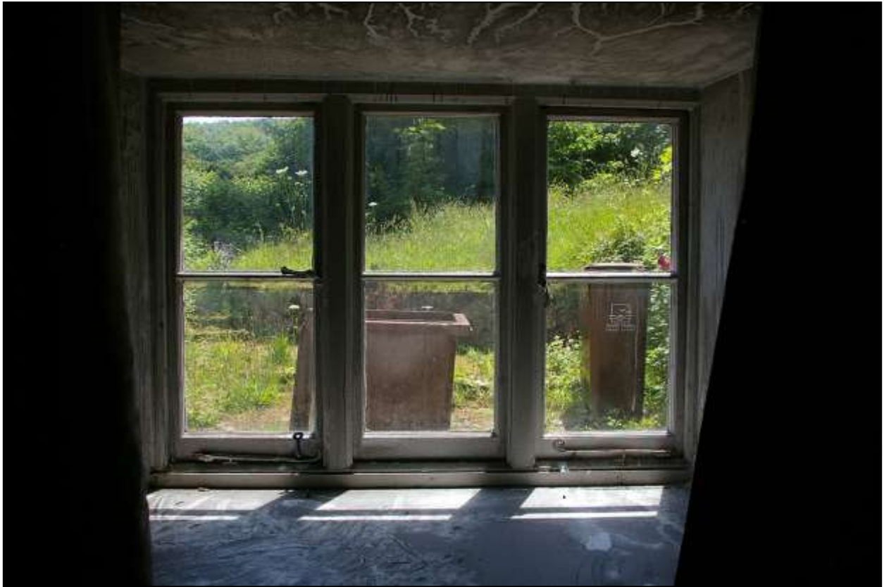
DETAIL OF THE GOOD 19 TH CENTURY THREE LIGHT CASEMENT WINDOW CW3; FROM THE NORTH.
