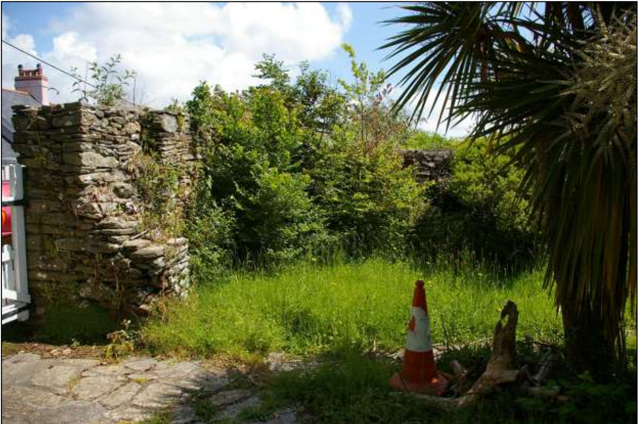
DETAIL OF THE NORTH GABLE END WALL OF THE EARLIER BUILDING, WHICH NOW FORMS THE GARDEN WALL, SHOWING A STUB RUNNING BACK TOWARDS THE HOUSE; FROM THE WEST, SOUTH-WEST.
