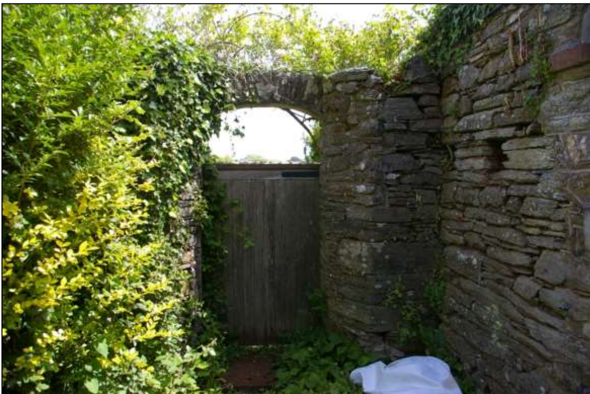
FIGURE 6: DETAILED VIEW OF THE FINE HEAVY SLATESTONE AND SOME DRESSED BLOCKS AND PUTLOGS, ALL OF WHICH IDENTIFY THESE GARDEN WALLS AS RUINS OF AN EARLIER QUITE FINE BUILDING.
