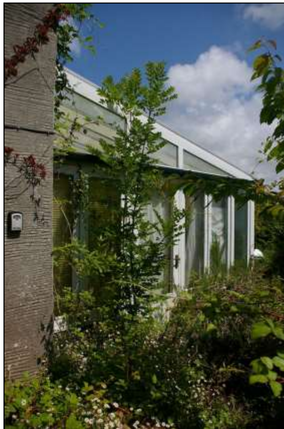
VIEW OF THE LARGE PLASTIC AND TIMBER CONSERVATORY WHICH DOMINATES THE EAST GABLE END OF THE FARMHOUSE AND THE GARDENS ON THIS SIDE; FROM THE SOUTH-WEST.
