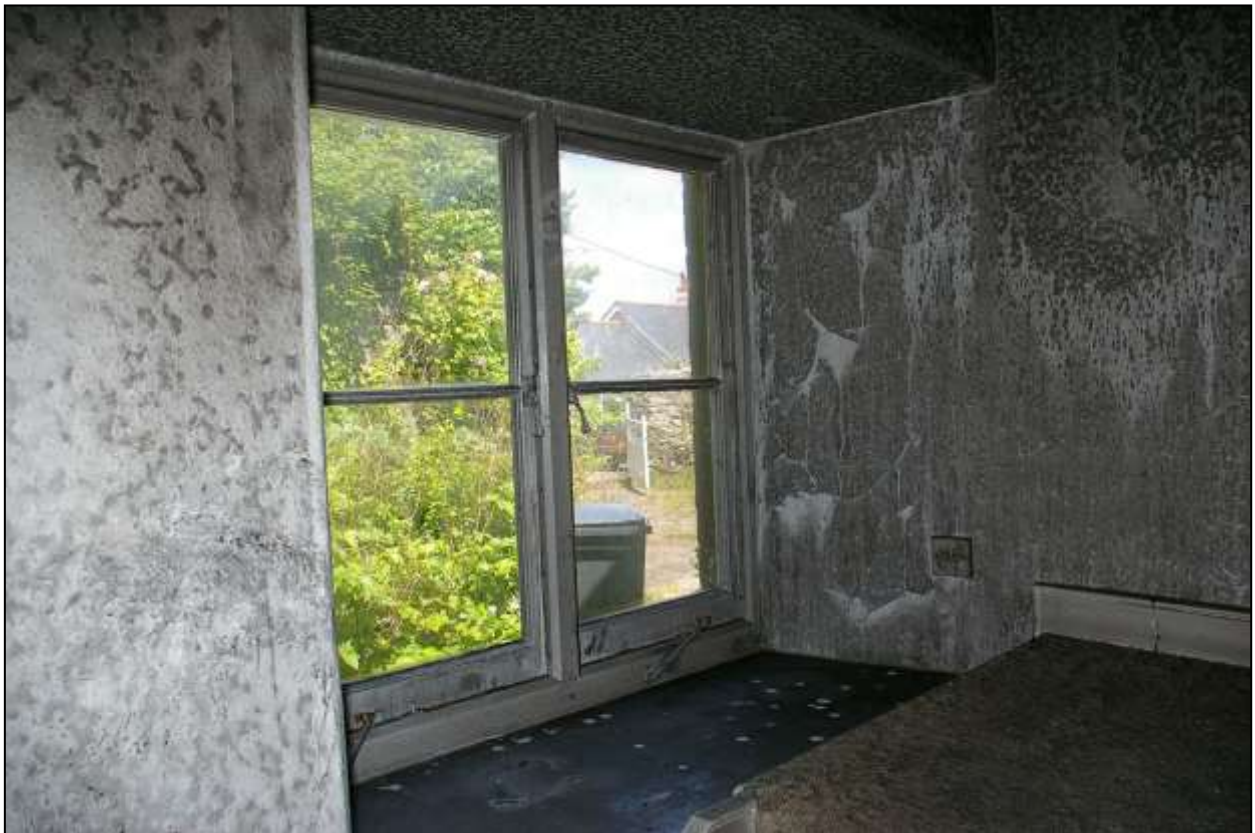
DEEP BEADED OPENING, PLANK SILL AND TWO LIGHT BEADED CASEMENT IN CHAMFERED PEGGED FRAME, A 19 TH CENTURY FEATURE CW1; FROM THE SOUTH-WEST.
