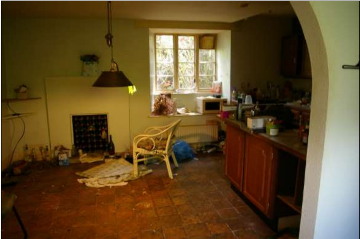
FIGURE 7: VIEW OF THE FITTED KITCHEN, WITH THE THREE LIGHT 19TH CENTURY CASEMENT AND WINDOW SEAT, BLOCKED FIREPLACE ON THE REAR WALL, MODERN QUARRY TILED FLOOR, BOARDED OUT CEILING; FROM THE NORTH, NORTH-EAST.
