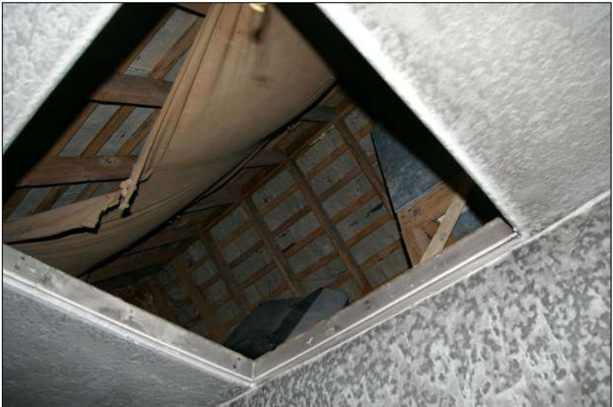
VIEW UP INTO THE LOFT, SHOWING THE MODERN COMMON RAFTER REPLACEMENT ROOF; FROM BELOW (NORTH-WEST).
