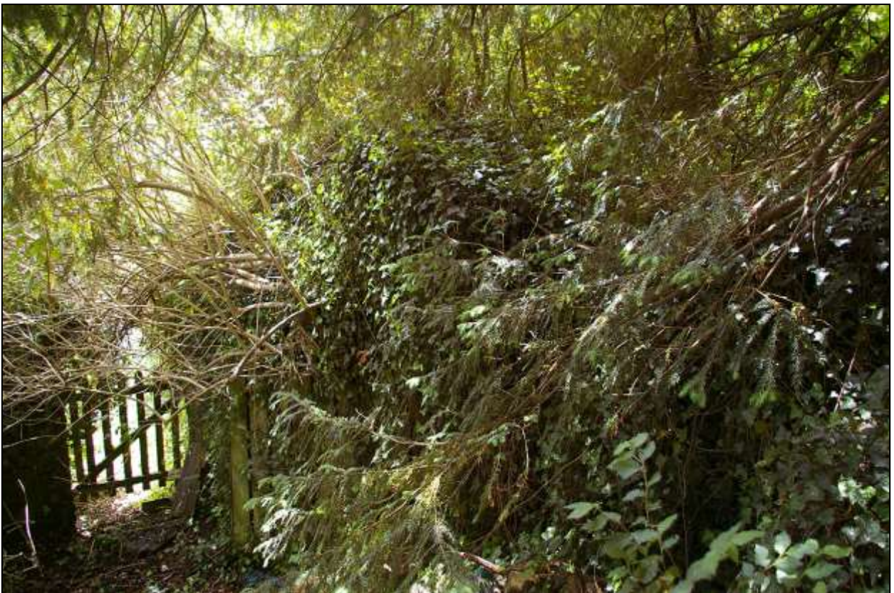
THE TALLER VERY THICK WEST WALL OF THE SQUARE BLOCK, WHICH LOOKS TO CONTAIN FURTHER OBSCURED FEATURES, POSSIBLY A STACK? FROM THE NORTH, NORTH-EAST.
