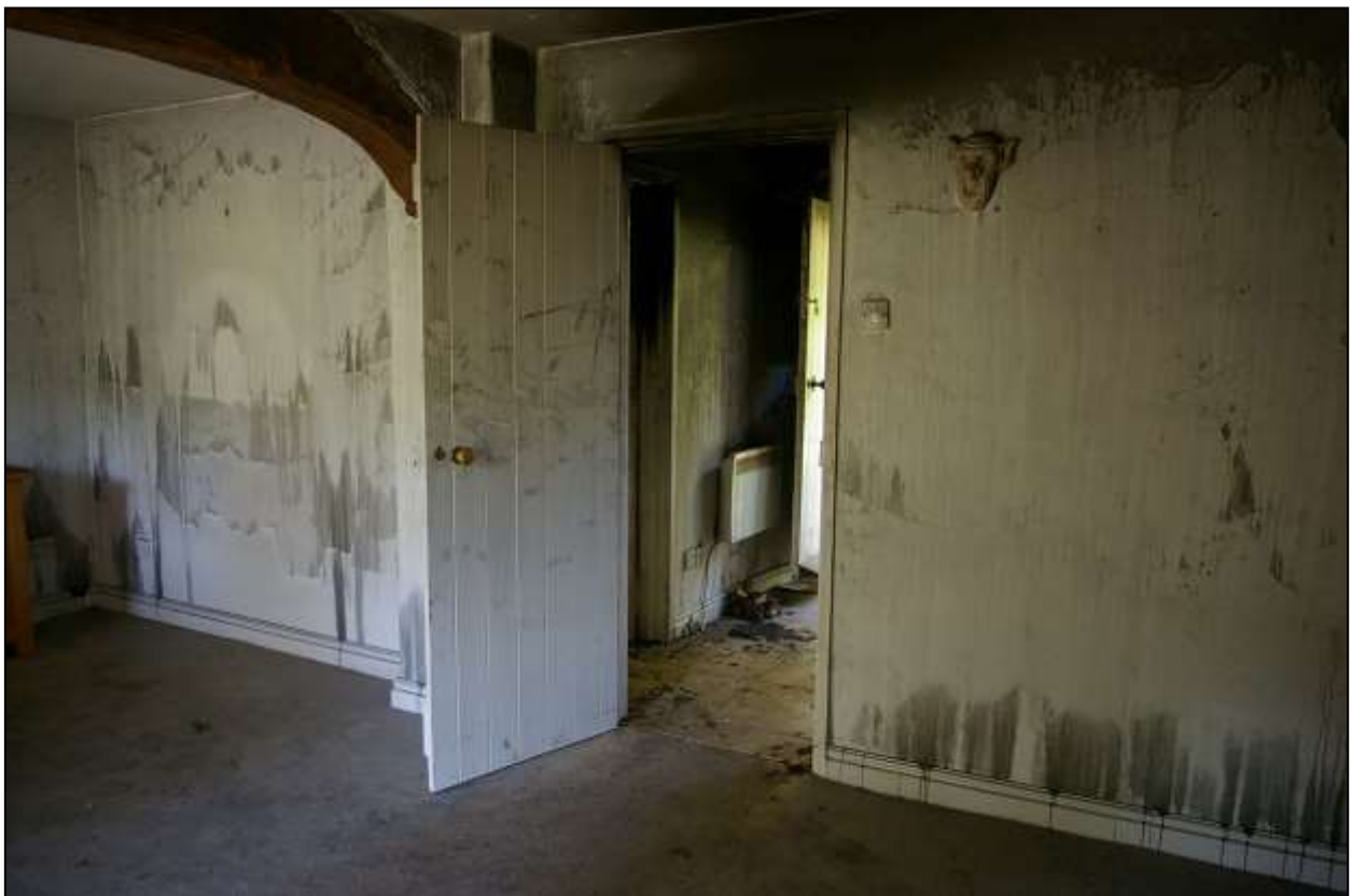
THE MODERN PARTITIONS, WITH A STUD OF EARLIER WALL BRACED BY A HACKED BACK BEAM IN CR3, THE SITTING ROOM, ALSO WITH DOOR BACK TO THE HALLWAY; FROM THE SOUTH-EAST.
