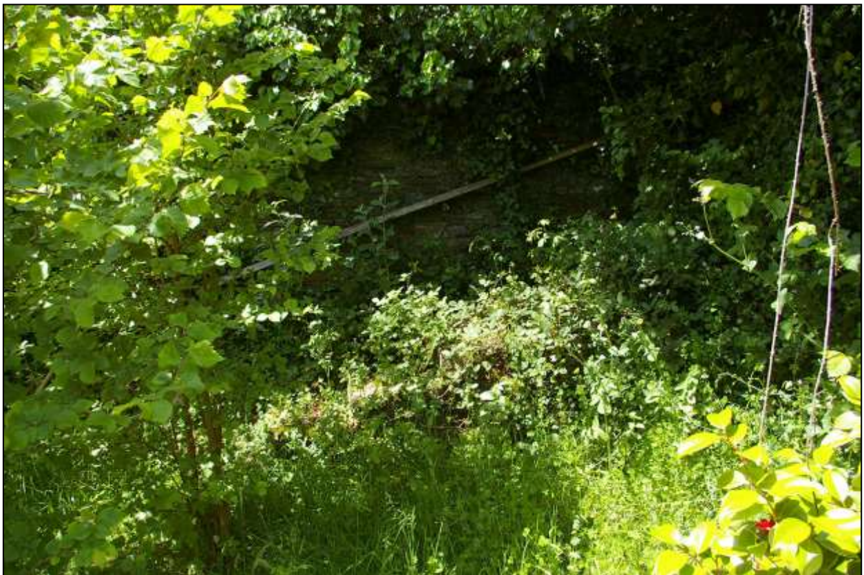
THE EAST WALL OF THE SQUARE BLOCK LARGELY OBSCURED BY IVY BUT ALSO WITH THE SET OF SATE GARDEN STEPS RISING ALONGSIDE IT; FROM THE EAST.
