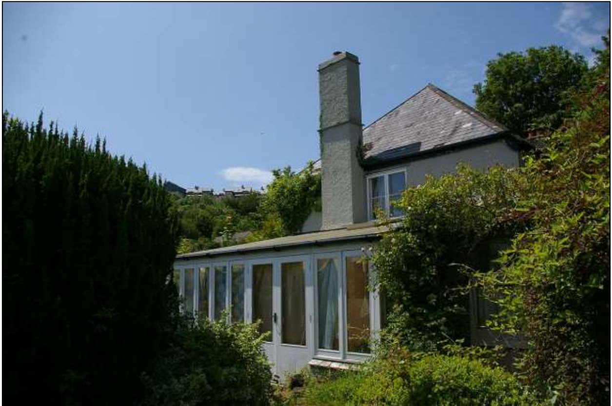
THE EAST GABLE END OF THE FARMHOUSE, WITH HIPPED ROOF, BOX STACK AND SHAFT AND LARGE MODERN CONSERVATORY; FROM THE NORTH-EAST.
