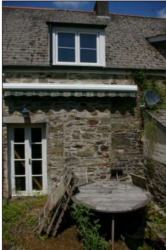
THE BLOCKED DOORWAY IN THE SOUTH ELEVATION OF THE COTTAGE IN THE SOUTH-EAST CORNER, SHOWING GOOD DRESSED REVEALS; FROM THE SOUTH.
