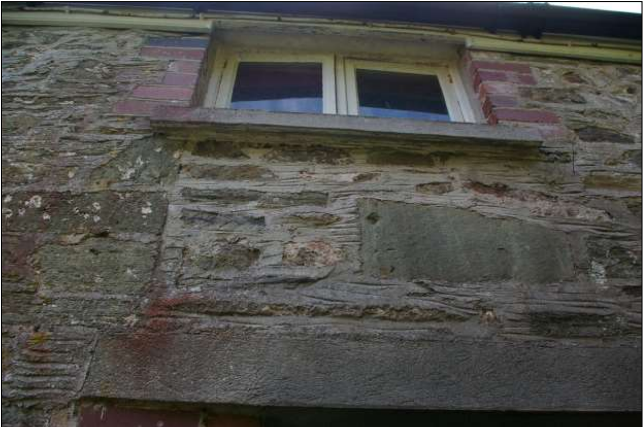
THE SMALL BLOCKED WINDOW WITH BRICK REVEALS SET INTO A LARGER OPENING, A LOADING DOOR ABOVE THE FORCED DOORWAY TO THE FRONT OF THE ATTACHED COTTAGE; FROM BELOW (NORTH-EAST).
