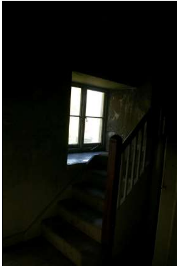
VIEW OF HOW THE STAIRCASE, MODERN CUTS THE HISTORIC WINDOW IN THE FRONT WALL OF THE COTTAGE IN CR1; FROM THE SOUTH-WEST.
