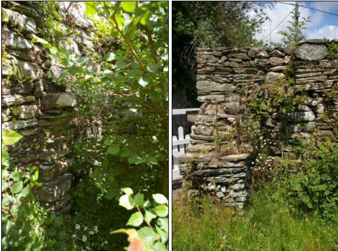
LEFT: VIEW OF THE RAISED FLAT BUILT PILASTERS AND PADSTONE WHICH WOULD HAVE CARRIED A STONE OR WOOD CORBELLED BRESUMMER OVER A LARGE OPEN FIREPLACE; FROM THE SOUTH-WEST.
