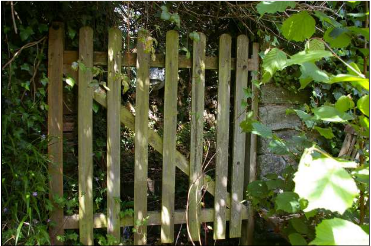
THE GATE IN THE SOUTH-WEST CORNER OF THE SQUARE RUINS, SHOWING FINE QUOINS TO THE EAST SIDE, BUT NARROW THIN BRICKS PATCHING THE WEST REVEALS; FROM THE SOUTH.
