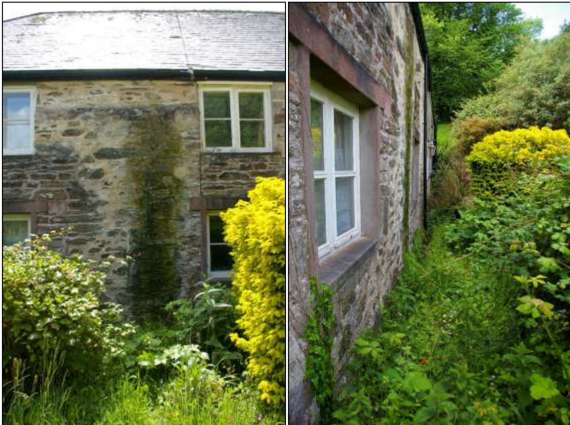
LEFT: DETAIL WITHIN THE RUINED WALL INCORPORATED INTO THE BUILDING SHOWING A POTENTIAL SET OF RAGGED LARGE SLAB QUOINS AND ALSO A POTENTIAL BLOCKED OPENING AT GROUND FLOOR; FROM THE NORTH.
