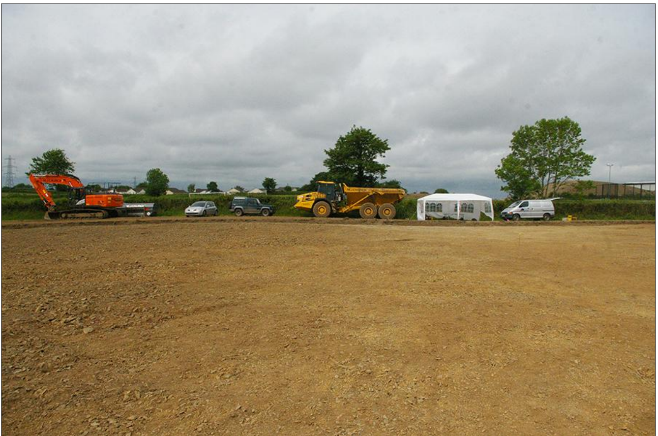
85. GENERAL SITE SHOT, EAST END; VIEWED FROM THE WEST (NO SCALE).
