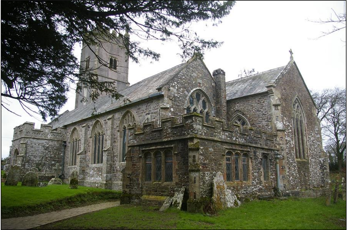
9. VIEW OF ST JAMES'S CHURCH; VIEWED FROM THE SOUTH-EAST (NO SCALE).
