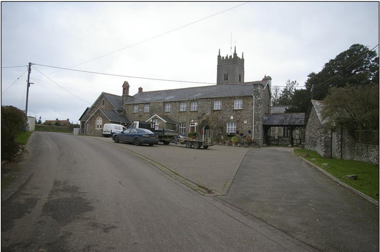
8. VIEW OF ST JAMES'S CHURCH; VIEWED FROM THE SOUTH-SOUTH-EAST (NO SCALE).
