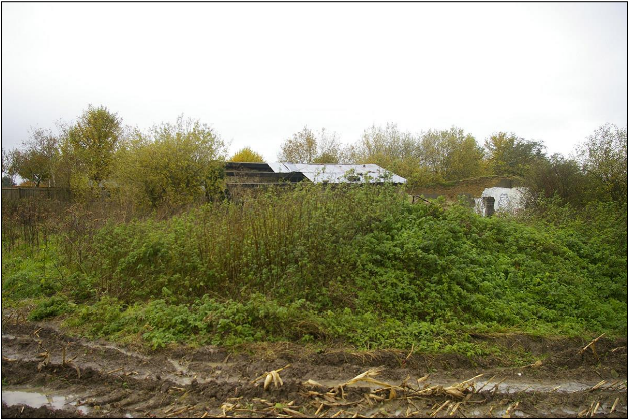
23. VIEW OF THE RUINED FARMHOUSE FROM FIELD J; VIEWED FROM THE EAST.
