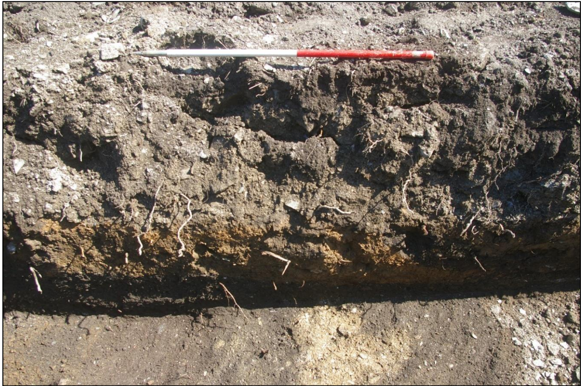
9. TRENCH 02, REPRESENTATIVE SOUTH-WEST FACING SECTION, SOUTH END; VIEWED FROM THE SOUTH-WEST (1M SCALE).
