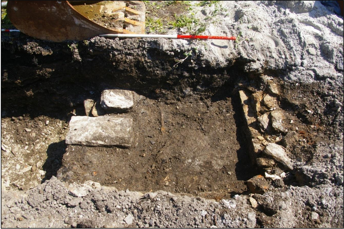
15. WALLS {307}, {308} AND {309}; VIEWED FROM THE NORTH-WEST (1M SCALE).
