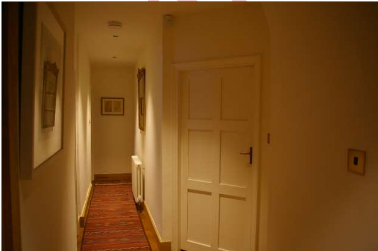
80. THE EAST END OF THE CORRIDOR, ROOM 12B, WHERE IT STEPS IN, IN WIDTH, OVER THE SERVICES, WITH FORMERLY SMALLER BEDROOMS; FROM THE WEST.
