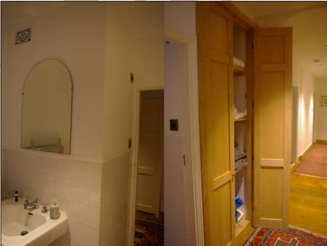
70. LEFT: THE BOXED IN AND TILED AIRING CUPBOARD, WITH GOOD STYLISED AIR VENT, IN THE BATHROOM, ROOM 19; FROM THE NORTH-WEST.
