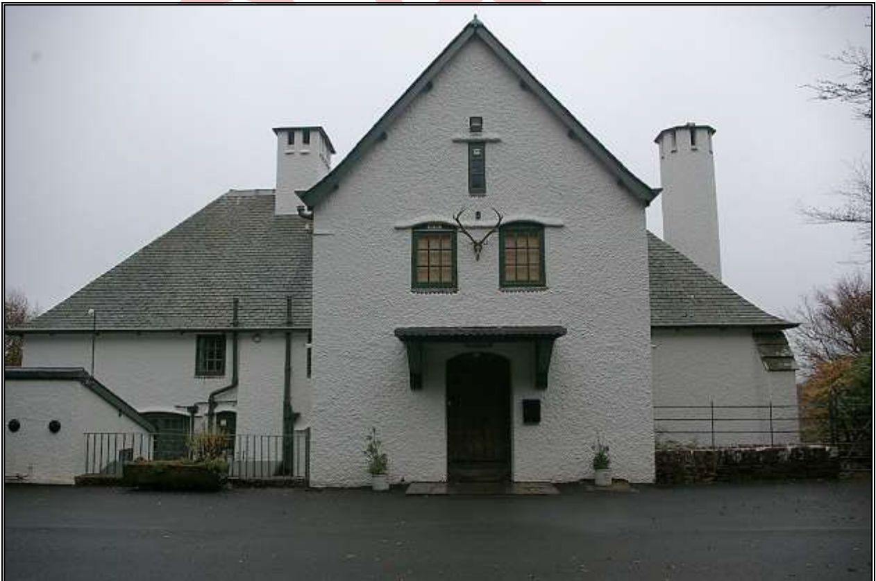
2. THE NORTH GABLED ENTRANCE WING TO LILLYCOMBE HOUSE; FROM THE NORTH.
