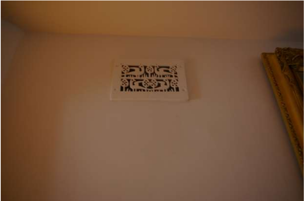
38. THE STYLISED AND VERY FINE 'ARTS & CRAFTS' AIR VENT IN THE STACK SERVING THE FIREPLACE IN AREA 5B, POTENTIALLY SHOWING 'PARTRIDGE IN A PEAR TREE' OR OTHER GAME BIRDS; FROM THE SOUTH-EAST.
