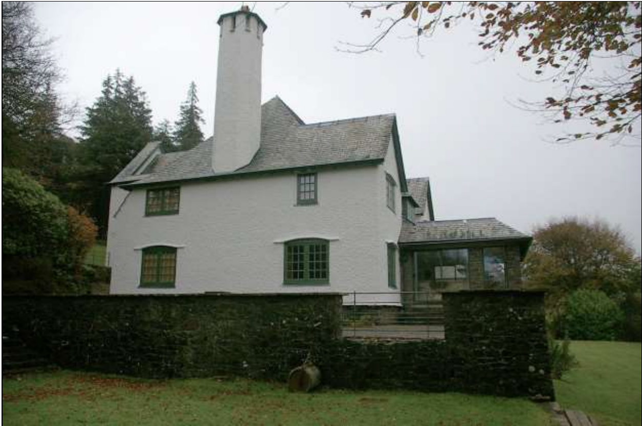
10. THE STONE-WALLED TERRACE WHICH WRAPS AROUND THE HOUSE AND SUNROOM BUILT OVER IT; FROM THE WEST-SOUTH-WEST.
