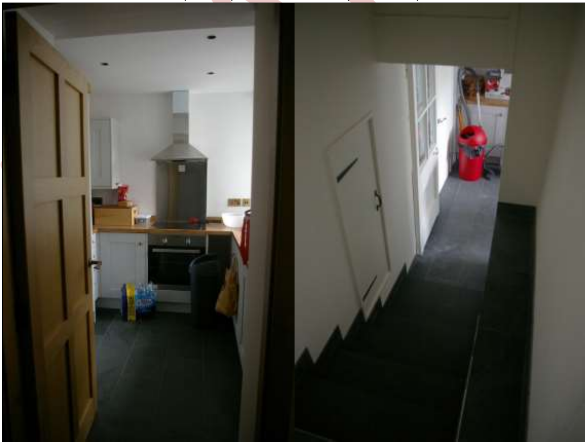
49. LEFT: THE UTILITY ROOM, ROOM 10; FROM THE SOUTH.
