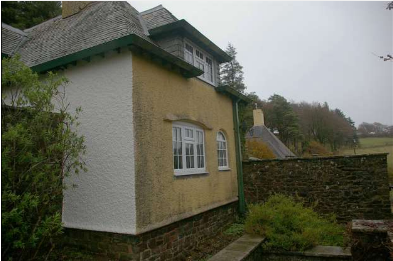
26. THE SOUTH GARDEN FRONT OF THE STABLES COTTAGE; FROM THE SOUTH-WEST.
