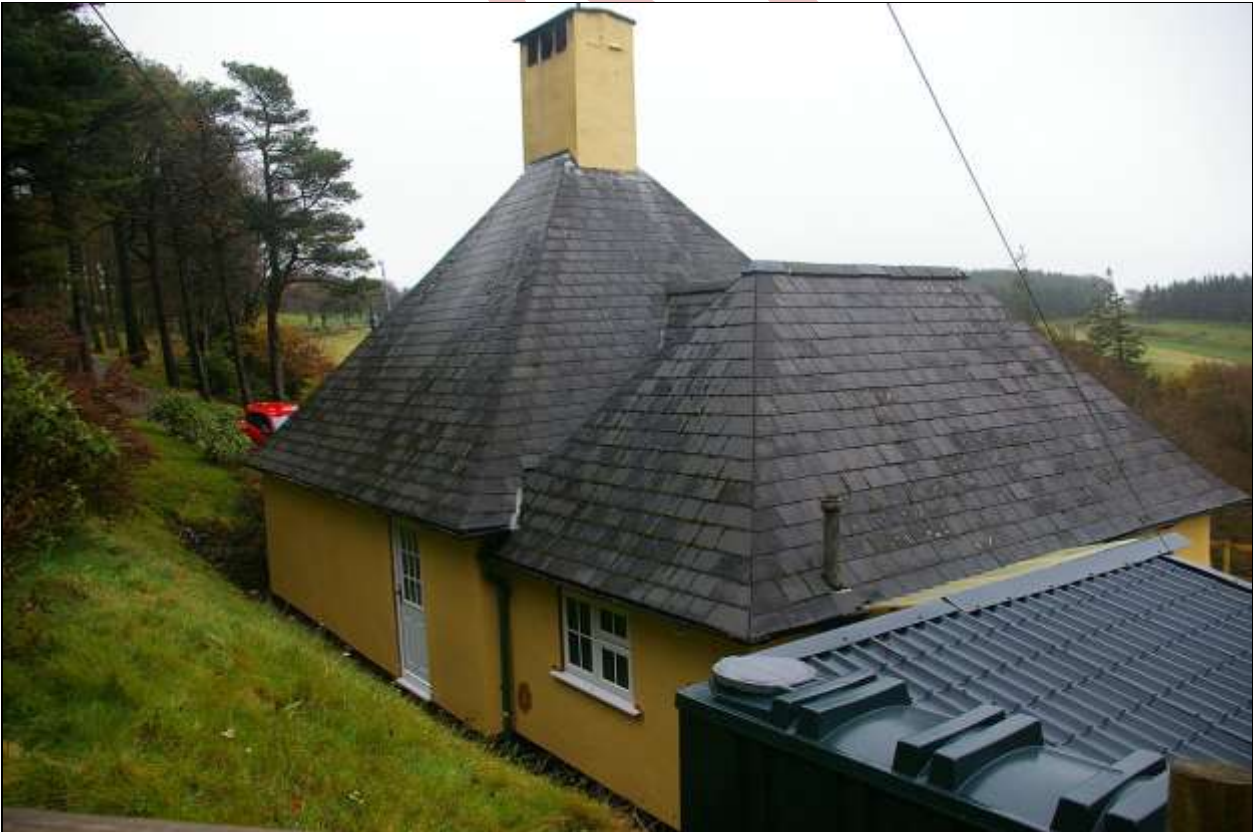
15. LILLYCOMBE BUNGALOW; FROM THE NORTH-WEST.
