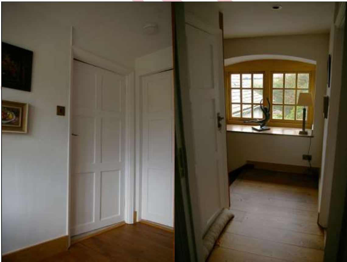
86. LEFT: THE SECOND FLOOR LANDING, DOORS TO ROOMS 25 AND 26; FROM THE NORTH-WEST.
