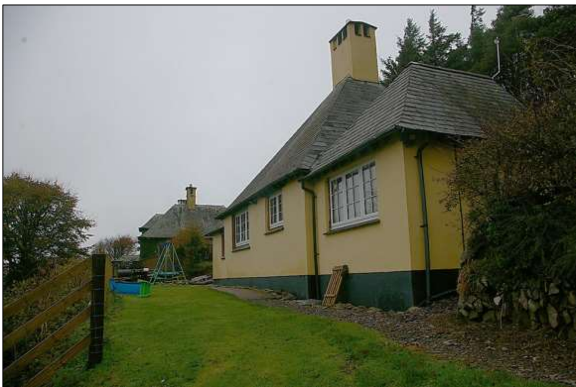
FIGURE 12: BUILDING 3; LILLYCOMBE BUNGALOW, WITH ITS ADDED FLANKING PAVILIONS AND STEEPLY PITCHED ROOF AND INSERTED STACK; FROM THE EAST-SOUTH-EAST.
