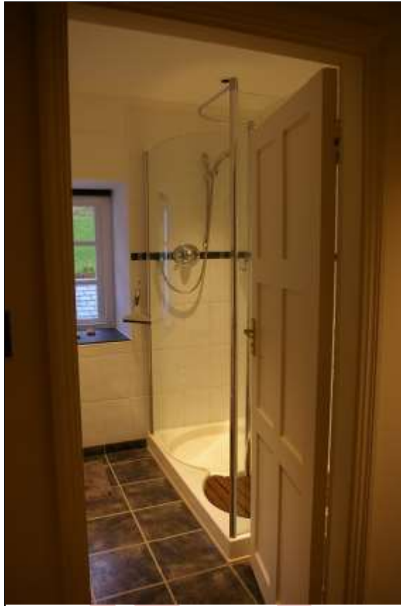
81. ROOM 21; ANOTHER SHOWER ROOM, POSSIBLY FORMERLY A DRESSING ROOM OR SERVANTS BEDROOM; FROM THE NORTH-WEST.
