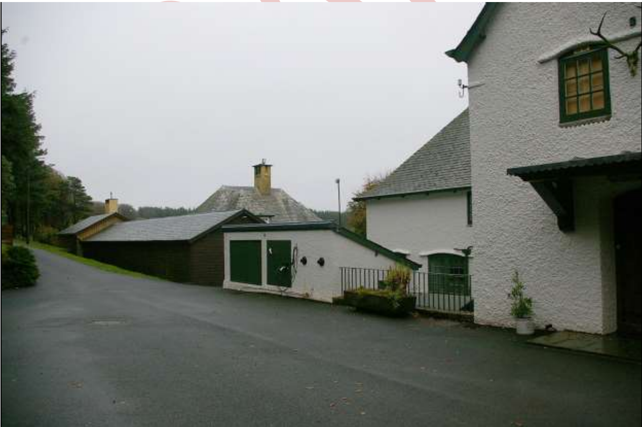
19. THE BUNGALOW AND STABLES COTTAGE, WITHIN A SERIES OF YARDS, EAST OF LILLYCOMBE HOUSE; FROM THE NORTH-EAST.
