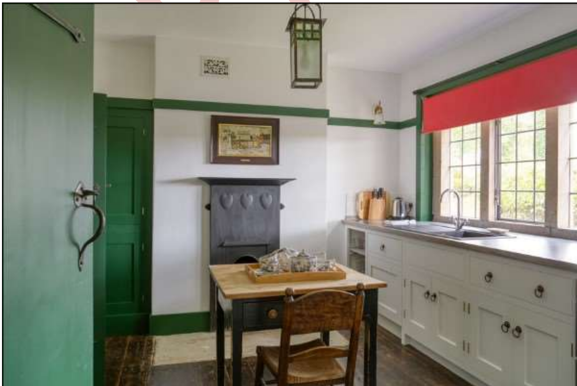
FIGURE 20: THE KITCHEN AT WINSFORD COTTAGE HOSPITAL, WITH AIR VENT TO STACK AND LEADED SMALL PANE CASEMENTS.
