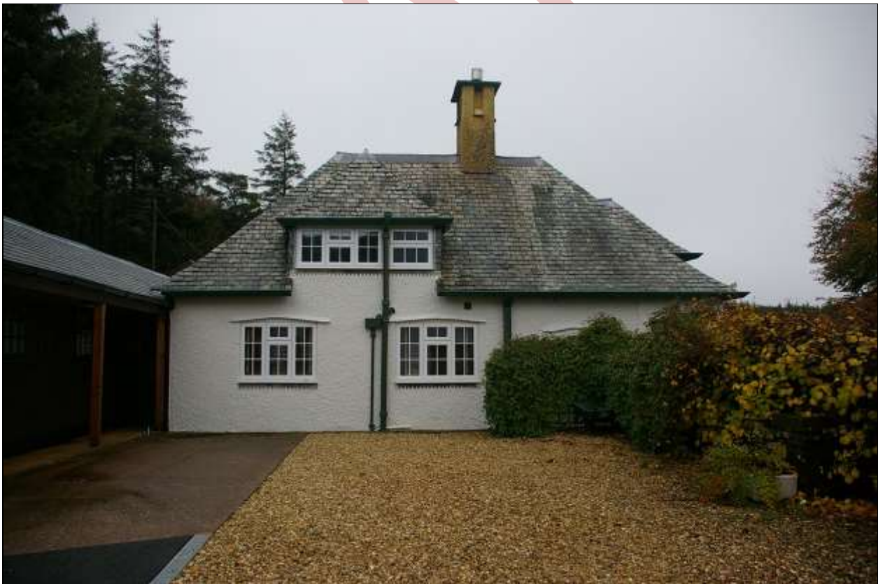
23. THE WEST ELEVATION OF THE STABLES COTTAGE, FACING ACROSS TO THE HOUSE; FROM THE WEST.
