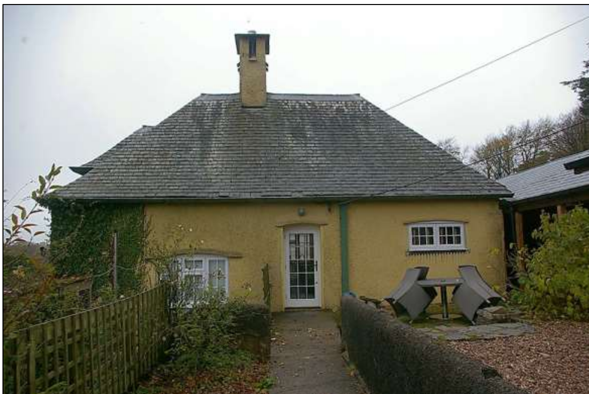
FIGURE 11: BUILDING 2; LILLYCOMBE STABLES COTTAGE WITH ITS OFF-CENTRE STACK AND DISTINCTIVE STEEP PITCHED ROOF; FROM THE EAST.
