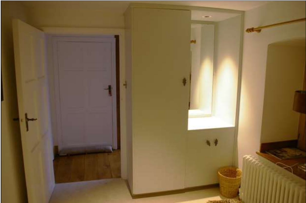
90. ROOM 25; FROM THE NORTH.
