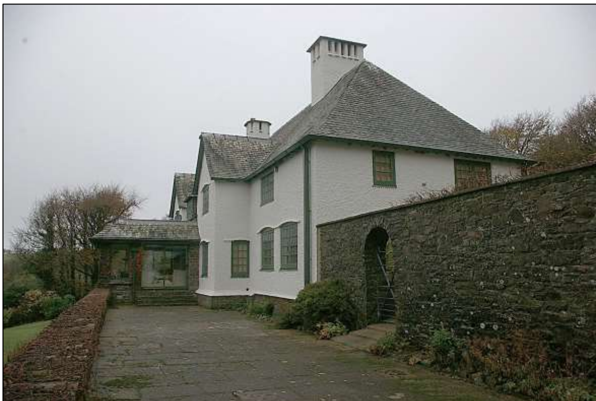
FIGURE 10: THE GARDEN FRONT OF LILLYCOMBE HOUSE, WITH INTEGRAL WALL AND TERRACE, WITH 1950S SUNROOM; FROM THE EAST.
