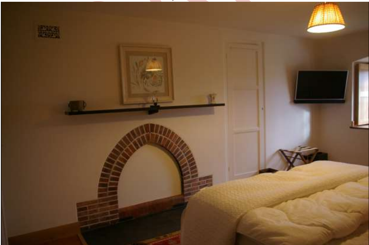
73. THE GOOD FIREPLACE IN ROOM 20, WITH SLATE MANTLE SHELF, ALSO WITH AIR VENT TO STACK; FROM THE NORTH-WEST.
