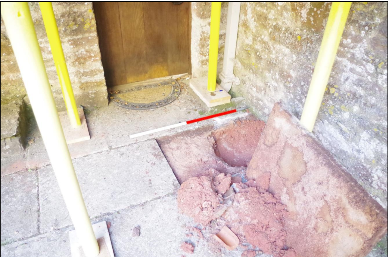
FIGURE 3: CONDUCTOR PIT 8; VIEWED FROM THE WEST (1M SCALE).
