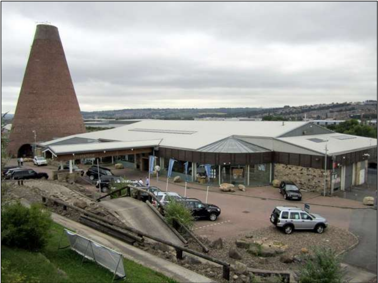
FIGURE 4: SHOT SHOWING THE PROXIMITY OF MODERN COMMERCIAL AND INDUSTRIAL UNITS TO THE REMAINING GLASSWORKS CONE, c.2010; ANDREW CURTIS.
