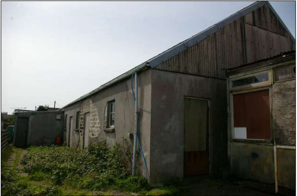
THE BARN, BUILDING F, THE NORTH AND EAST WALL, SHOWING IT IS MADE OF CONCRETE BLOCKS; FROM THE NORTH-EAST.
