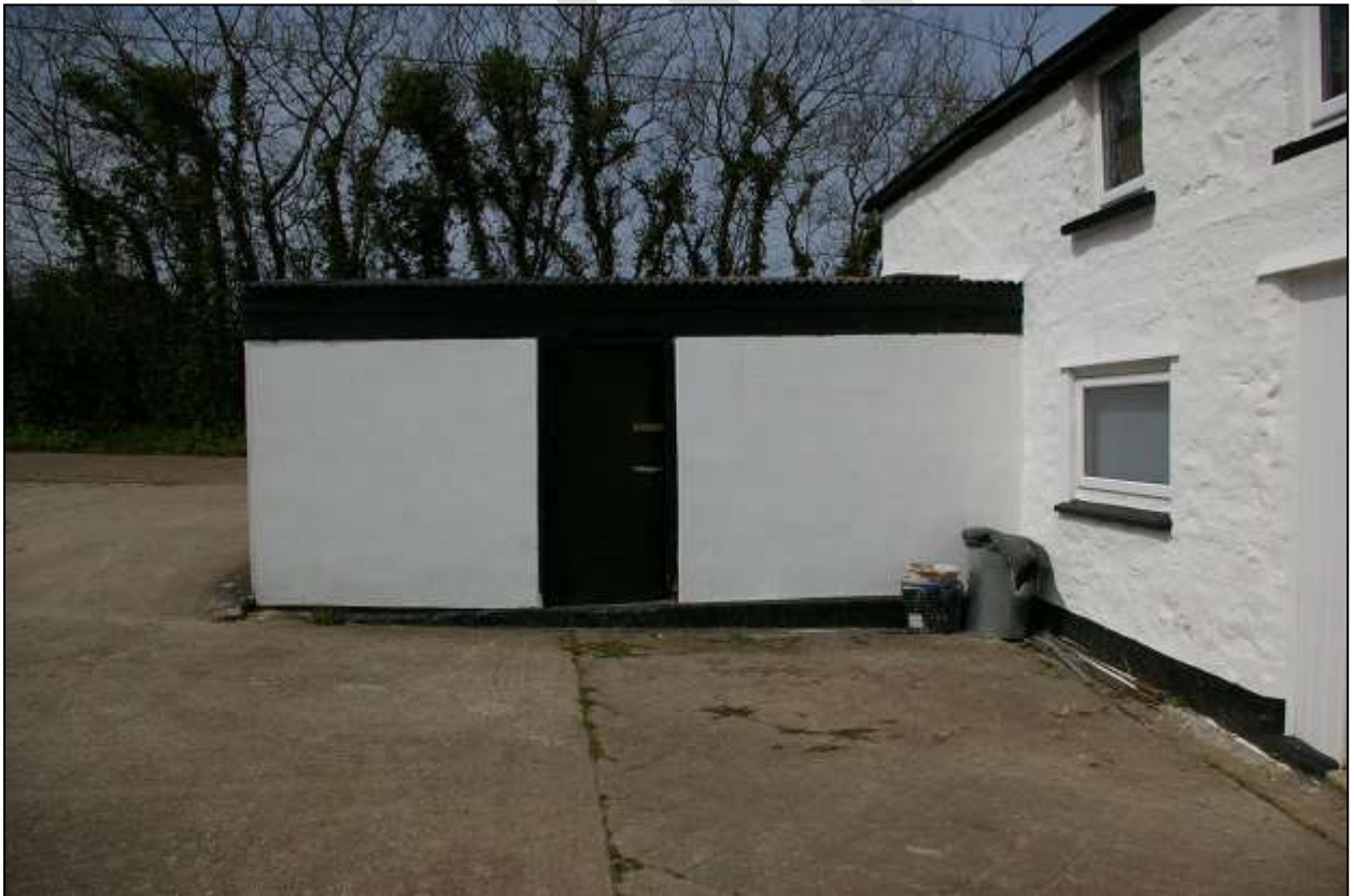
THE FLAT ROOFED SHED ATTACHED TO BUILDING D; FROM THE EAST.
