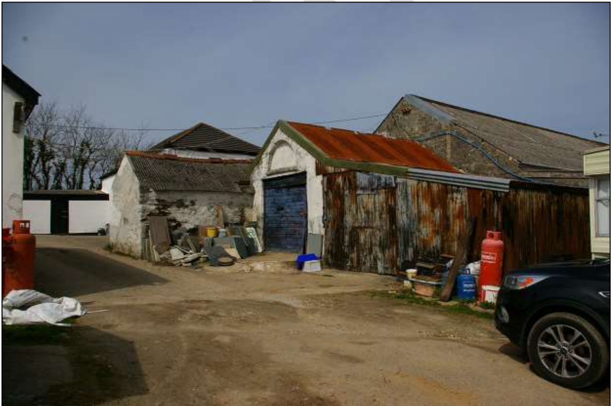
THE SECOND GARAGE BUILDING G; FROM THE SOUTH-EAST.
