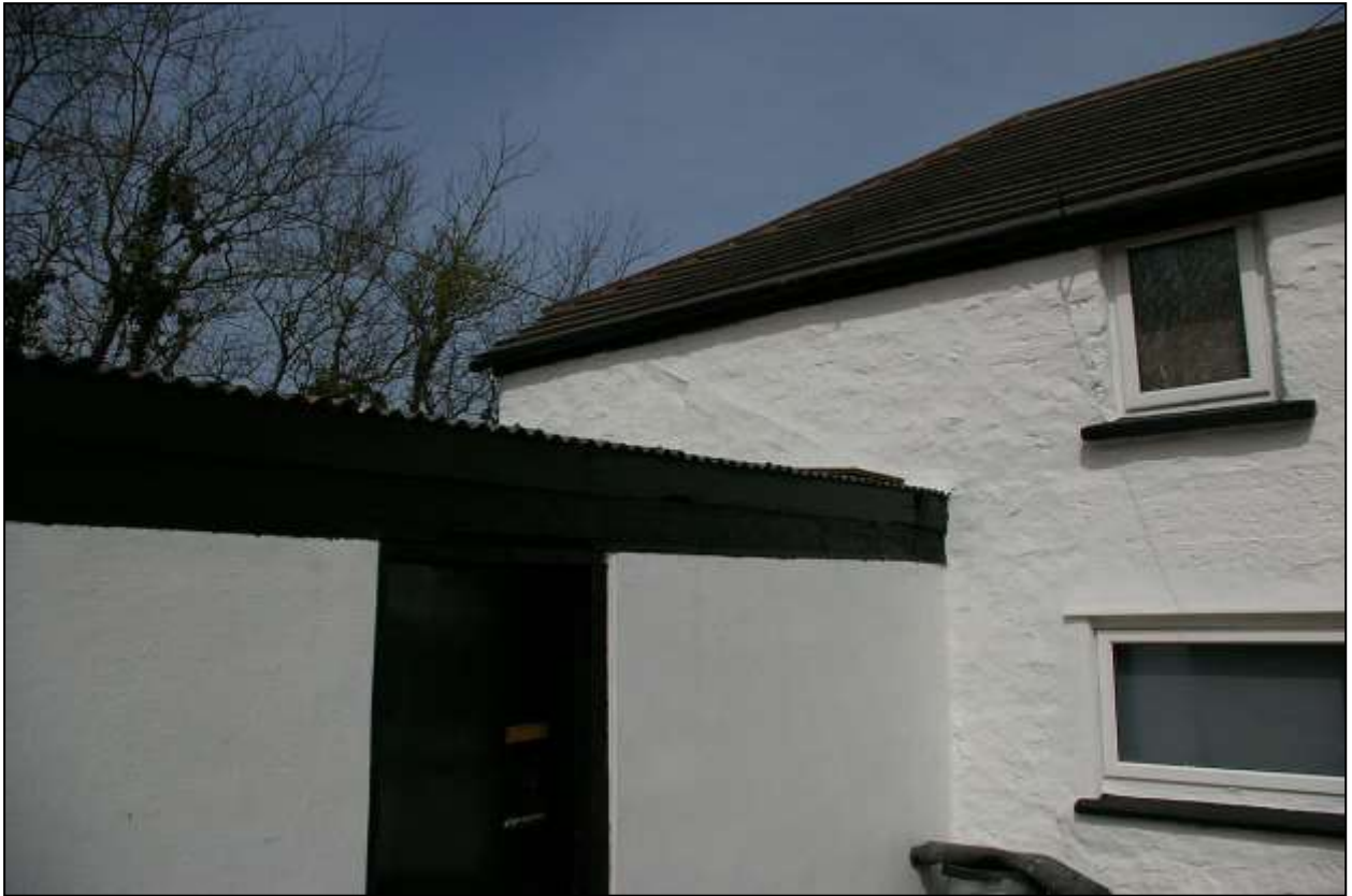
THE ROOFLINE SCAR AT THE WEST END OF BUILDING D; FROM THE SOUTH-EAST.
