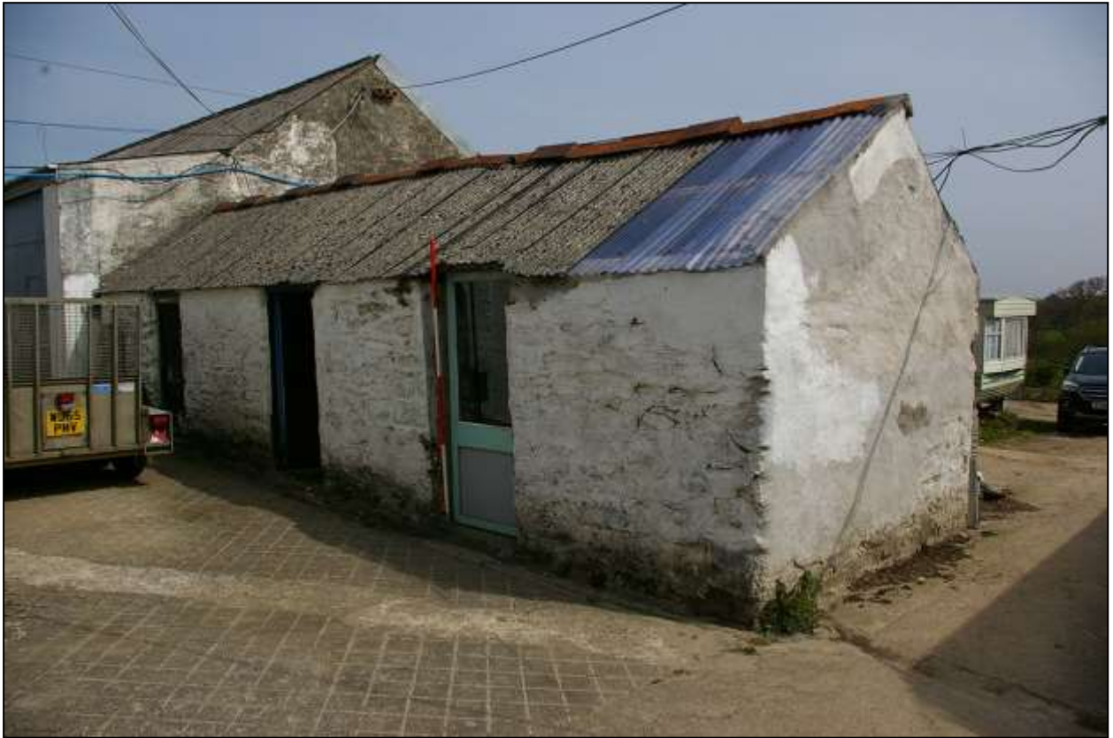
BUILDING E, WITH 2M SCALE; FROM THE SOUTH-WEST.
