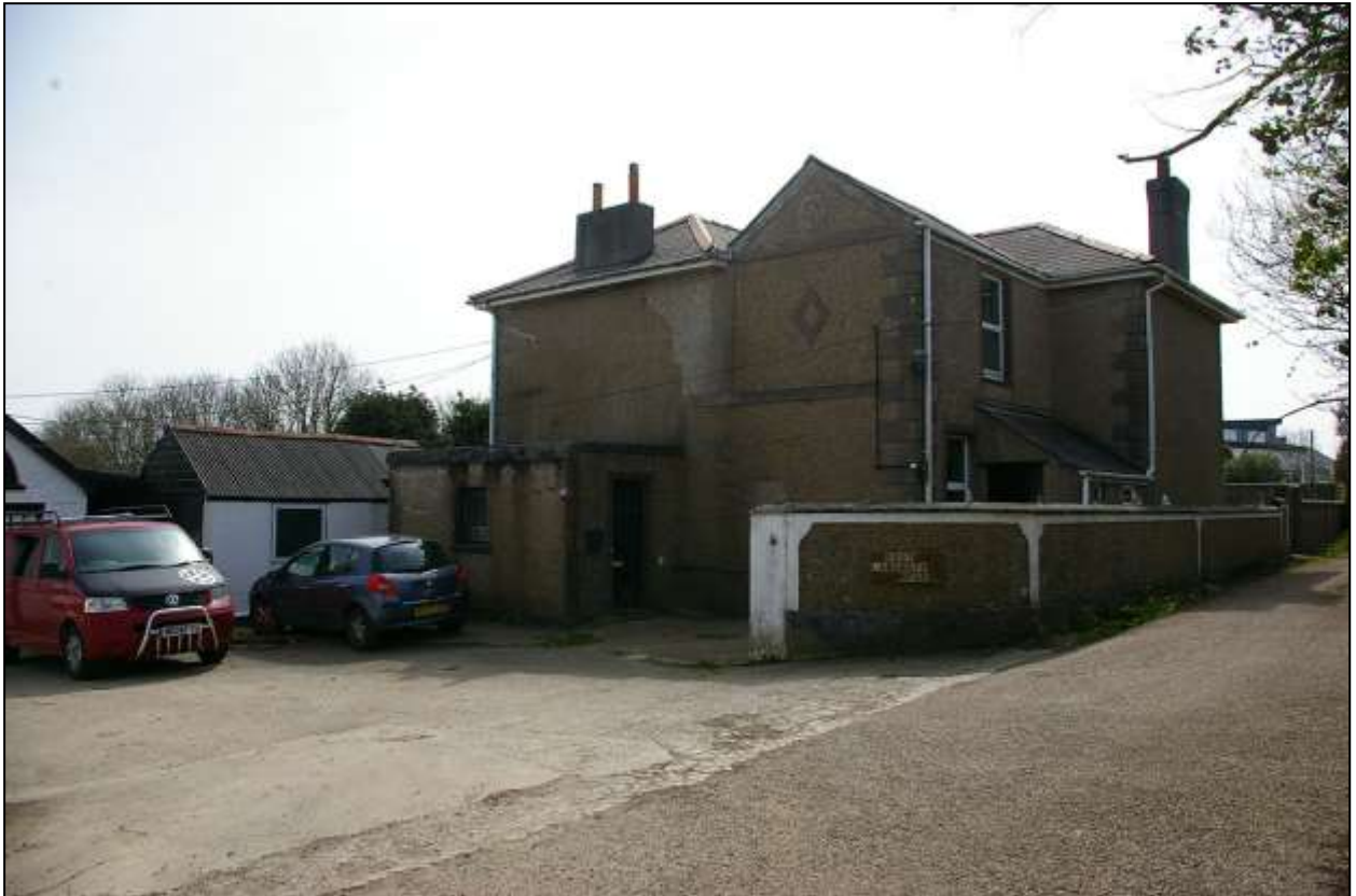
VIEW OF THE NORTH AND WEST ELEVATION OF THE FARMHOUSE, SHOWING MAIN L-SHAPED RANGE AND SMALL INFILL EXTENSION ON THE NORTH-WEST CORNER; FROM THE NORTH-WEST.
