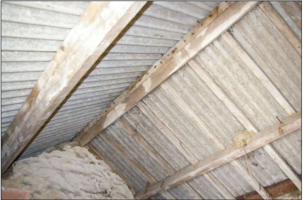
THE MODERN ROOF AND CORRUGATED SHEETING ON THE OLDER RUBBLE STONE WALLS; FROM THE SOUTH-WEST.
