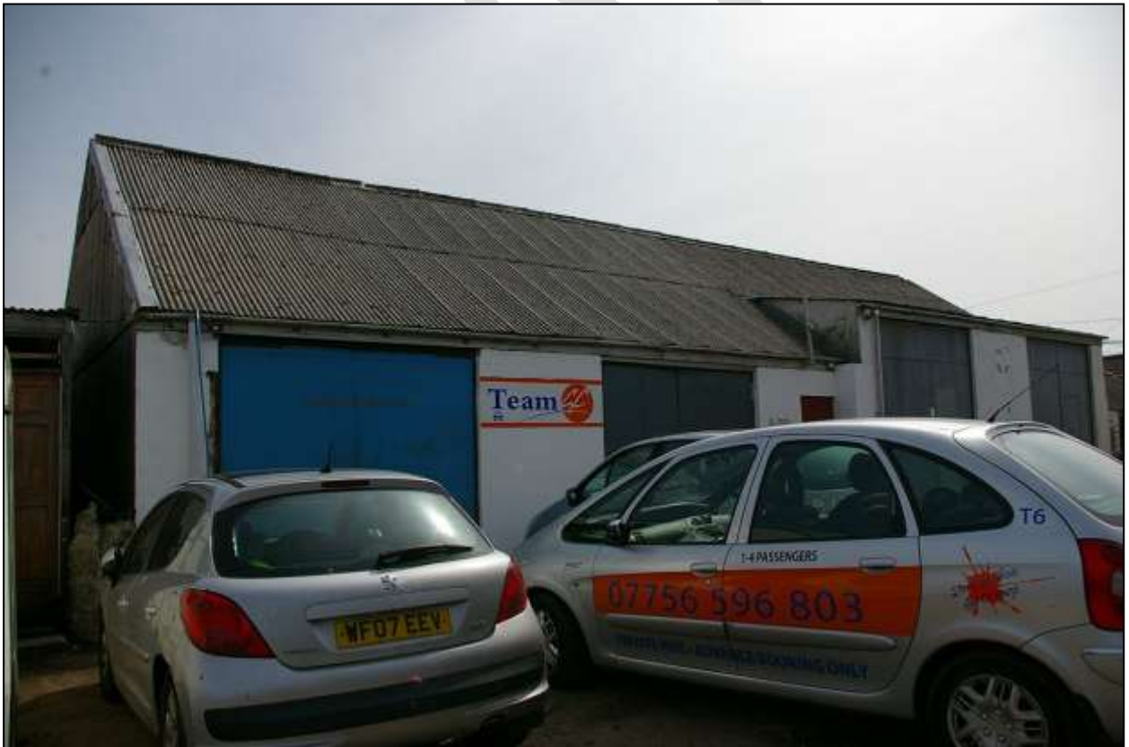
THE WEST WALL OF BUILDING F; FROM THE NORTH-WEST.
