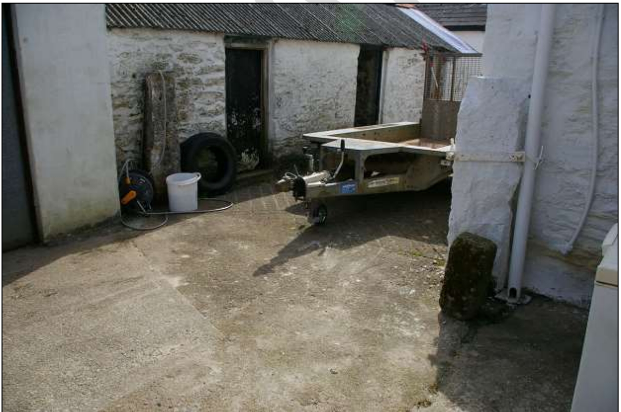
VIEW OF THE HISTORIC GRANITE GATE PIERS, BETWEEN BUILDINGS D AND E; FROM THE NORTH-WEST.
