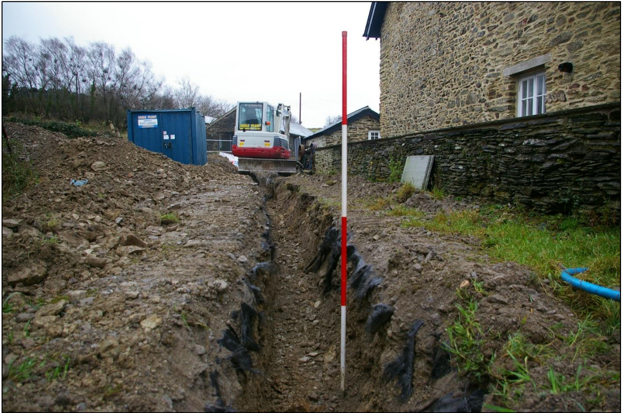
11. LOOKING DOWN TRENCH 1 FROM THE EAST. (2M SCALES).
