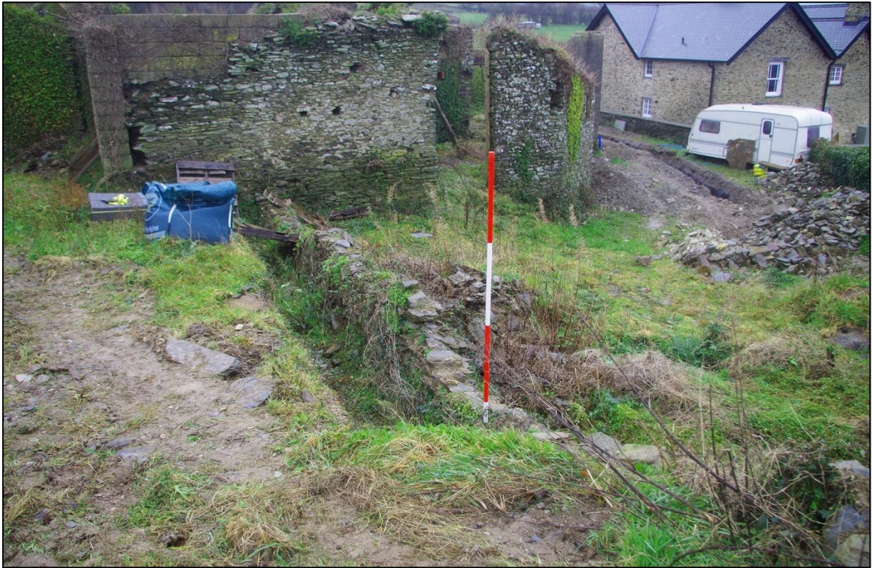
5. BUILDING 1; LOOKING DOWN ON TO THE FARM COMPLEX, WITH BUILDINGS B2A AND B3 VISIBLE. (WITH 2M SCALES). TAKEN FROM THE NORTH EAST.
