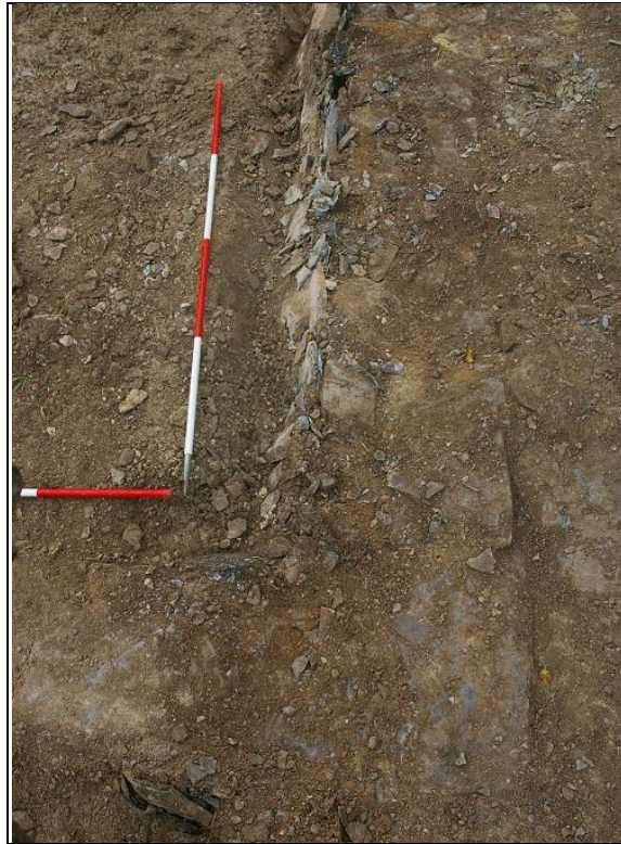
17. THE DRESSED QUOINS TO THE NORTH-EAST CORNER, WITH 2M X 1M SCALE, SHOWING THE CONTINUITY OF THE FOUNDATIONS; FROM THE EAST.
