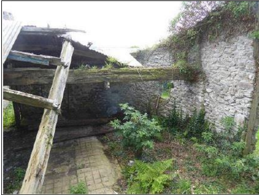
7. B3 PICTURED IN 2011 WITH TRUSSES. (SOURCE: NIMROD, 2017).
