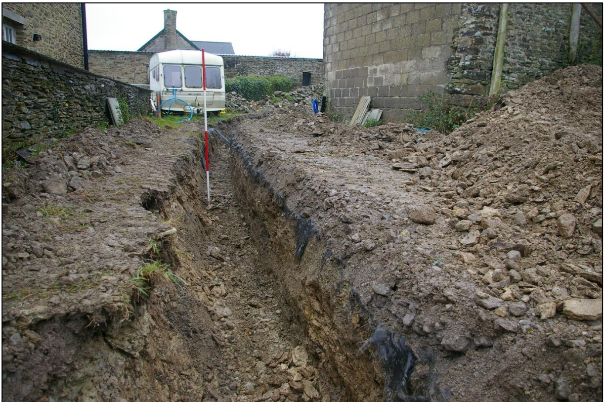
10. LOOKING DOWN TRENCH 1 FROM THE WEST. (2M SCALES).
