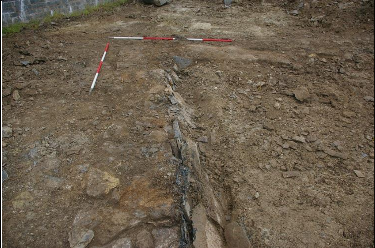
15. THE NORTH AND EAST WALLS OF B2A, DURING FLOOR CLEARANCE, EXHIBITING INTERNAL AND EXTERNAL DRAINS; FROM THE WEST (2X2M SCALES).
