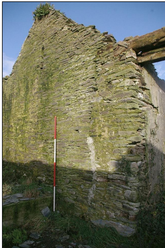
34. BUILDING 4 THE STABLES. (WITH 2M SCALES). FROM THE SOUTH WEST.
