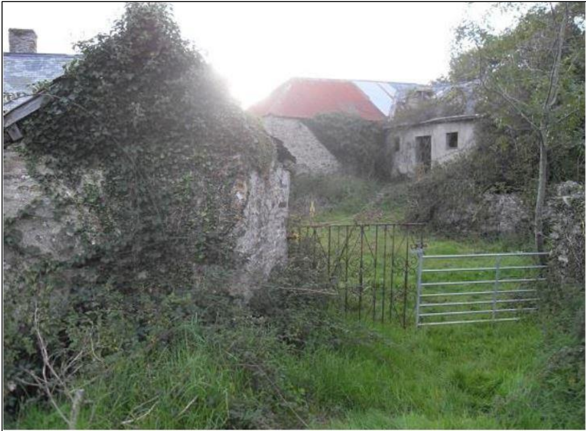
5. B2B AND STABLES. NOTE CORRUGATED ROOFING. PICTURED 2011. (SOURCE: NIMROD, 2017).
