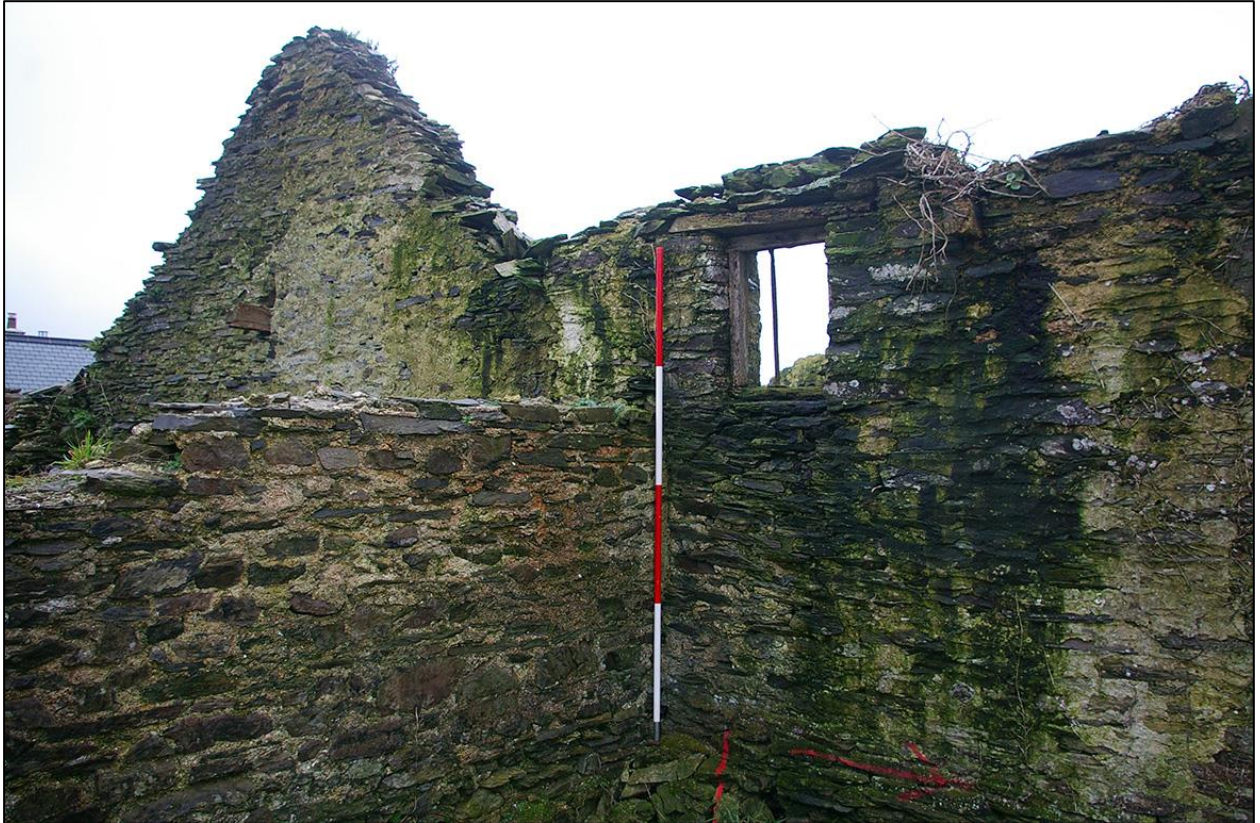
51. THE STABLES BUILDING 4 ABUTTING THE OLDER EASTERN BARN WALLS OF B2A; SHOWING THE EXTERIOR STONE PLINTH. (WITH 2M SCALES). TAKEN FROM THE NORTH.
