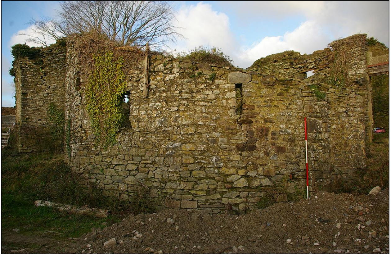
55. EXTERNAL WALL SECTION OF B3 SHOWING THE SMALL WINDOWS. (WITH 2M SCALES). TAKEN FROM THE SOUTH.
