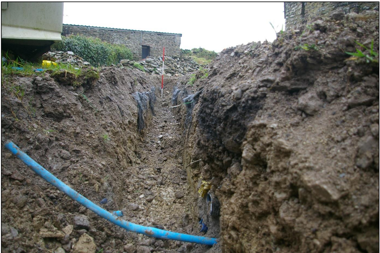
12. LOOKING DOWN TRENCH 1 FROM THE SOUTH EAST. (2M SCALES).
