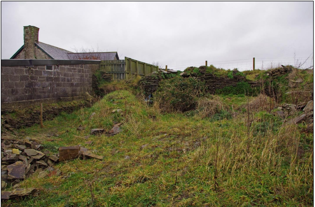
1. BUILDING 1; LOOKING TOWARDS THE EASTERN CORNER. (WITH 2M SCALES). TAKEN FROM THE EAST.
