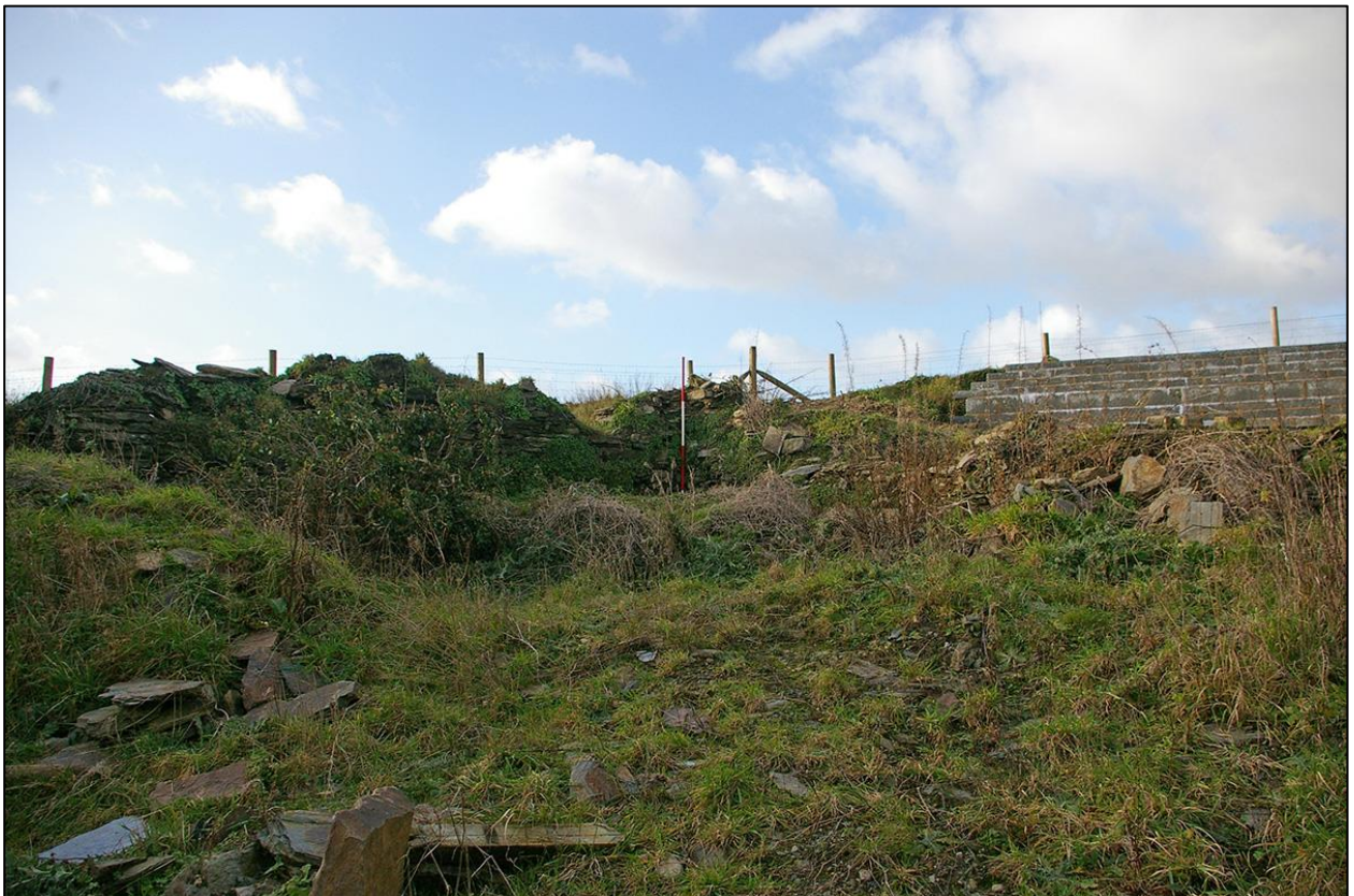
2. BUILDING 1 OUTER RUINOUS WALL. (WITH 2M SCALES) TAKEN FROM THE SOUTH EAST.
