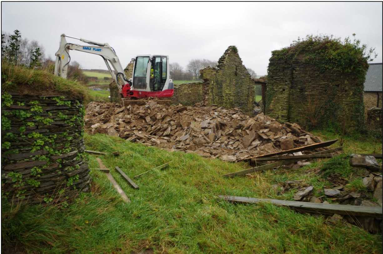
6. B2A DEMOLISHED. TAKEN FROM THE WEST.
