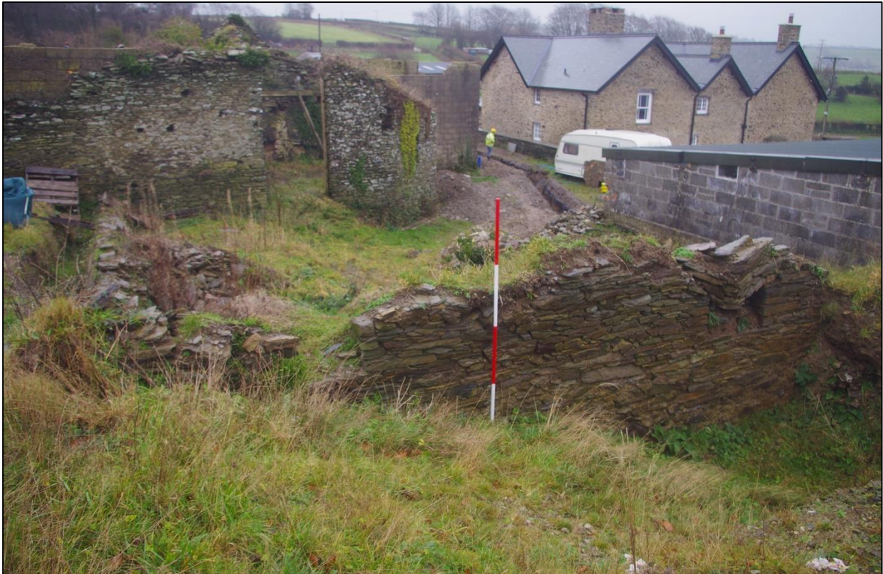
6. BUILDING 1; SOUTHERN CORNER, LOOKING DOWN ONTO B3 (WITH 2M SCALES). FROM THE NORTH WEST.
