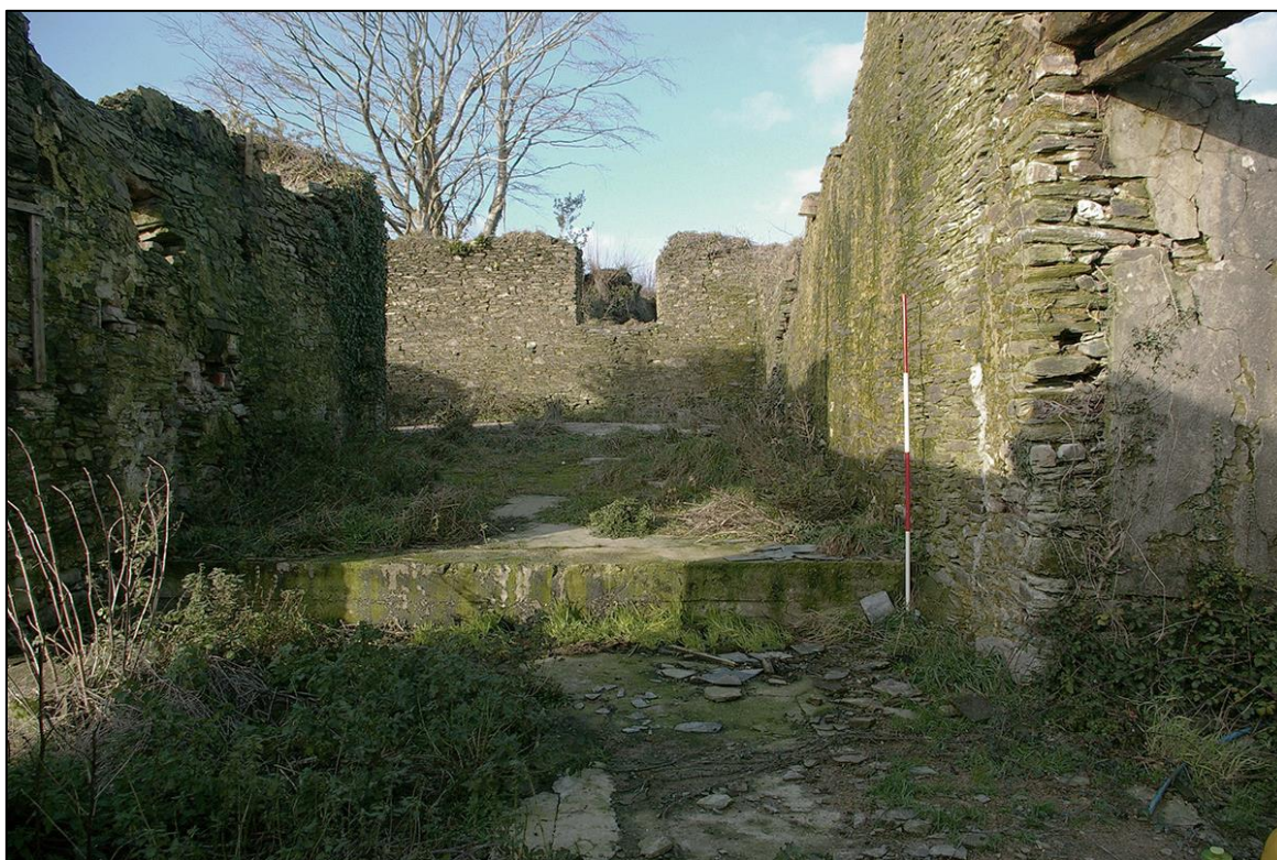
FIGURE 14: B2B INTERIOR, SHOWING HOW IT ADJOINS B2A, TO THE NORTH; FROM THE SOUTH (2M SCALE).
