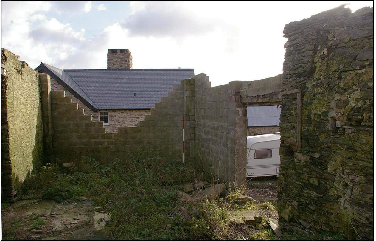
39. B2B SHOWING THE FORCED DOORWAY INTO B3. TAKEN FROM THE NORTH.
