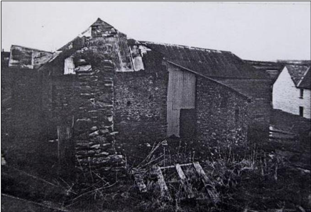
4. B3 AND B2A LOOKING DOWN TOWARD THE FARMHOUSE. PICTURED 1989. (SOURCE: NIMROD, 2017).
