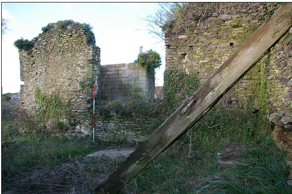
FIGURE 13: B2A, SOUTH WALL, SHOWING THRESHING DOOR; FROM THE SOUTH-EAST (2M SCALE).
