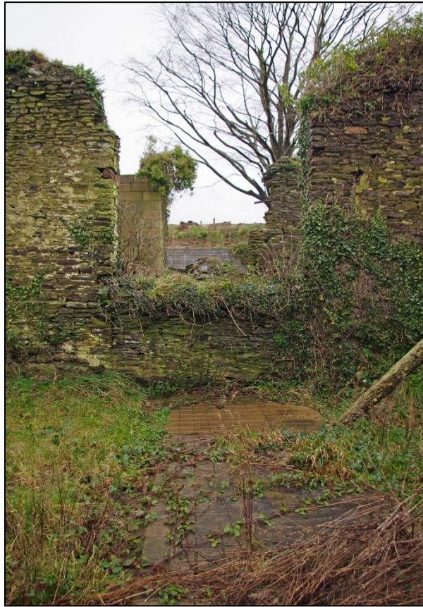
17. LOOKING INTO BUILDING 2A FROM B3. FROM THE SOUTH.
