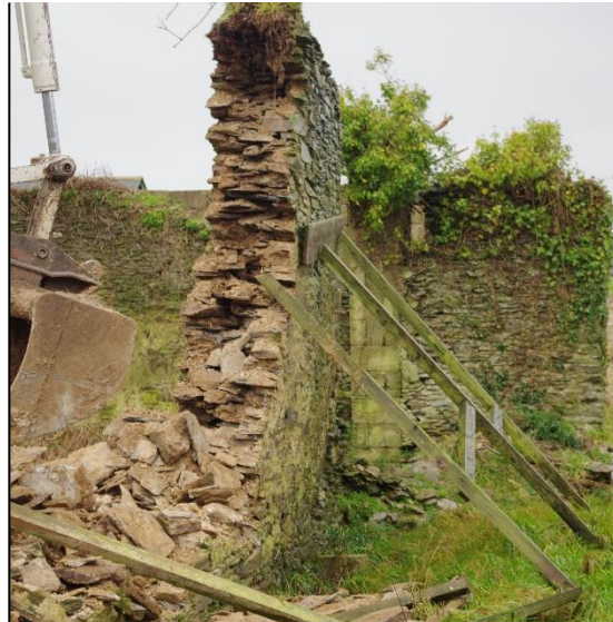
5. DEMOLITION OF THE NORTHERN WALL OF B2A.
