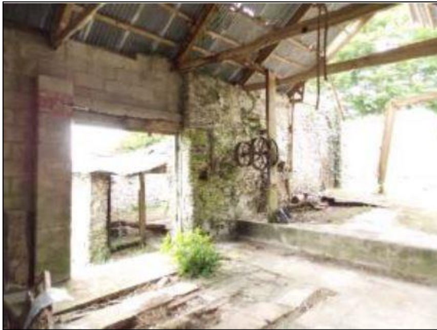
8. B2B LOOKING DOWN INTO B3. PICTURED 2011. (SOURCE: NIMROD, 2017).
