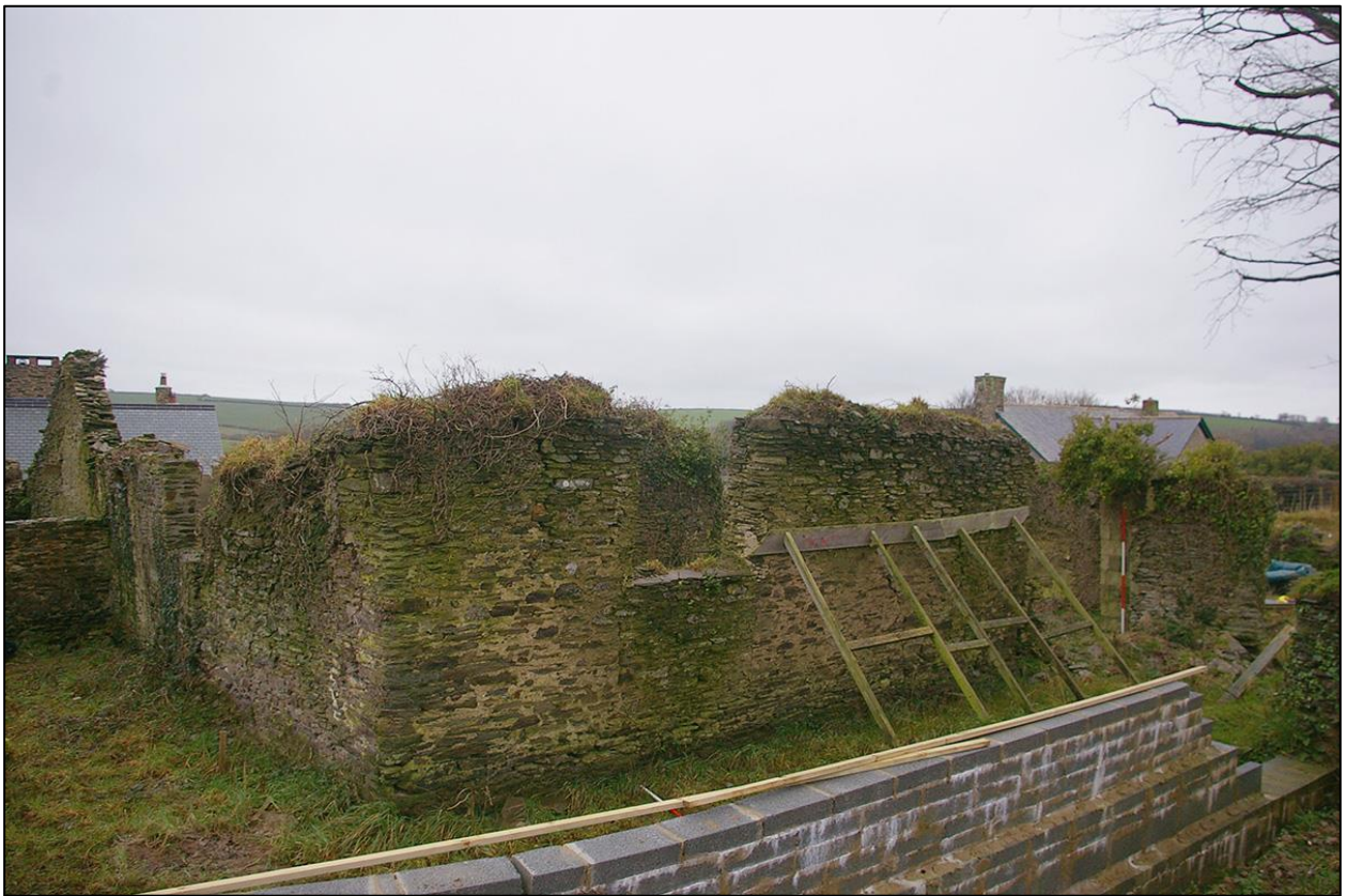
11. LOOKING SOUTH IN BUILDING 2A (WITH 2M SCALES). TAKEN FROM THE NORTH.
