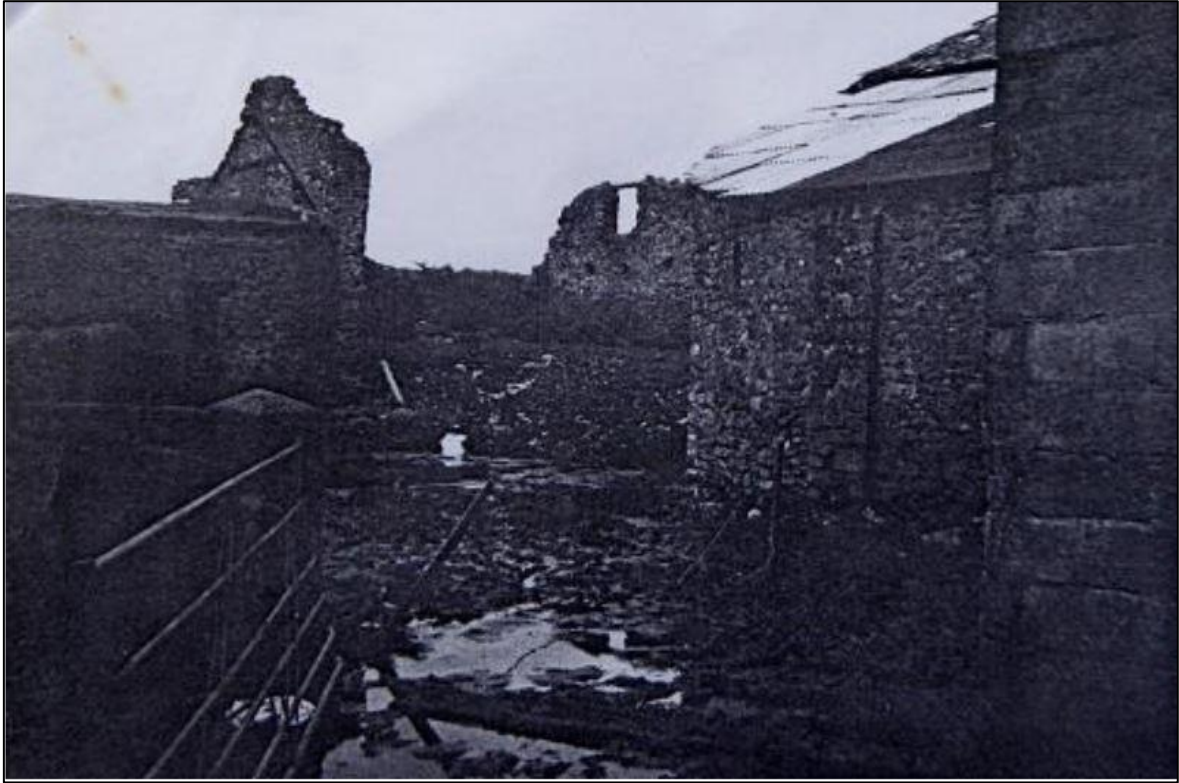
3. B1 AND B3 IN THE FORMER FARMYARD. PICTURED 1989. (SOURCE: NIMROD, 2017).
