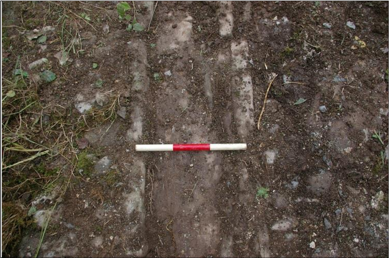
21. DETAIL OF THE SLATE SLAB DRAIN IN B4, WITH 0.3M SCALE; FROM ABOVE.
