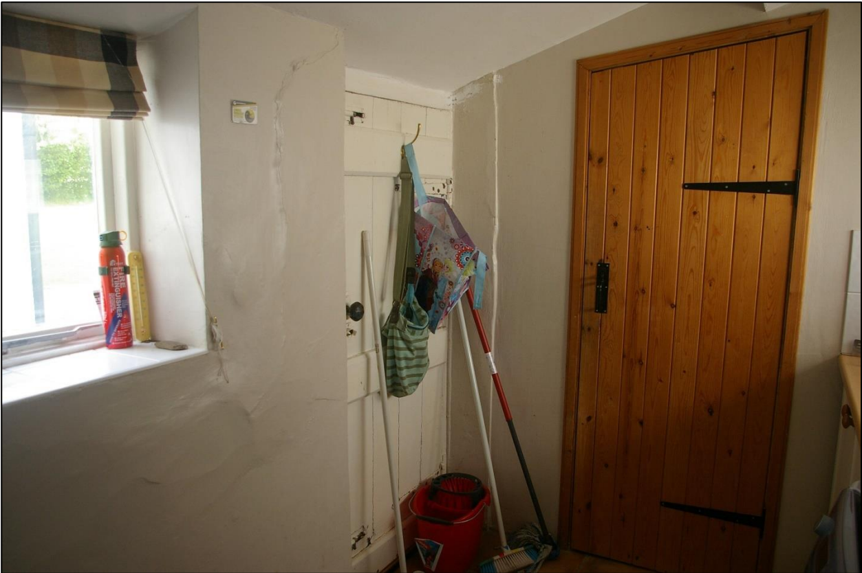
16. ROOM 6; SINGLE STOREY OUTBUILDING EXTENSION; FROM THE SOUTH-EAST.
