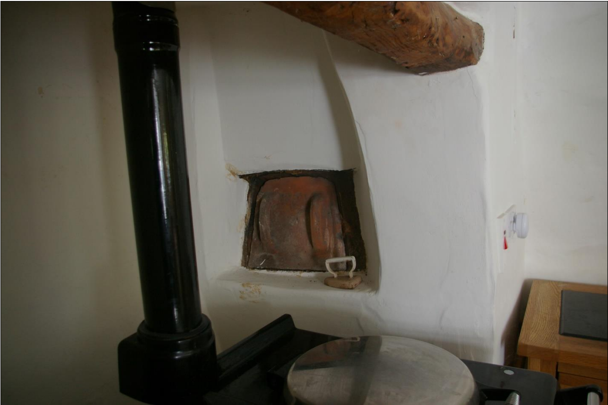
14. THE BREAD OVEN, WITH INFILLED PYRAMIDAL OPENING AND CLAY-CLOAM OVEN WITH CLAY DOOR, ROOM 5; FROM THE NORTH-WEST.
