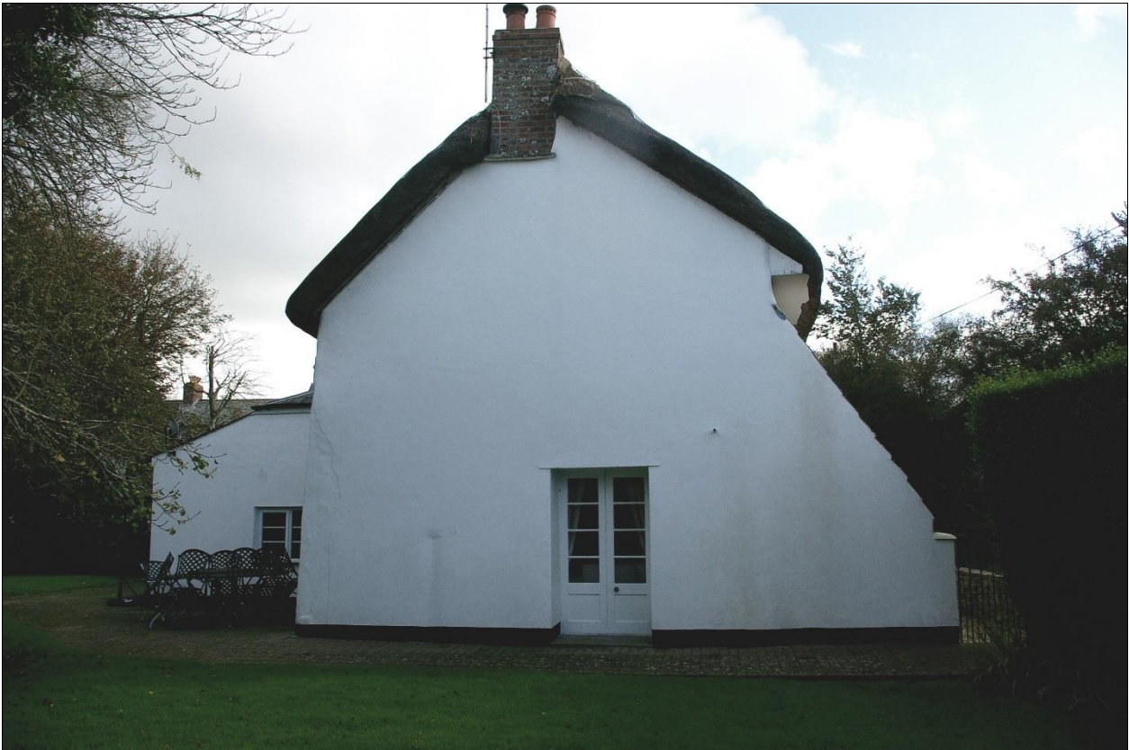
1. THE WEST GABLE, WITH 18 TH OR 19 TH CENTURY BRICK STACK AND MODERN FORCED FRENCH WINDOWS; FROM THE WEST.
