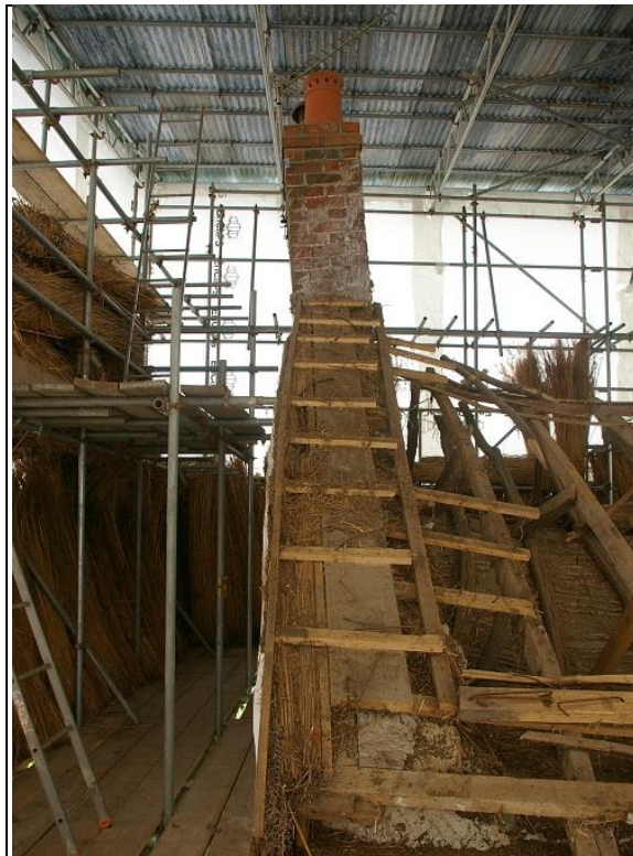
36. THE WESTERN CORNER GABLE STACK, SHOWING THE SHAFT REBUILT IN THE EARLY 20 TH CENTURY, C.1910-1920; FROM THE SOUTH.
