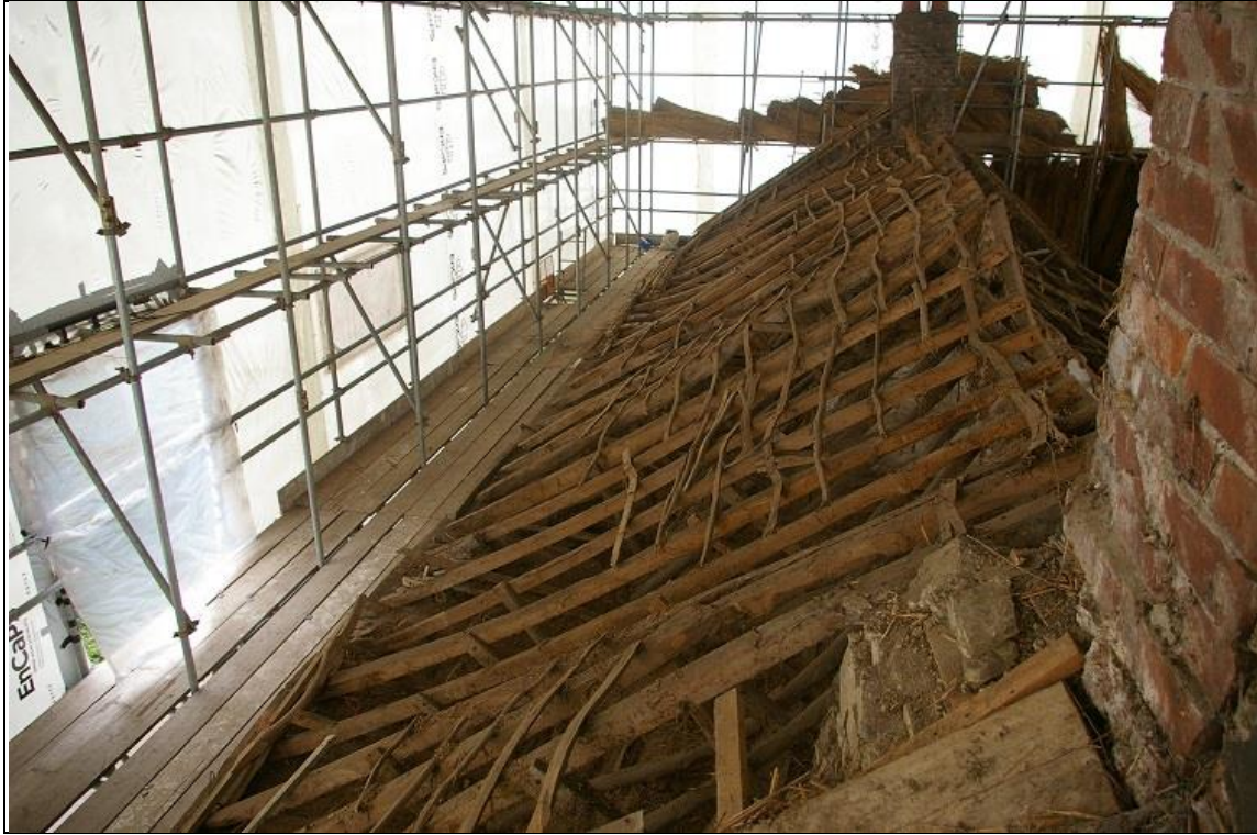
33. WESTACOMBE ROOF, STRIPPED OF THATCH, FROM THE EAST END, SOUTH SIDE.
