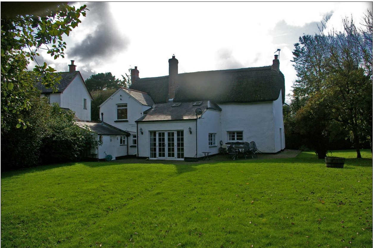
2. THE REAR OF THE COTTAGE, SHOWING THE SMALL GABLED KITCHEN EXTENSION, LONG OUTBUILDING AND LARGE MODERN EXTENSION TO THE WEST; FROM THE NORTH-WEST.
