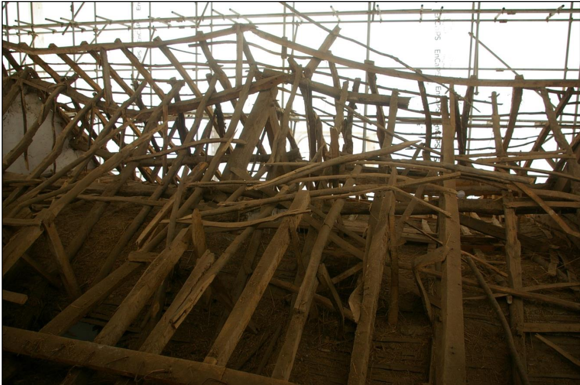
48. TRUSS 2 FROM THE NORTH SIDE OF THE ROOF; FORM THE NORTH-WEST.
