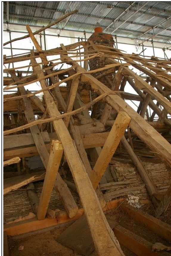
49. TRUSS 2, FROM THE SOUTH SIDE OF THE ROOF; FROM THE SOUTH-WEST.
