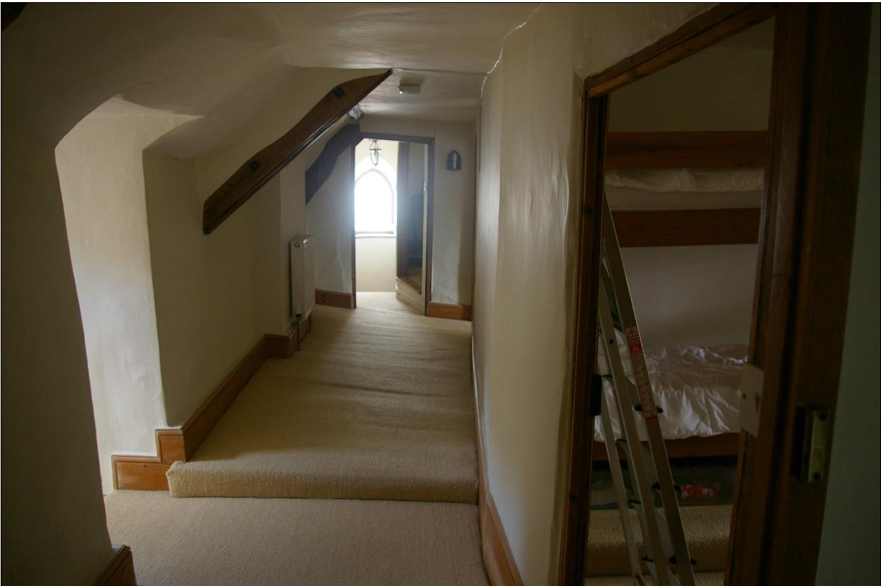
22. ROOM 11, THE CORRIDOR, SHOWING FLOOR LEVEL RAISE OVER FORMER HALL AND ANGLE CHANGE TO INSERTED PARTITIONS; FROM THE WEST.
