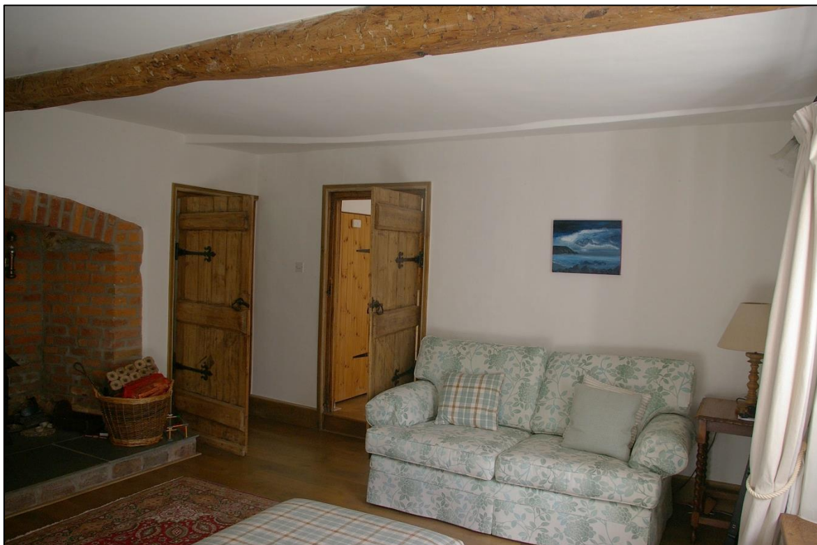
FIGURE 7: THE FORMER HALL, ROOM 3, WITH PLASTERED OVER POTENTIAL JETTY TO THE EAST; FROM THE SOUTH-WEST.
