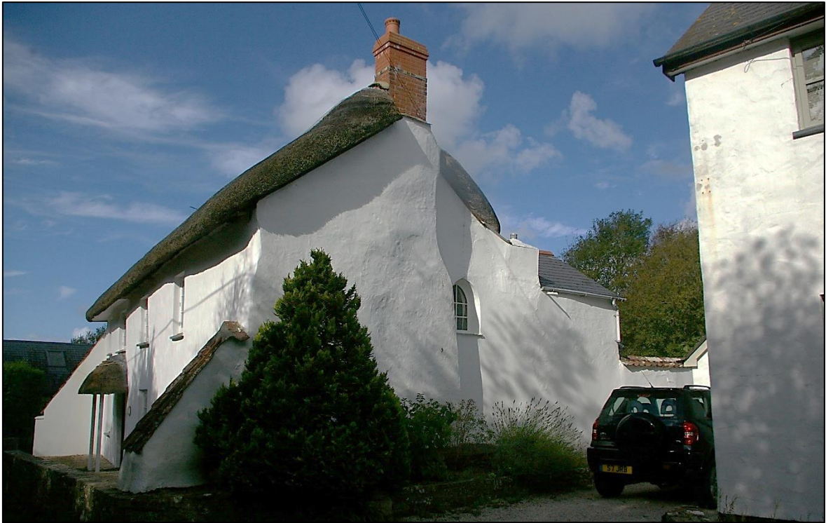
FIGURE 5: THE EAST GABLE OF WESTACOMBE COTTAGE; FROM THE EAST-SOUTH-EAST.
