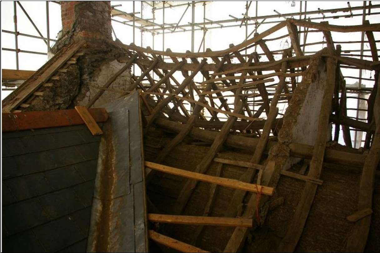
54. BAY 4 OF THE ROOF; FROM THE NORTH SIDE; FROM THE NORTH-WEST.
