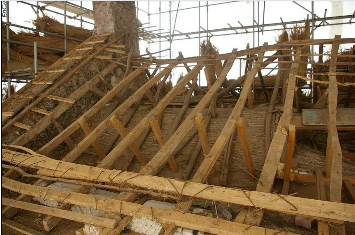
41. BAY 1 OF THE ROOF (FROM THE WEST END); FROM THE SOUTH-EAST.
