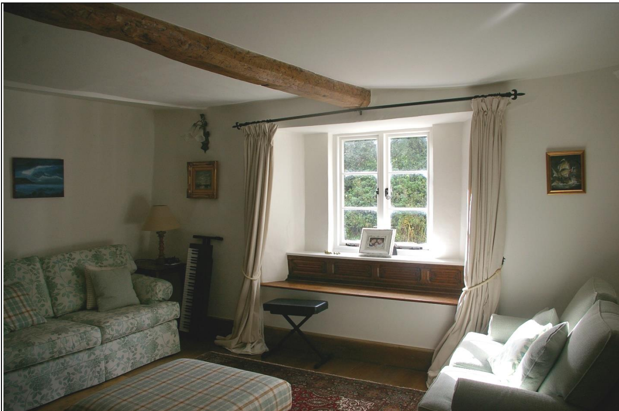
7. THE WINDOW IN ROOM 3, WITH LINEN FOLD PANNELLING RESET FORMING A WINDOW SEAT; FROM THE NORTH-WEST.
