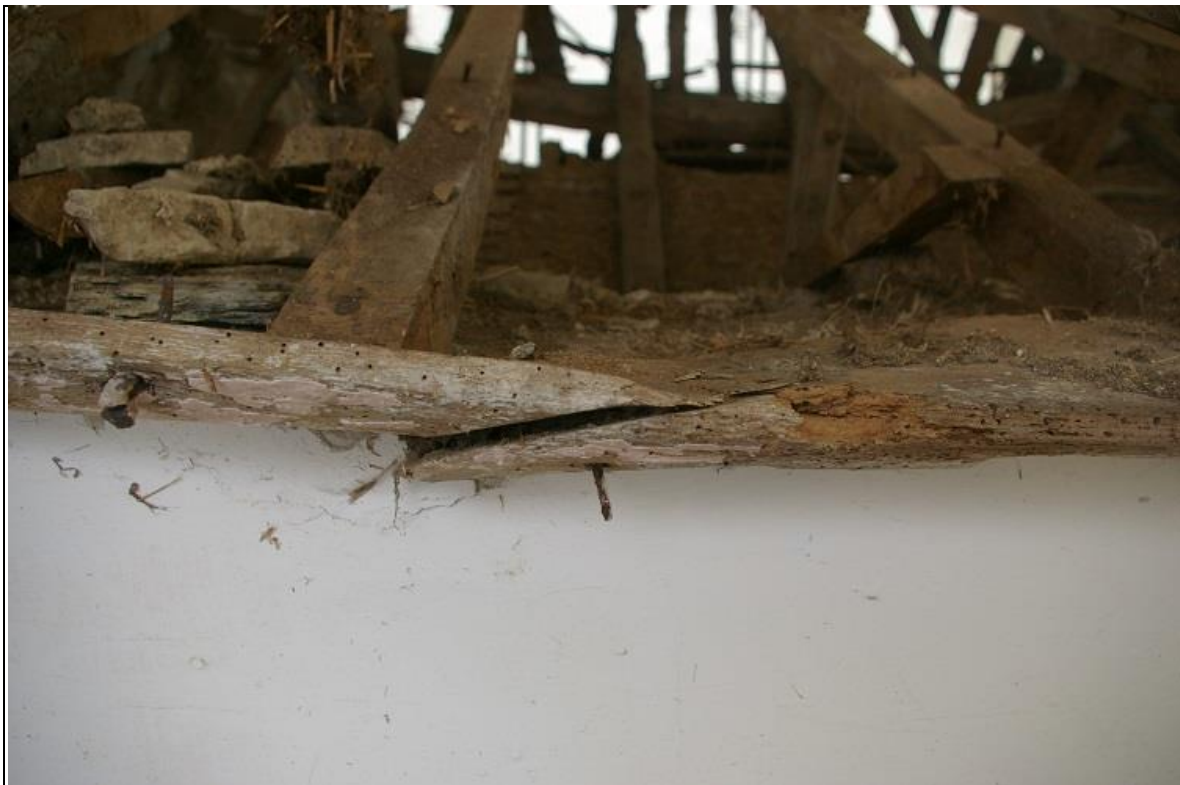
38. THE WALL-PLATE WHICH WAS REFITTED TO THE SOUTH SIDE OF THE HOUSE AFTER THE COTTAGE WAS RE-FRONTED WAS RE-ATTACHED USING CLENCH NAILS IN THE PEG HOLES; FORM THE SOUTH.
