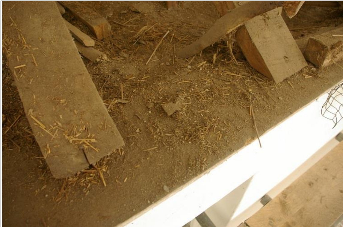
37. THE LATER 18 TH OR 19 TH CENTURY ROOF EXTENSION WHICH RESPECTS THE RE-FRONTING OF THE COTTAGE ARE SPIKED TO THE EARLIER CARVED WALL-PLATE/EAVES BOARD, WHICH HAS BEEN RE-SITED, PEGGED TO THE COB WITH LARGE SQUARE WOODEN PEGS; FROM THE SOUTH-WEST, SOUTH SIDE OF THE HOUSE.
