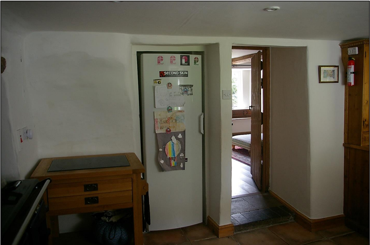
12. THE PAIRED DOORWAYS TO THE MAIN RANGE FORM ROOM 5, THE KITCHEN BLOCK, ONE ORIGINAL DOORWAY, NOW BLOCKED, ONE MORE MODERN FORCED DOORWAY; FROM THE NORTH-NORTH-EAST.
