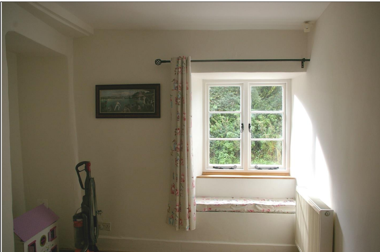
9. ROOM 4, WITH WINDOW WITH SLATE SHELF BELOW AS WINDOW SEAT AND LARGE FORCED/BLOCKED DOORWAY TO THE SOUTH-EAST CORNER; FROM THE NORTH-WEST.
