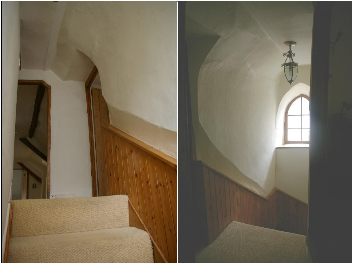
17. LEFT: THE WINDER STAIRS AS THEY RISE TO A SMALL LANDING FORMED BY A COB PARTITION TRUNCATING ROOM 9; FROM THE EAST-SOUTH-EAST.
