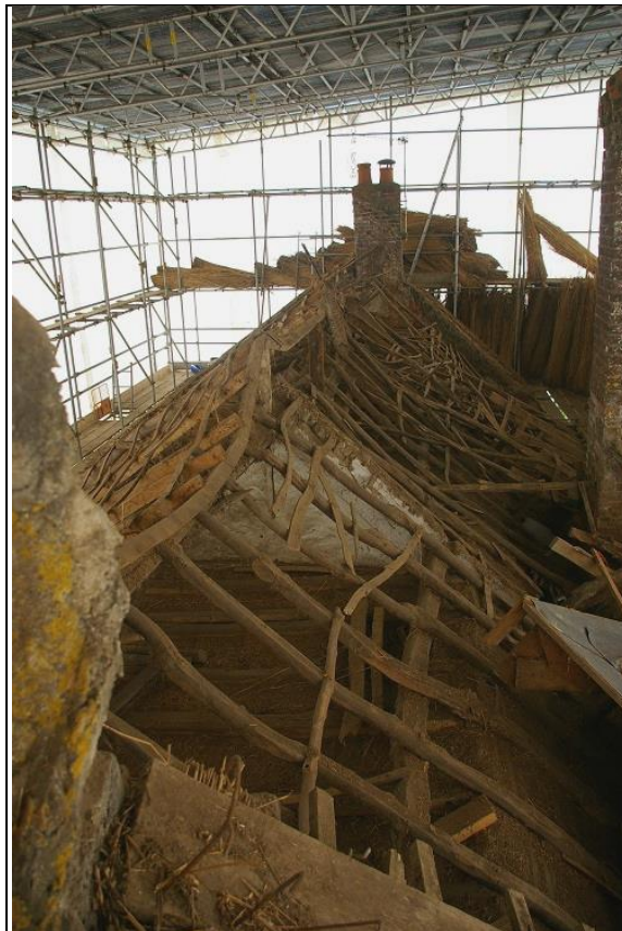
32. WESTACOMBE ROOF STRIPPED OF THATCH, FROM THE EAST END, NORTH SIDE.
