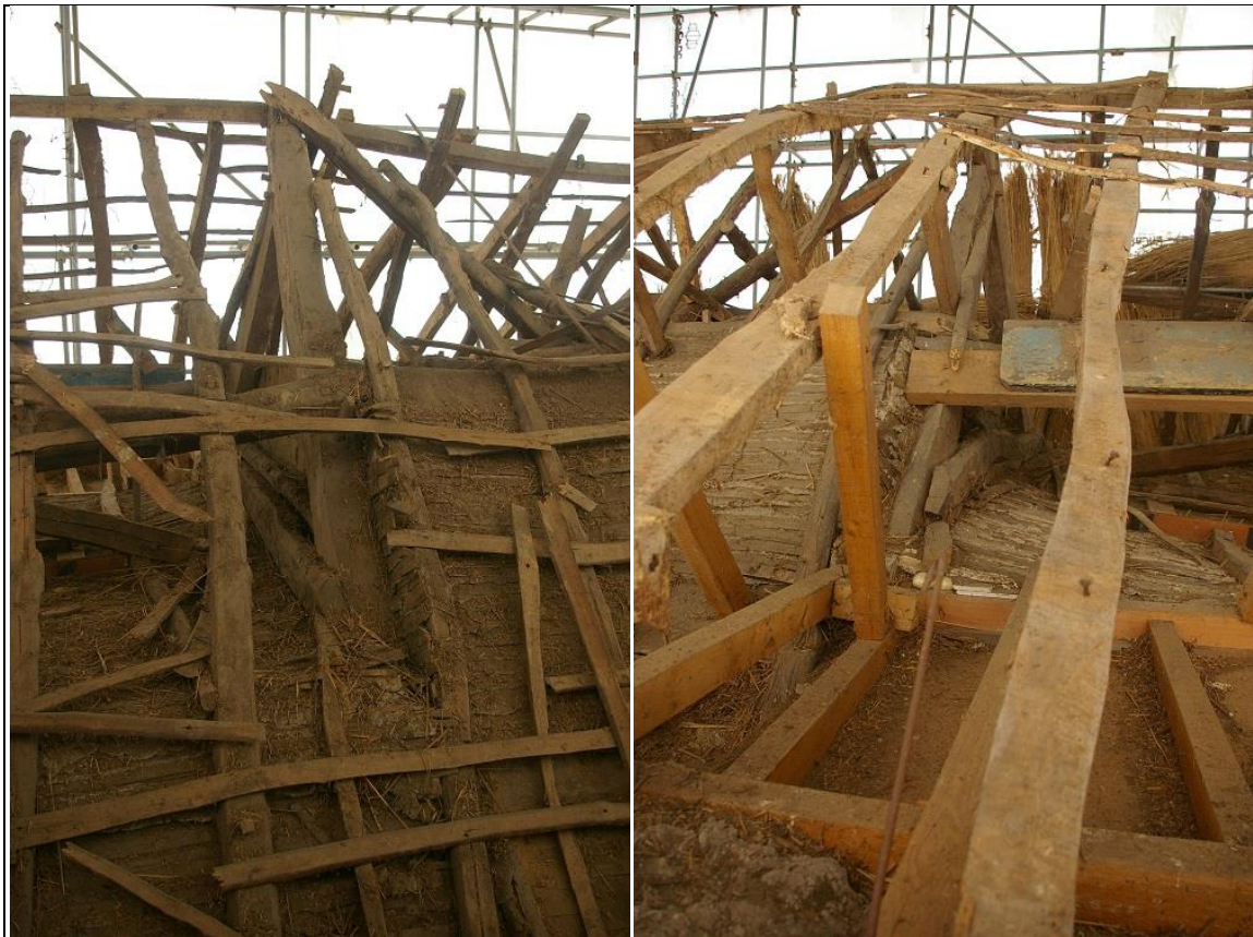
42. LEFT: TRUSS 1 FROM THE NORTH.
