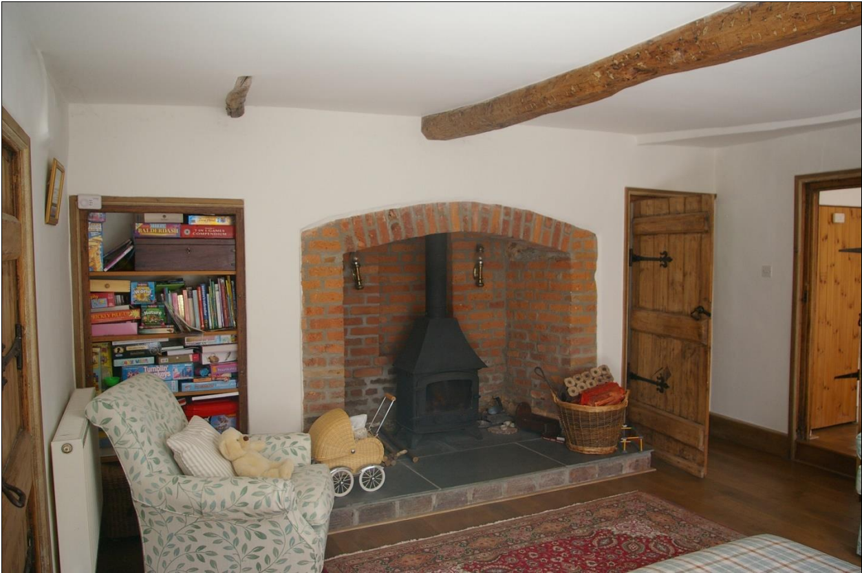
6. THE FORMER HALL, ROOM 3, WITH REMODELLED LATERAL STACK, LATER CEILING BEAM, EARLIER STAIR AND POTENTIAL PLASTERED JETTY; FROM THE SOUTH-WEST.
